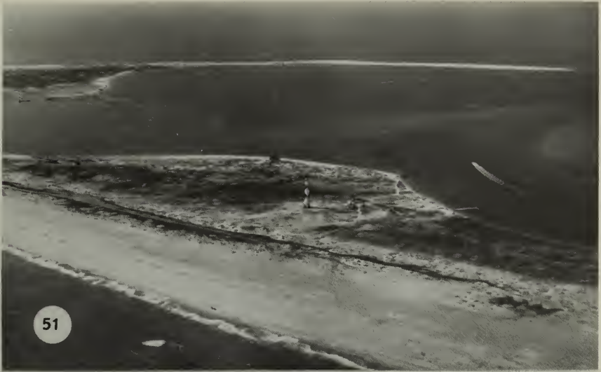
Fig. 51. Cape Lookout Lighthouse, built in 1859, showing the normal wide berm and dune line between the building and the beach. Storm waters are free to move right over the island and no erosion is apparent in the 113 years since the lighthouse was built.
