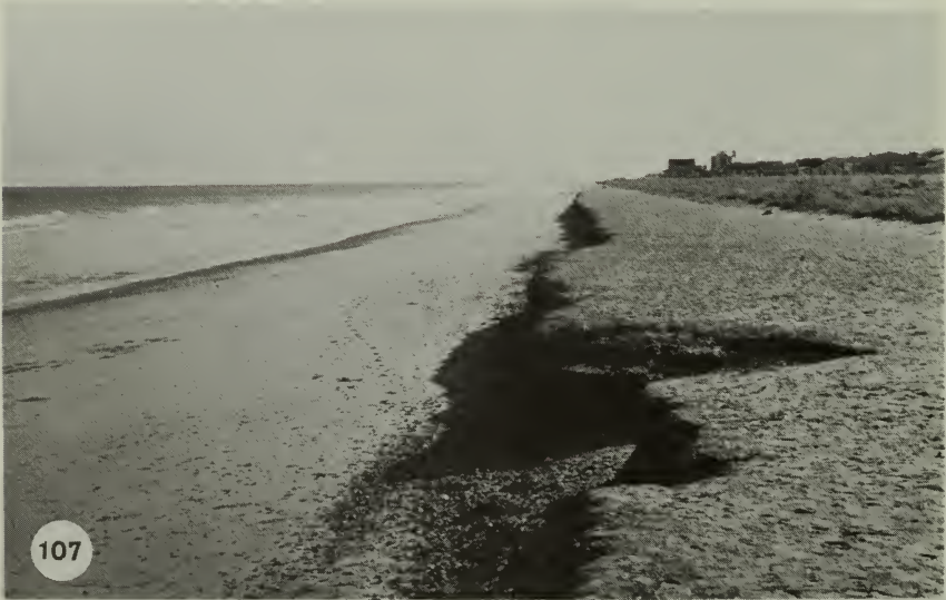
Fig. 107. The eroded scarp typical of beaches artificially built of fine sediment dredged out of the sound.
