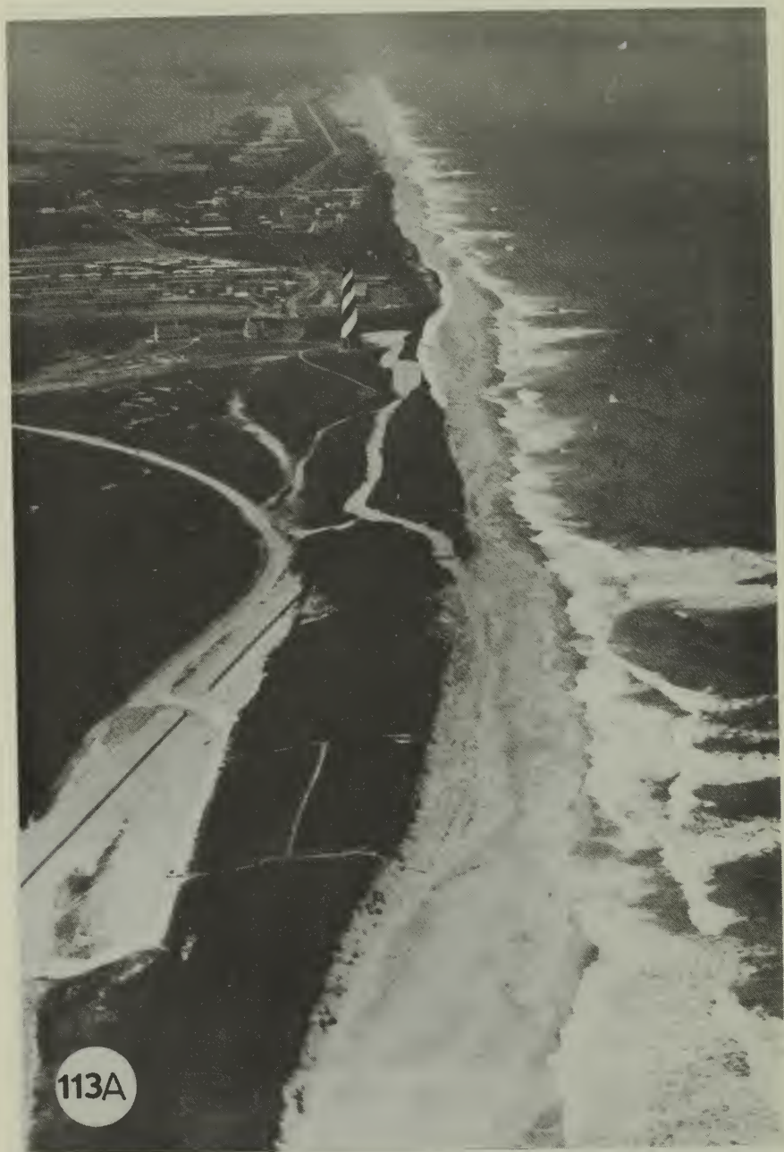
Fig. 113. (A) In 1969, Cape Hatteras Lighthouse and the naval facility just beyond were in serious danger from the sea. The white strip in front of the lighthouse is plastic bags filled with sand. Note the narrowness of the beach, the irregularity of its outer edge, and the artificial dunes in the foreground. (Photo by Cape Hatteras National Seashore.) (B) The ►
