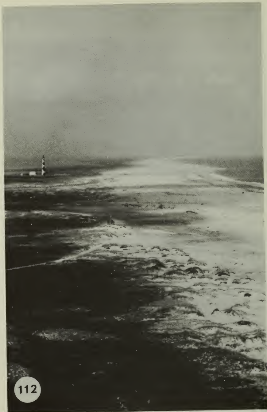
Fig. 112. Cape Lookout Lighthouse. Thirty or forty years ago the Hatteras Lighthouse was separated from the ocean by a similarly wide berm. (Photo by R. Simpson.)
