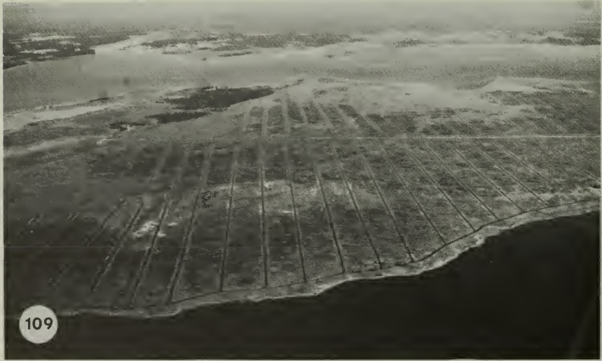
Fig. 109. Salt marsh mosquito ditches in eastern North Carolina. The ditches are 6 ft. (1.8 m) wide, very deep, and built without regard for natural drainage patterns.
