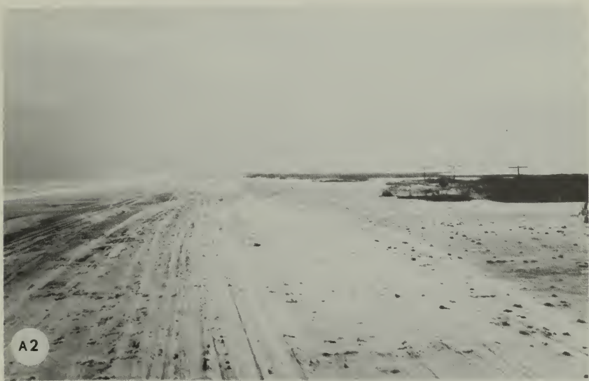
Fig. 29. Effects of Hurricane Ginger on Core Banks, where the storm crossed the Outer Banks causing heavy overwash just south of the Old Atlantic Coast Guard Station. (A1) View looking south of the berm and dune line in June 1971 (photo taken with a wide-angle lens). (A2) The same general area following Hurricane Ginger. The berm crest moved back and edges of the dunes along overwash passes were eroded. Even when the photo was
