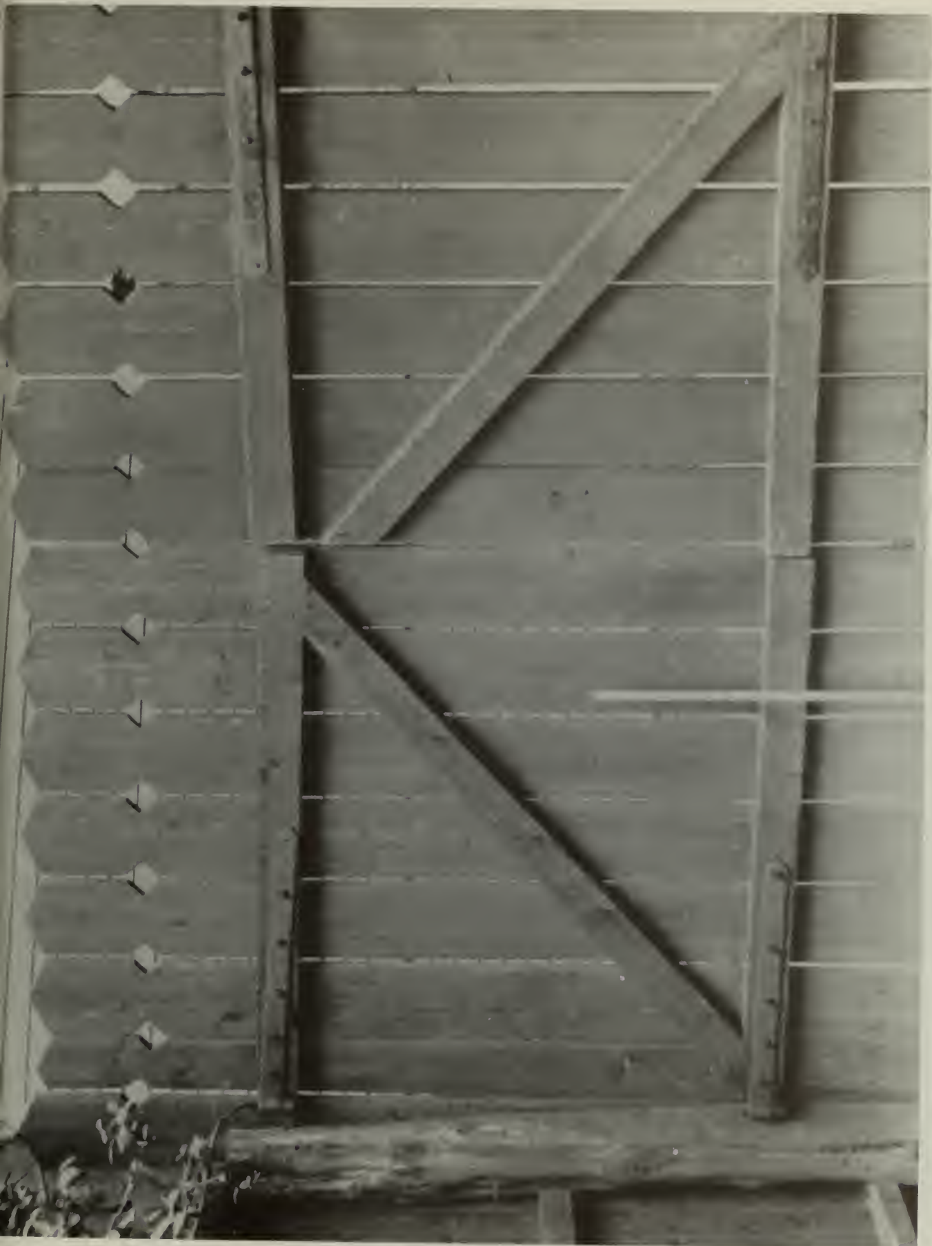
Figure 63. Stockade board fence: gate to wood yard, and spruce pole fence along back driveway, May 31, 1901.
