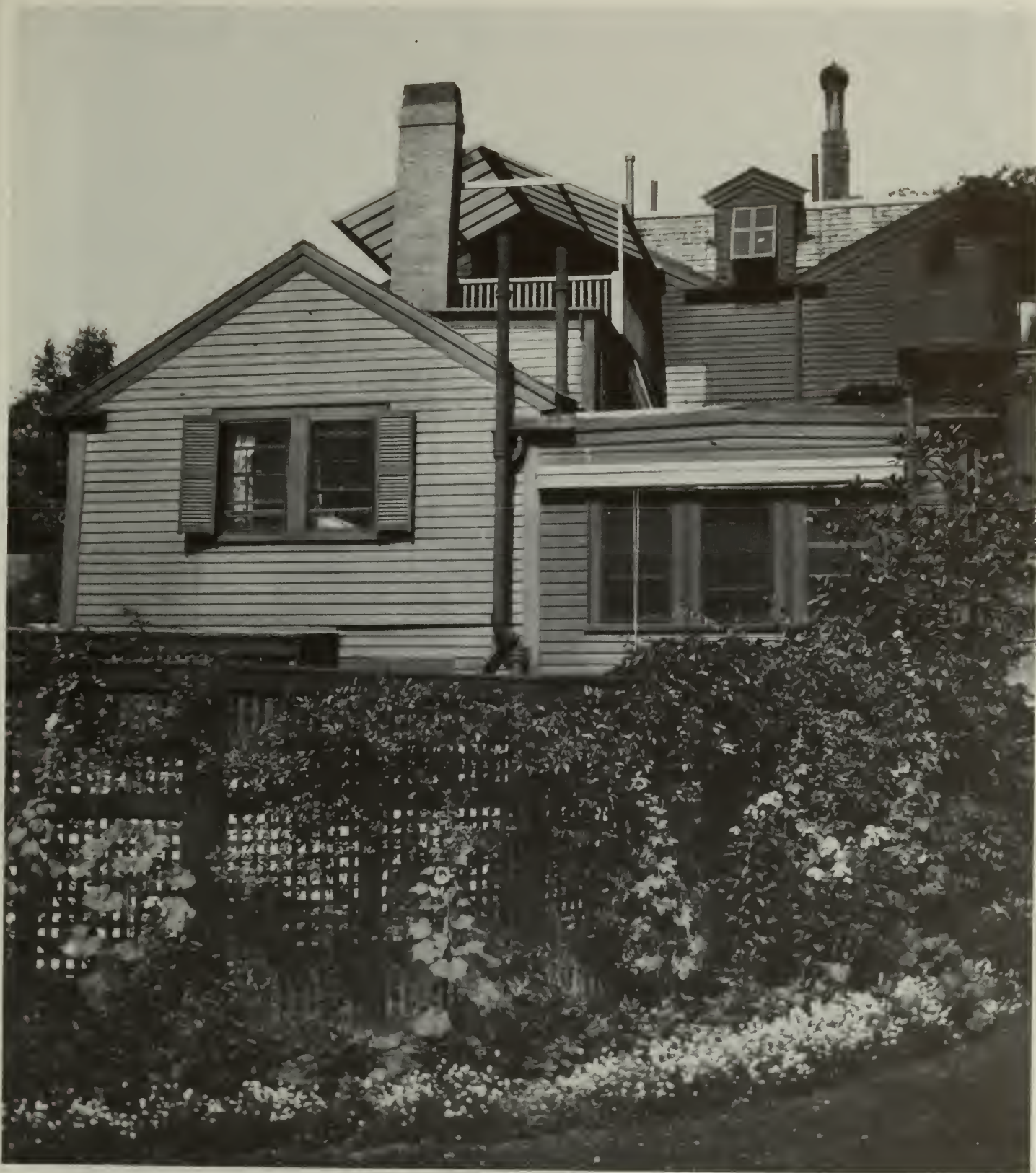
Figure 67. Lattice fence around laundry yard, 1910.
