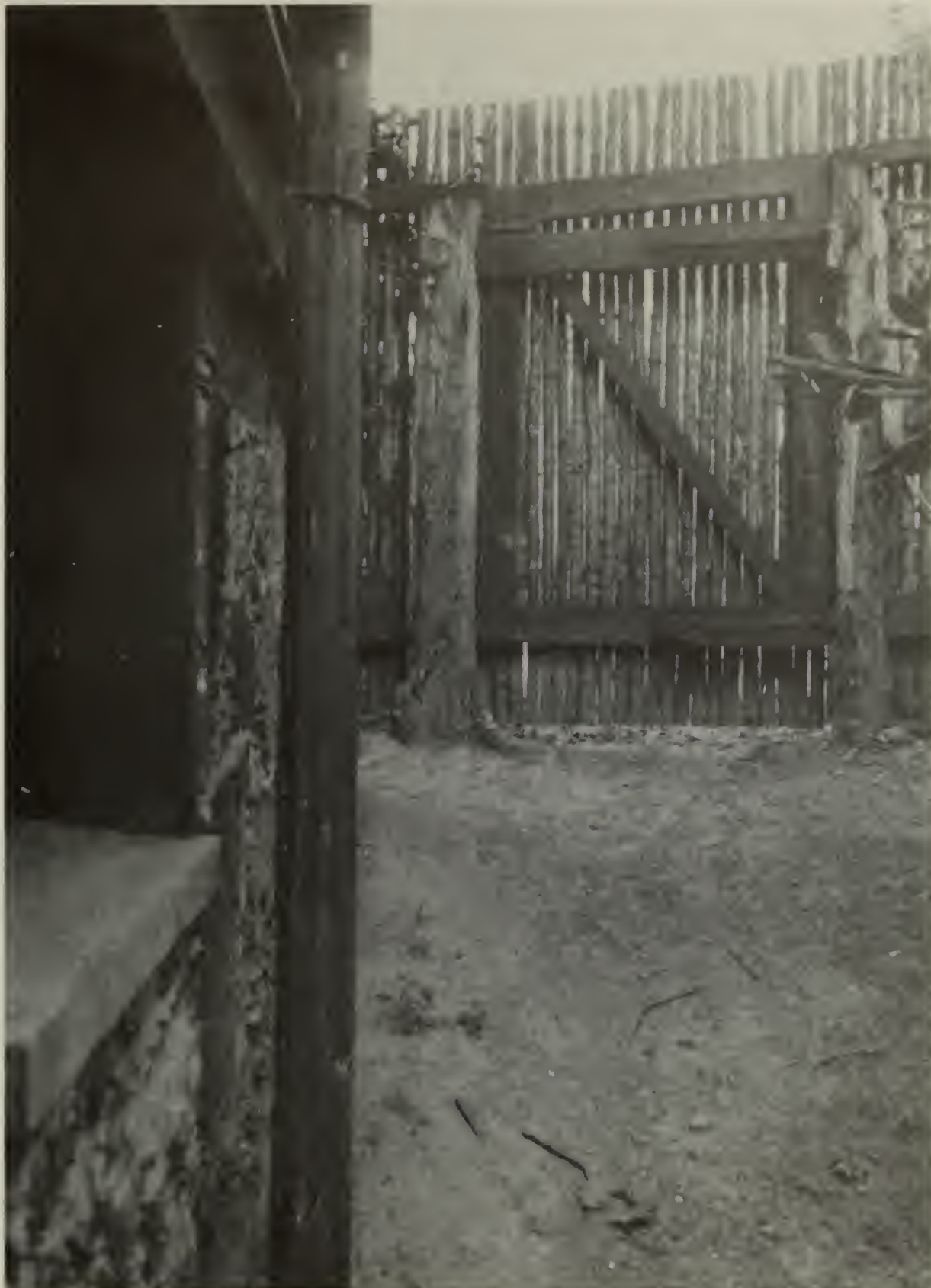
Figure 47. Spruce pole fence: gate at northeast corner of North Drafting Wing, circa 1930.
