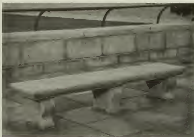
Fig. 38 One of the nine historic benches located on the upper plaza [by author].
