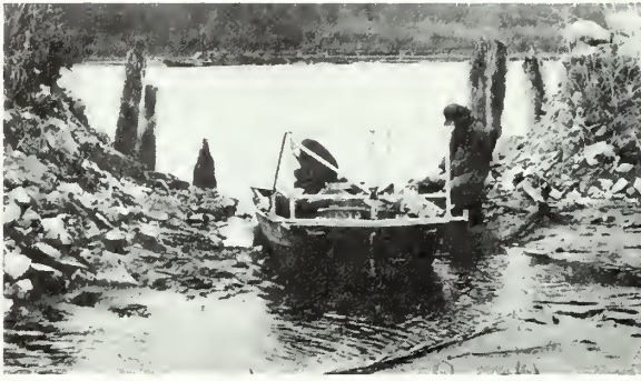
Notches have been cut in rock dikes along the Missouri River to increase diversity of fish habitat and connect backwater areas to the main river channel. Researchers at Iowa Cooperative Fishery Research Unit are conducting a study to determine benefits to the fishery from notch construction. Photo by Ross V. Bulkley.
