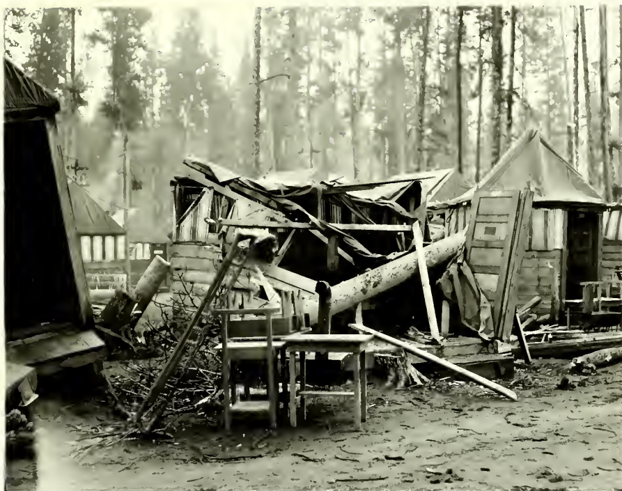
Damage done by windstorm at Fishing Bridge on 7/23/37.
