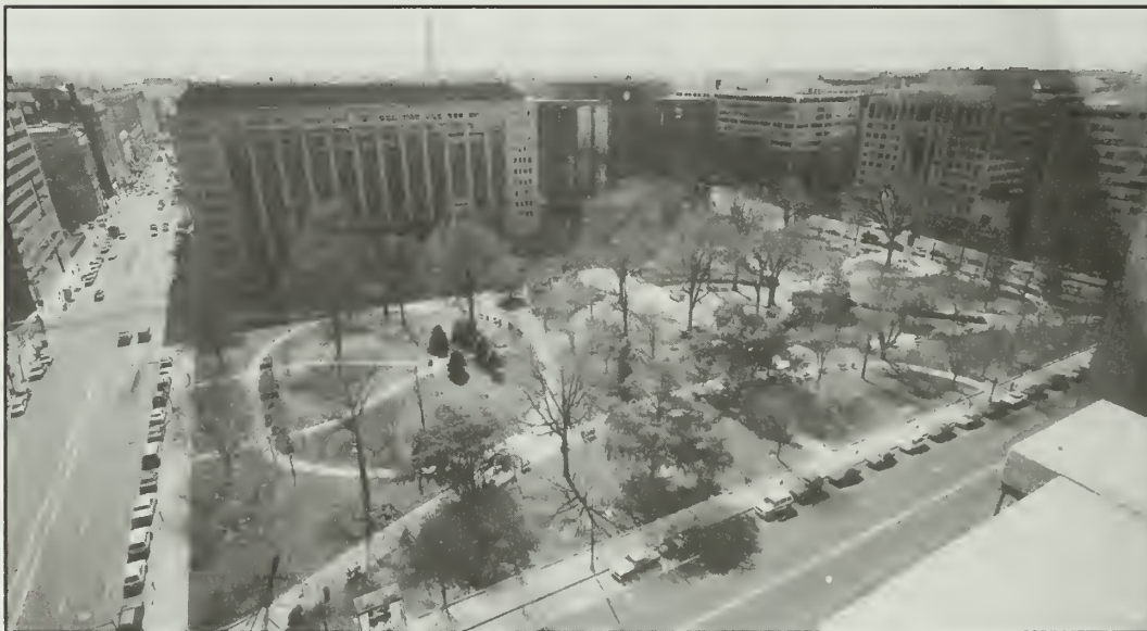
View of Franklin Square, looking southwest from the roof of One Franklin Square on K Street, NW. Photographer: John McWilliams, 1991
