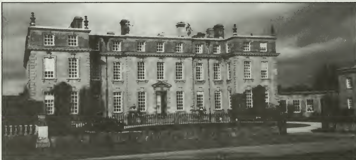
Ditchley House, Oxfordshire, England, c. 1722. James Gibbs, architect. Photographer: Paul D. Dolinsky, 1992
