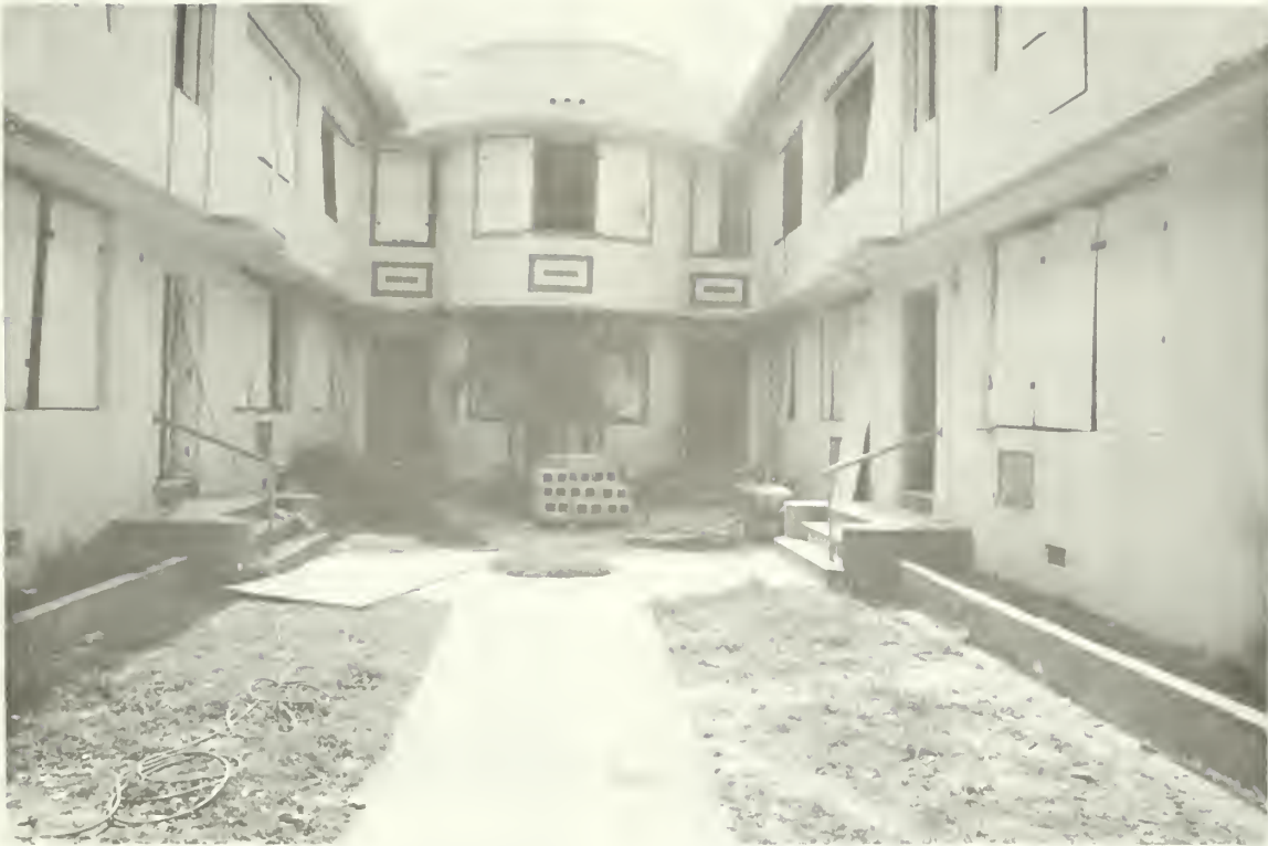
1. The primary entrances to this early 1940s Moderne apartment building are located in the courtyard of the U-shaped structure. Note the overall plainness of the building before rehabilitation, which is highlighted only by horizontal banding and raised geometric panels.
