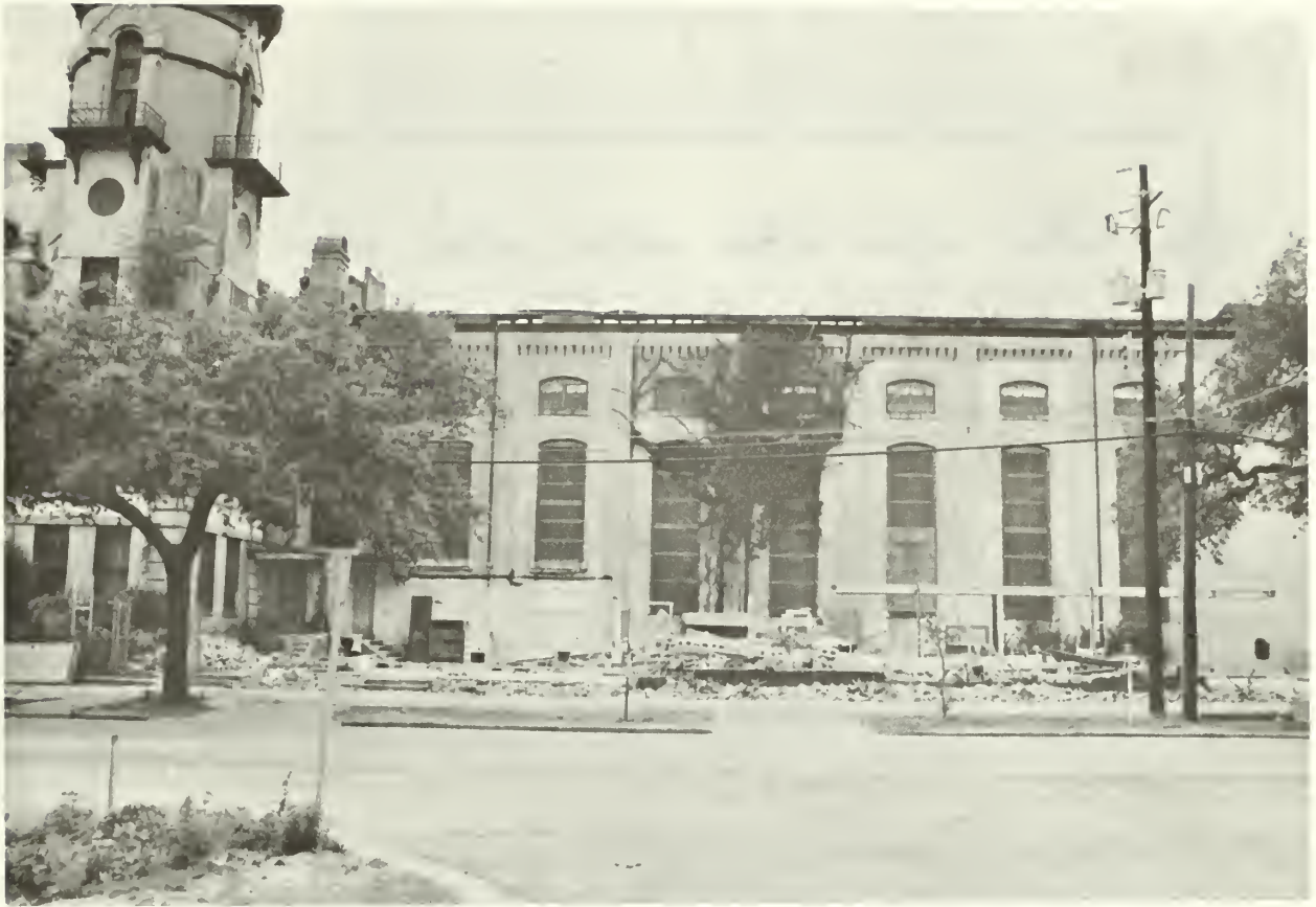
1. The property undergoing rehabilitation consisted of a three-story warden's house (partially visible, left) and a four-story cell block.
