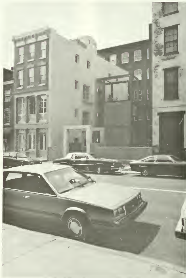
7. The new site work subordinates the independent historic building to a larger composition of radically new and incompatible elements.
