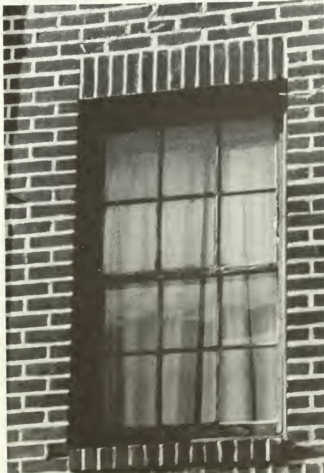
4-5. Pre-rehabilitation views of the deteriorated historic windows. Note beaded mullion above, thin muntins, meeting rails and sash on paired windows and the simple double-hung window below.
