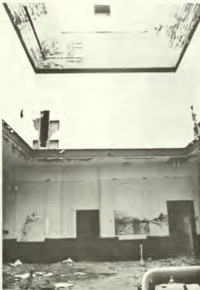
3. View of central space showing atrium extending through the second and third floors, with skylight above. The second floor doors shown lead to rooms beyond. Windows have been blocked in, but their configuration is still apparent from the surrounding trim. On the third floor the open hallway had been partitioned.
