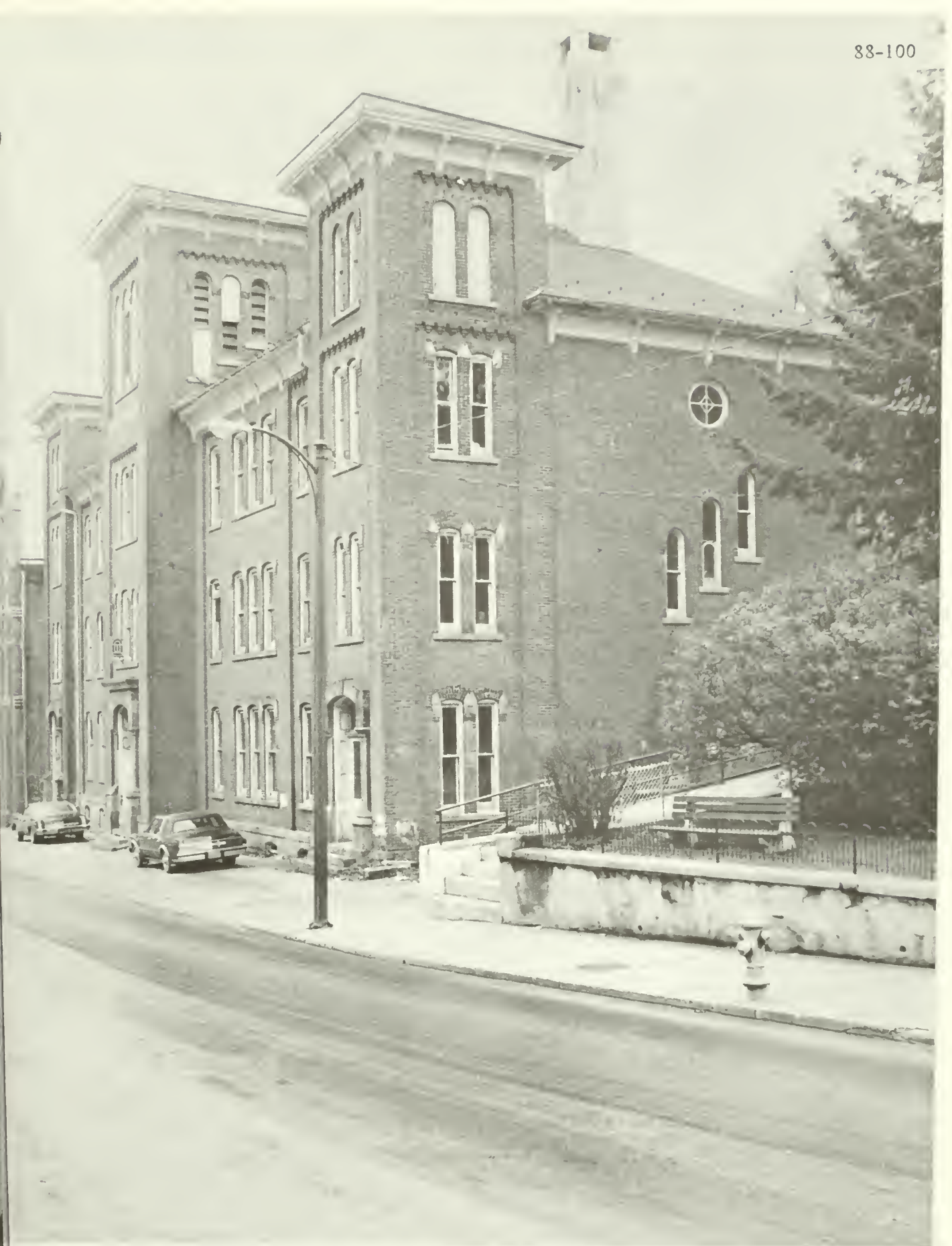
Pre-rehabilitation photograph of school building.
