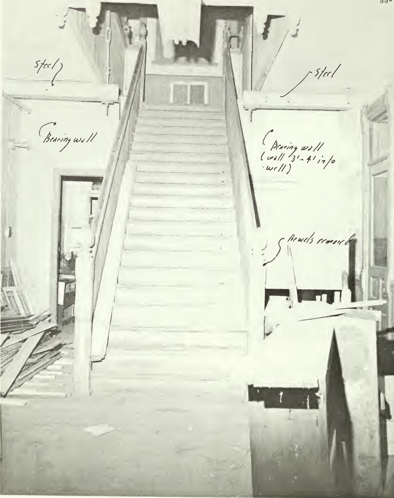
2. Pre-rehabilitation photograph of first floor center stair and hall. This stair was removed in the process of rehabilitation.
