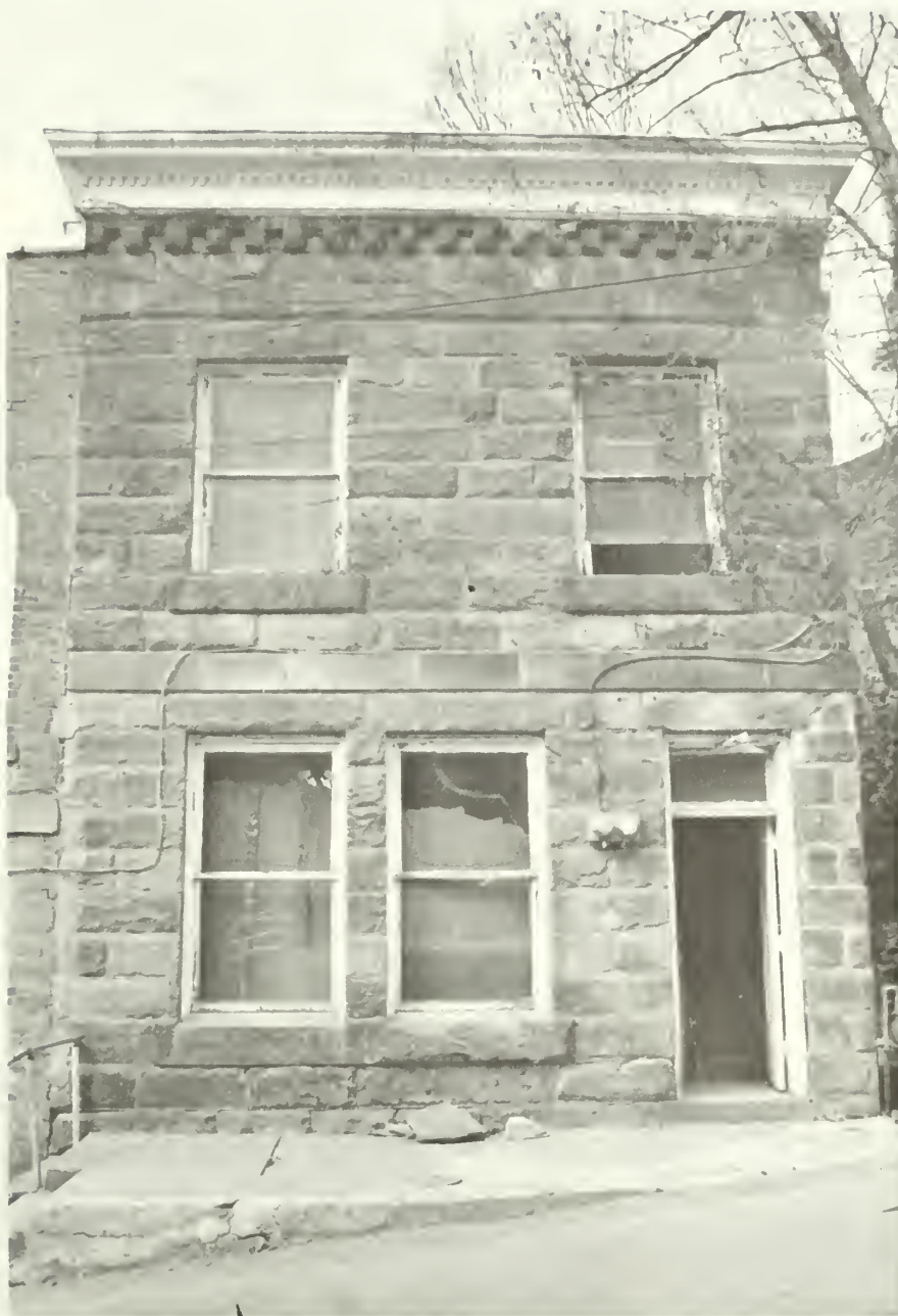
1. This small, semi-detached building was constructed in 1891 as a law office. A narrow walkway to the rear separates the building from the steep hill that abuts it on the right.
