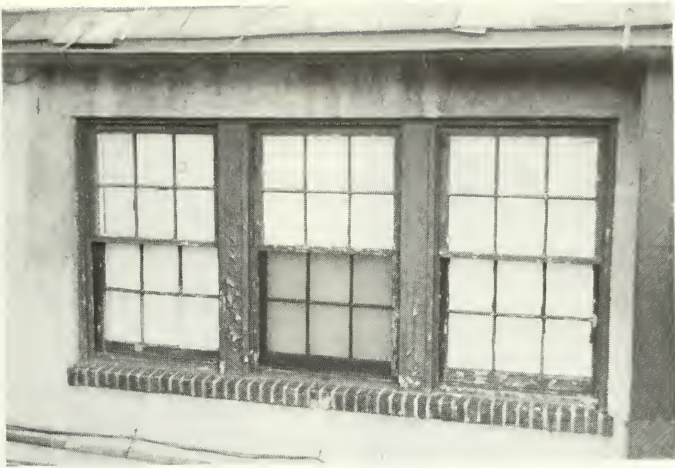
4-5. Pre-rehabilitation views of the deteriorated historic windows. Note beaded mullion above, thin muntins, meeting rails and sash on paired windows and the simple double-hung window below.
