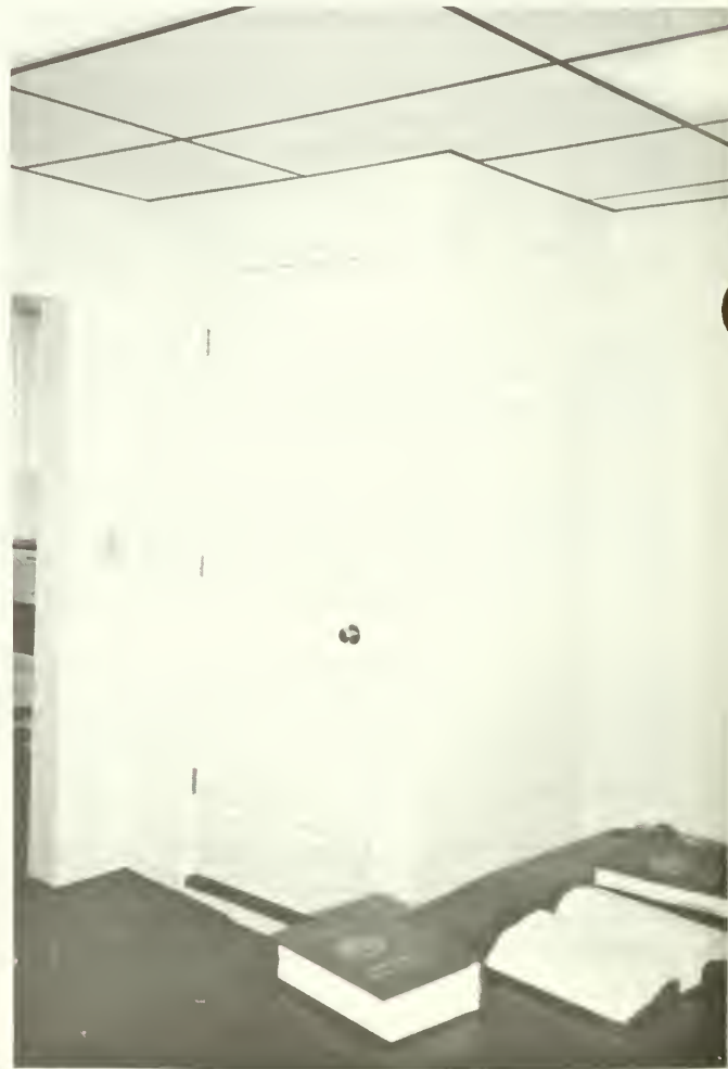
2. This view shows the distracting metal grid and ceiling illumination of the new dropped ceiling.
