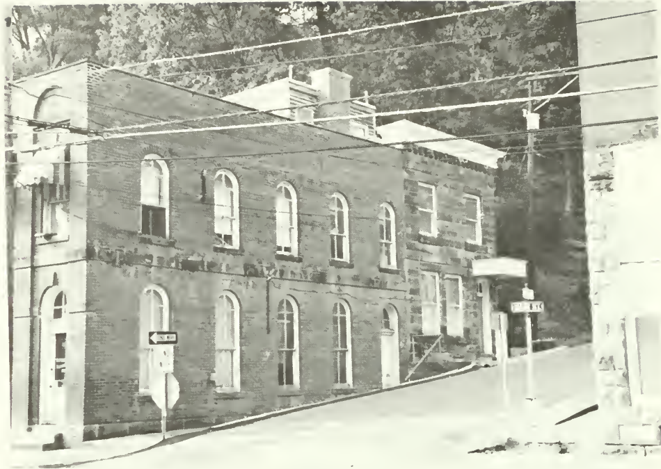
2-3. After rehabilitation, the new rooftop addition is highly visible within the historic district, both from below the building at the main intersection at the foot of the hill, and from above the building higher on the hillside.
