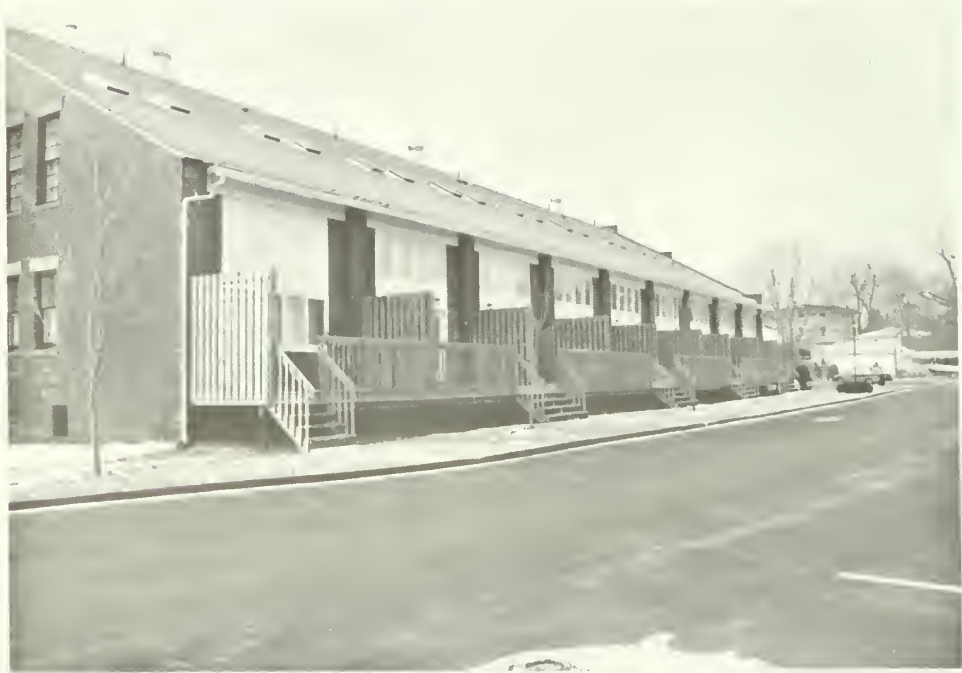
7. The rear of the drill shed showing the completed rehabilitation with the new skylights in the roof, the prefabricated panels filling the former bricked areas, and the new wood decks and privacy fences facing onto a parking lot at the rear of the property.
