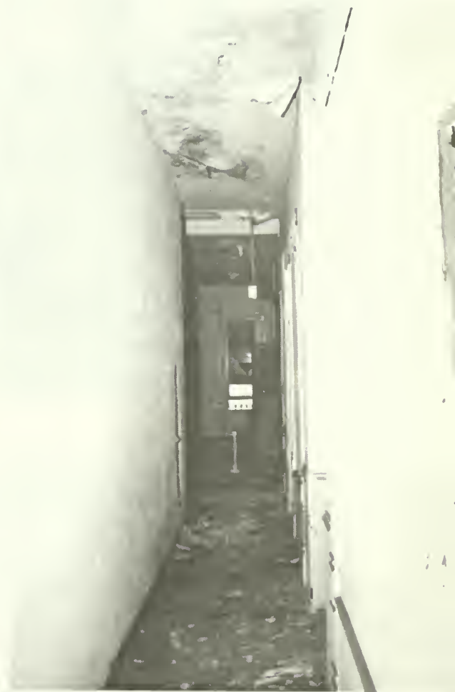
5. On the third floor, the historic hallway, originally open, had been fitted with a solid partition; the offices behind it, however, were relatively unaltered.
