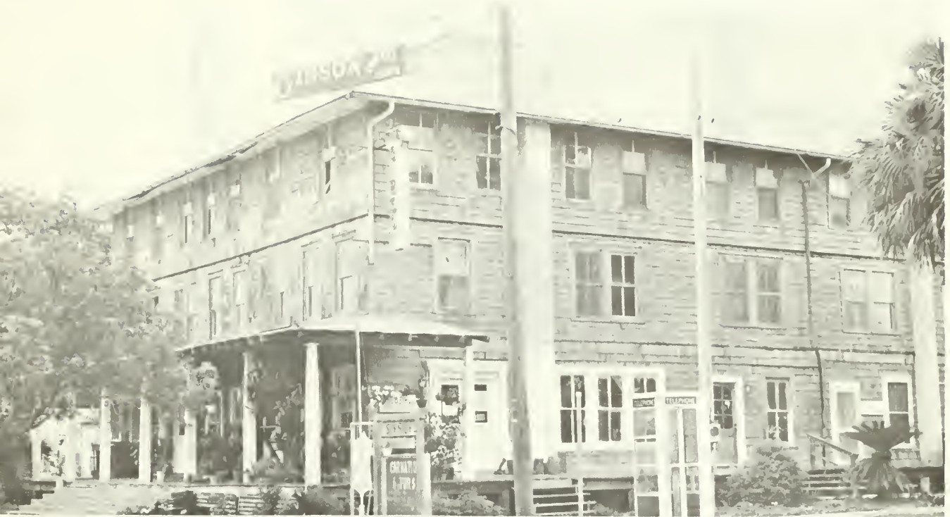
2. The hotel in 1984, prior to rehabilitation. The cupola and dormers are missing, and although a one-story front porch spans the primary elevation, it bears little resemblance to the two-story historic porch shown in the 1907 photograph. The hotel was certified as contributing to the significance of the historic district in its existing condition.
