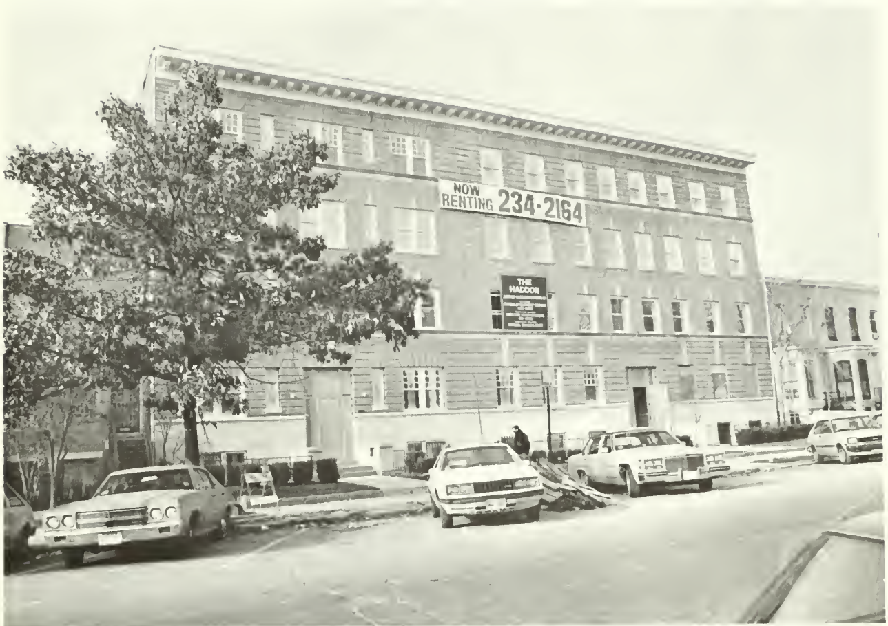
1. This early twentieth century apartment building was actually constructed as two buildings of harmonious but slightly different design.
