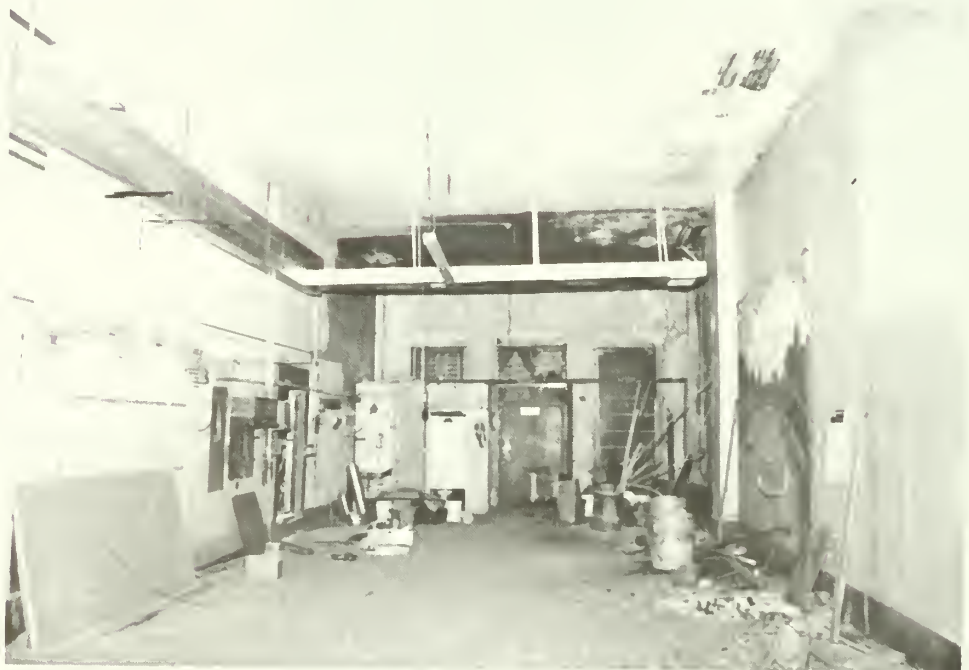
2. Typical ground floor space before rehabilitation.
