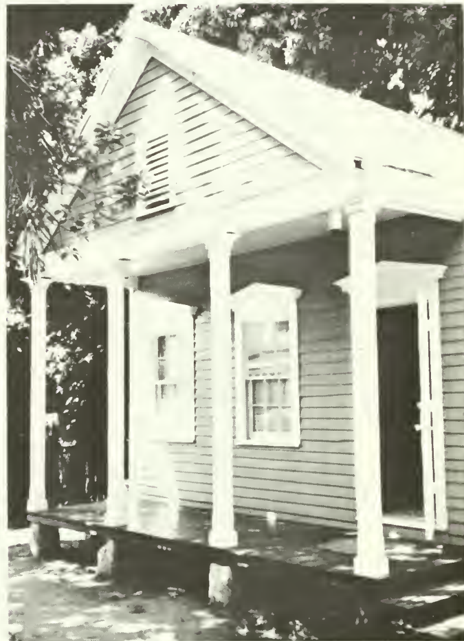
2. The dramatic shift in appearance from a vernacular structure to a higher style building is achieved with Greek Revival posts and triangular window pediments. The building was not originally fitted with these details, nor is there any occurrence of these features on a facade of this size within the district.
