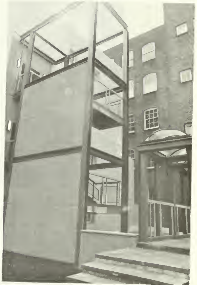
4. Stairtower provides fire exit from building at left.
