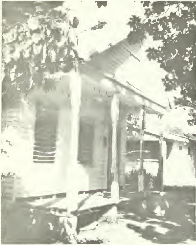
1. Simple turned posts and plain windows were the only expressive details of the vernacular frame building.
