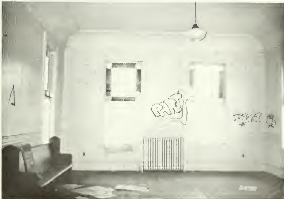
2. Interior view of waiting room prior to rehabilitation. Note wooden ceiling and wide covered cornice.
