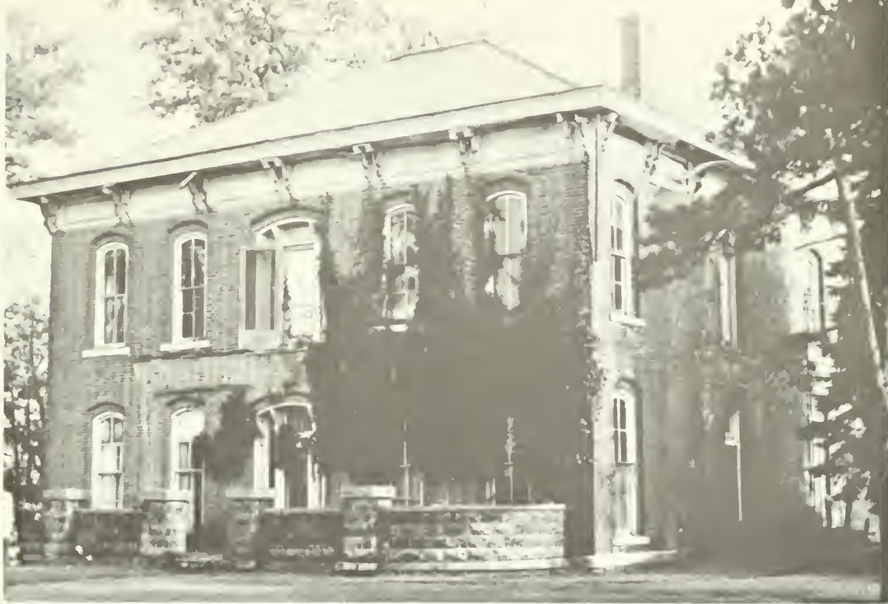
1. The house as it appeared when acquired by the current owner. Note the "ghost" outline of a porch on the front, the second floor exterior doors, and the elliptical cast stone terrace.
