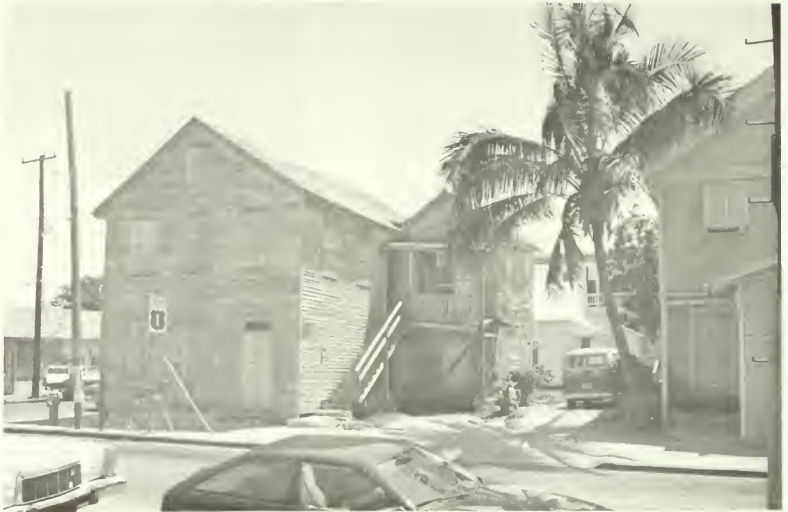
1. This view shows the exterior staircase in place before rehabilitation. Although this staircase was a replacement of the original, the feature was significant because it had remained in the same location and because it announced a separate use and function for the second floor of the ell.
