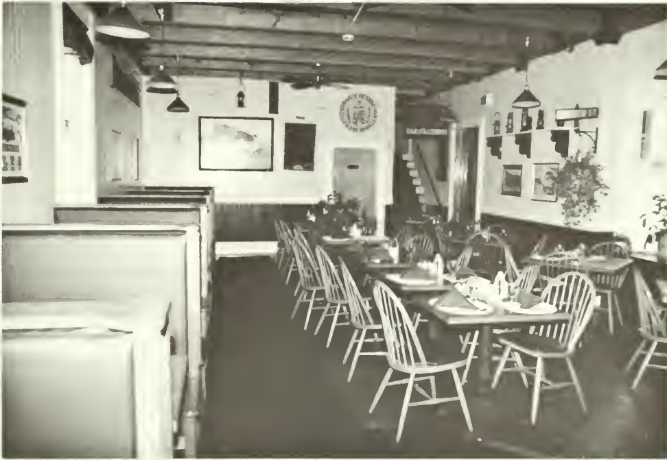
5. Post-rehabilitation view of waiting room. Note the removal of existing ceiling, and the addition of exposed ceiling joists above.
