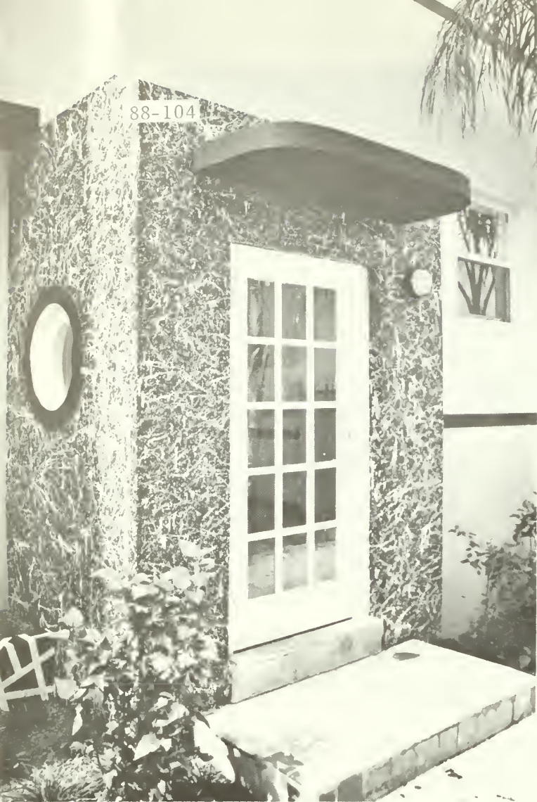
3-5. After rehabilitation the character of the building has been greatly changed by the application of a variety of decorative painted finishes, in particular the "faux" stone surfaces around doors, the contemporary patterned design used above doors and on balconies, and the "cracked tile" pattern on the planters that surround the building.
