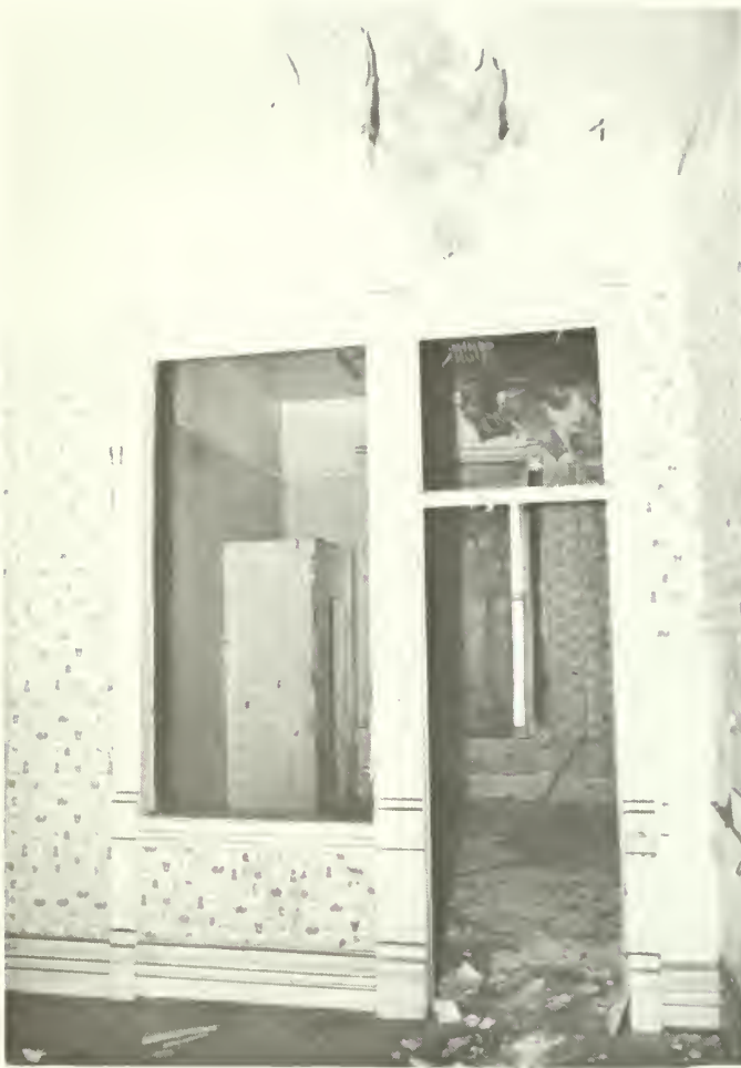
4. Interior rooms were fitted with windows and doors with transoms to borrow light from both the exterior window walls and the rooms facing the lighted atrium.
