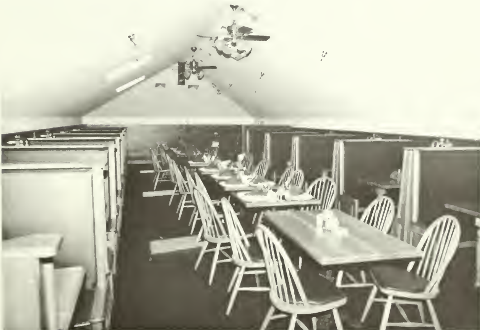
6. Post-rehabilitation view of second floor. Original attic space converted to restaurant space by lowering the ceiling below.
