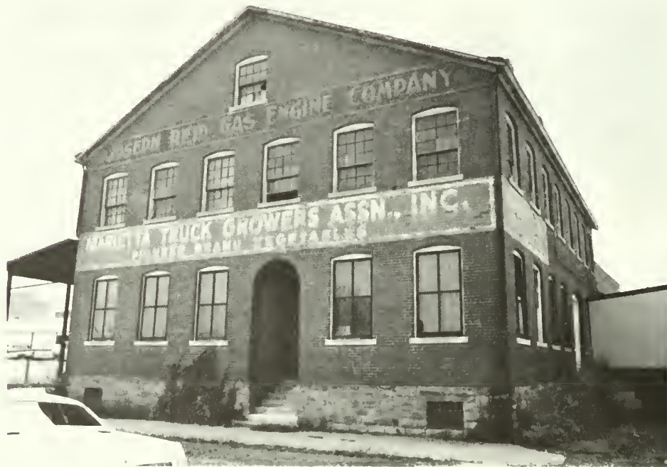
1. Front elevation of the 1880 manufacturing facility as it appeared prior to the rehabilitation.
