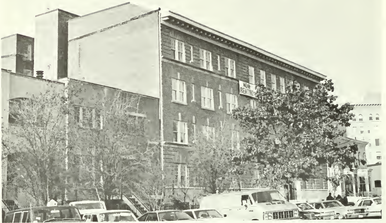
2. New rooftop addition and stairtower visible on the south elevation.
