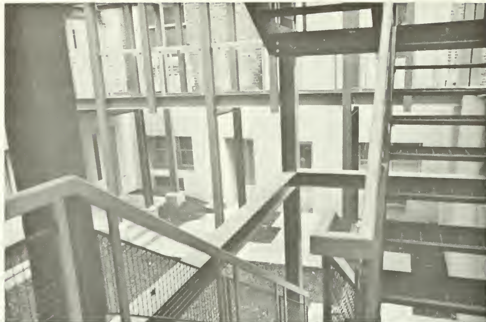
6. The covered walkway spans a courtyard excavated for new below-grade apartments.
