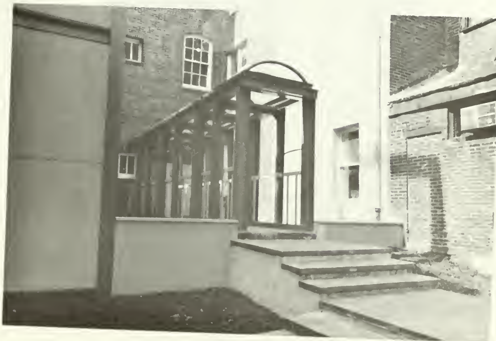
5. Covered walkway serves as the principal entrance to all four rehabilitated structures.
