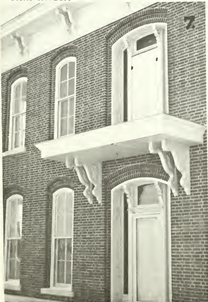
2-3. The reconstructed front porch (left) and the side porch (right). Their designs were based on bracket fragments found on the property combined with area residents' descriptions of the porches as they remembered them, but did not match the "ghost" outlines that had existed on the brick prior to cleaning.
