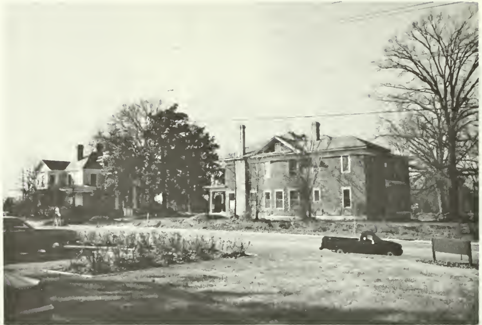
5. Turned 180 degrees, the moved building faces the historic one from a distance of 60 feet.
