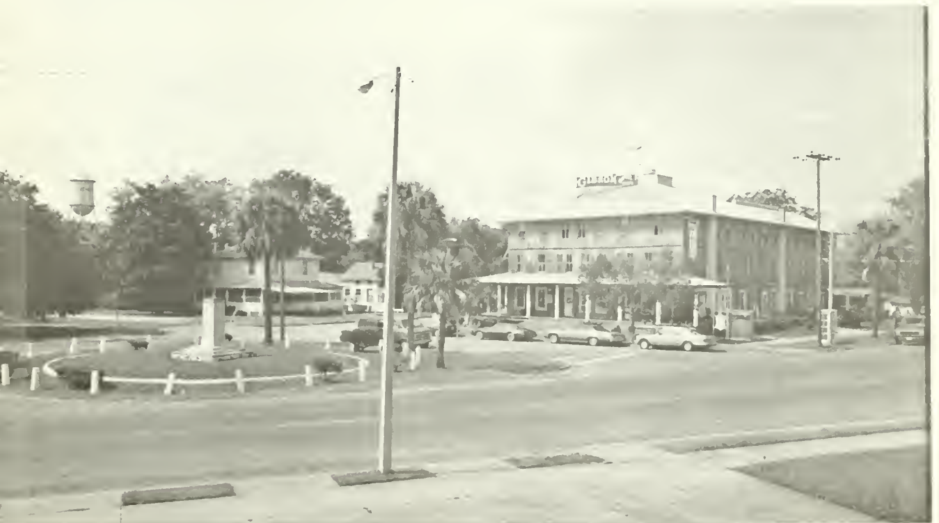
2. The hotel in 1984, prior to rehabilitation. The cupola and dormers are missing, and although a one-story front porch spans the primary elevation, it bears little resemblance to the two-story historic porch shown in the 1907 photograph. The hotel was certified as contributing to the significance of the historic district in its existing condition.
