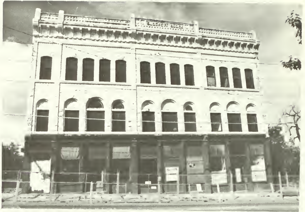
1. 1890 commercial building prior to rehabilitation.
