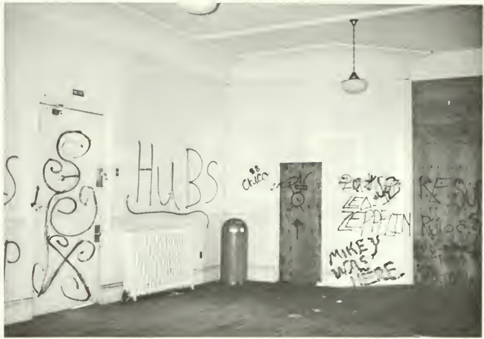
3. Interior view of ticket booth prior to rehabilitation. This historic feature was removed in the process of rehabilitation.
