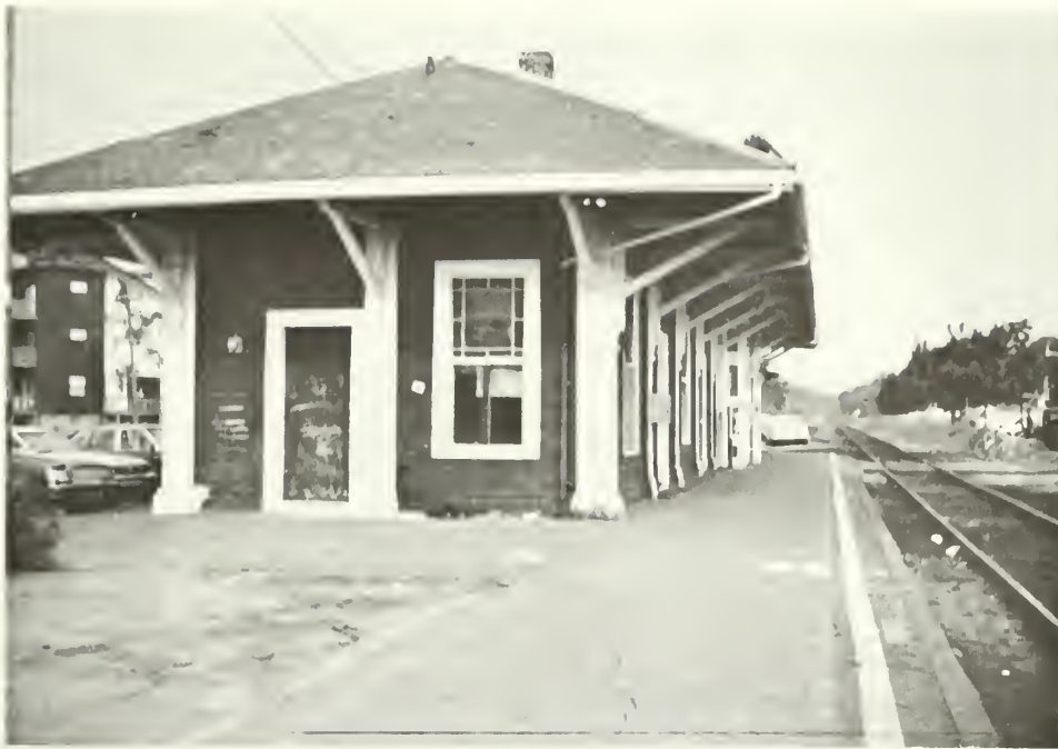
1. Railroad depot prior to rehabilitation.
