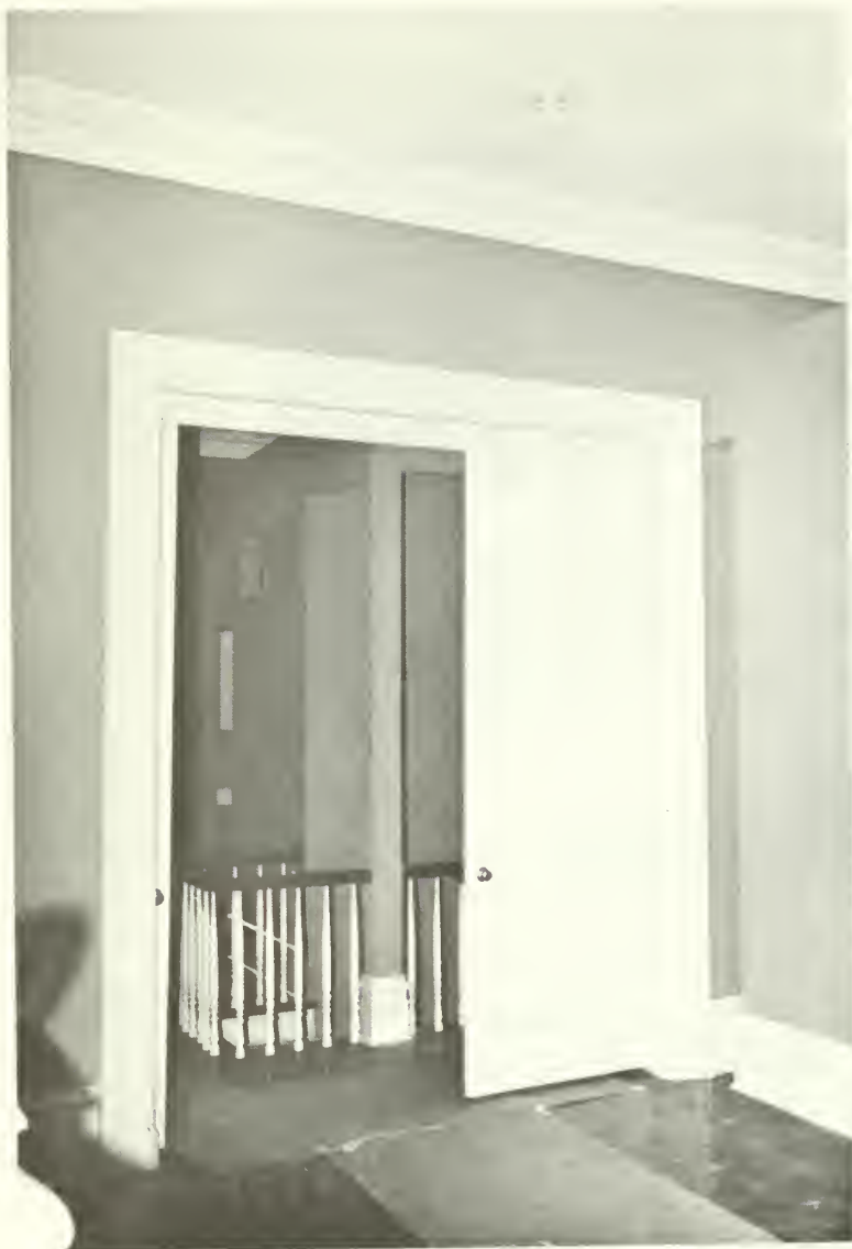
5. Post-rehabilitation: 2nd floor. Note new staircase and partition in center parlor room, new freestanding partition to the right of parlor door in front room.
