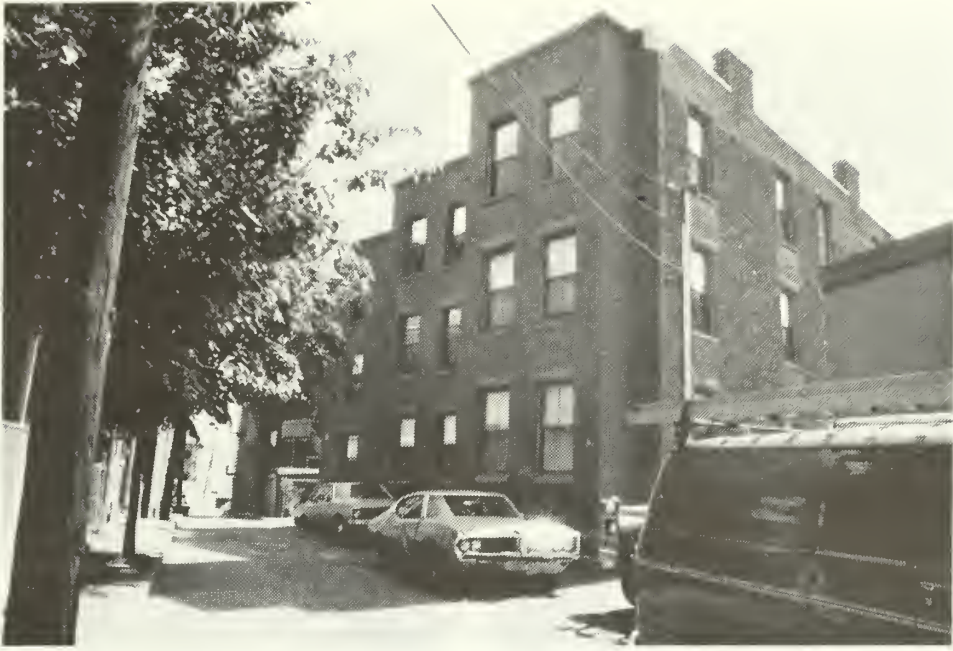
1. Pre-rehabilitation photograph of workers' rowhouses (front elevation).
