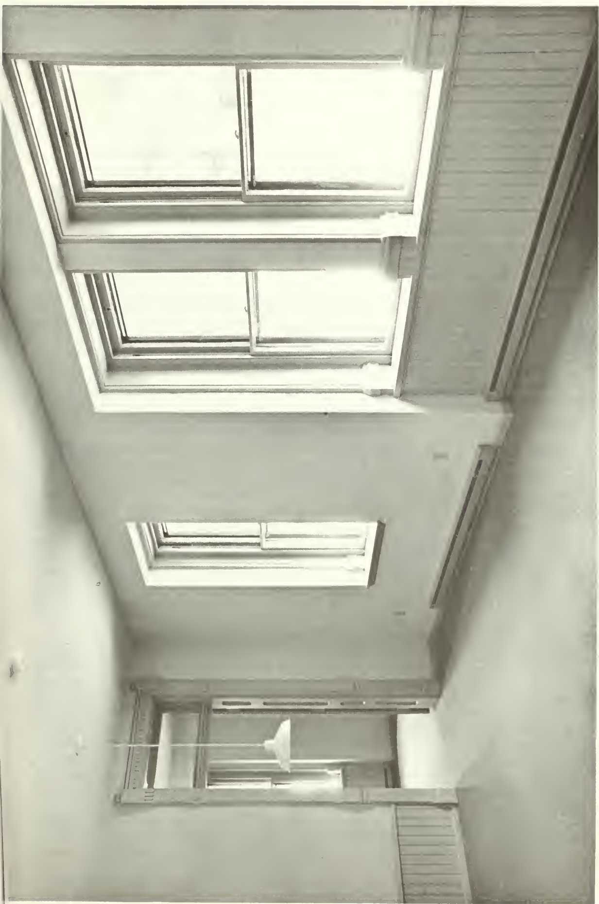
6. Third floor classroom as modified for apartments in rehabilitation.
