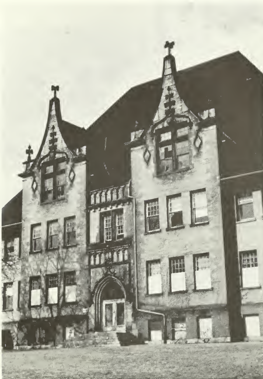
1. The former school building is characterized by its distinctive form--massive yet only three stories in height--its twin towers, unusual arch-shaped entrance and series of large-scale, twelve-over-one windows that were designed to provide maximum daylight in the classrooms.
