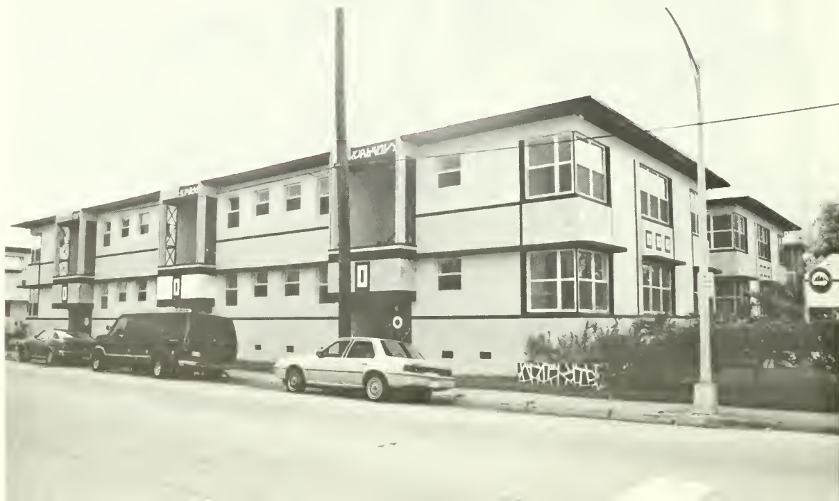
3-5. After rehabilitation the character of the building has been greatly changed by the application of a variety of decorative painted finishes, in particular the "faux" stone surfaces around doors, the contemporary patterned design used above doors and on balconies, and the "cracked tile" pattern on the planters that surround the building.
