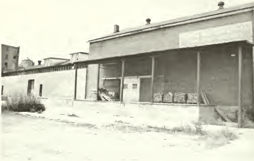
2. South side elevation of the building with roof-covered loading dock prior to rehabilitation.
