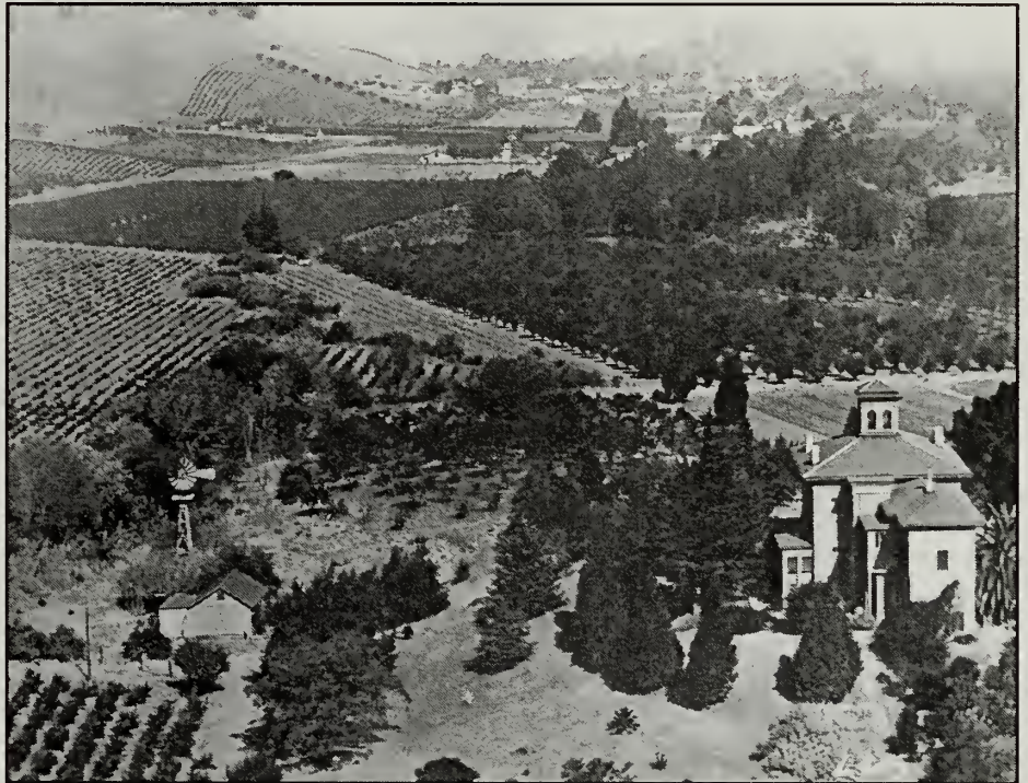
Figure 2.10: View taken c.1910 from Mt. Wanda looking north at the Muir House and towards the town of Martinez and the Straits of Carquinez. (A1-19, JOMU, Ref: 1910-14cP27. Same as Figure 3.15 in Volume 1 of the CLR).
