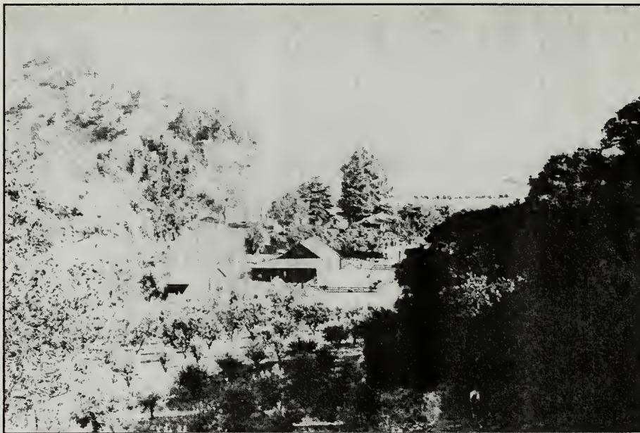
Figure 2.20: This photograph, taken c.1901 from a hillside south of Franklin Creek, is the only known picture of the outbuildings and orchards south of the Martinez Adobe. The Ranch Foreman's House can be seen next to the adobe. (From "Historic Structures Report, Martinez Adobe, John Muir National Historic Site, California." Same as Figure 3.10 in Volume 1 of the CLR).
