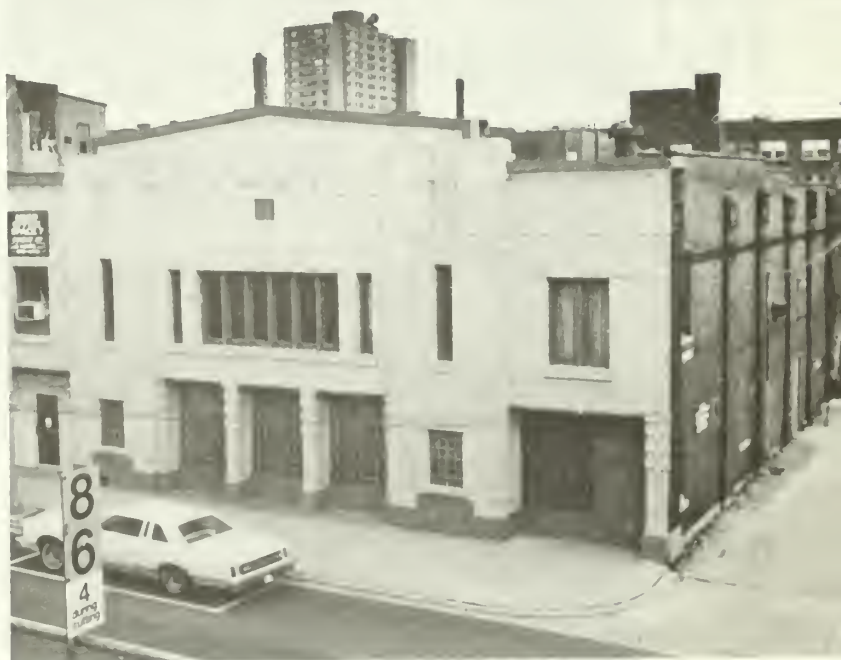
5. Theatre building as it appeared at the commencement of rehabilitation. The wooden doors had been removed in an earlier "renovation" and the openings filled-in with glass block. In addition, the masonry was painted a uniform gray. The stone sills cover a 22-inch-thick concrete floor inside.
