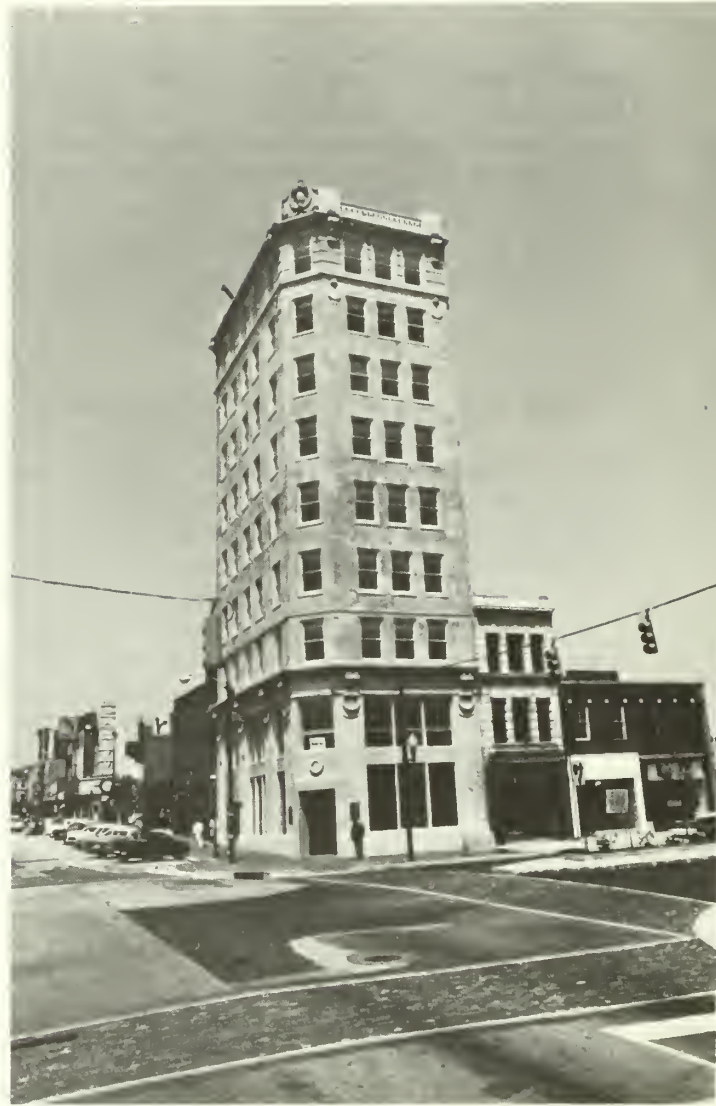
2. Office building after chemical cleaning showing splotchy and discolored brick.
