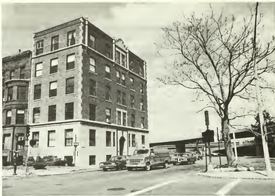
1. This 20th century building served as an anchor at the end of the small historic district and had three highly visible facades. Note how the location, design, and even the color of the wooden sash and frames matched that of the adjacent older properties.
