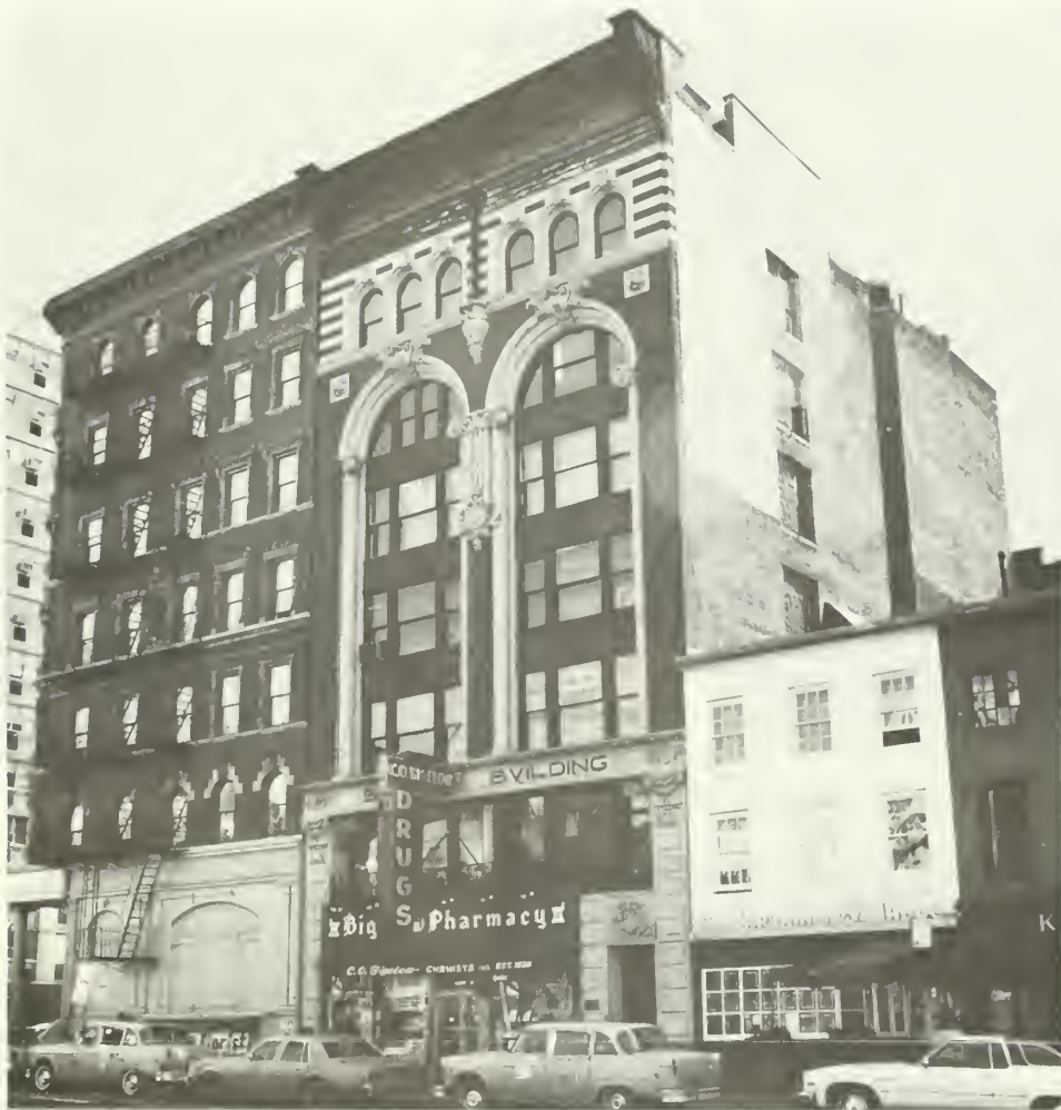
1. Rehabilitation project work on an early 20th century building focused upon meeting health and safety code requirements for the new use.
