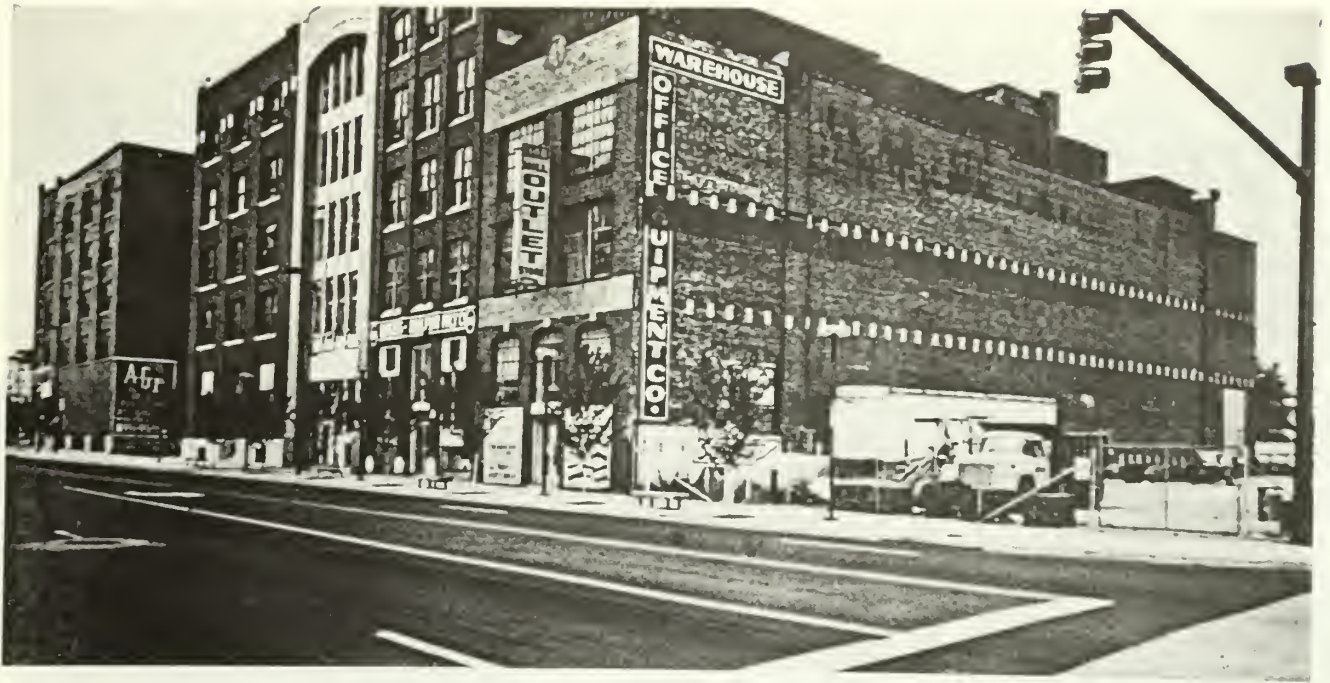
2. This view of a portion of the historic district is looking north. Note the road which divides the district into two blocks. This is the site of the proposed new addition and "pedway."
