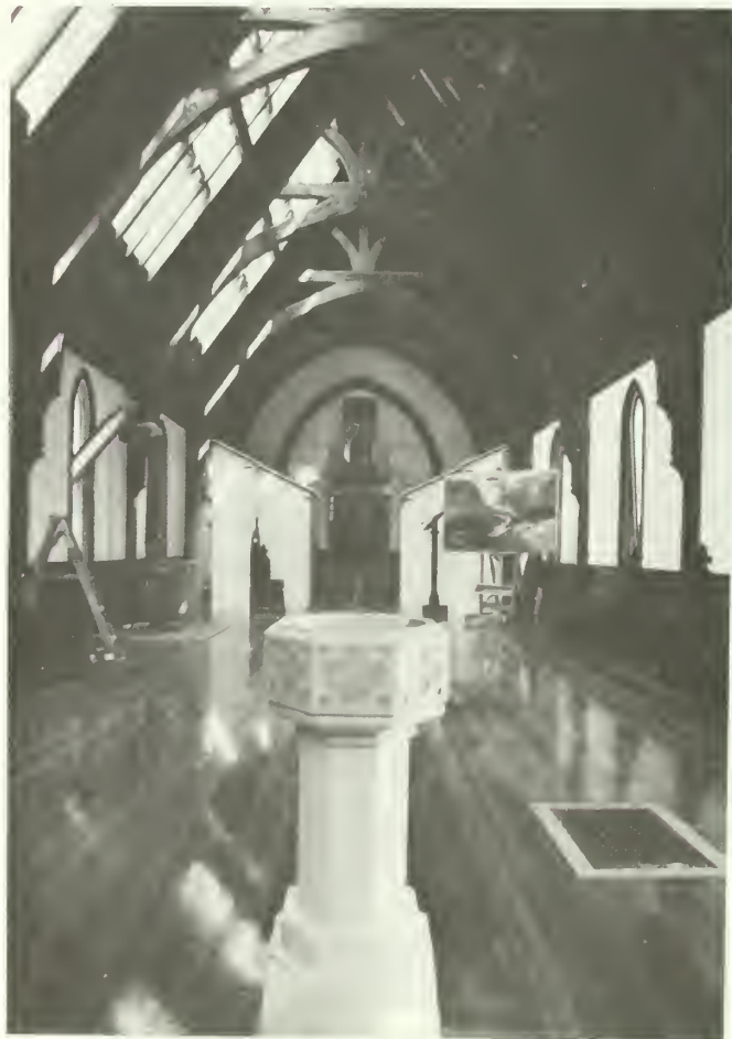
6. View of nave looking east. Note the 2 new sheds in front of and on either side of spiral stairs in center of sanctuary arch leading to mezzanine.
