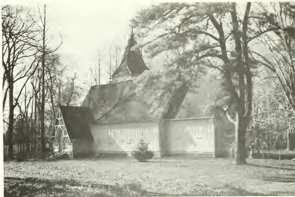
1. South elevation of church before rehabilitation.
