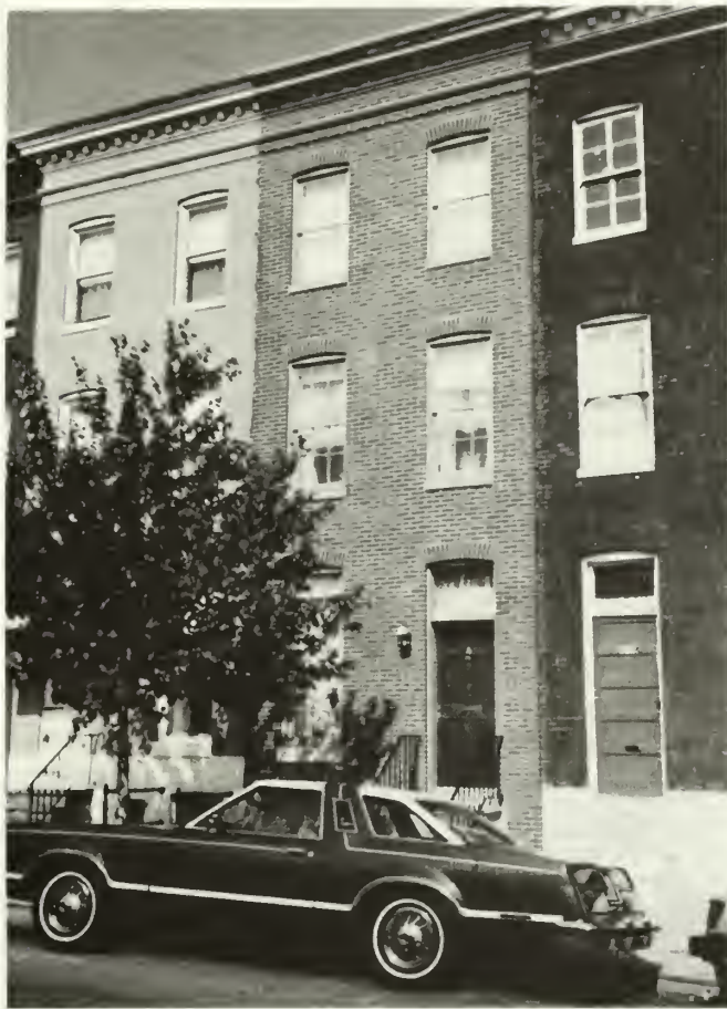
3. Brick rowhouse in center after paint removal using sodium hydroxide stands out conspicuously from its still painted neighbors.
