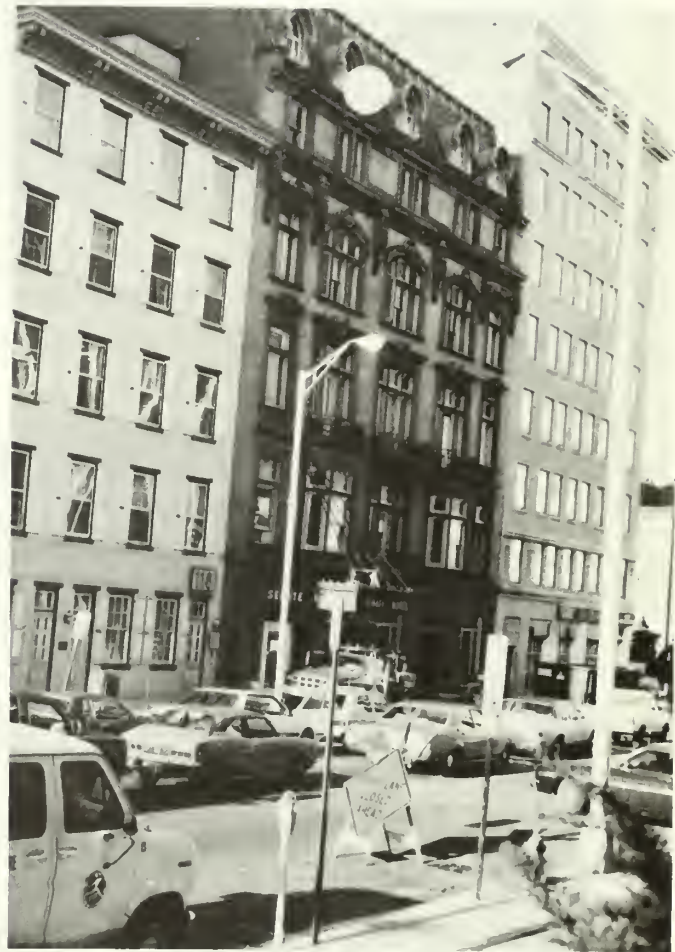
2. During rehabilitation into an office building the first floor is being reconstructed according to the original architectural drawings.
