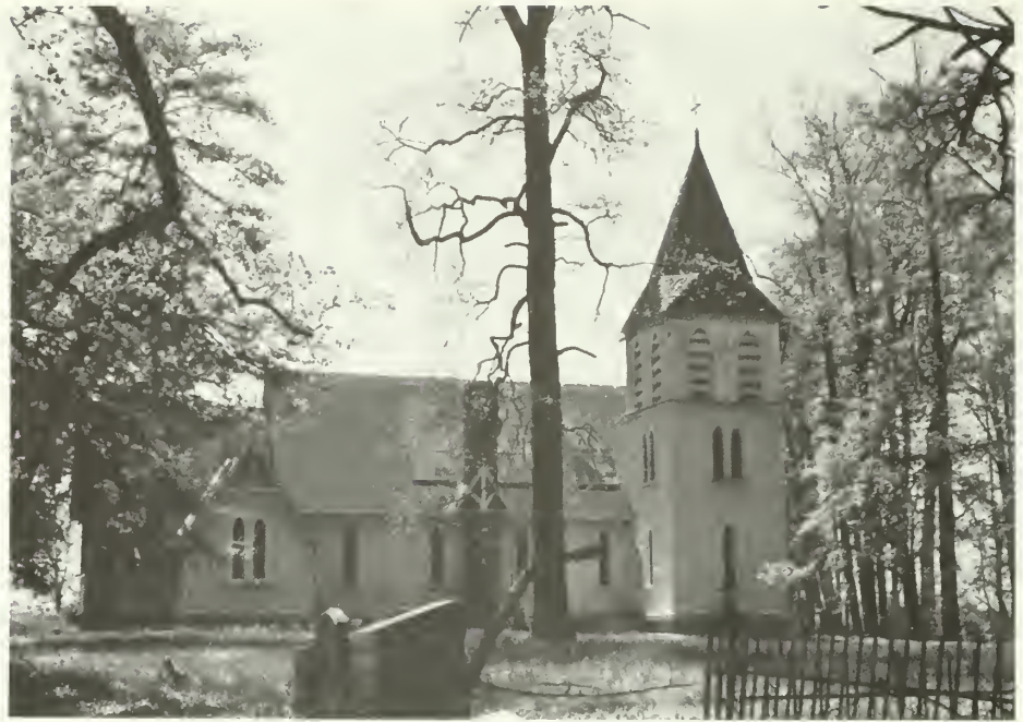
5. North elevation showing new skylights inserted in nave roof after rehabilitation.
