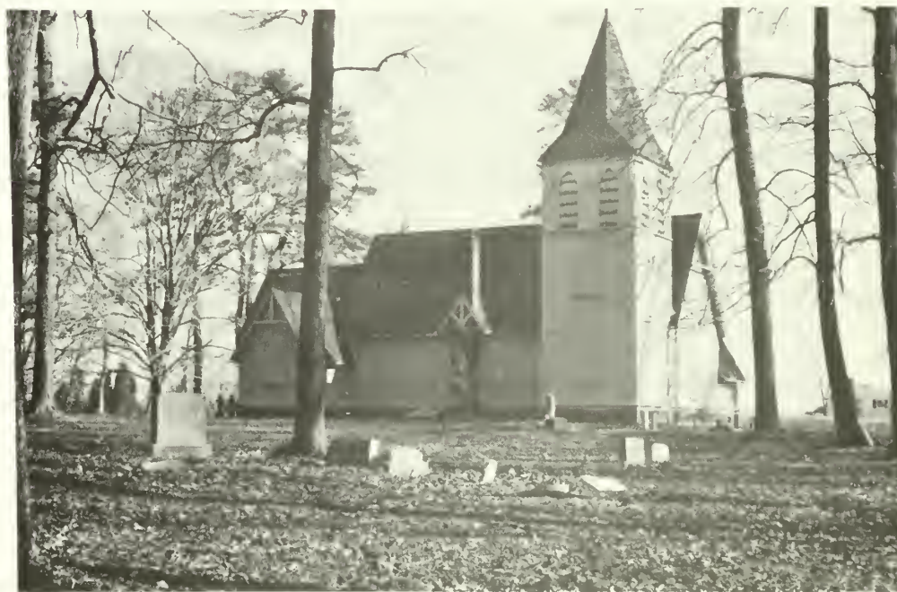
2. North elevation of church before rehabilitation.
