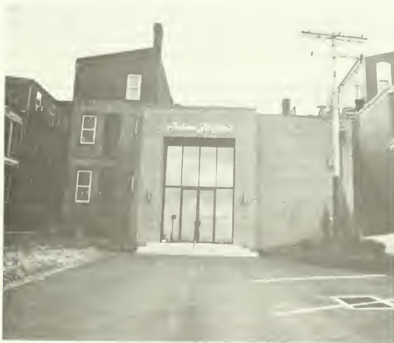
3. Completed work, rear elevation. The project was denied, largely based on demolition of the rear wing and porch and construction of a large addition that changed both the exterior form and interior plan.
