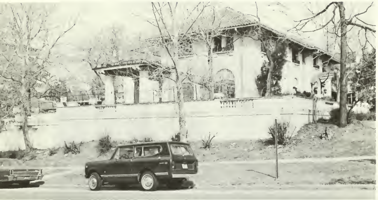
1. Side view of the house, showing the retaining wall around the site and the front terrace.
