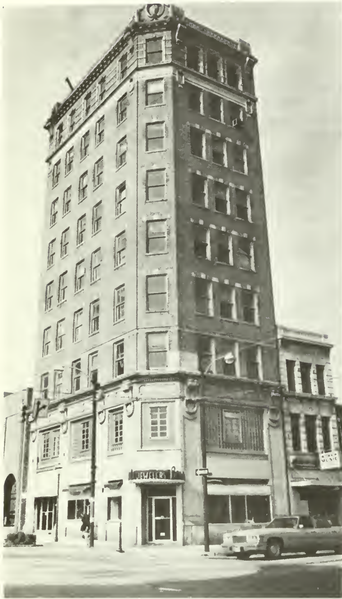
1. Nine story bank and office building before rehabilitation. Note uniformity of brick color.
