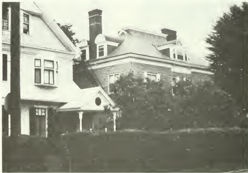
6. The building is shown here on the right in relationship to another building in the district. Although the historic wood sheathing has been obscured with formstone that is heavy and gray in appearance, the surviving physical characteristics of the rest of the building were sufficient to convey historic and architectural significance. This includes the roof shape and materials, and a decorative cornice and portico. Part I was issued. In the rehabilitation, the concrete veneer was simply patched and retained as part of overall work.
