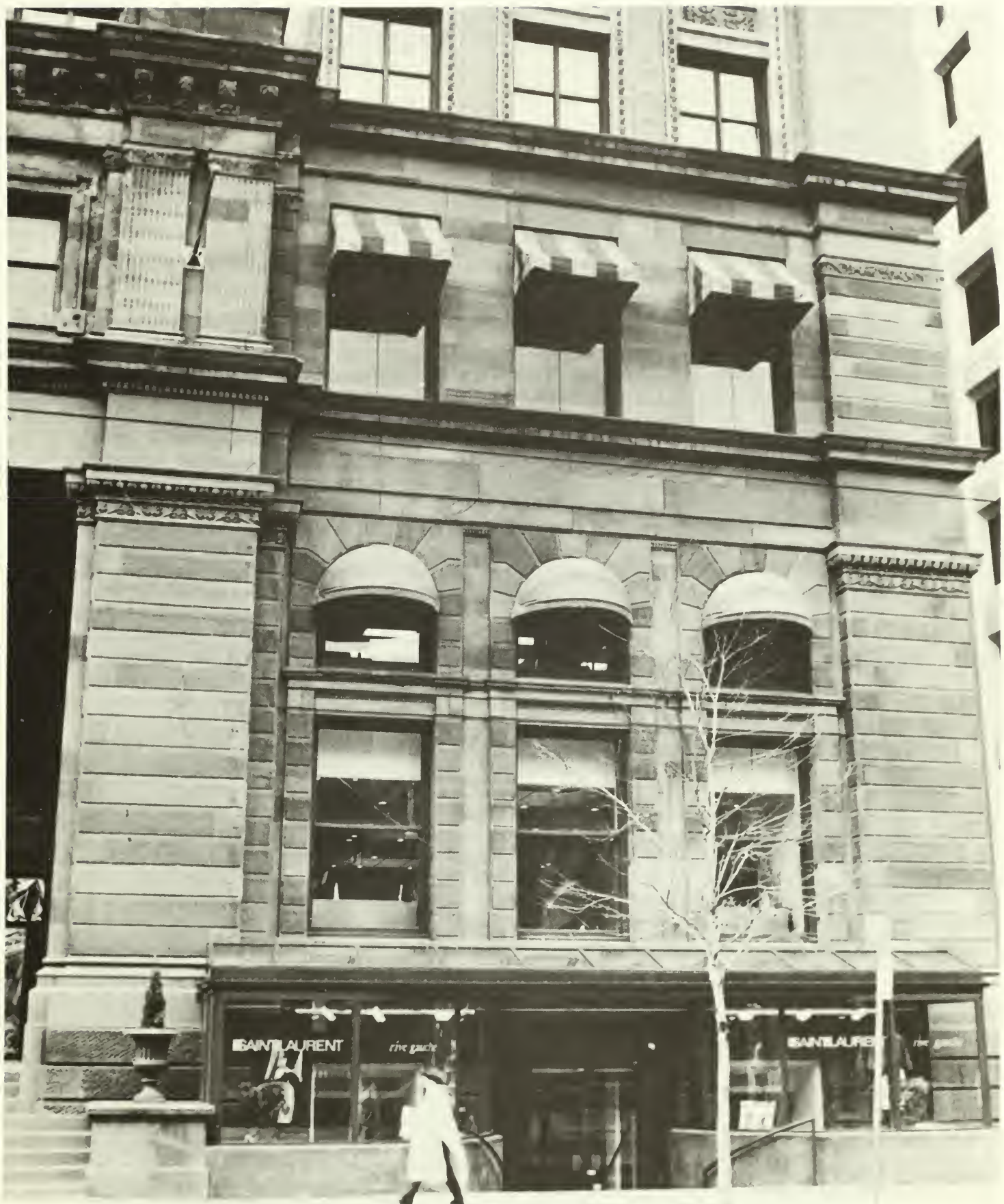
6. The Option A entrance canopy in place.
