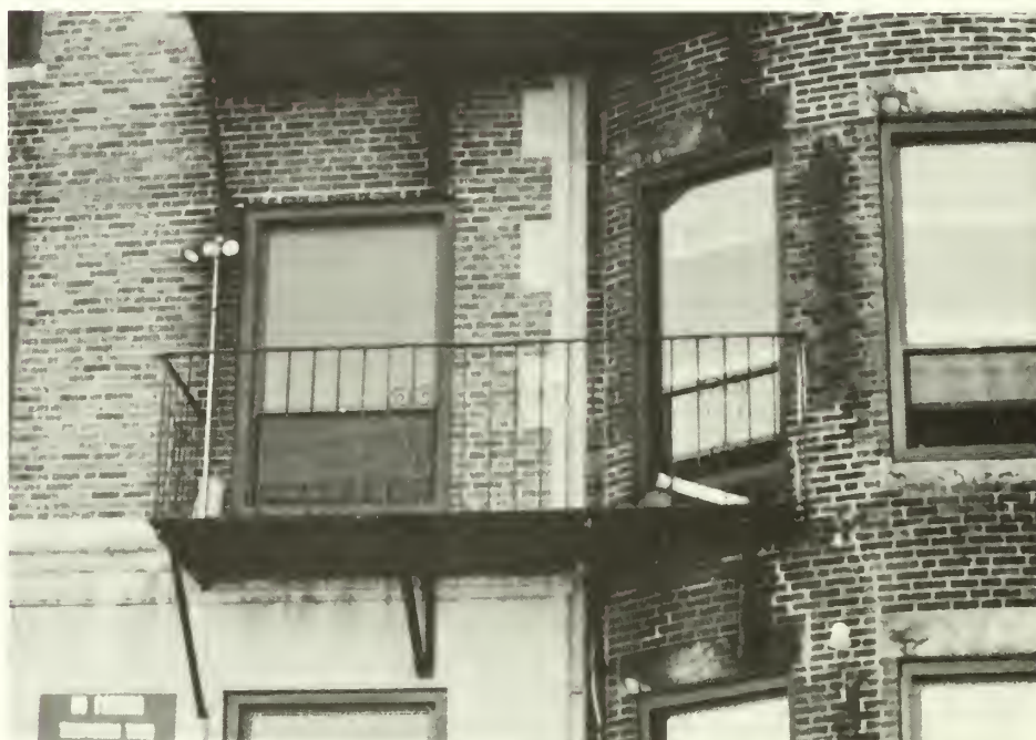
2. This is a close-up view of the contemporary window units which were installed. They had flat framing detail, bronze-anodized finish, tinted glass, and a lowered meeting rail.
