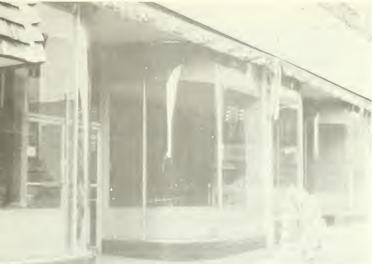
3. The entire storefront was replaced following breakage, during rehabilitation of one of the curved sheets of glass. Expediency and difficulty in locating a manufacturers of curved glass were cited by the owner as reasons for the change.
