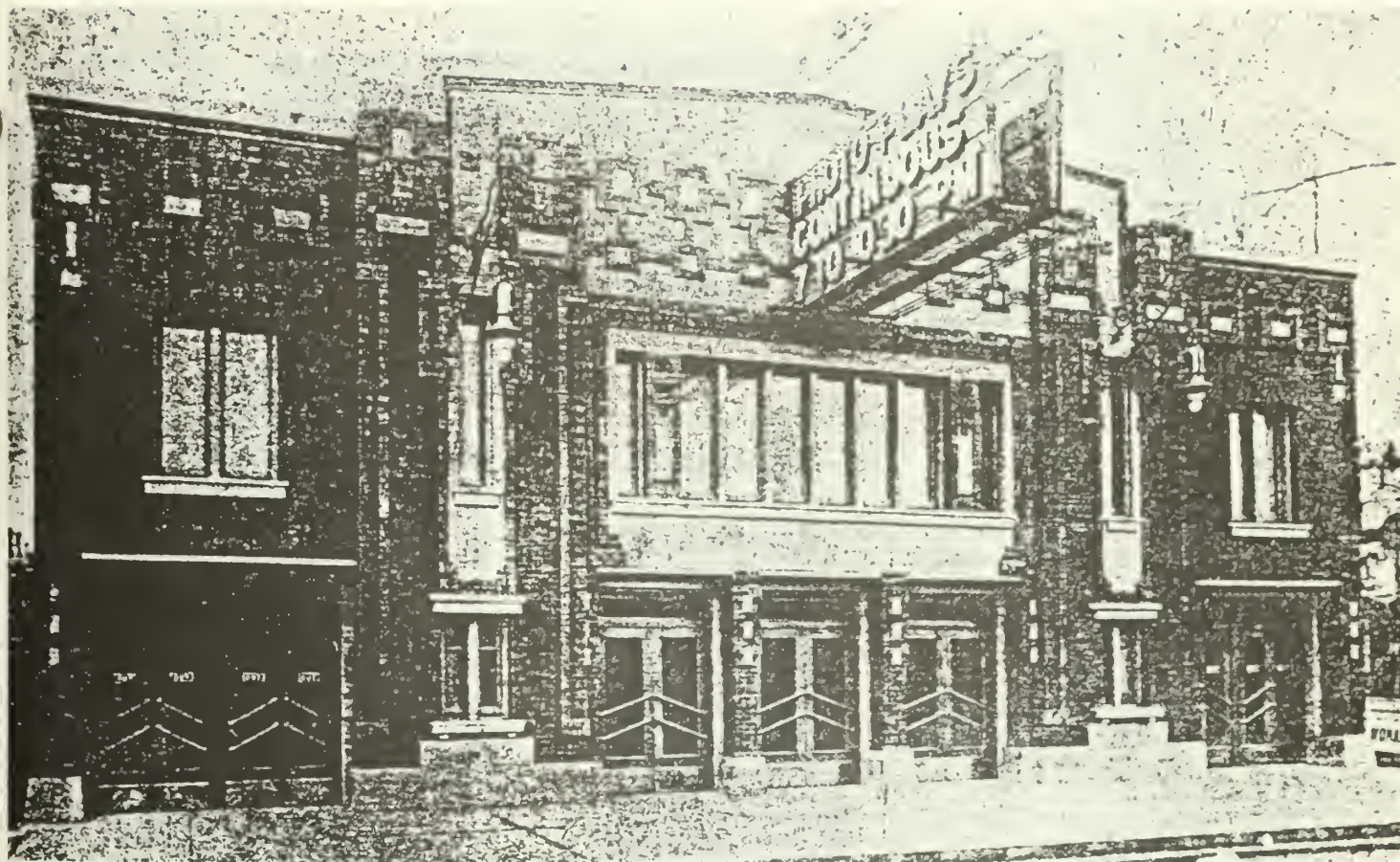
4. Historic photograph of the theatre's facade as it appeared in 1913. Note the glazed wooden double doors, repetitive features that, together with the distinctive rectangular openings themselves and the patterned brickwork, define the architectural character of the building.
