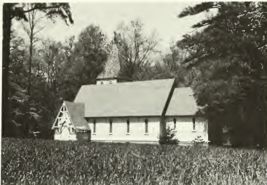
7. South elevation of church after rehabilitation.
