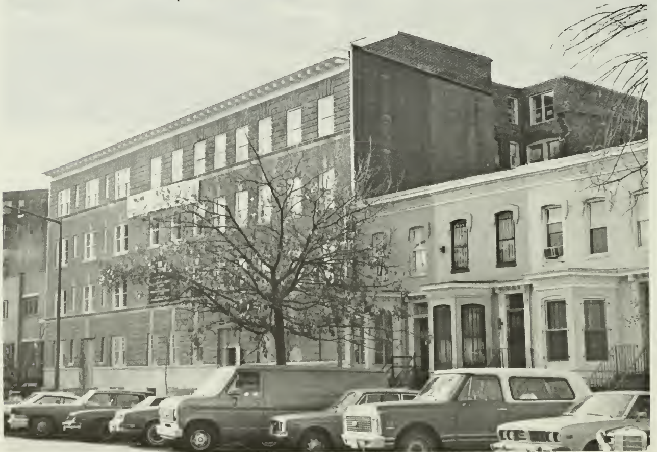
3. New rooftop addition visible on the north elevation.
