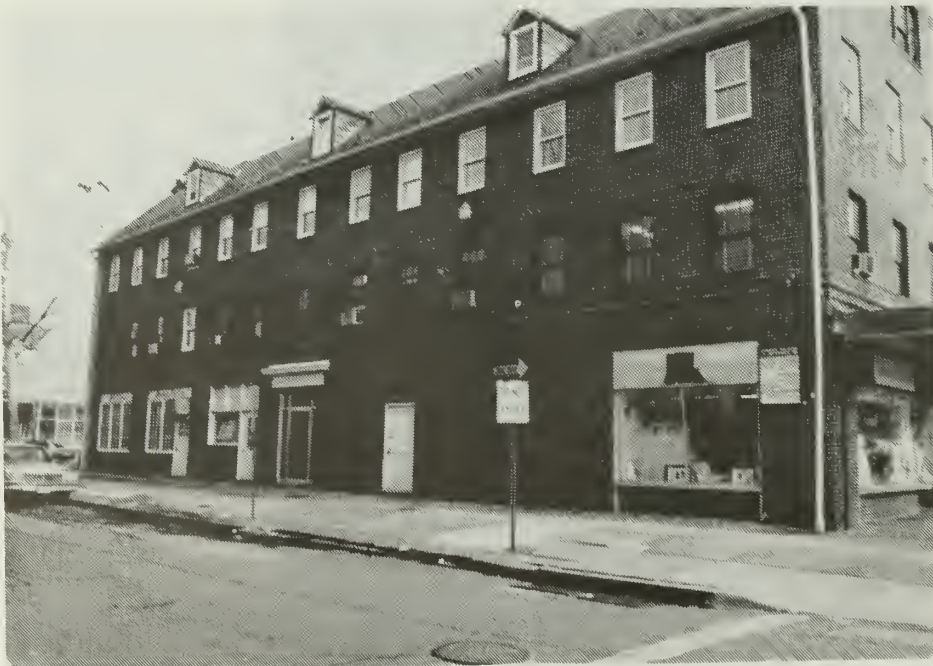
8. Proposed replacement windows on third floor and original windows below. Note how dark sash and frames are unobtrusive, light sash and frames create a striking pattern on the red brick facade.
