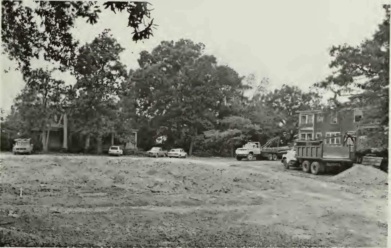
3. The front yard of the mansion has been prepared for the relocation of the neighboring house, seen at right.
