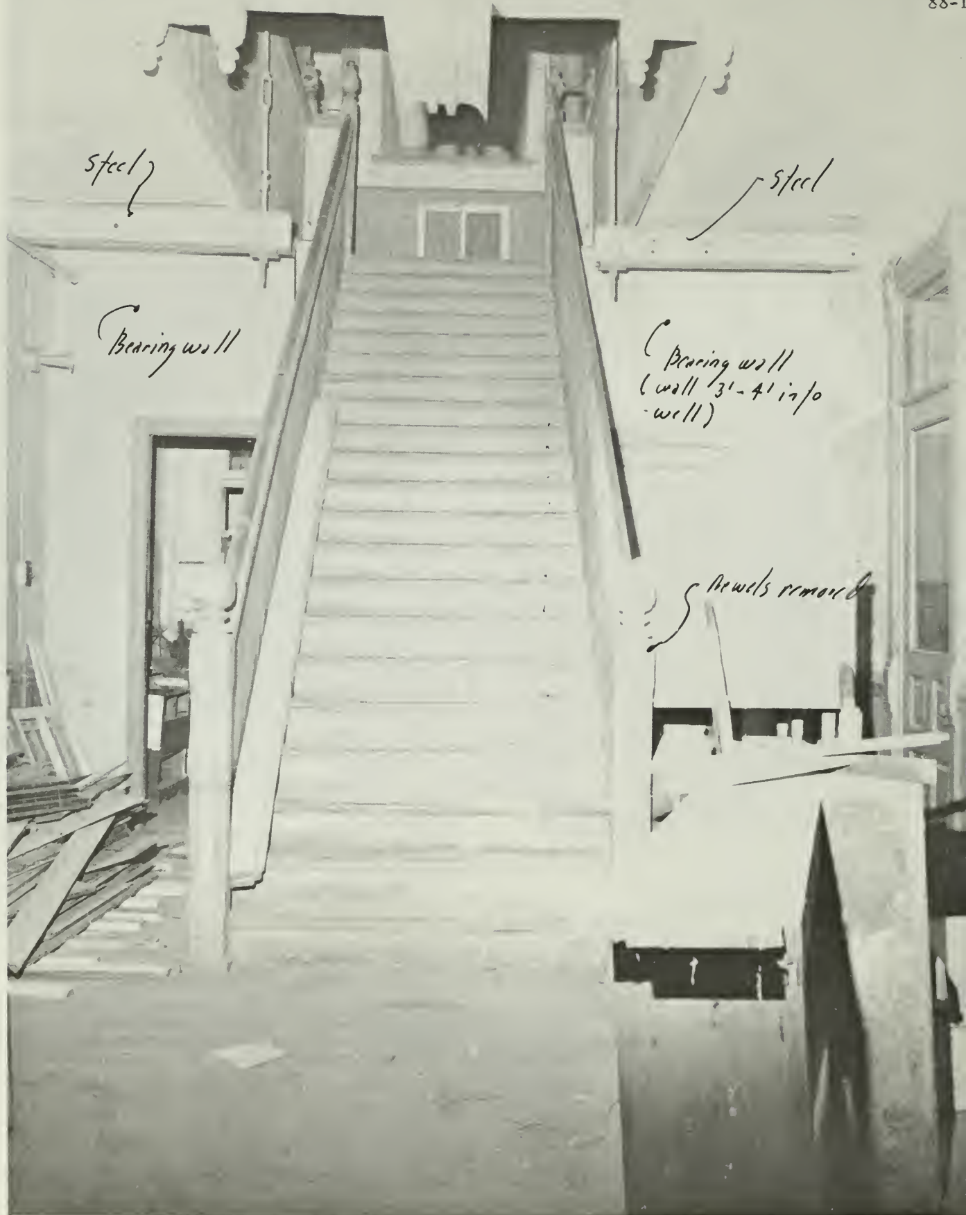
2. Pre-rehabilitation photograph of first floor center stair and hall. This stair was removed in the process of rehabilitation.
