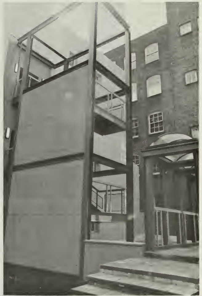
4. Stairtower provides fire exit from building at left.
