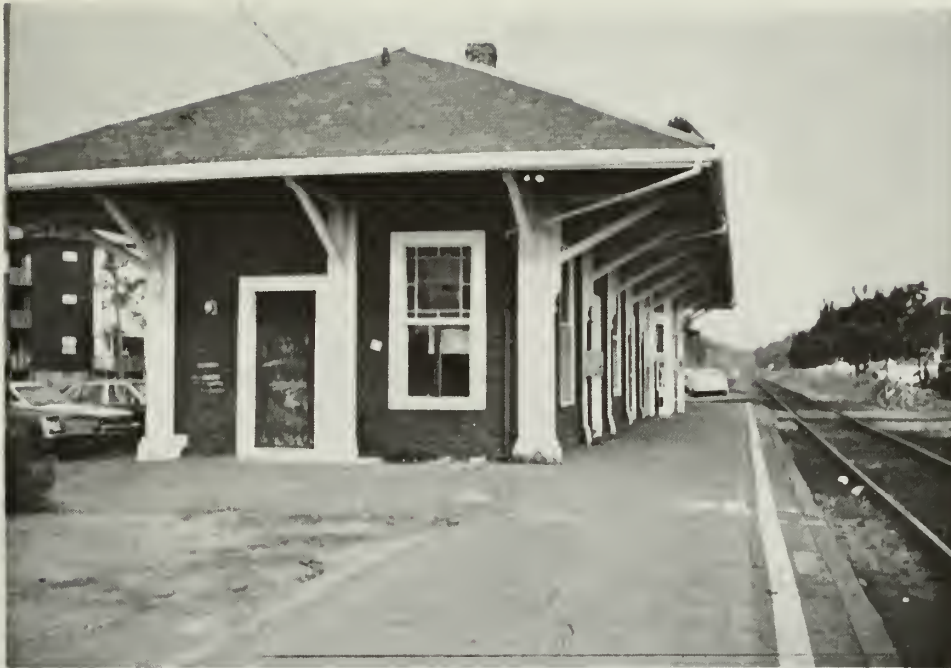
1. Railroad depot prior to rehabilitation.
