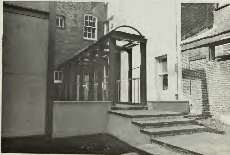
5. Covered walkway serves as the principal entrance to all four rehabilitated structures.
