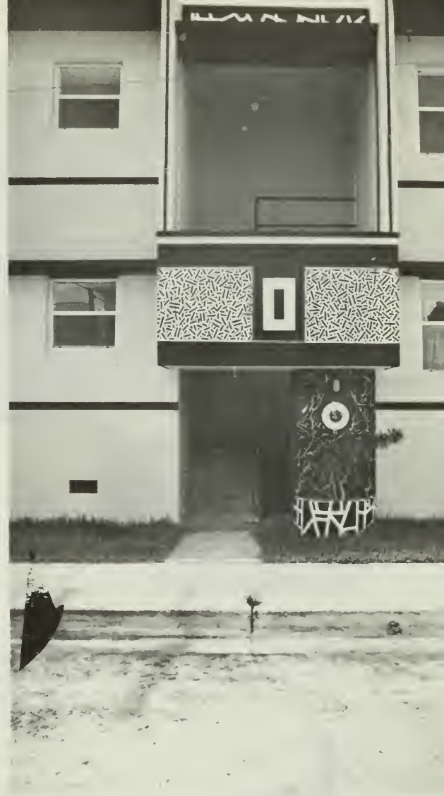
3-5. After rehabilitation the character of the building has been greatly changed by the application of a variety of decorative painted finishes, in particular the "faux" stone surfaces around doors, the contemporary patterned design used above doors and on balconies, and the "cracked tile" pattern on the planters that surround the building.
