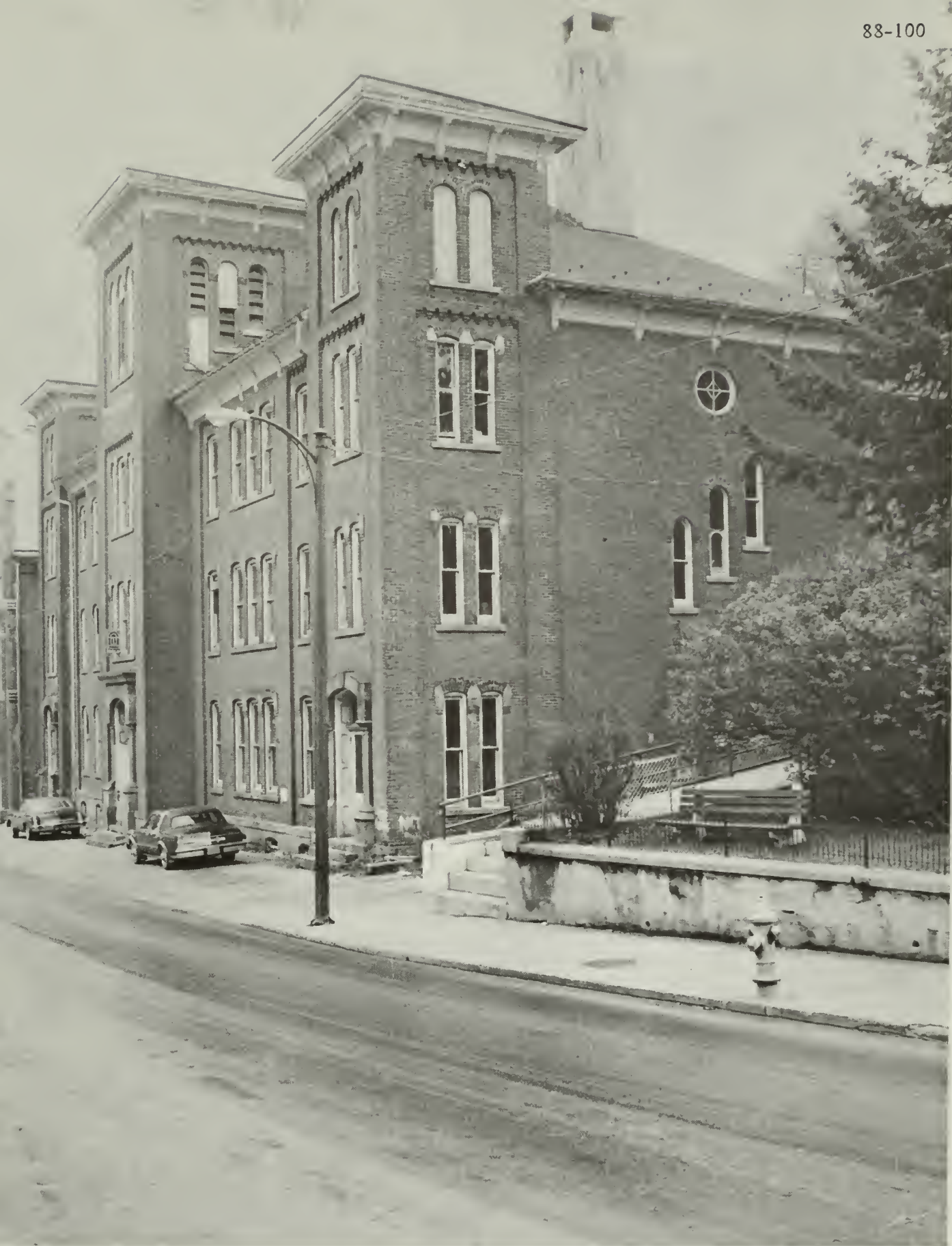
Pre-rehabilitation photograph of school building.
