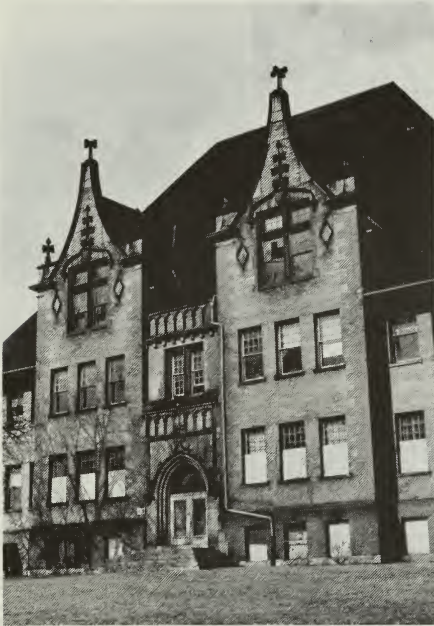
1. The former school building is characterized by its distinctive form--massive yet only three stories in height--its twin towers, unusual arch-shaped entrance and series of large-scale, twelve-over one windows that were designed to provide maximum daylight in the classrooms.
