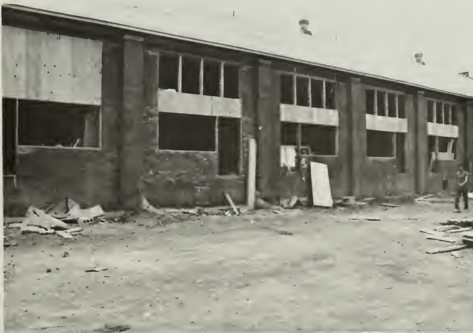
5-6. The rear elevation of the drill shed during rehabilitation. Note the extensive loss of brick, and how the character has changed with the removal of the multi-paned wood sash and the creation of large openings.
