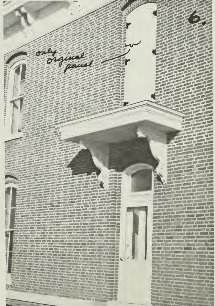
2-3. The reconstructed front porch (left) and the side porch (right). Their designs were based on bracket fragments found on the property combined with area residents' descriptions of the porches as they remembered them, but did not match the "ghost" outlines that had existed on the brick prior to cleaning.
