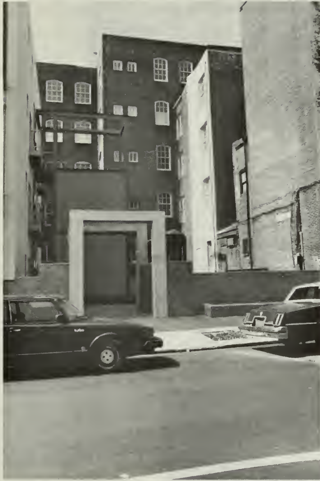
3. Entrance pavilion, front wall and stairtower are prominent new site features.
