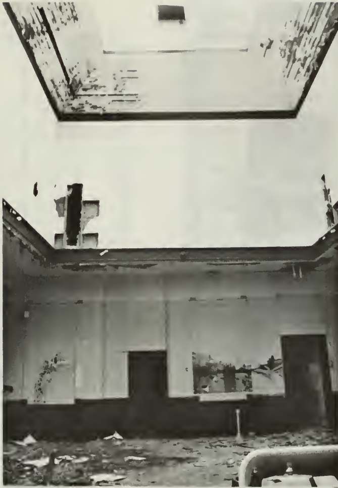
3. View of central space showing atrium extending through the second and third floors, with skylight above. The second floor doors shown lead to rooms beyond. Windows have been blocked in, but their configuration is still apparent from the surrounding trim. On the third floor the open hallway had been partitioned.
