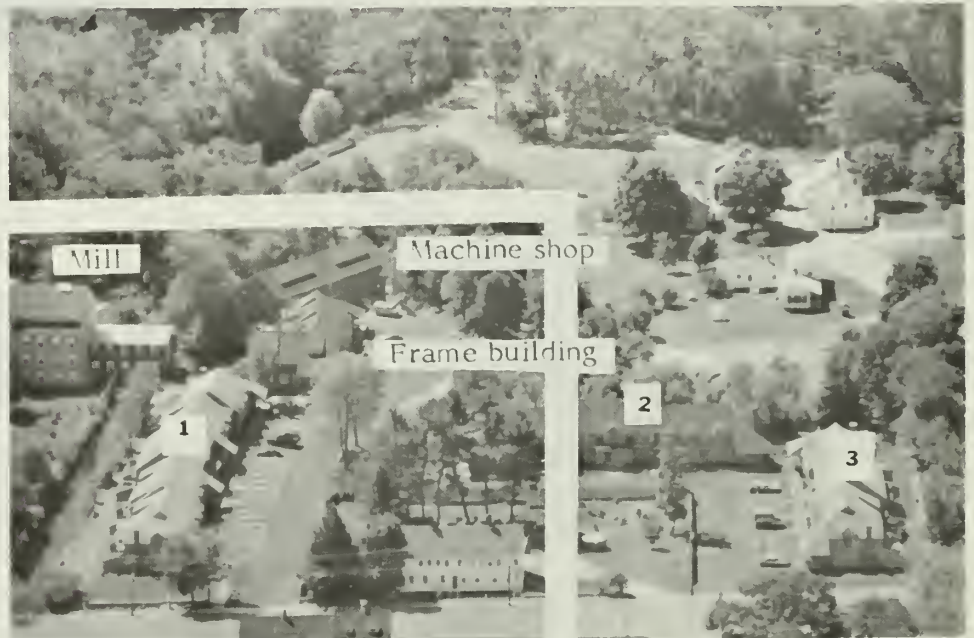
7. Aerial view showing blocks of new construction identified as 1, 2, and 3. White line is the approximate boundary of this part of the district.
