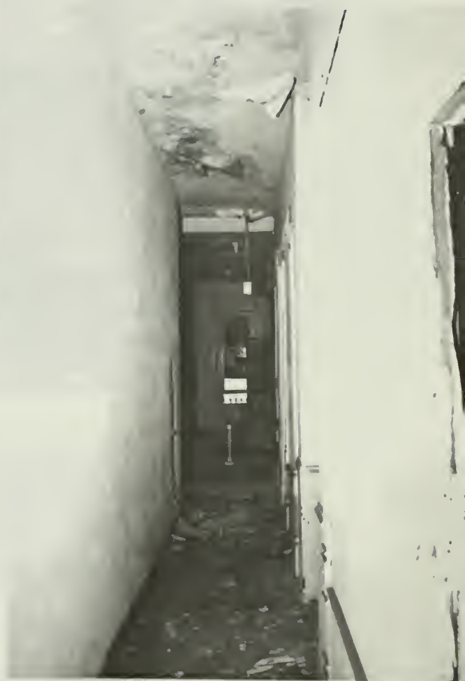
5. On the third floor, the historic hallway, originally open, had been fitted with a solid partition; the offices behind it, however, were relatively unaltered.
