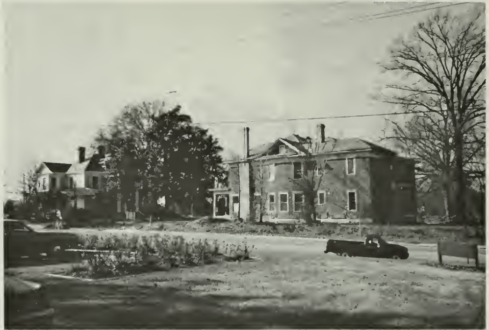
5. Turned 180 degrees, the moved building faces the historic one from a distance of 60 feet.
