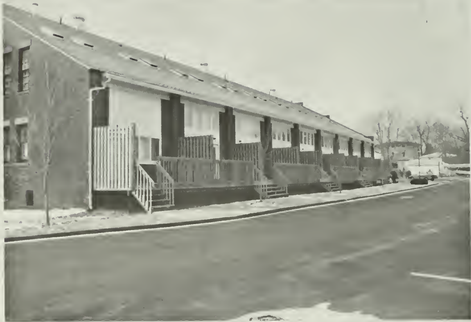
7. The rear of the drill shed showing the completed rehabilitation with the new skylights in the roof, the prefabricated panels filling the former bricked areas, and the new wood decks and privacy fences facing onto a parking lot at the rear of the property.
