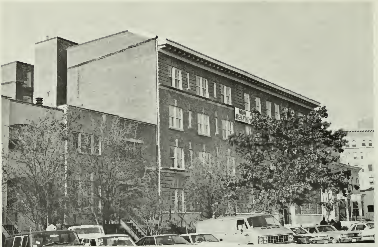
2. New rooftop addition and stairtower visible on the south elevation.
