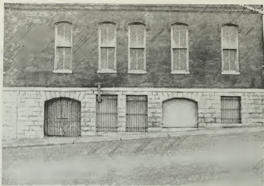
3. Before rehabilitation, the windows on another street elevation were four-over-four units that feature delicate, attenuated muntins. The historic window is a double-hung design; the shadow line that the meeting rail casts at the center of the two-part window is a distinctive quality.
