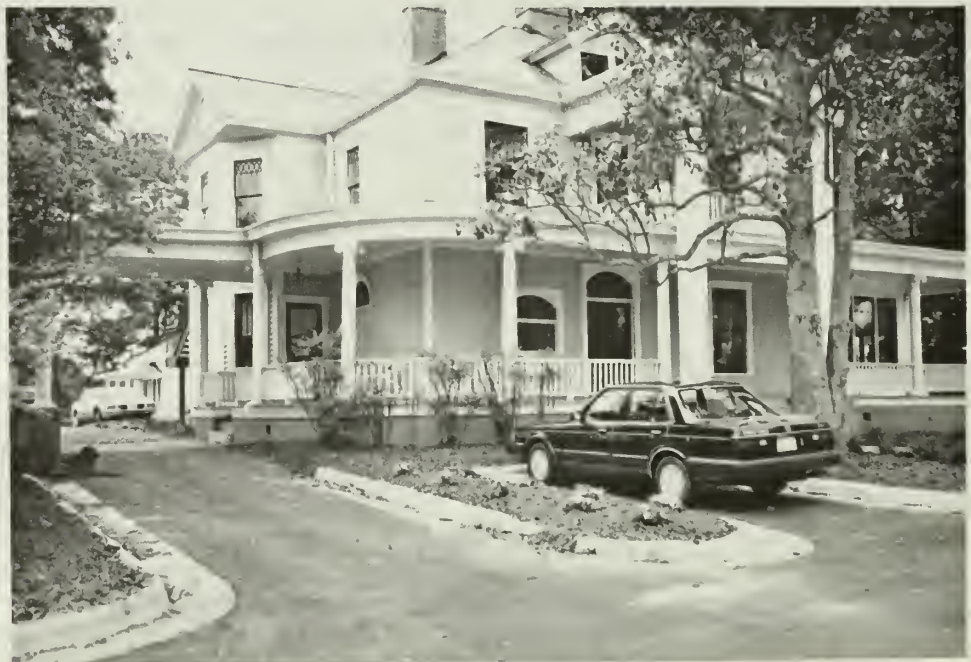
6. The parking lot completes the drastic alteration of the setting. The second relocated structure is seen through the porte-cochere at left
