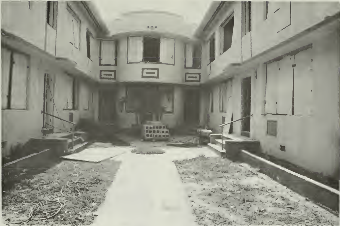
1. The primary entrances to this early 1940s Moderne apartment building are located in the courtyard of the U-shaped structure. Note the overall plainness of the building before rehabilitation, which is highlighted only by horizontal banding and raised geometric panels.
