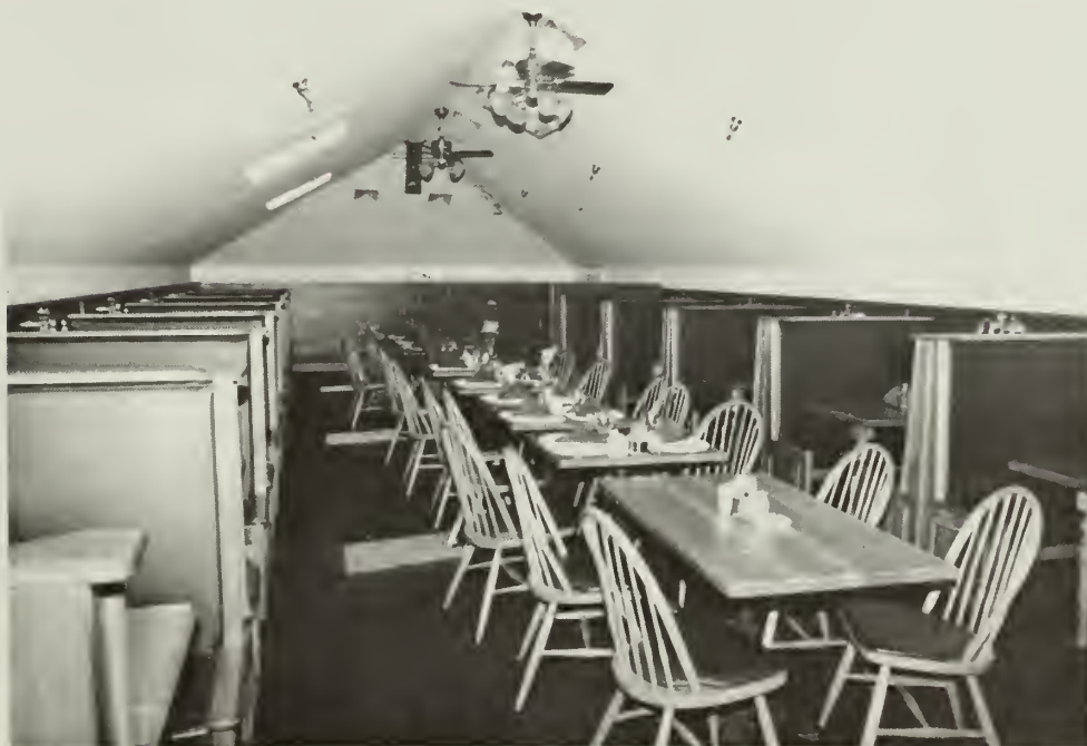
6. Post-rehabilitation view of second floor. Original attic space converted to restaurant space by lowering the ceiling below.
