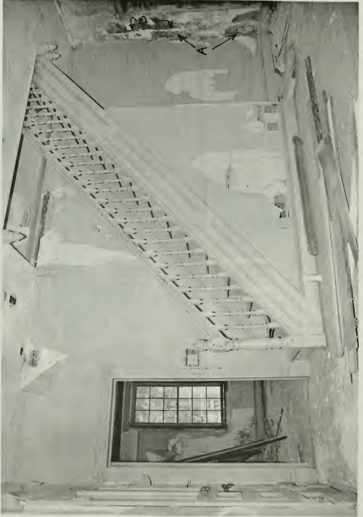
2. Circa 1912 stair prior to rehabilitation. Moldings, floor plan, and other detailing are all 20th century.
