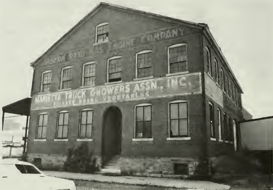
1. Front elevation of the 1880 manufacturing facility as it appeared prior to the rehabilitation.
