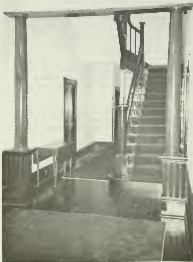
1. The only primary space on the first floor left unaffected after rehabilitation was the central hall, shown here with its original ceiling height and column divider.
