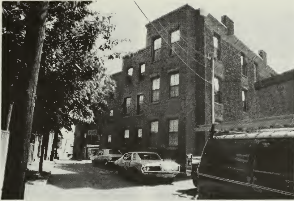
1. Pre-rehabilitation photograph of workers' rowhouses (front elevation).
