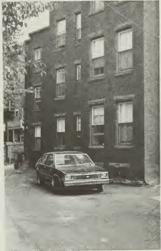
6. Post-rehabilitation photograph of historic rowhouses with matching wood windows.
