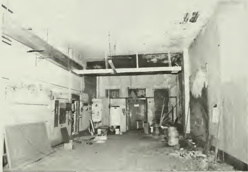
2. Typical ground floor space before rehabilitation.
