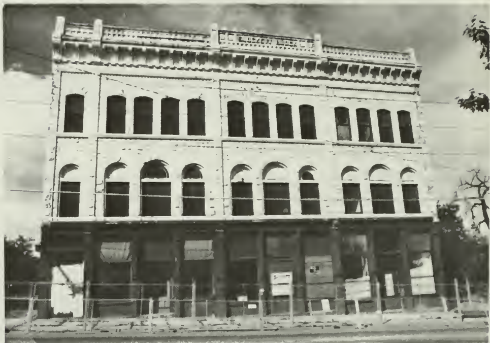
1. 1890 commercial building prior to rehabilitation.
