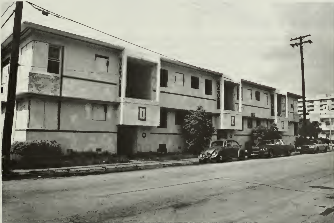
2. The street elevation of the building where patch repair work has already begun shows the decorative panels of local stone under the second story windows at either end of the building.
