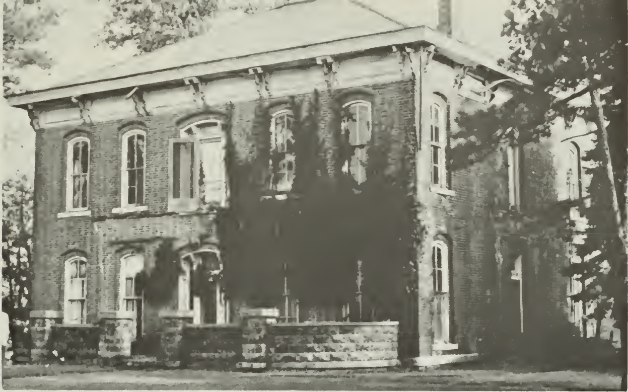
1. The house as it appeared when acquired by the current owner. Note the "ghost" outline of a porch on the front, the second floor exterior doors, and the elliptical cast stone terrace.
