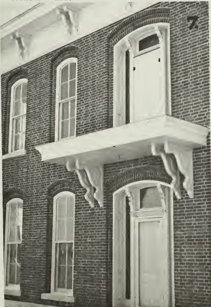
2-3. The reconstructed front porch (left) and the side porch (right). Their designs were based on bracket fragments found on the property combined with area residents' descriptions of the porches as they remembered them, but did not match the "ghost" outlines that had existed on the brick prior to cleaning.
