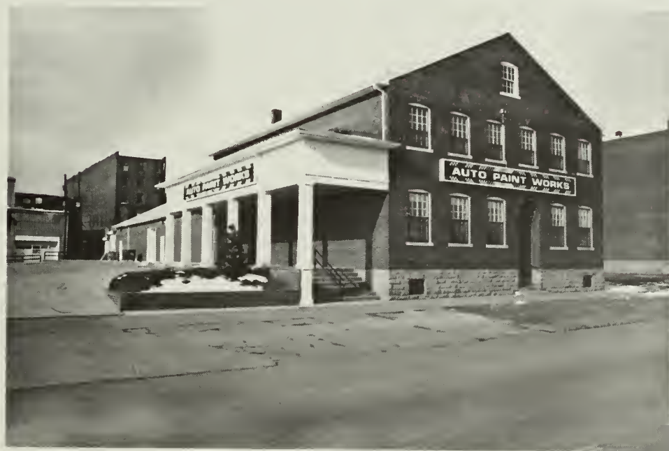
3. Photograph of building after rehabilitation with construction of portico.
