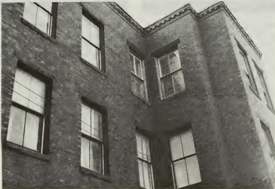
2. Pre-rehabilitation photograph of historic two-over-two double-hung windows that had a thin vertical muntin and wooden molding (brick molding) around the frame.
