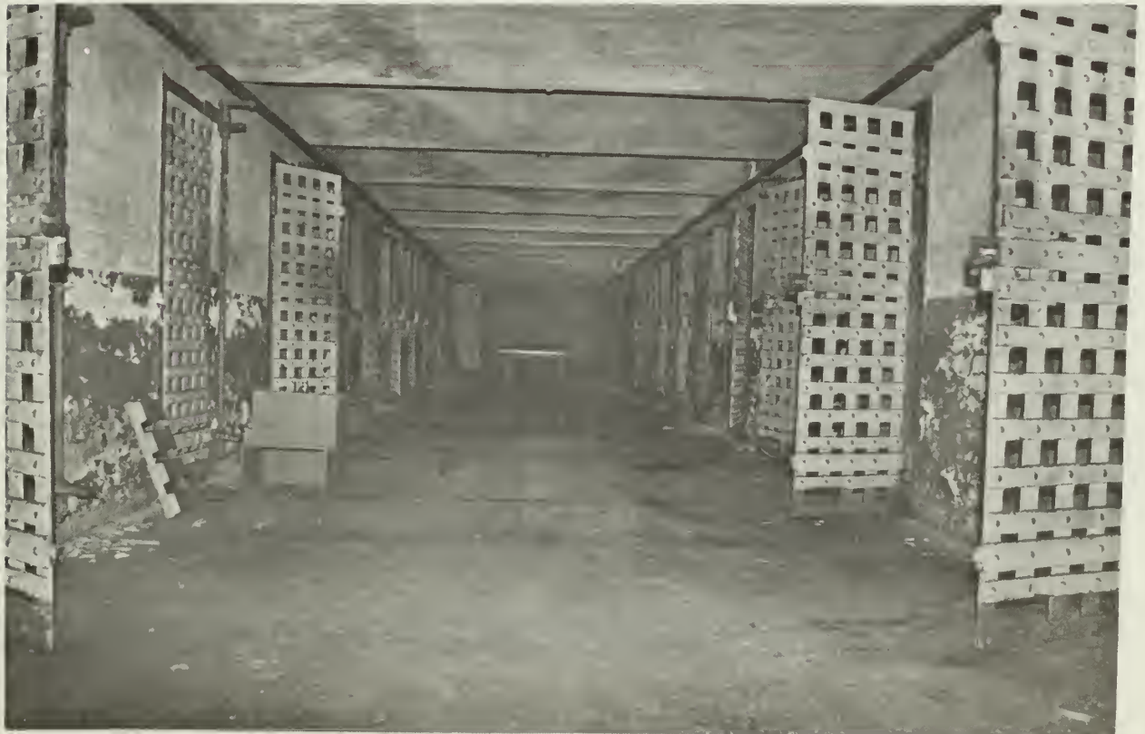
2. Interior of the cell block. Cells were 5' x 8', separated by 18" load-bearing walls.
