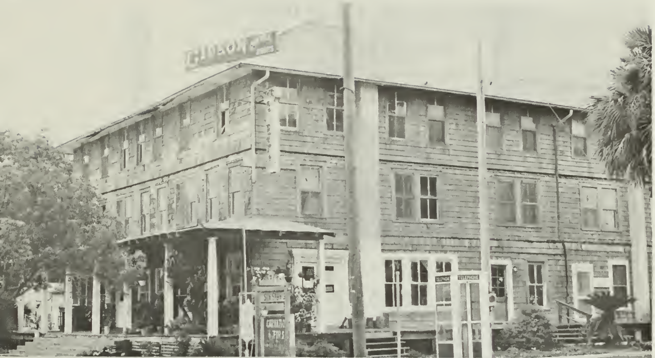
2. The hotel in 1984, prior to rehabilitation. The cupola and dormers are missing, and although a one-story front porch spans the primary elevation, it bears little resemblance to the two-story historic porch shown in the 1907 photograph. The hotel was certified as contributing to the significance of the historic district in its existing condition.
