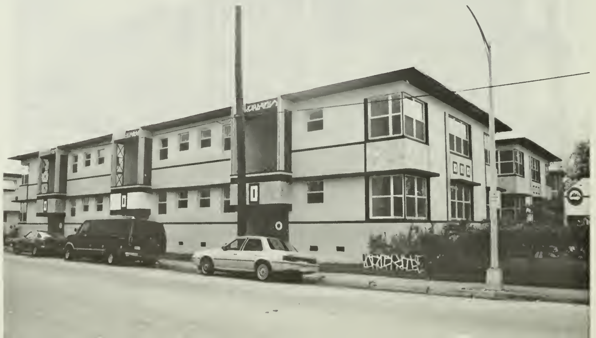
3-5. After rehabilitation the character of the building has been greatly changed by the application of a variety of decorative painted finishes, in particular the "faux" stone surfaces around doors, the contemporary patterned design used above doors and on balconies, and the "cracked tile" pattern on the planters that surround the building.
