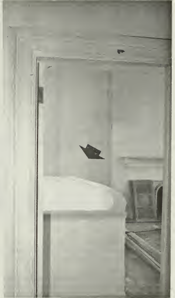
8 and 9. Fourth floor room, pre-rehabilitation (left) and in-progress (above). Note the insertion of the new staircase into the original bedroom in the post-rehab view.
