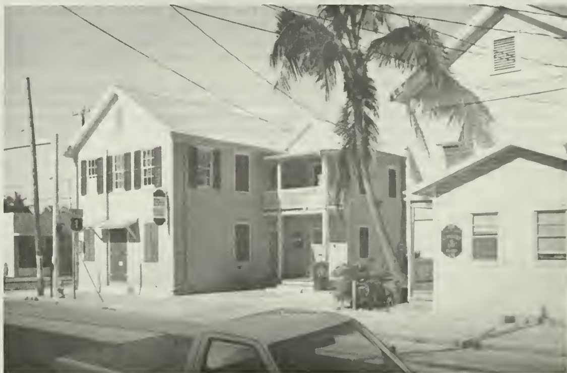
2. With the removal of the staircase there is no longer an indication of the second floor's independence from the first. The two floors of the ell addition appear to be functionally integrated.
