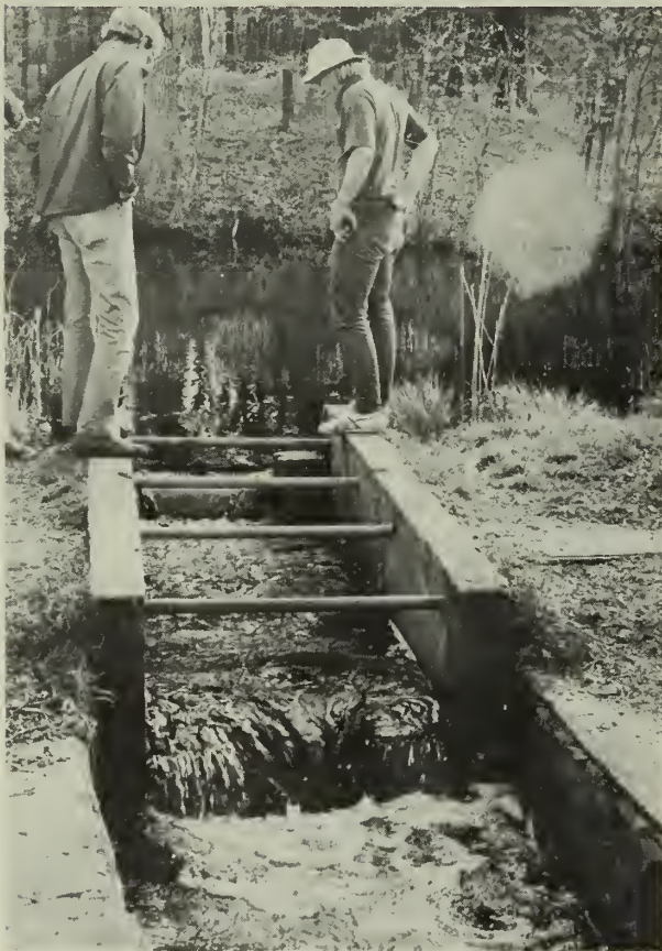
A fishladder designed for the passage of alewives in the Parker River. These anadromous fishes are being studied at the Massachusetts Cooperative Fishery Research Unit.
