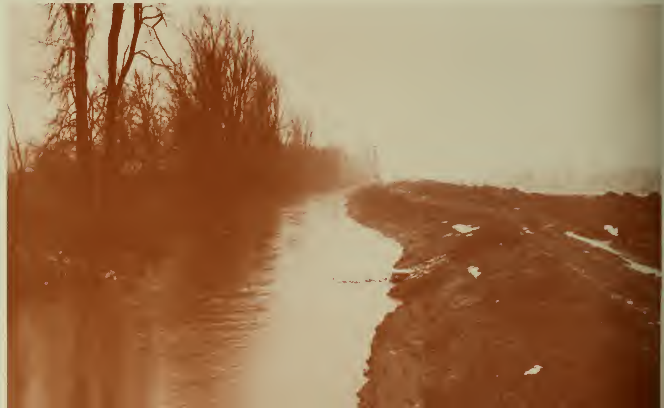
Rock Creek, Wells County, Ind., before (above) and after (below) channelization. The objectives of the National Stream Alterations Research Program are to investigate the effects of stream channelization on fish and wildlife and to provide technical advice and recommendations for mitigating those effects. As an example, the Service recommended alternate bank clearing for the Rock Creek project. (Photos by Jay F. Watson)
