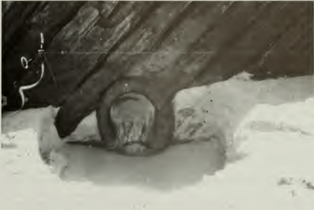
Figure 4.102. Comet's port-side hawse pipe. NPS photo by Don Morris.
