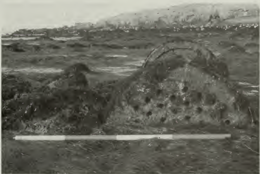
Figure 4.12. End view of the donkey boiler. NPS photo by Adriane Neidinger.
