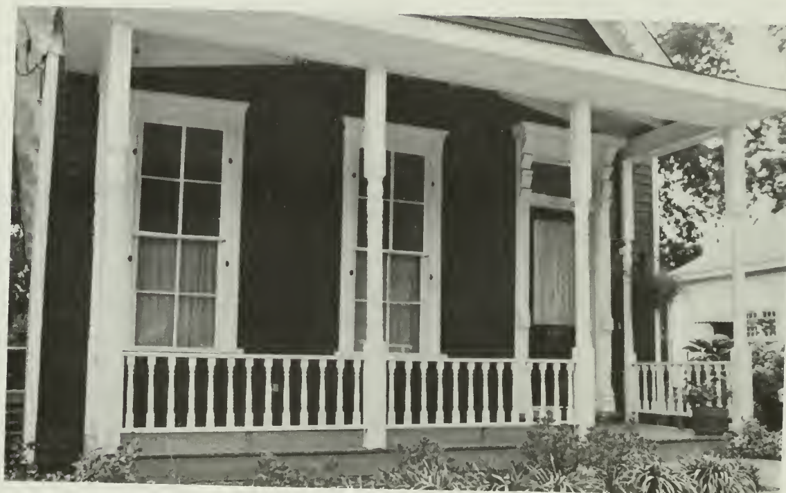
4. The 1880s cottage was in deteriorated condition prior to rehabilitation. Ghost marks of missing porch are evident. The original 2 over 2 windows had survived on the front and were to be repaired according to the plans submitted to NPS for prior review.
