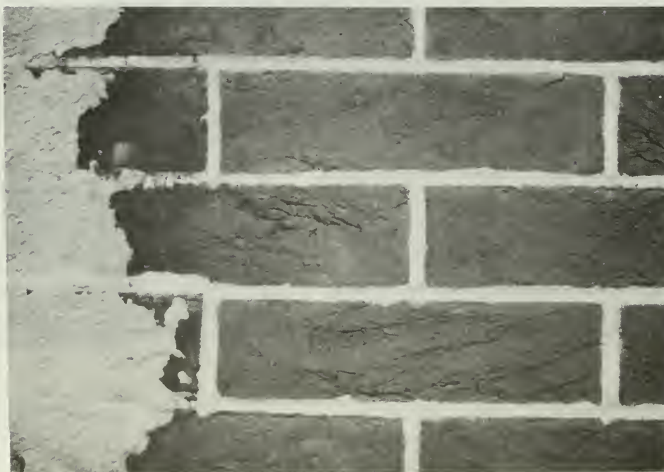
5. Close-up view of chemically cleaned brick showing deep ridges and newly abraded texture.
