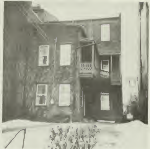
1, 2. The 3-story brick rowhouse, front and rear elevations, prior to conversion into a dress shop. Although many rear elevations are not particularly distinctive, this one featured a second story gallery and brick kitchen wing that were characteristic of the rear elevations of other residences in the district. Demolition of the wing and gallery preceded construction of a massive new addition that interrupted the former visual unity of the neighborhood.
