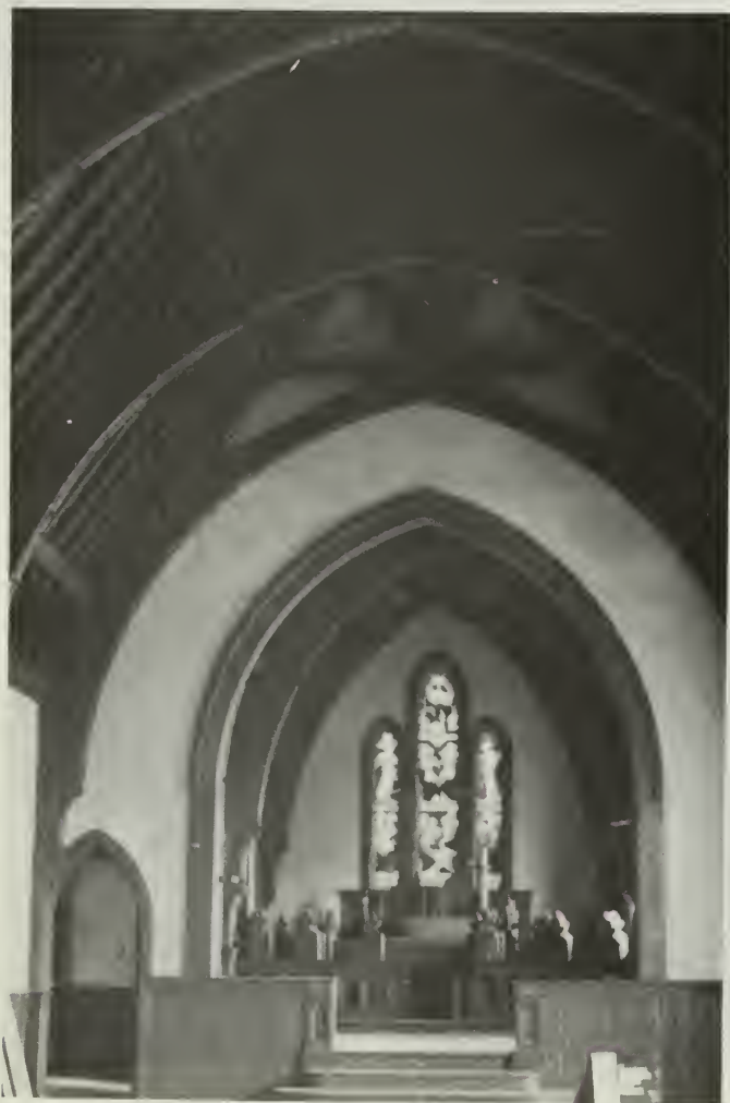
4. View of nave looking east into apse and sanctuary before rehabilitation.
