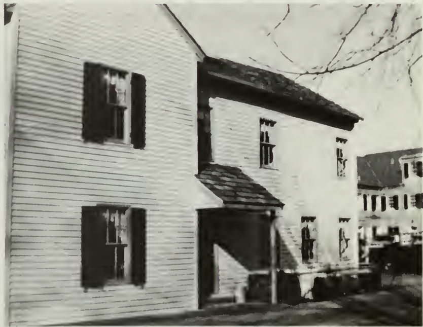
2, 3. The same building shown after rehabilitation is essentially new construction. Rather than targeted replacement of deteriorated materials, the owner replaced all of the siding, roofing, windows, sills, shutters, and trim. Some of the replacement features, such as the use of thick, cedar shakes on the roof and side porch were considered inappropriate. The owner was denied Part 2 certification on appeal. As a result of material loss during rehabilitation and the earlier loss of interior features and spaces, the Part 1 certification was also withdrawn because the building could no longer meet integrity requirements.
