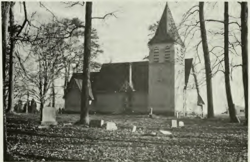
2. North elevation of church before rehabilitation.
