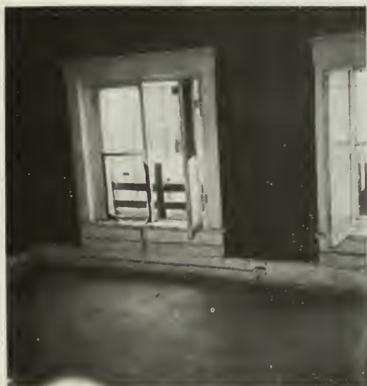
2. Modest interior detailing, such as window and baseboard trim, and diagonally placed mantels contribute to the historic character of the 1894 townhouse and thus should have been preserved to the greatest extent possible.
