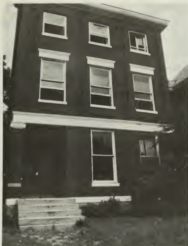
1. The townhouse, with its simple detailing, pictured before rehabilitation. The owner's proposal for exterior work was considered to be in conformance with the Secretary's Standards.
