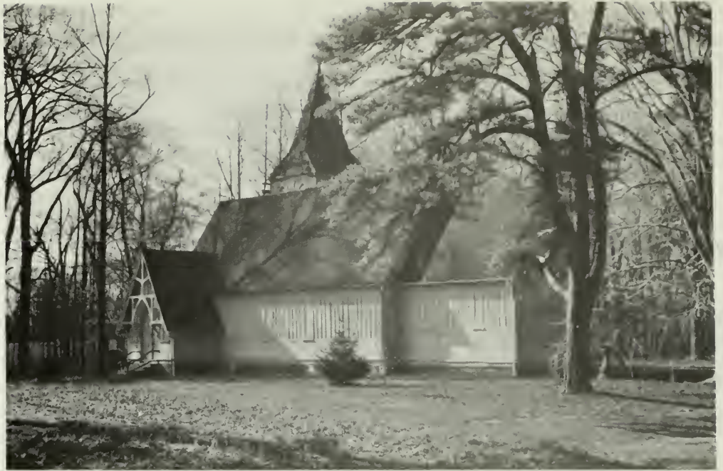
1. South elevation of church before rehabilitation.
