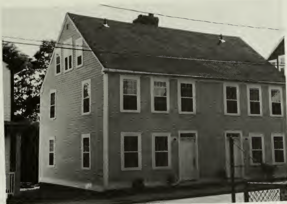
5-6. The two houses after rehabilitation, their porches removed to reveal the original early nineteenth-century character. (Twelve over twelve window replacement was based on remaining original sash still extant in several of the third floor windows.)
