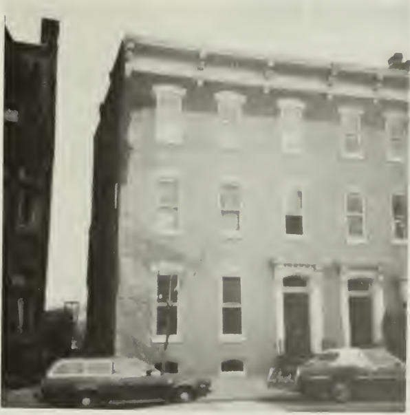
1, 2. The 3-story brick rowhouse, front and rear elevations, prior to conversion into a dress shop. Although many rear elevations are not particularly distinctive, this one featured a second story gallery and brick kitchen wing that were characteristic of the rear elevations of other residences in the district. Demolition of the wing and gallery preceded construction of a massive new addition that interrupted the former visual unity of the neighborhood.
