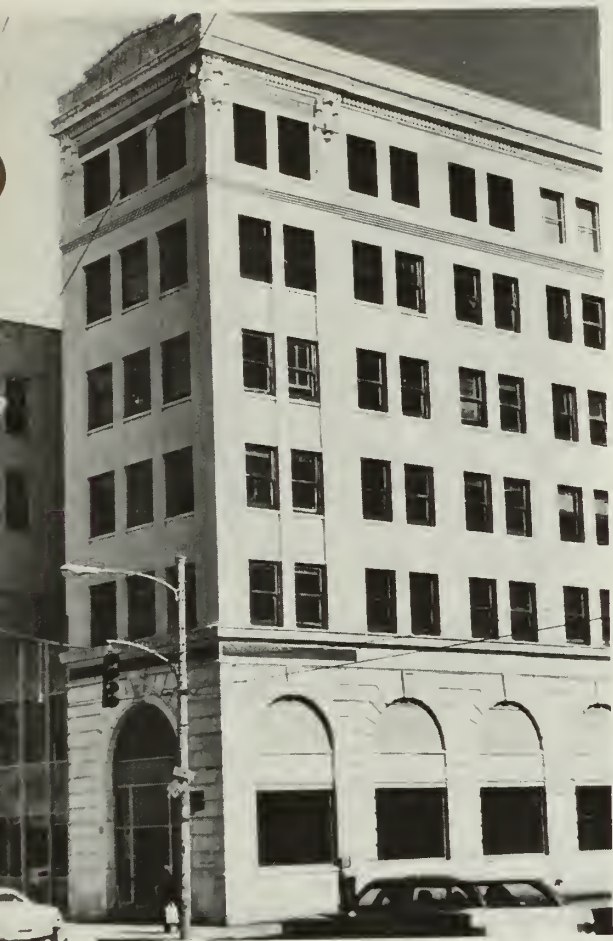
1. The original windows were of clear glazing and were of a one over one pane configuration.
