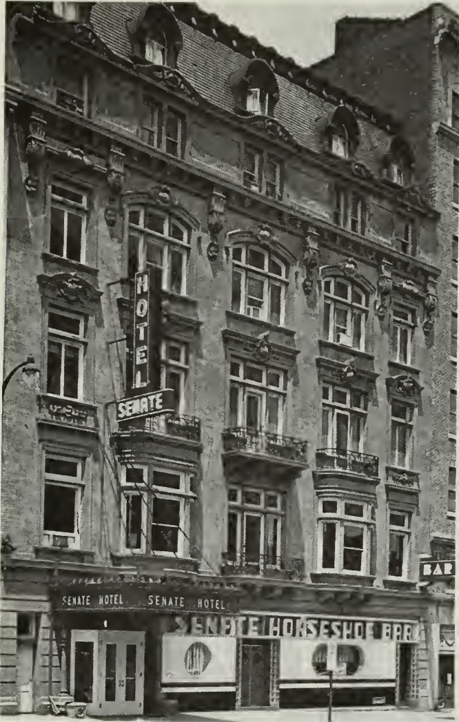
1. The 1906 hotel before rehabilitation. Note the Art Moderne facade and copper marquee on the first floor.
