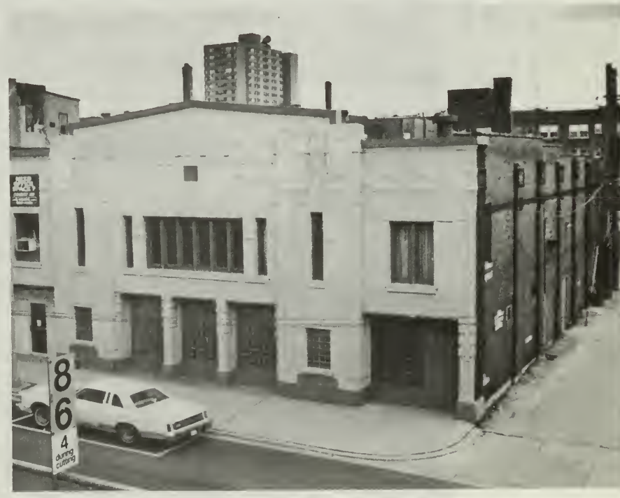
Theatre building as it appeared at the commencement of rehabilitation. The wooden doors had been removed in an earlier "renovation" and the openings filled-in with glass block. In addition, the masonry was painted a uniform gray. The stone sills cover a 22-inch-thick concrete floor inside.
