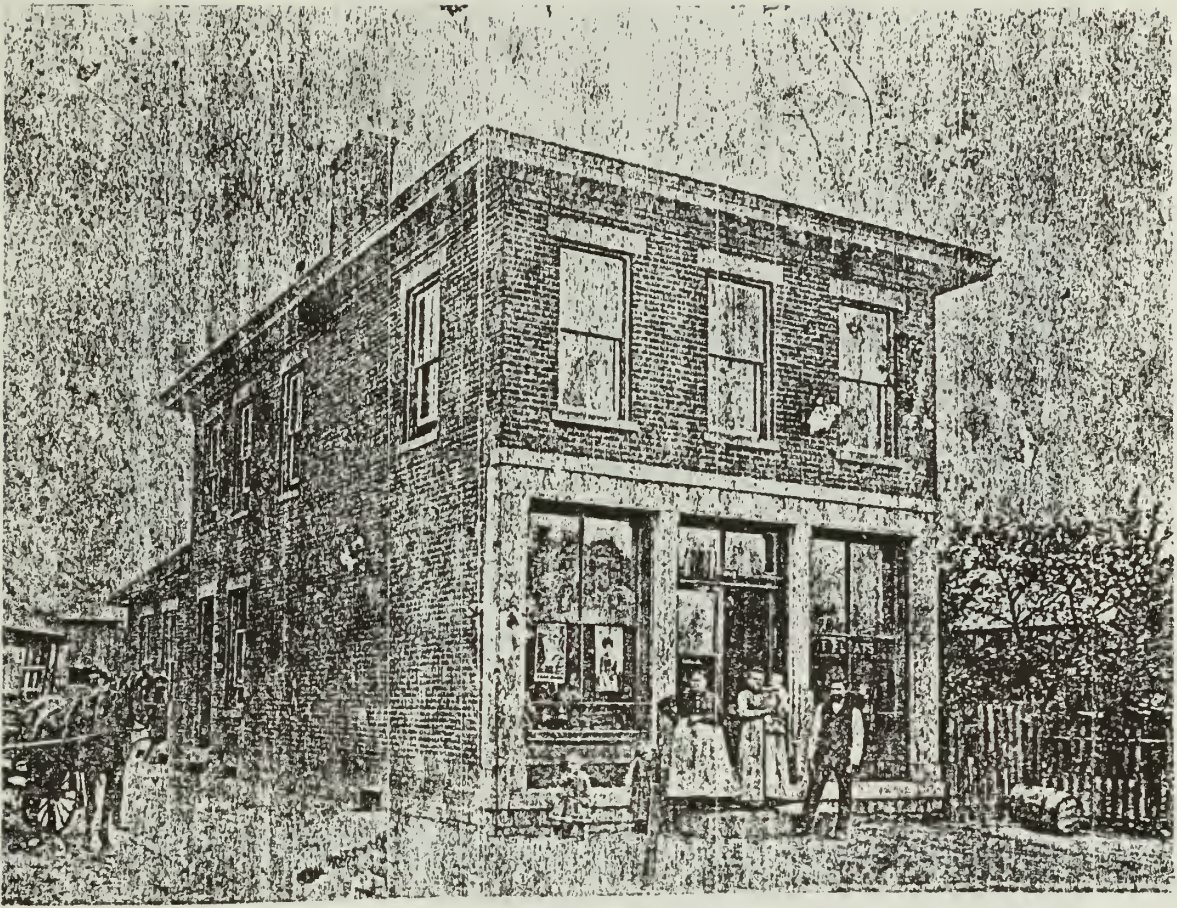
1a. and 1b. Historic photograph (1a) showing original three-bay storefront building (ca.1880-1890). With minor alterations, this storefront survived until most recent rehabilitation. Side door led to second floor apartments. Drawing (1b) shows the building's main features clearly.
