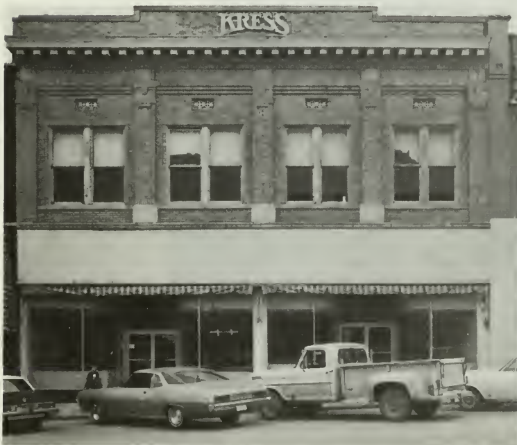
1. Prior to rehabilitation, the 1930s Kress Company storefront had survived in place with nice curved entrances although the transoms had been covered over.
