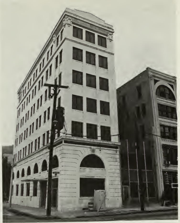
2. New windows with dark tinted glass and a vertical division on the upper floors were not in keeping with the character of the building.
