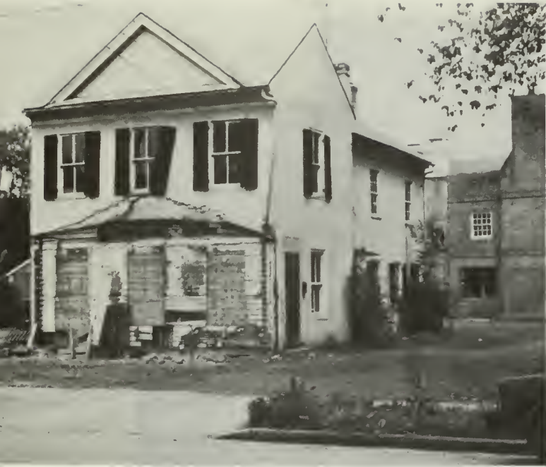
1. Front and side elevations of a ca. 1865-1870 wood frame building prior to rehabilitation. Stucco had been applied over the exterior wood at a later date and had caused rotting and termite infestation of historic wood. The building was certified as meeting Part 1 integrity requirements in its deteriorated and damaged condition.
