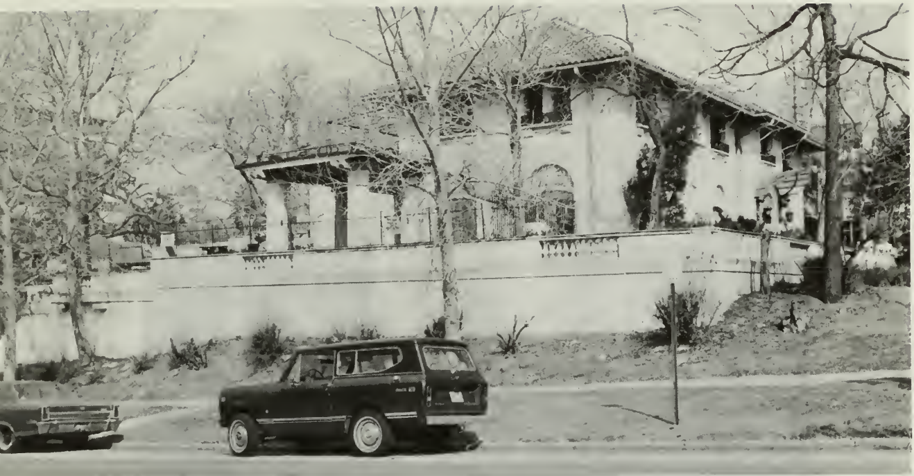
1. Side view of the house, showing the retaining wall around the site and the front terrace.
