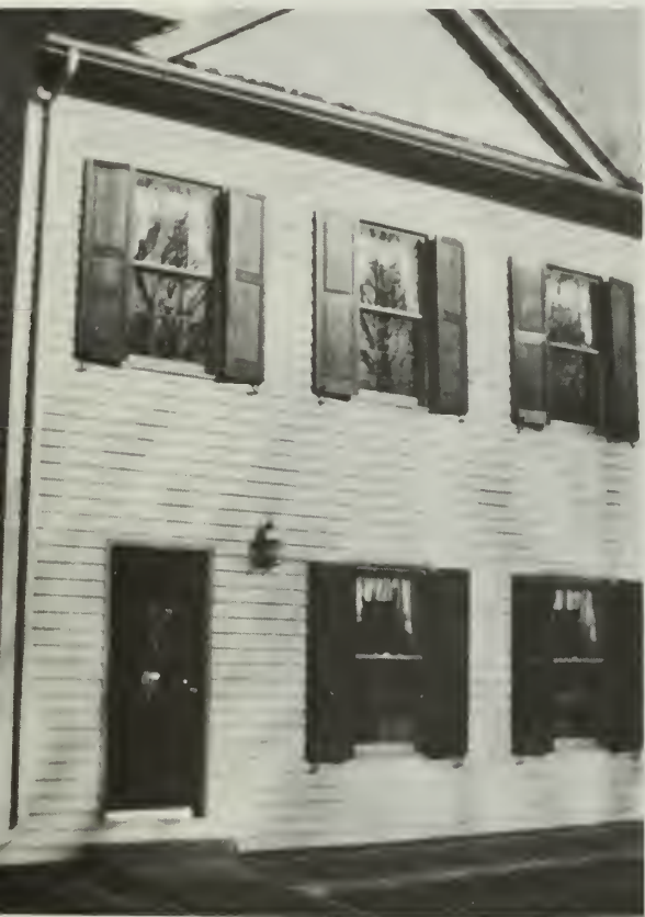
2, 3. The same building shown after rehabilitation is essentially new construction. Rather than targeted replacement of deteriorated materials, the owner replaced all of the siding, roofing, windows, sills, shutters, and trim. Some of the replacement features, such as the use of thick, cedar shakes on the roof and side porch were considered inappropriate. The owner was denied Part 2 certification on appeal. As a result of material loss during rehabilitation and the earlier loss of interior features and spaces, the Part 1 certification was also withdrawn because the building could no longer meet integrity requirements.
