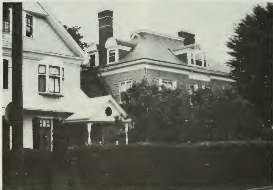
6. The building is shown here on the right in relationship to another building in the district. Although the historic wood sheathing has been obscured with formstone that is heavy and gray in appearance, the surviving physical characteristics of the rest of the building were sufficient to convey historic and architectural significance. This includes the roof shape and materials, and a decorative cornice and portico. Part 1 was issued. In the rehabilitation, the concrete veneer was simply patched and retained as part of overall work.
