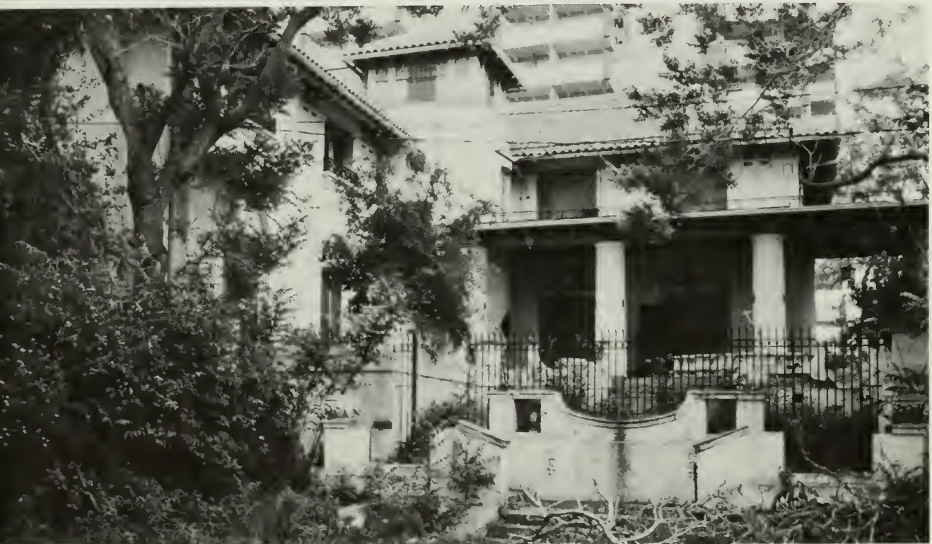
2. View of the rear of the house before rehabilitation began. There is a rear terrace with a pergola and a small walled garden with ornamental walls and an iron fence.
