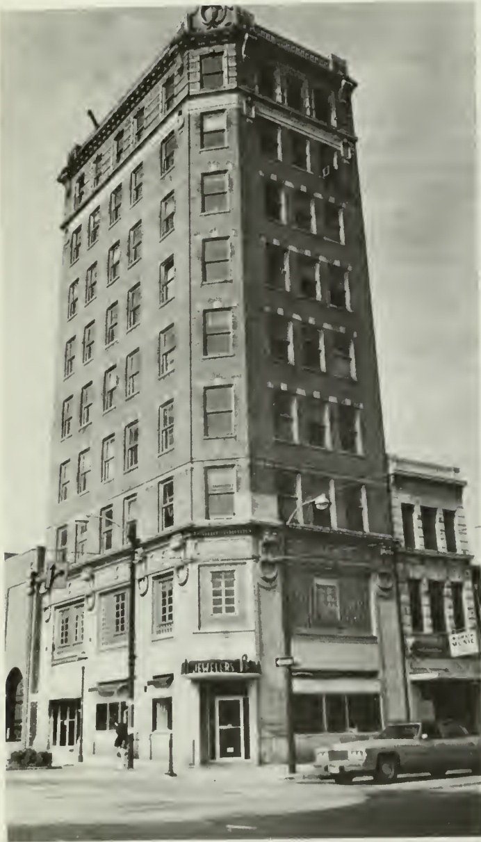
1. Nine story bank and office building before rehabilitation. Note uniformity of brick color.
