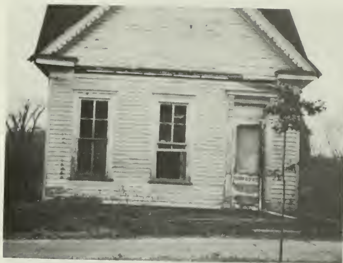
4. The 1880s cottage was in deteriorated condition prior to rehabilitation. Ghost marks of missing porch are evident. The original 2 over 2 windows had survived on the front and were to be repaired according to the plans submitted to NPS for prior review.
