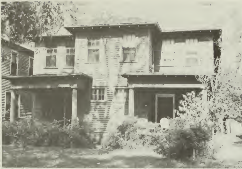
1. Prior to rehabilitation, the historic twin porch design and center projecting bay were strong architectural features.
