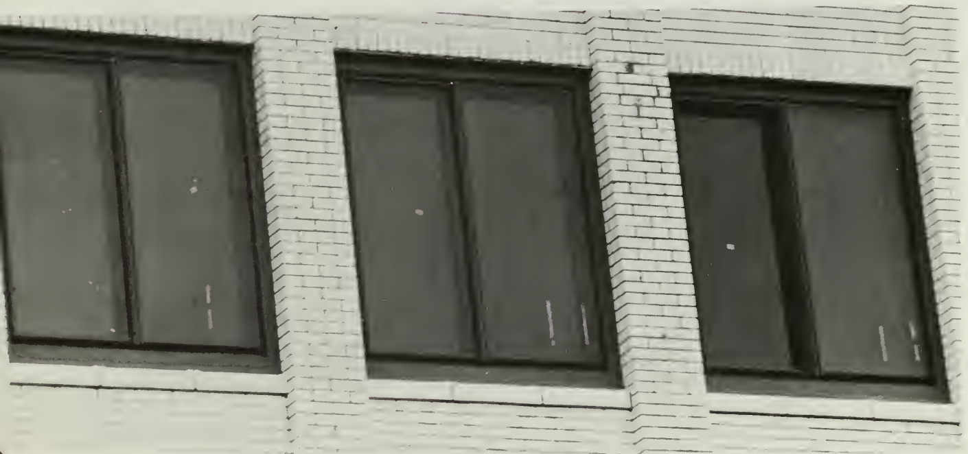
2. New windows with dark tinted glass and a vertical division on the upper floors were not in keeping with the character of the building.
