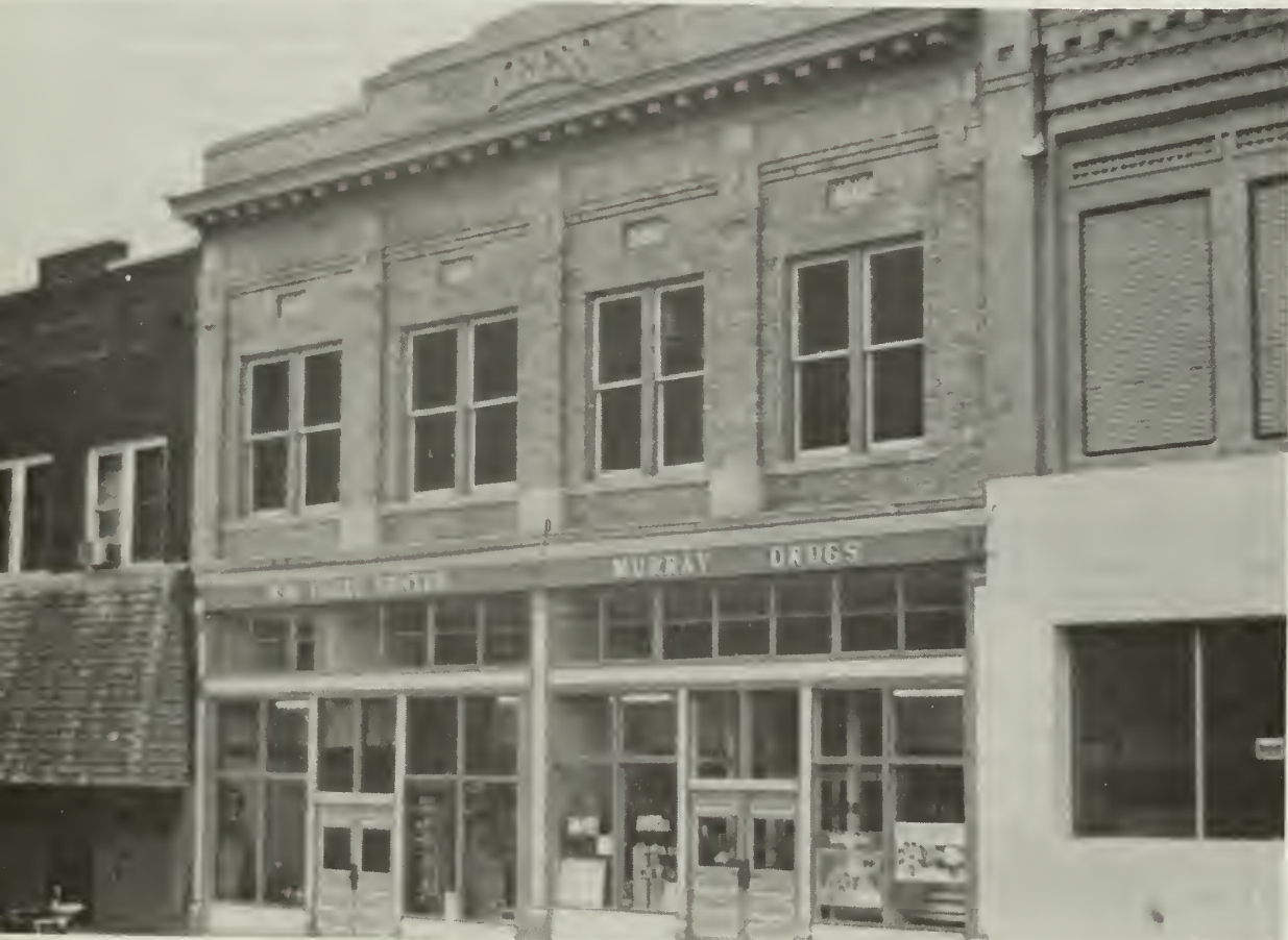
4. View of storefront after rehabilitation showing conjectural appearance of the original storefront — note inappropriate detailing of the transoms and small size of the doors.
