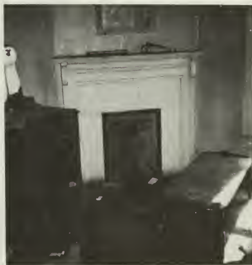
2. Modest interior detailing, such as window and baseboard trim, and diagonally placed mantels contribute to the historic character of the 1894 townhouse and thus should have been preserved to the greatest extent possible.
