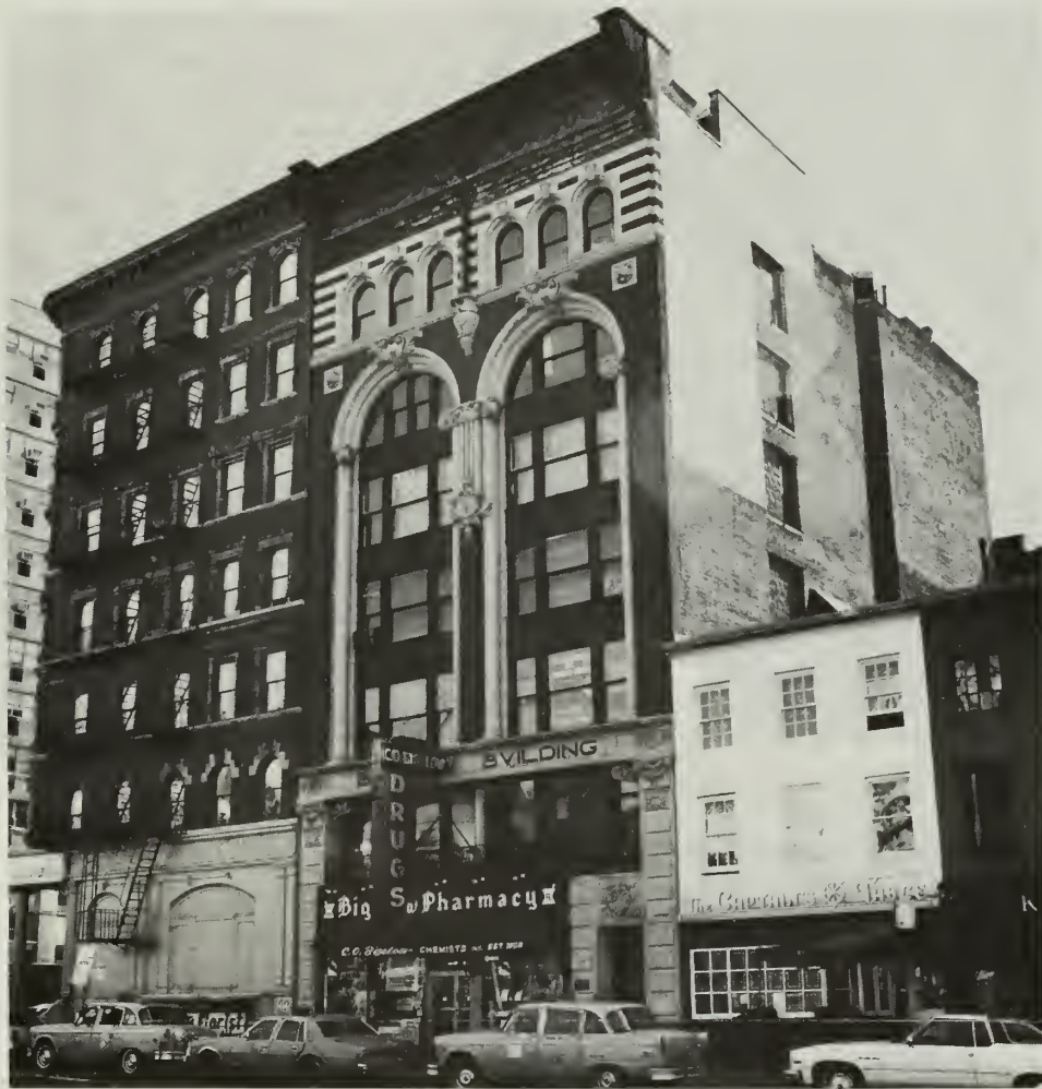
1. Rehabilitation project work on an early 20th century building focused upon meeting health and safety code requirements for the new use.
