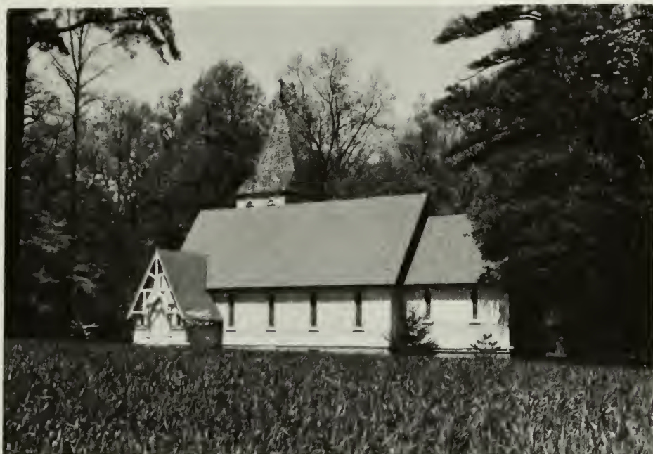
7. South elevation of church after rehabilitation.
