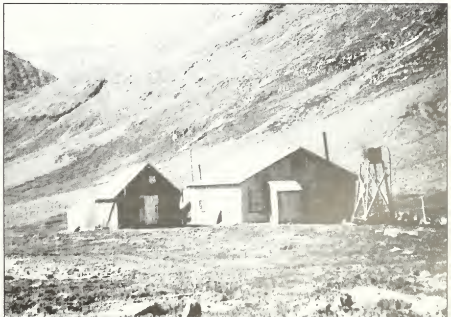
Figure 4.6. Bremner Gold Mining Company camp, circa 1938, looking southwest. In addition to the frame tent, storage shed, bunkhouse/cookhouse, and water tank, a third wooden structure (log frame) is also visible between the bunkhouse and shed. To provide additional warmth, the bunkhouse was lined with celetex, a lightweight cane board. View looking southwest toward the Lucky Girl Mine. Photo courtesy of Sylvia Baldwin.
