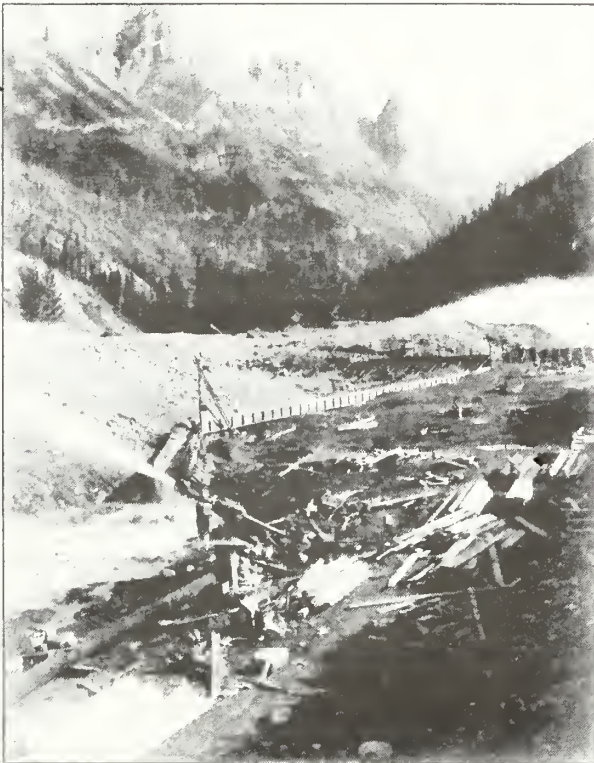
Figure 3.8. Hydraulic mining operations on Dan Creek in the Nizina District, circa 1916. Work by the Dan Creek Mining Company, seen in foreground, differed from conventional practice by eroding gravel banks in the same direction as bedrock drains and sluice boxes (outside of photo), yielding slight improvements to overall operational efficiency. Photo MR 16129, courtesy of University of Washington.
