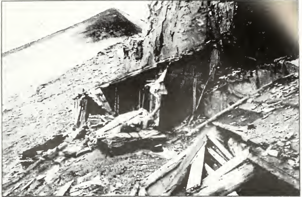
Figure 5.17. “Cliff House” at the Sheriff Mine. Much of the bunkhouse remains intact, although slides have damaged the later extension to the structure (compare with figure 4.22). The collapsed structure in the foreground is the site of the former blacksmith shop, later converted into a dry room. Photo by Will Updike. MTU #BL-8.24.97.
