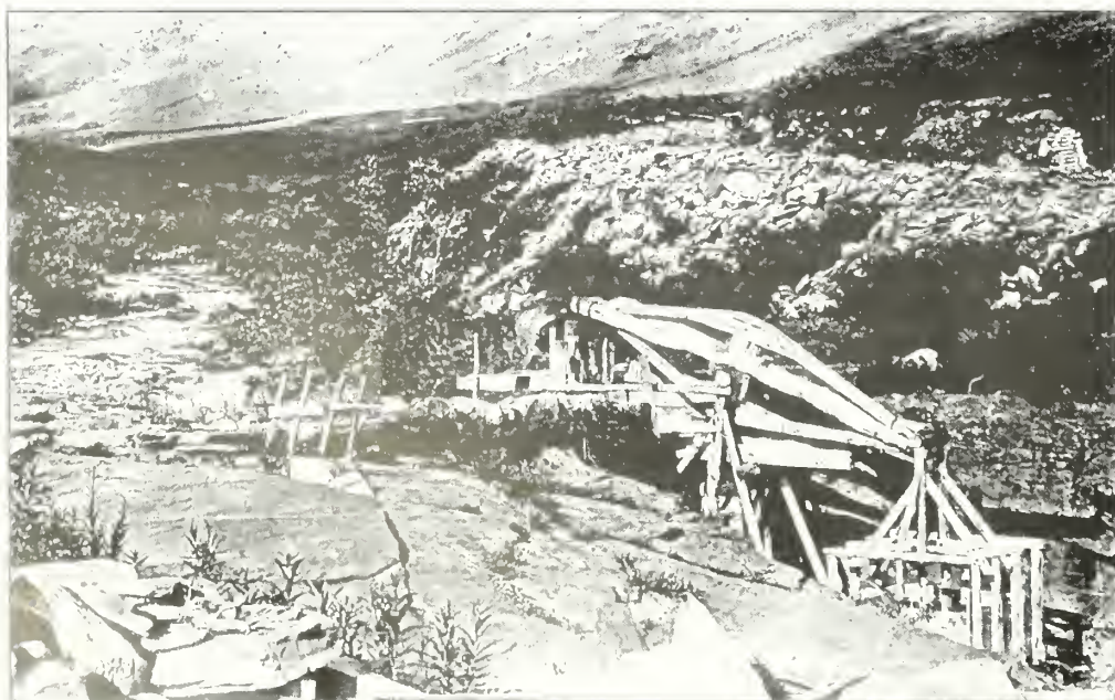
Figure 3.7. Boomer dam on Golconda Creek, circa 1911, looking northeast. A wooden flume (visible at center right) directed overflow into a bucket attached to the wooden arm on the downstream (right hand) side of the dam. When the bucket lowered, the arm raised up sluice gates, and the water "boom" aided the sorting of placer gravels. Note high bar deposits in background. Fred Mollit Collection, 509, United States Geological Survey.
