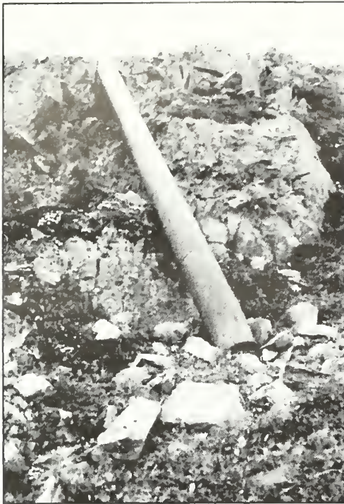
Figure 5.25. Remnants of the mill water supply system. The metal pipe (left) channeled water from a tributary stream into a shallow ditch, which transported water to settling tanks (right) located outside the No. 2 Adit. Photos by author, MTU #BL-4.1.98; #26978-4.
