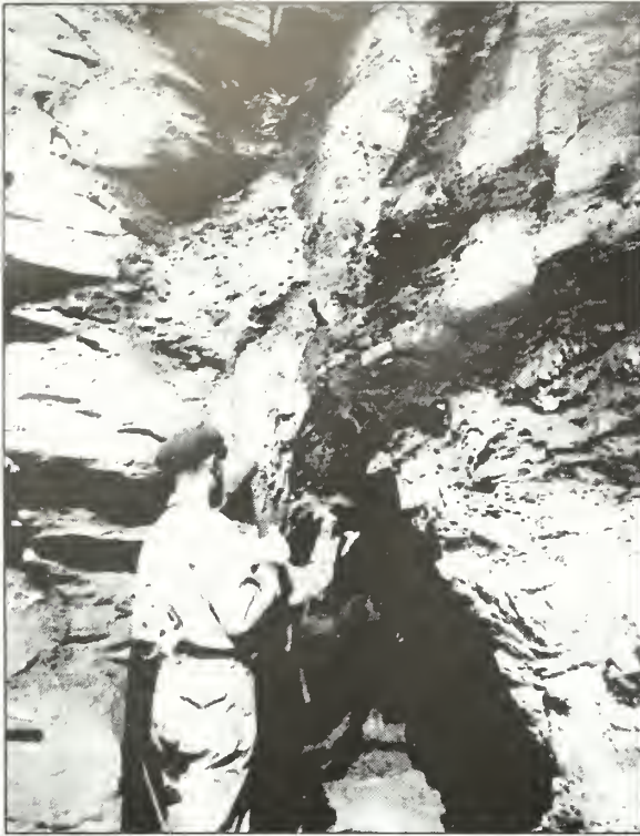
Figure 4.23. Drilling techniques employed on the No. 5 vein at the Sheriff Mine, circa 1938-39. Hand drilling (left) required two miners at the face, one to hold the drill, and the other to wield the sledgehammer. These tasks were regularly rotated to allow rest. The use of compressed air drills (right) greatly improved the speed and efficiency of operations, with only one miner having to operate the drill. Both photographs courtesy of Sylvia Baldwin.
