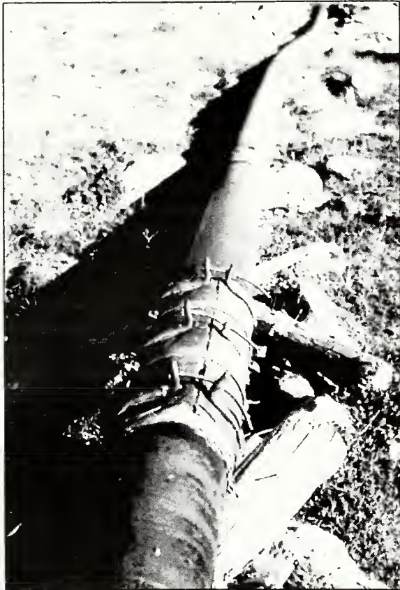
Figure 6.6. Minor equipment repairs were a frequent occurrence at the lode mines, and circulation systems were no exception. The conveyance of water from Falls/Power Creek was particularly essential to operations given the large reliance on hydroelectric power. Repair methods were not standardized, and a variety of materials and sealing techniques were employed. Photo by author. MTU #BL-2.14.97.
