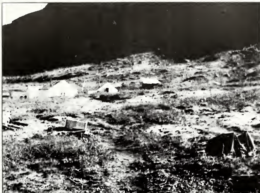
Figure 4.11. Yellow Band lower camp, circa 1938. The closest tent-frame in the picture may have served as the cookhouse. View looking northeast with wood storage area in left foreground. Photo courtesy of Sylvia Baldwin.
