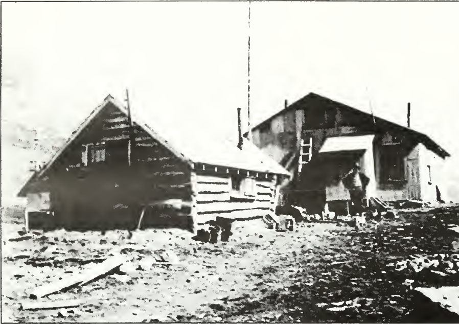
Figure 4.7. Bremner Gold Mining Company camp in the process of removal to a new site. The storage shed has already been moved. The log cabin in front of the bunkhouse was not shifted by Yellow Band Gold Mines Inc. to the new location—perhaps due to the instability of its foundations. Photo courtesy of Sylvia Baldwin.
