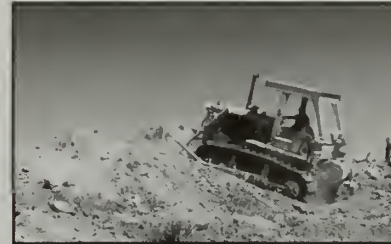
An Army Reserve bulldozer recontours the sandstone quarry at El Malpais National Monument
