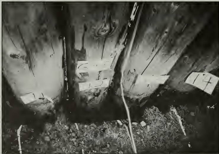
Figure 1. Vital Signs can mean many things in many different places. Here at Fort Vancouver National Historic Site in Vancouver, Washington, (destination of one of the conference field trips), being alert to vital signs that signal overall condition of a cultural treasure includes a periodic check for decay at the base of the fort's palisades wall. The palisades are cultural, but the decay agents are natural, so vital signs can overlap and bring together the cultural and natural elements of park management.
