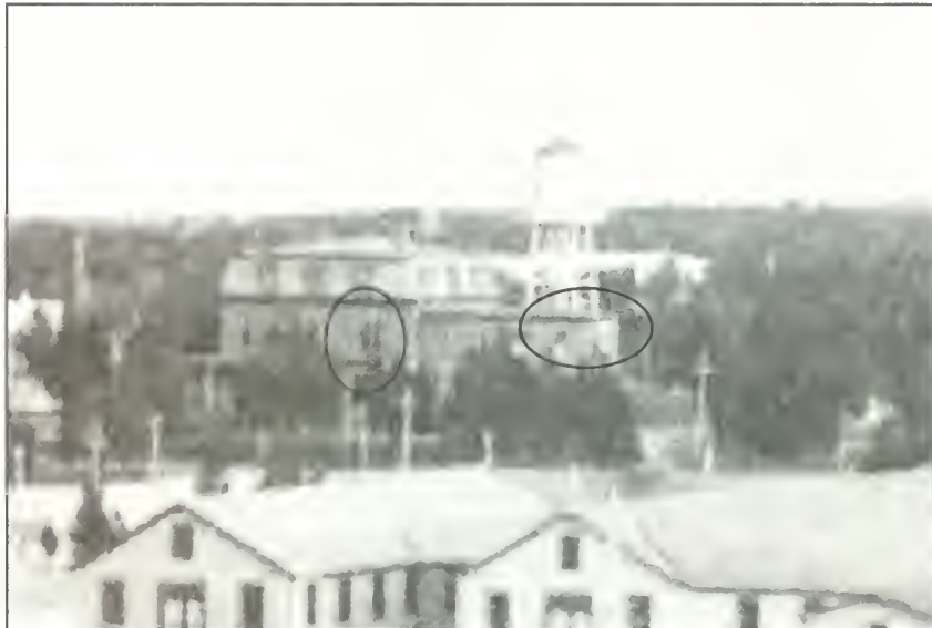
Figure 27. Officers Club, showing window openings, ca. 1904.
