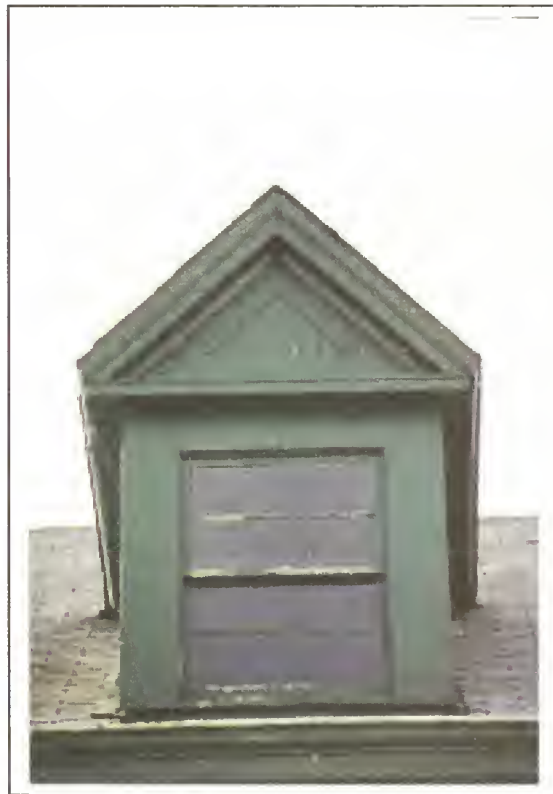
Figure 54. Officers Club, north elevation of rear ell, showing dormer of ca.- 1905 addition, 2005.
