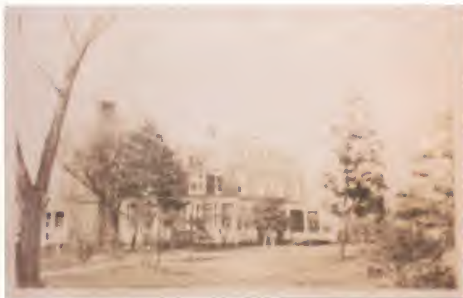
Figure 66. Officers Club, west and south elevations, ca. 1940; note enclosed porch.
