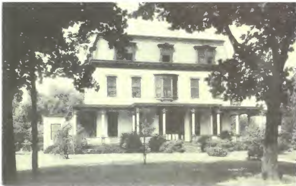
Figure 72. Officers Club, east facade, ca. 1941; note south- elevation addition and exterior paint colors.
