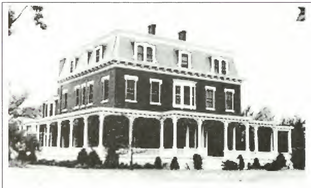
Figure 68. Officers Club, east façade and south elevation, ca. 1937.
