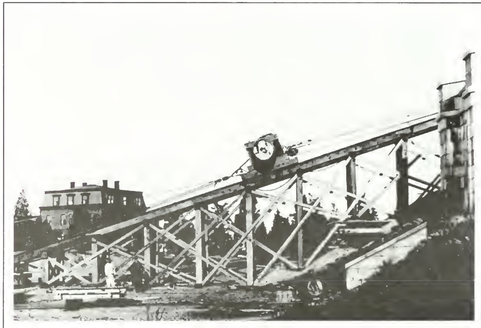
Figure 37. Construction of Battery Potter, looking northwest; Officers Club in background, ca. 1895.
