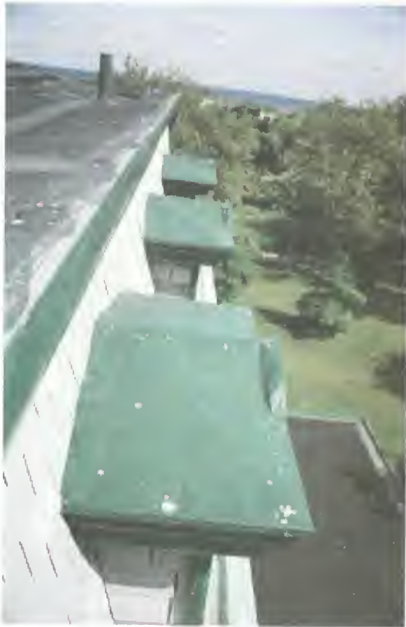
Figure 33. Officers Club, mansard roof, dormer roofing material, 1992.
