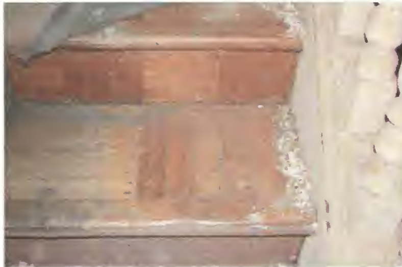
Figure 44. Officers Club, center hallway (Room 102), stairway, showing parquet pattern on treads and risers, 2005.
