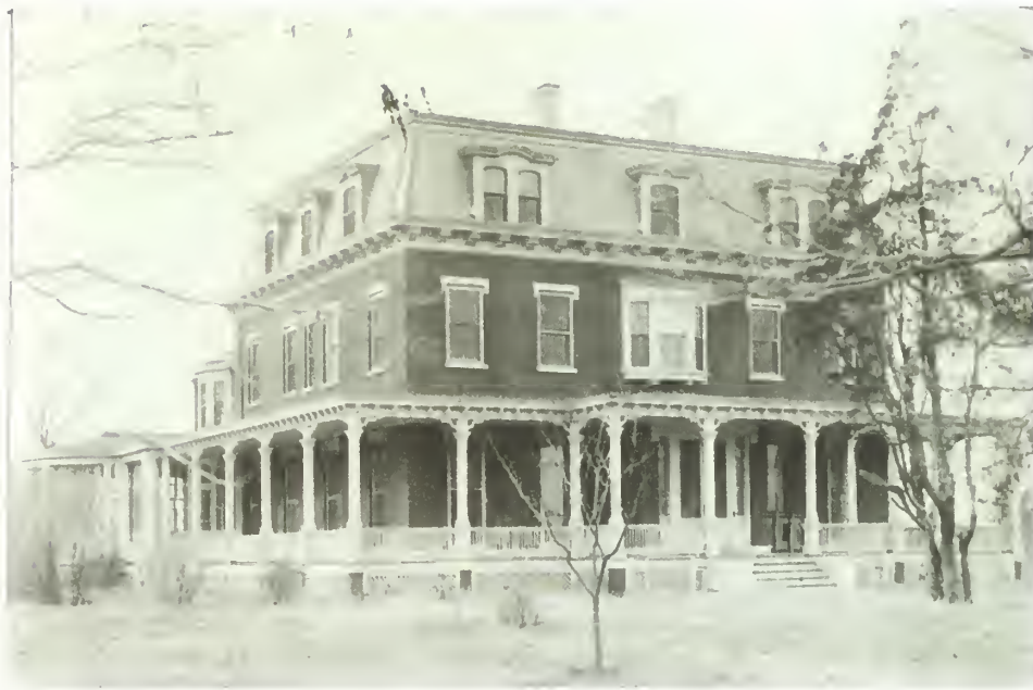
Figure 65. Officers Club, east façade and south elevation, "Feb 1922"; note enclosed porch.
