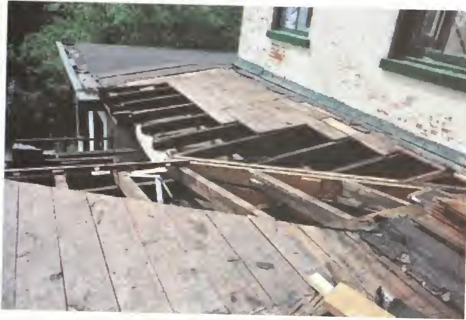
Figure 34. Officers Club, east façade, piazza roof, showing original framing and repairs, 1991.
