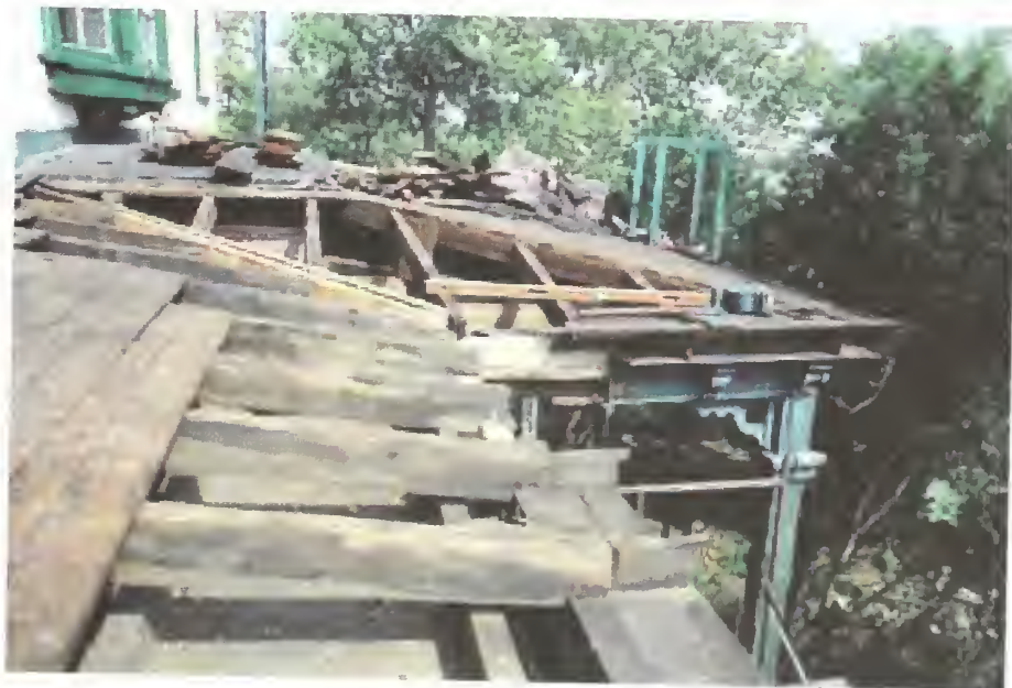
Figure 35. Officers Club, east facade, piazza roof, showing original framing with extended rafters for integral gutters.
