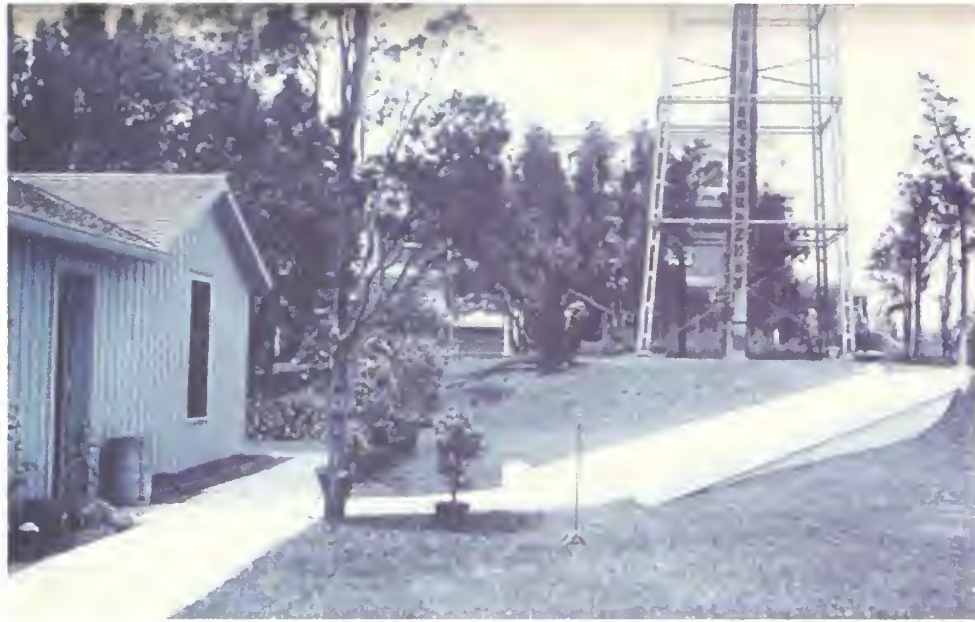
Figure 49. Sandy Hook Proving Ground, Greenhouse, with Officers Club in background, south elevation; note details of rounded porch.
