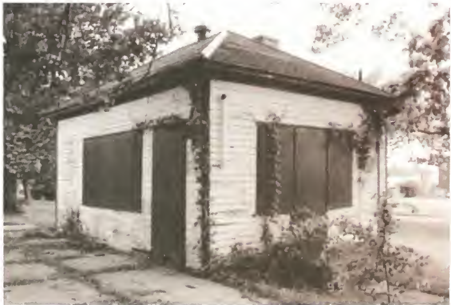
Figure 81. Laundry/Caddy House, Building No. 113, 1995.
