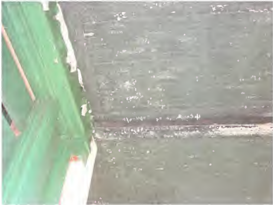
Figure 23. Officers Club, east façade , piazza ceiling, 2005.
