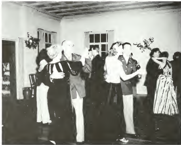
Figure 77. Officers Club, New Dining Room (Room 107), south and east walls; note doorway to Room 109 at left on east wall, 1944.
