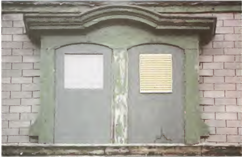
Figure 28. Officers Club, east elevation of mansard roof, showing dormer with paired windows, 2005.
