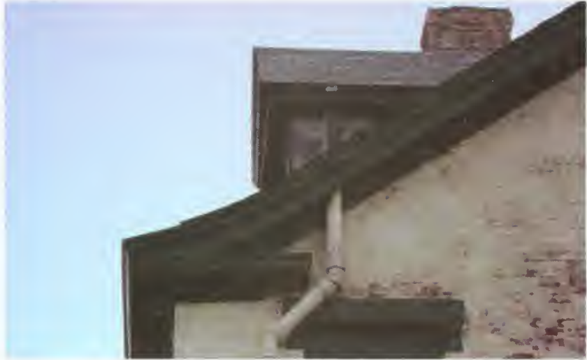
Figure 53. Officers Club, west elevation of rear ell, flared eave of ca.- 1905 addition, 2005.
