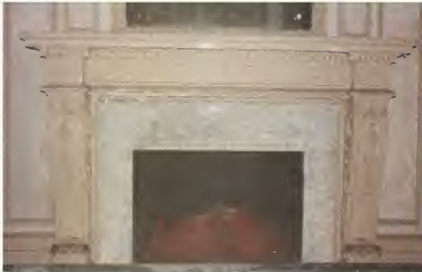
Figure 63. Officers Club, Lounge (Room 108), fireplace surround and mantelpiece, 2005.
