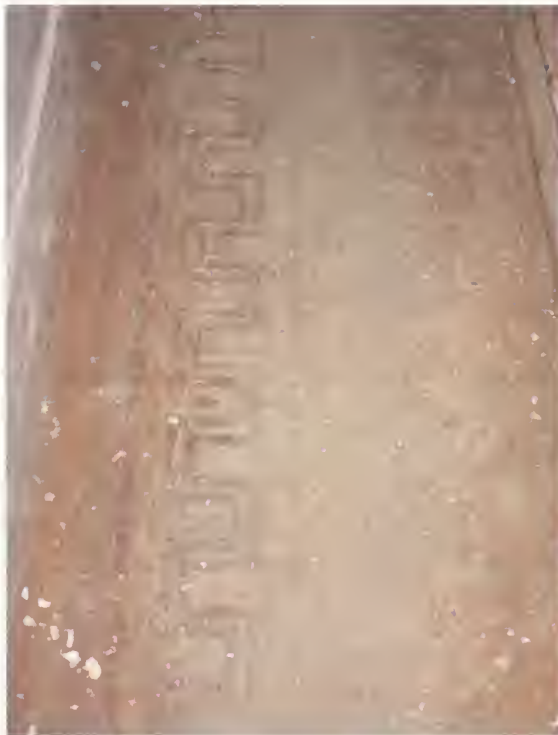
Figure 47. Officers Club, second- story center hallway (Room 201), parquetry floor, 2005.
