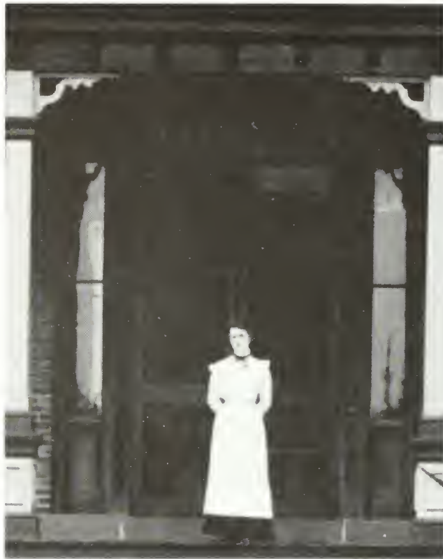
Figure 24. Officers Club, east façade, showing front entrance, ca. 1900.
