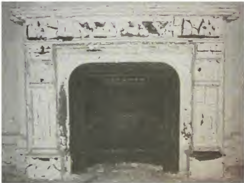
Figure 45. Officers Club, Ladies' Lounge (Room 103), south- wall fireplace, 2005.
