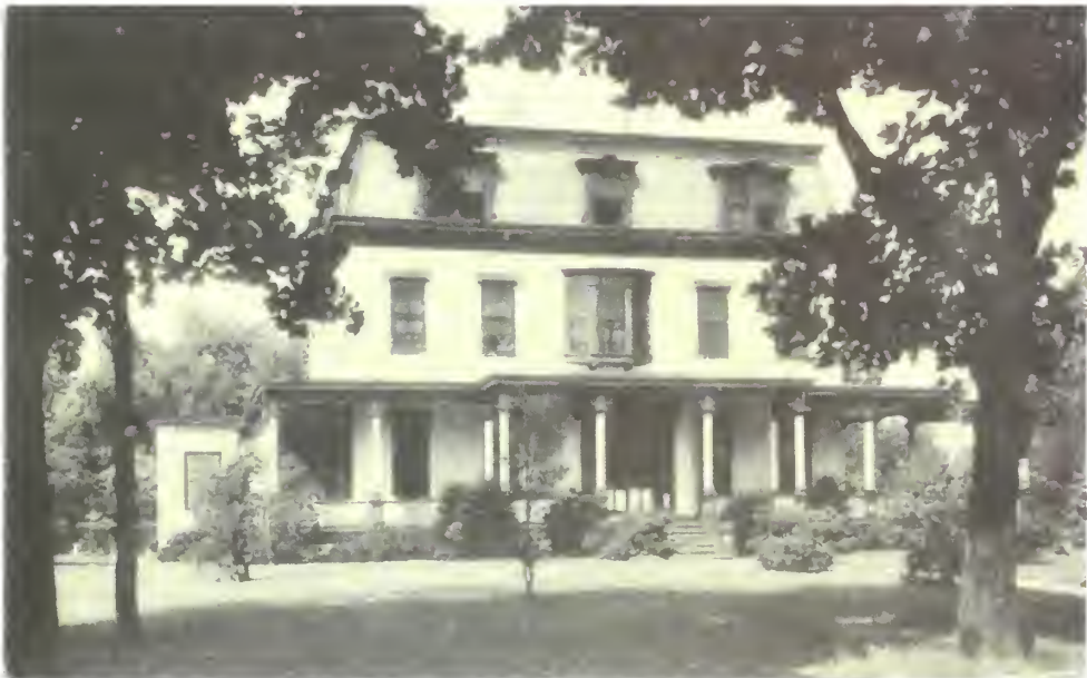
Figure 72. Officers Club, east facade, ca. 1941; note south- elevation addition and exterior paint colors.
