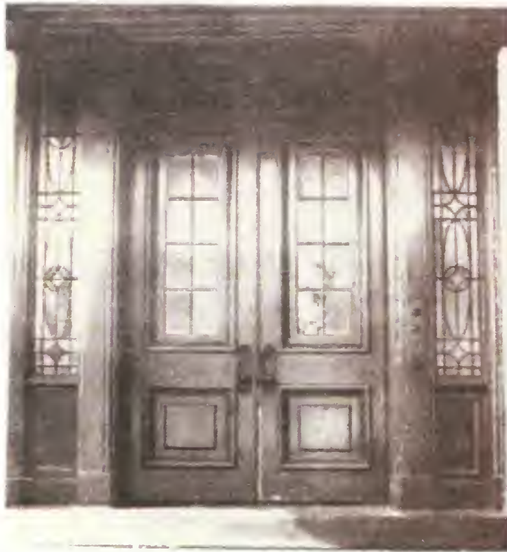
Figure 60. Officers Club. east- façade main entrance. Photograph taken after October 1979 and before June 1986.
