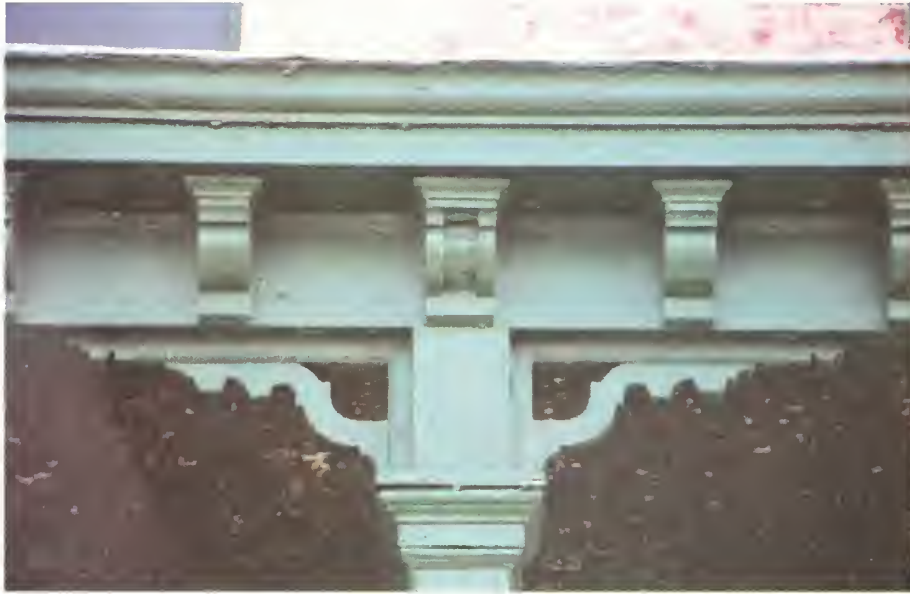
Figure 22. Officers Club, north elevation, piazza brackets, 2005.
