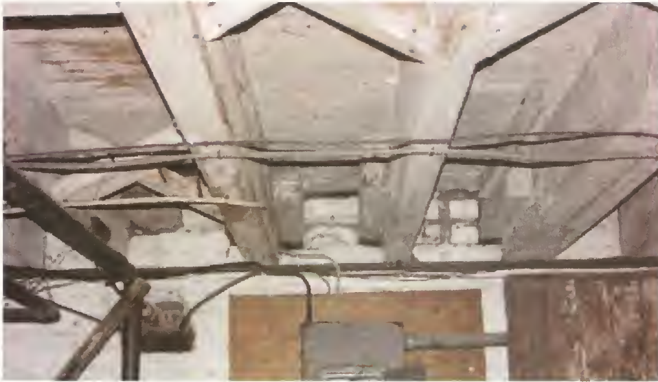
Figure 30. Officers Club, basement of rear ell, south wall, showing extant framing and brick infill that is evidence of earlier opening, 2005.
