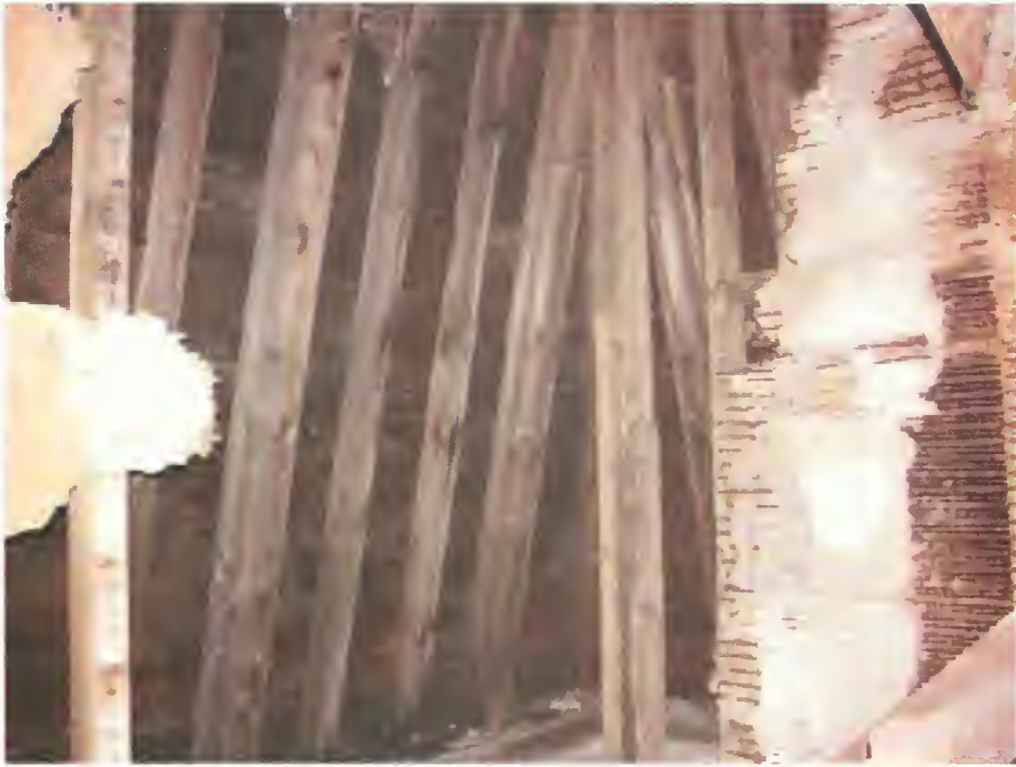
Figure 40. Officers Club, attic, showing framing of lower slope of mansard roof with alternating jack rafters, 2005.
