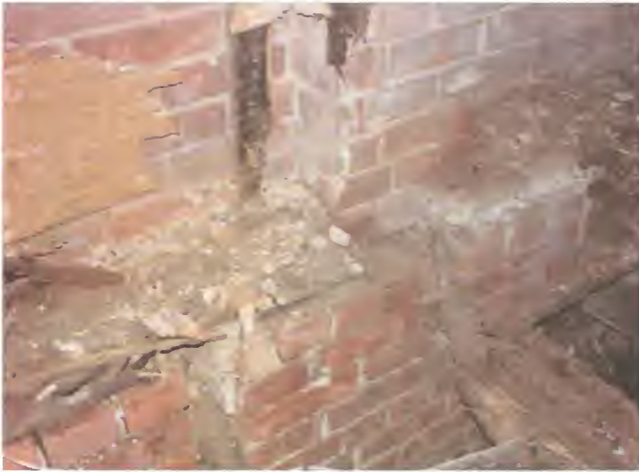
Figure 38. Officers Club, showing exterior bearing-wall construction at transition from first story to second story; also shows pockets in masonry for framing, 2005.
