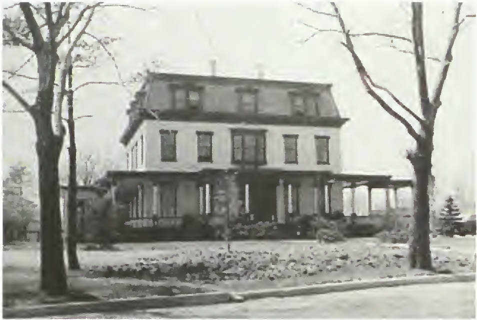
Figure 71. Officers Club, east facade, ca. 1940; note south- elevation addition and exterior paint color.
