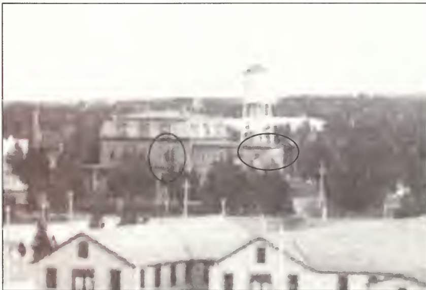
Figure 27. Officers Club, showing window openings, ca. 1904.
