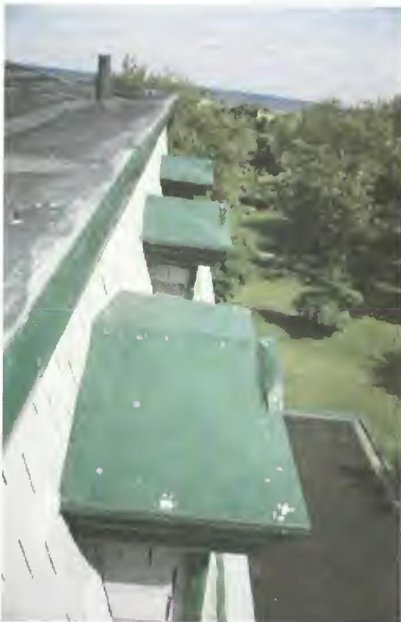
Figure 33. Officers Club, mansard roof, dormer roofing material, 1992.
