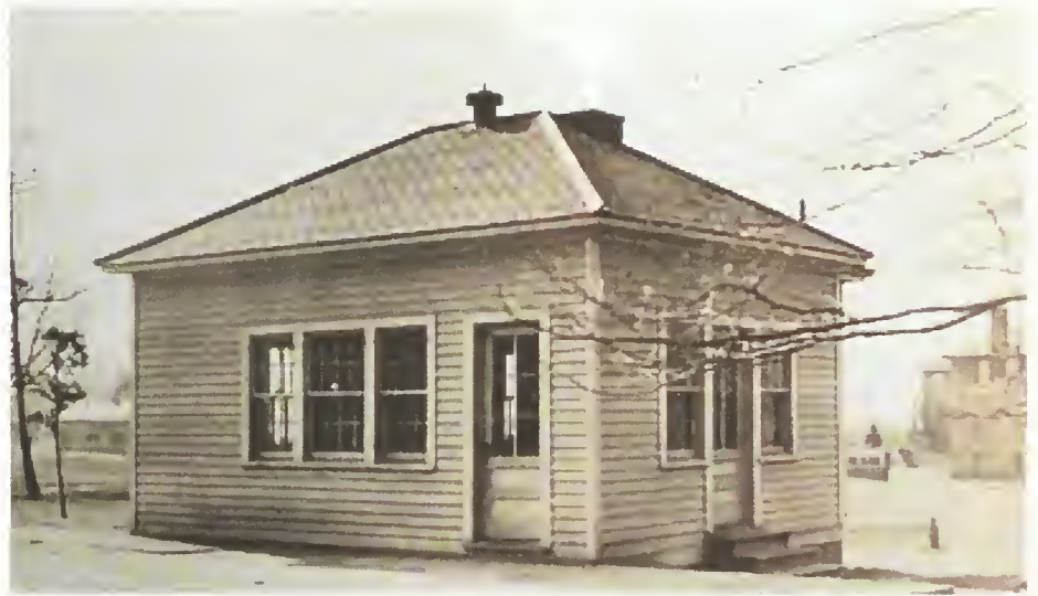
Figure 80. Laundry/Caddy House, Building No. 113, ca. 1940.
