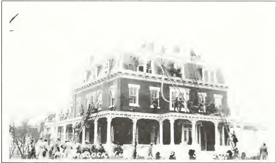
Figure 69. Officers Club, east façade and south elevation, April 9, 1938.
