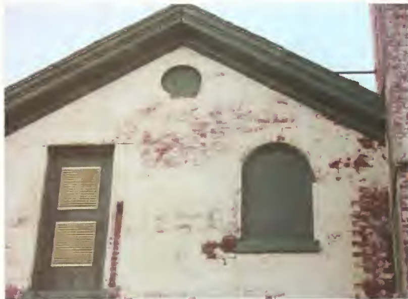
Figure 52. Officers Club, west elevation of rear ell, ca.- 1905 portion; shows oculus window (W311) and arched window (W312) in gable end, 2005.
