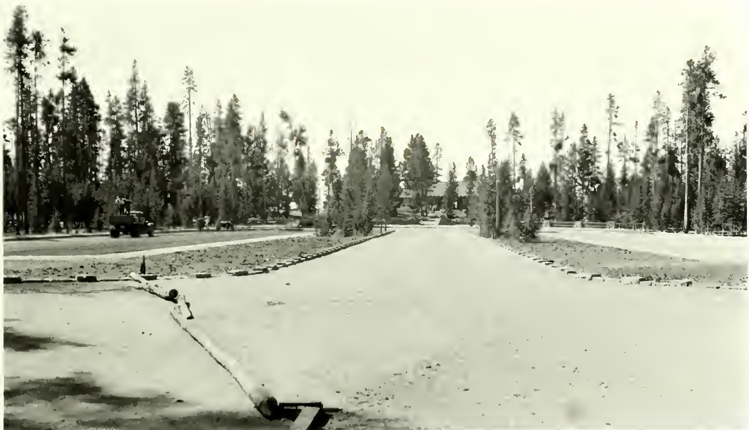
11305-4 Project F.P. 224.8 - Fishing Bridge Museum Street and Parking area nearing completion. Seal coat being applied August 29.
