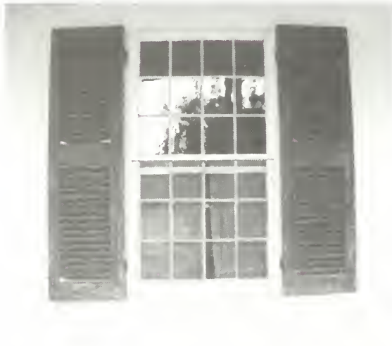
Figure 38 Typical 12/12, double-hung window with louvered shutters, c. 1835. (NPS-SERO-CRS, 2001)
