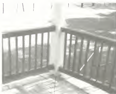
Figure 45 Typical gallery post, balustrades, and flooring. (NPS-SERO-CRS, 2001)
