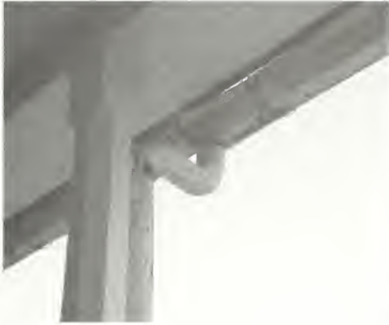
Figure 36 Typical semi-octagonal gutter and round downspouts, which date to early twentieth century. (NPS-SERO-CRS, 2001)
