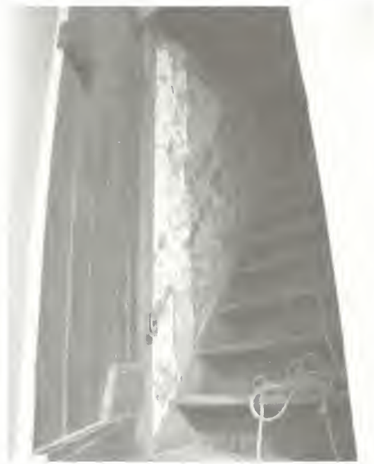
Figure 98 View of attic stairs where one of the early bousillage walls is still visible. (NPS-SERO-CRS, 2001)
