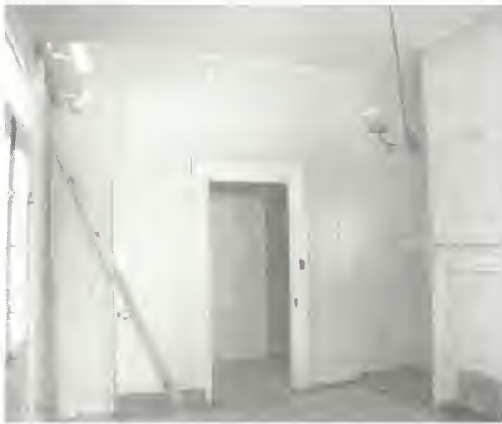
Figure 80 View south in Room 207 showing wall added c. 1880 to create central hall. (NPS-SERO-CRS, 2001)
