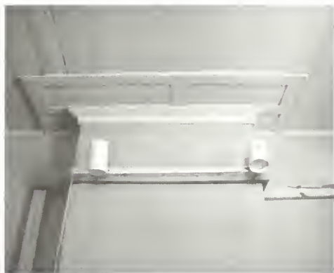
Figure 49 Board ceiling, typical of those found in most rooms on the main floor of the house. Paneling detail around chimney breast is typical of that found in 202, 205, 206, and 210, although molding details are different in each room. (NPS-SERO-CRS, 2001)
