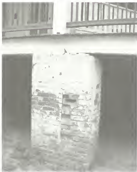
Figure 31 Brick piers on north end of east gallery. Pier at left is from the original house, c. 1821; pier at right is from the first expansion of the house, c. 1825. (NPS-SERO-CRS, 2001)
