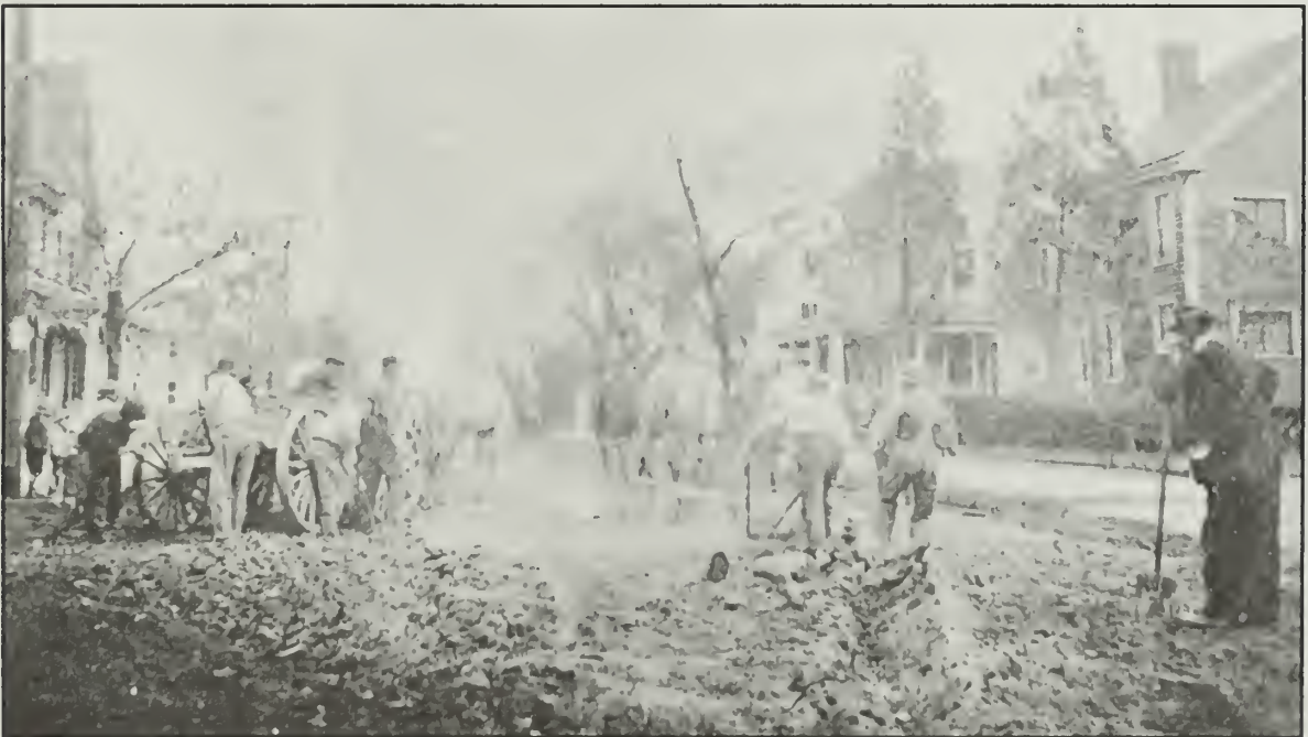
Figure 93. Working on the roadbed in Millville, Main Street/Route 49 at Fifth Street. Wettstein, 1915.
