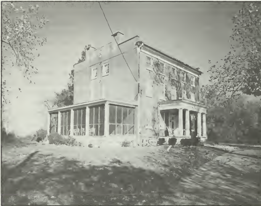
Figure 49. The Abbott Tide-Mill Farm House (1845), replaced the earlier John Denn home, part of which may be enclosed in this three-story Federal block.
