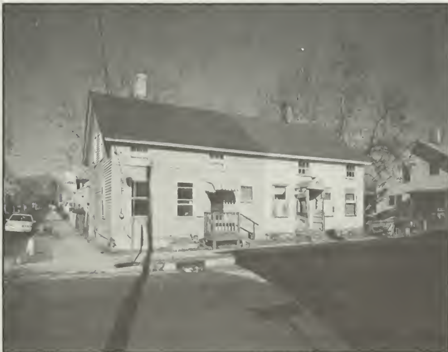
Figure 74. Many of the employees of Millville Manufacturing lived in worker housing. This example is located on Foundry Street in Millville.
