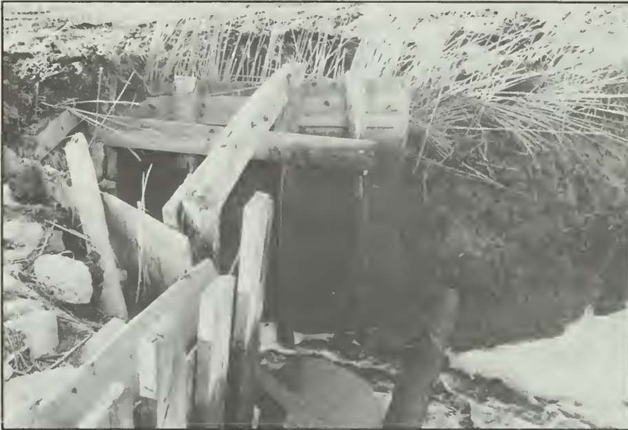
Figure 54. Sluice gates around a drain pipe let water escape from fields at low tide; as the tide rises, the gates press shut so as not to flood the fields. Sebald.
