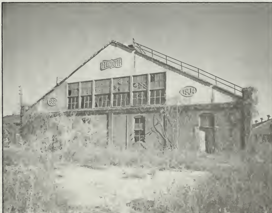
Figure 70. This largest of the Ferracute buildings is structurally sound, but the presses and other equipment have been removed.
