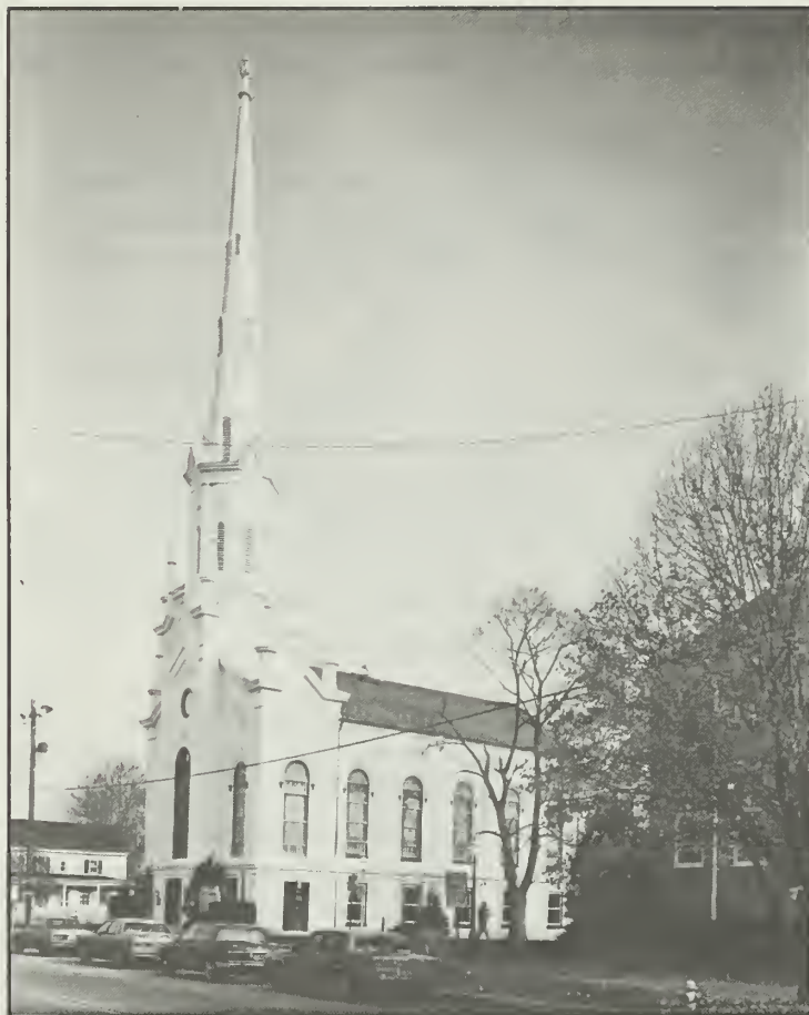
Figure 109. First Presbyterian Church (1856) facade has a projected entrance with a series of recessed facade and cornice lines, decorated steeple base and matching narthex-end walls.
