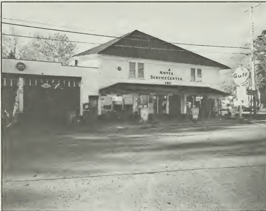
Figure 94. Noyes [Gulf] Service Station (ca. 1940). This typical rural station is shared with a general store and other roadside businesses; the storefront, gas pumps and service bay are modern.
