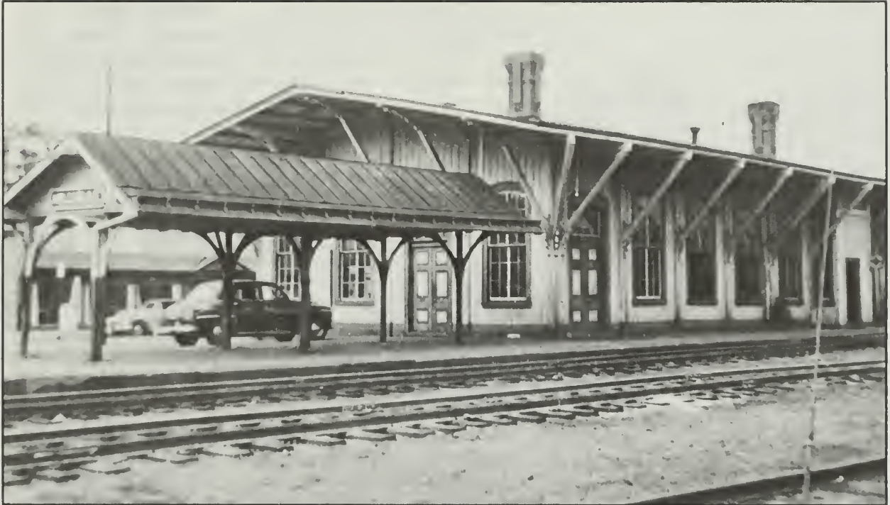
Figure 89. Pennsylvania-Reading Seashore Railroad Millville Station (ca. 1870). This depot with deep, braced eaves and large windows was at Broad and High streets. Wettstein, 1958.
