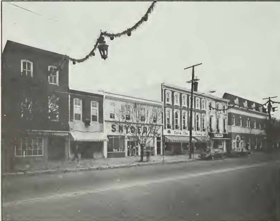
Figure 14. View of High Street, Millville.
