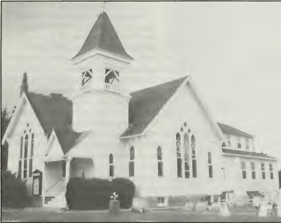
Figure 113. Goshen Methodist Church (ca. 1870). This church is an example of the irregular Victorian plan and abundant architectural texture. Leach.
