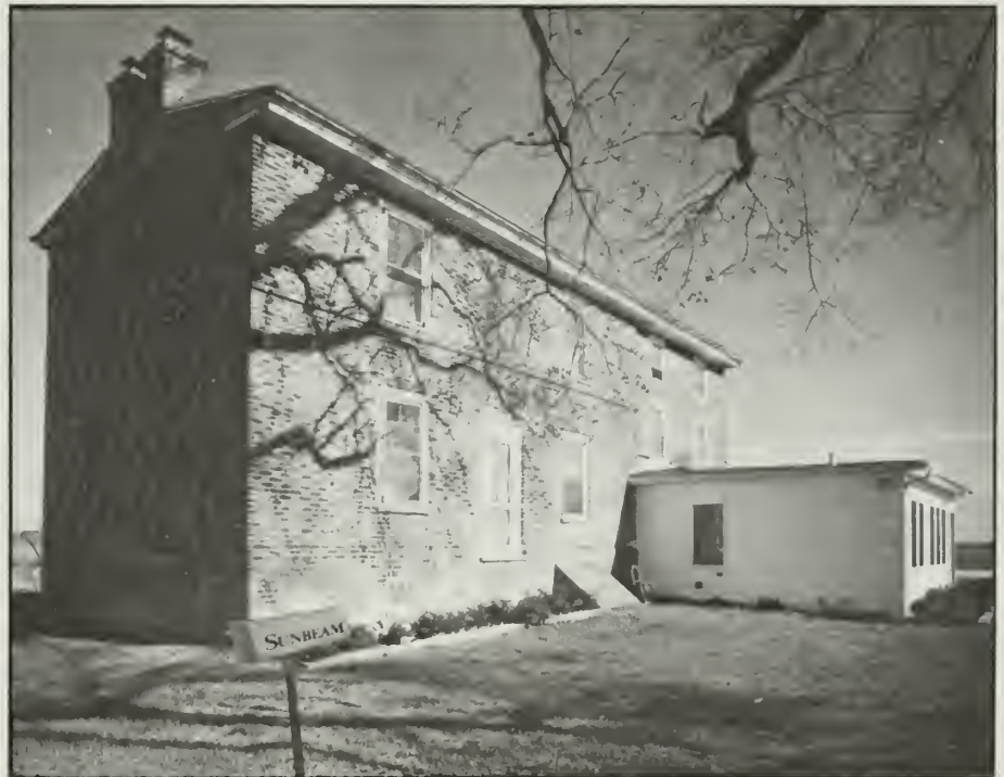
Figure 127. Nathaniel Chambliss House (1730), originally a three-bay block with zigzag pattern gable end, has two later additions.
