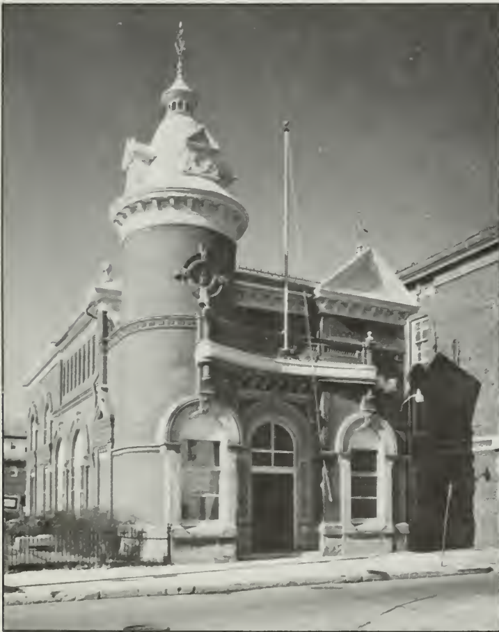
Figure 6. Salem Municipal Building (1899)--with contrasting red brick, stone, and white trim--is exemplary Queen Anne styling.
