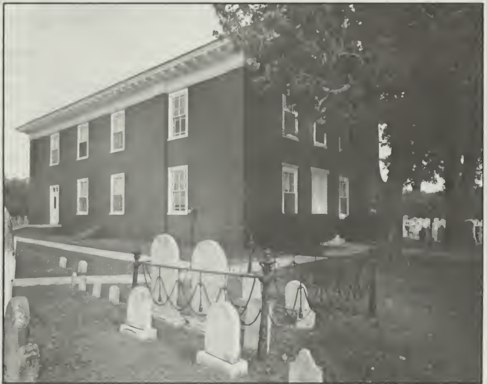
Figure 110. Cold Spring Presbyterian Church (1823, NJ-270). Two-story brick, with cornice and pediment with dentils. Three bays wide by four bays deep.
