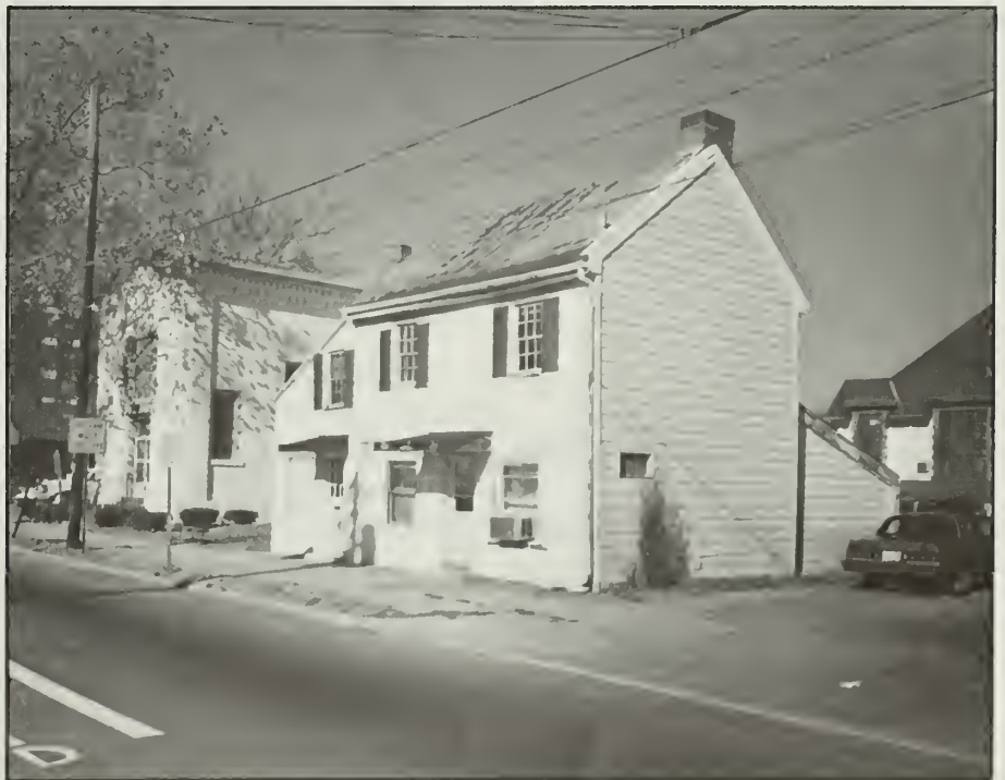
Figure 128. Typical stack house, Millville, showing the main "stacked" one-cell arrangement with shed units on the side and rear facades.
