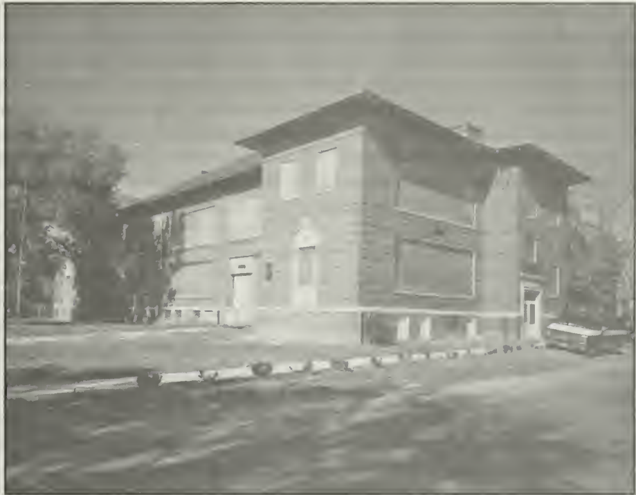
Figure 100. Vine Street School (1906). The two-story, H-plan building has a formal three-part brick facade with hipped roof and raised basement.
