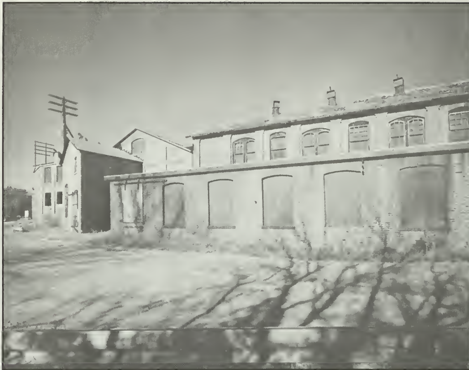
Figure 75. Now owned by Wheaton Industries, this complex of buildings includes the pump house once used by Millville Manufacturing Company.
