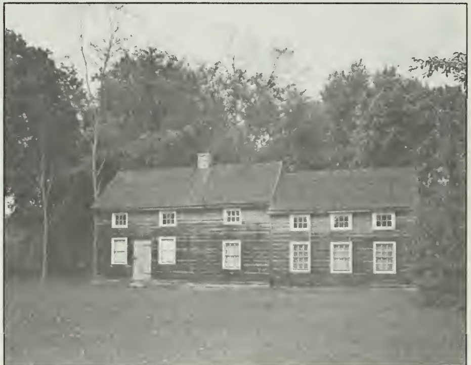
Figure 44. Thomas Ludlam House (1743), originally a hall-and-parlor plan, has been enlarged with the addition of four bays and relocated below Dennisville.
