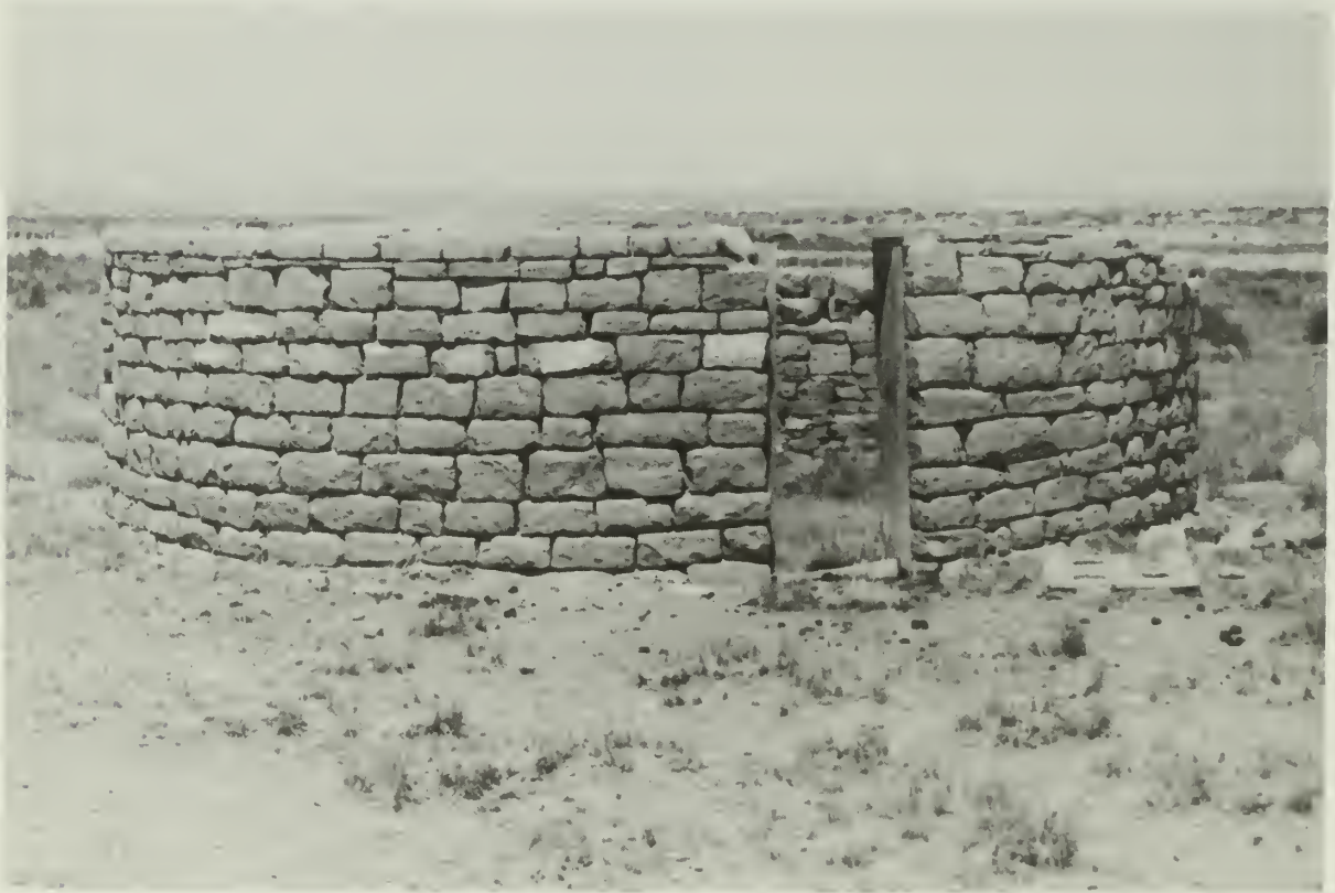
Hogan of dressed sandstone blocks, Site A13.
