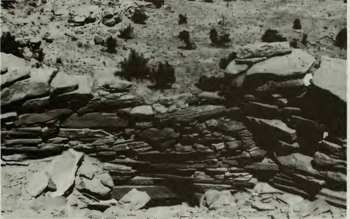
Parapet around roof of Room 1, Pueblito 1, Site K5. The hole in center foreground is for the chimney
