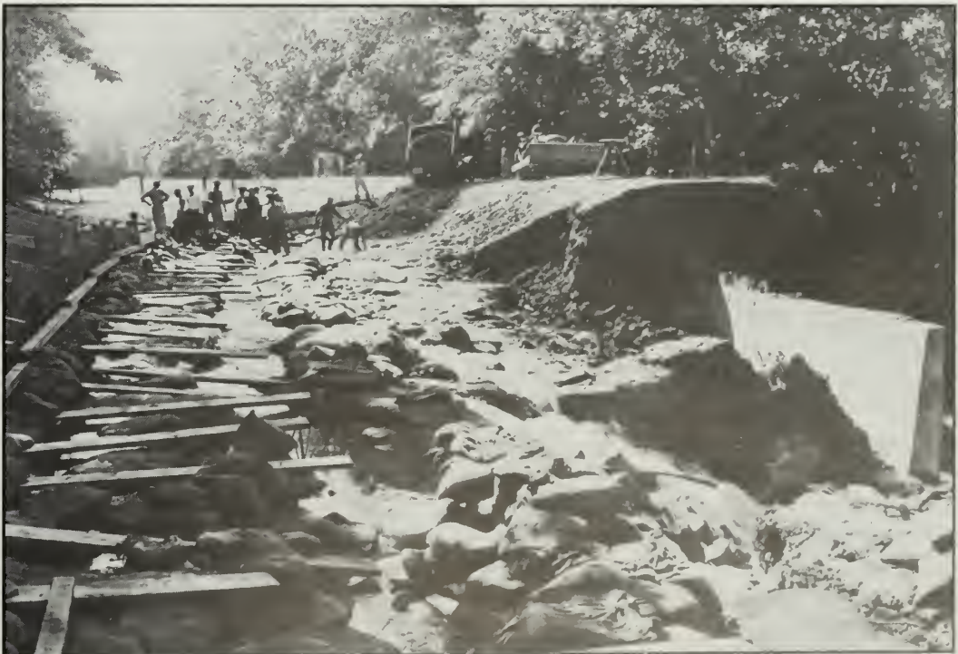
CCC reconstructs towpath at Widewater, July 9, 1941.
