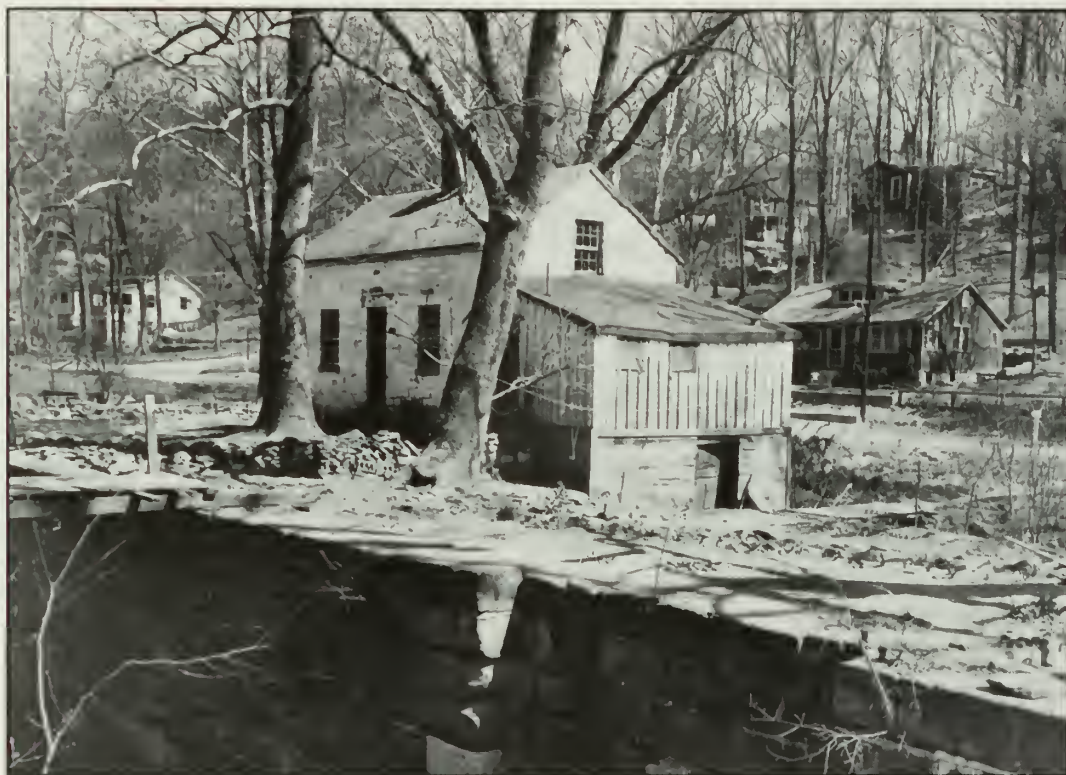
Lockhouse at Lock 6 before restoration.
