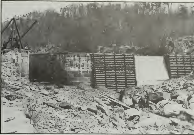
CCC reconstruction of Lock 15, April 4, 1940.
