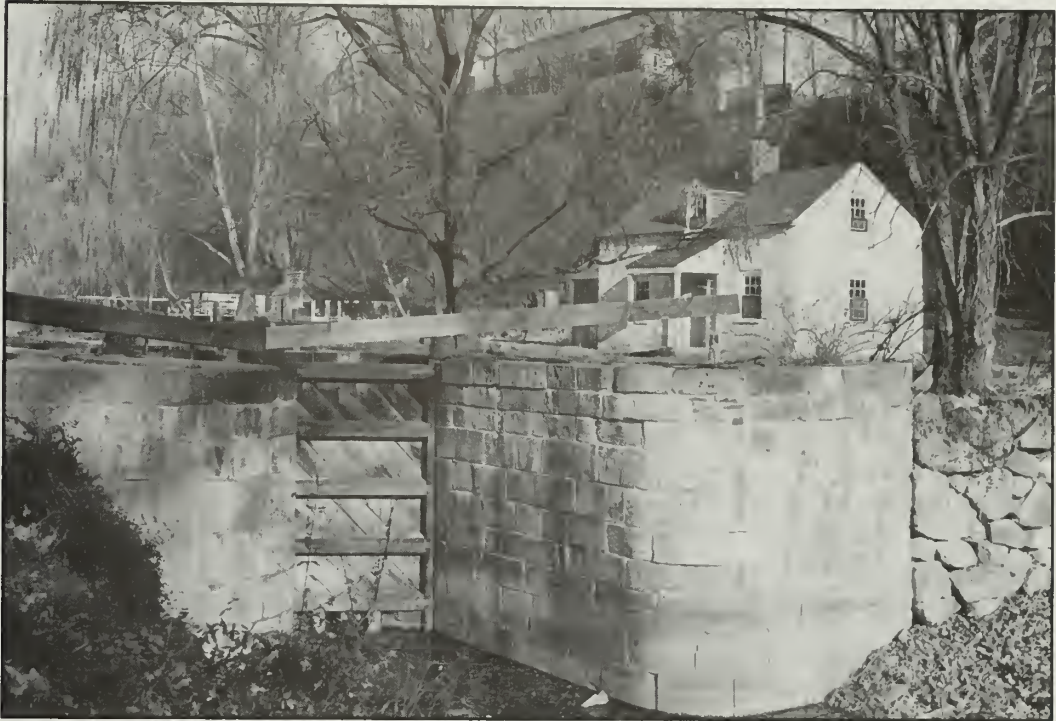
Lock 7 and lockhouse after restoration, 1943.
