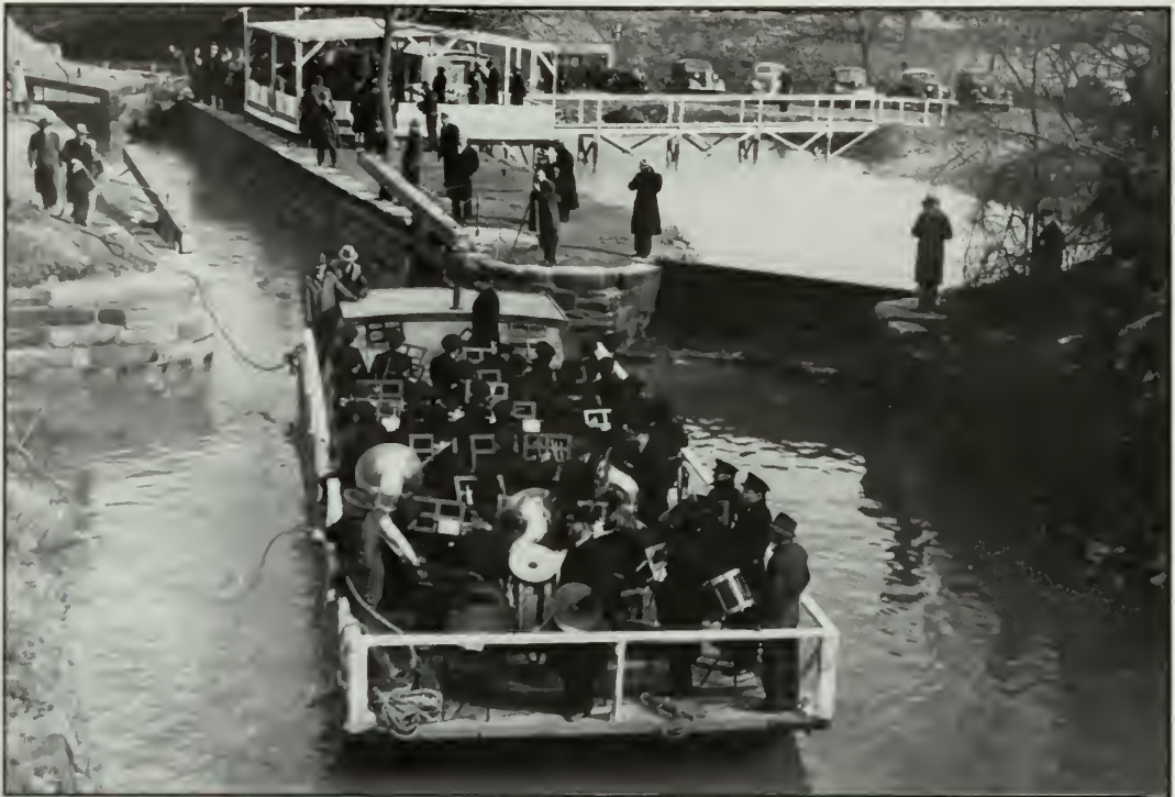
Ceremony at Lock 1, February 22, 1939. (GSA's West Heating Plant now occupies area to right of lock.)
