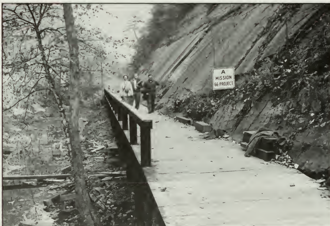
Restoration work below Paw Paw tunnel, 1956.
