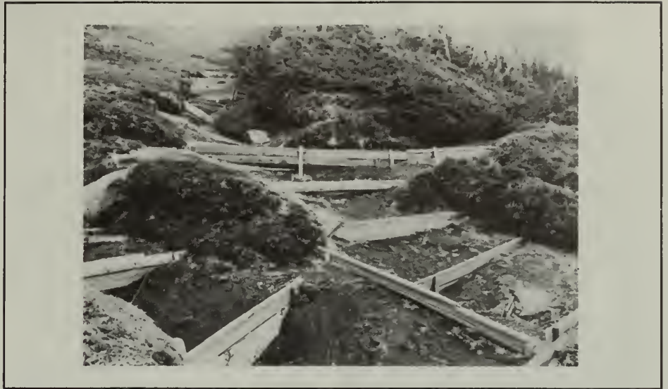
Impact sites are stabilized with silt bars, ready for filling and revegetation.
