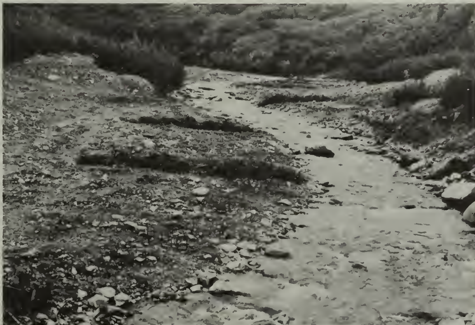
Feltleaf willow cuttings for revegetation are shown here, along with brush bars for floodplain stabilization on a reclaimed section of Glen Creek.
