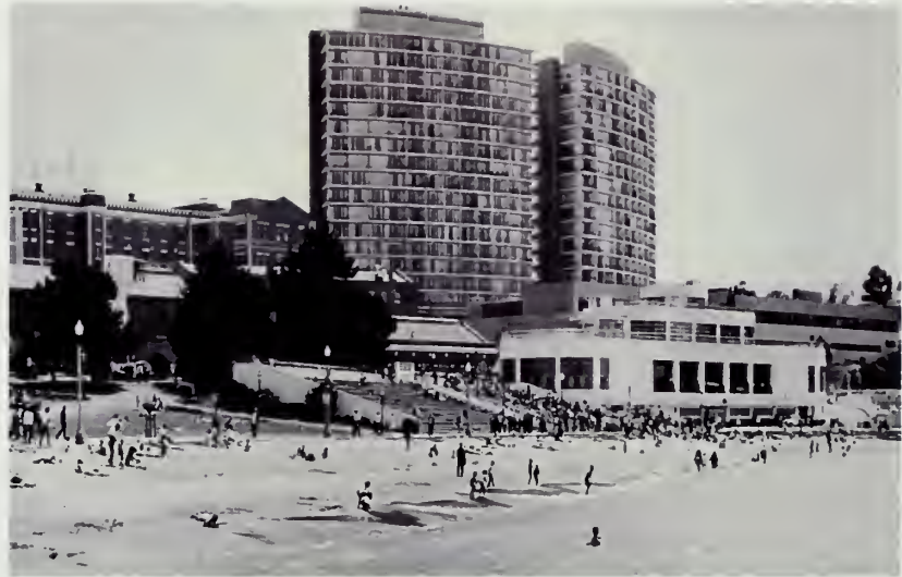
Figure 37 View of Aquatic Park, ca. late 1970s. View looking southwest. (San Francisco Maritime NHP, Historic Documents , A12.40, 891n)
