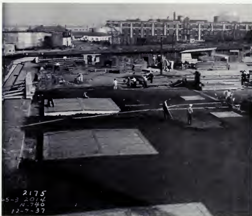
Figure 21. By December, 1937, finish grading around the skylights provided the level area needed for the establishment of turf grass and planting beds east of the Bathhouse. View looking east. ( San Francisco Maritime NHP, Historic Documents, Photograph Collection, P88-035.00102 )
