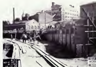
Figure 49. WPA photograph showing the retaining structures required prior to relocation of the State Belt Railroad tracks. ( San Francisco Maritime NHP, Historic Documents, Photograph Collection, SAFR-N-2-26 )
