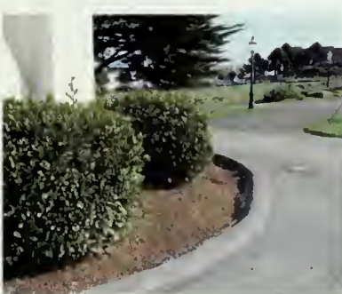
Figure 106 Raised asphalt curb around the East Speaker Tower planting bed. (NPS, 2008)
