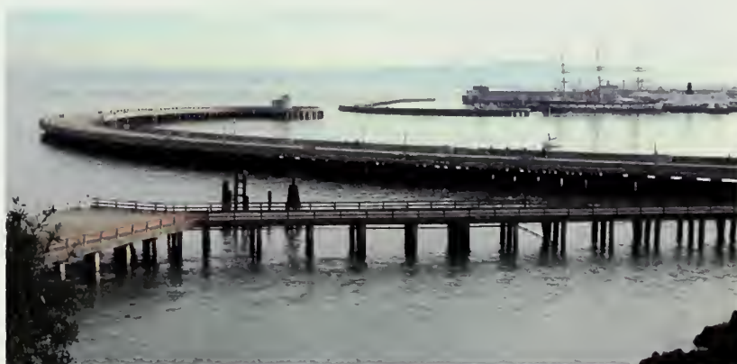
Figure 43. View to the Municipal Pier as it arcs around Aquatic Park Cove. Fort Mason Pier 4 in the foreground. View looking northeast. (NPS, 2007)
