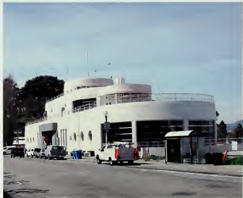
Figure 53 The Bathhouse today, view looking west. (NPS, 2010)
