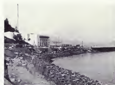
Figure 9 Large amounts of debris and rubble dumped along the shoreline of the cove were used to construct a crude seawall. ( San Francisco Maritime NHP, Historic Documents, Photograph Collection, P88-035.00033 )
