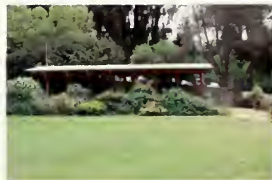
Figure 44 View of the overhead structure covering the Bocce Ball Courts located in the southwest corner of the park. (NPS, 2007)
