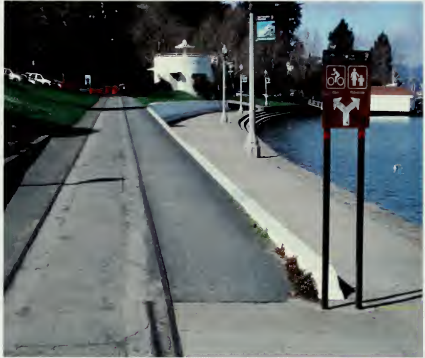
Figure 102. In most cases the separation between bicycles routed on the upper walkway and tracks (left) and pedestrians along the shoreline on the Beach Promenade helps mitigate potential pedestrian/bicycle conflicts. Over the years, asphalt paving and patching around the tracks has created uneven surfaces and in some cases, presents safety hazards. This view looking west. (NPS, 2005)
