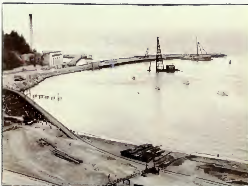
Figure 10 Municipal Pier under construction in 1932. Note the realigned State Belt Railroad trestle in the foreground. ( Courtesy of the San Francisco History Center, San Francisco Public Library, AAC 2288 )
