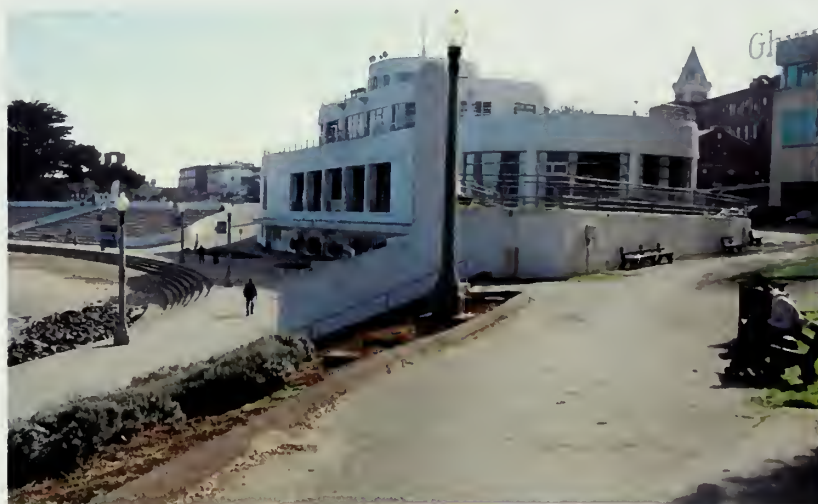
Figure 104 View of the Upper Promenade showing the rolled curb along the edge of the walkway and planting bed (left), and the patching and expansion of paving leaving a relatively undefined edge on the right side. (NPS, 2006)
