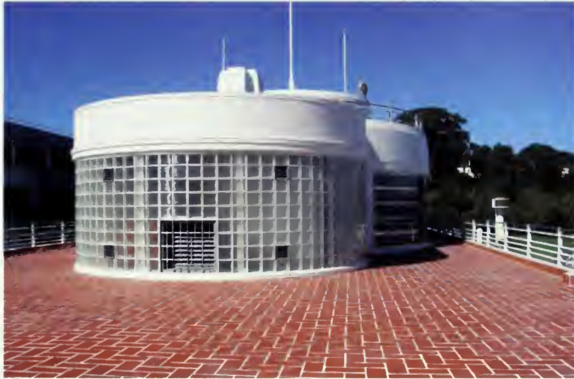
Figure 55 Rehabilitation work at the Bathhouse in 2008 included the installation of a new stainless steel window system; and a modern waterproofing system for the building roofs with new roof tiles to match the historic ones that could not be salvaged. The rehabilitated glass block pantry is now the elevator lobby on the 3rd floor. (NPS, 2008)
