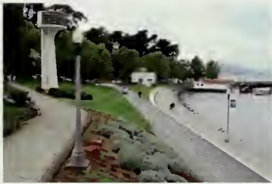
Figure 71. View of three components of the pedestrian circulation system in Aquatic Park. The Beach Promenade along the shoreline, the State Belt Railroad tracks (asphalt), and a portion of the Upper Promenade as it passes the West Speaker Tower. (NPS, 2008)
