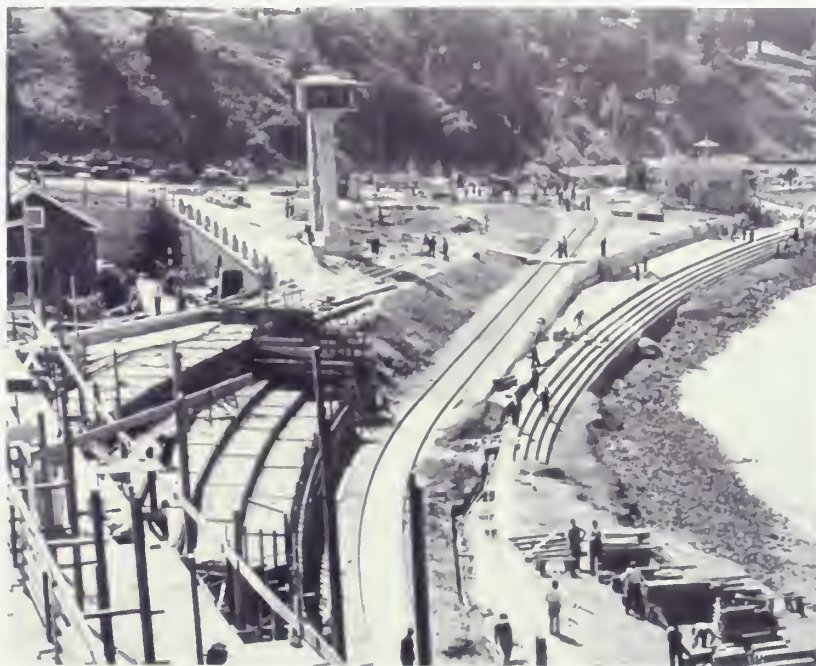
Figure 50 Detail of WPA photograph showing the number of topographic modifications to the slope around the cove that were part of the site design and construction of Aquatic Park, 1938 ( San Francisco Maritime NHP, Historic Documents, Photograph Collection, P88-035.00139 )
