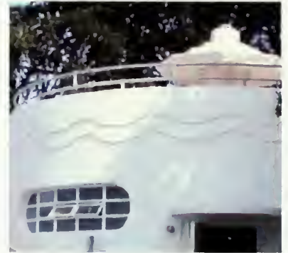
Figure 14 Architectural details such as wavy lines, metal railings, and nautical-style windows are characteristic of the Streamlined Moderne style expressed in the structures and grounds at Aquatic Park. (NPS, 2008)
