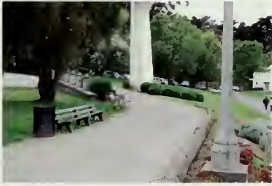
Figure 101. Rolled asphalt curbing along the Upper Promenade. View looking west. (NPS, 2008)
