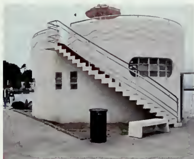
Figure 59 East Convenience Station. View looking west. (NPS, 2007)
