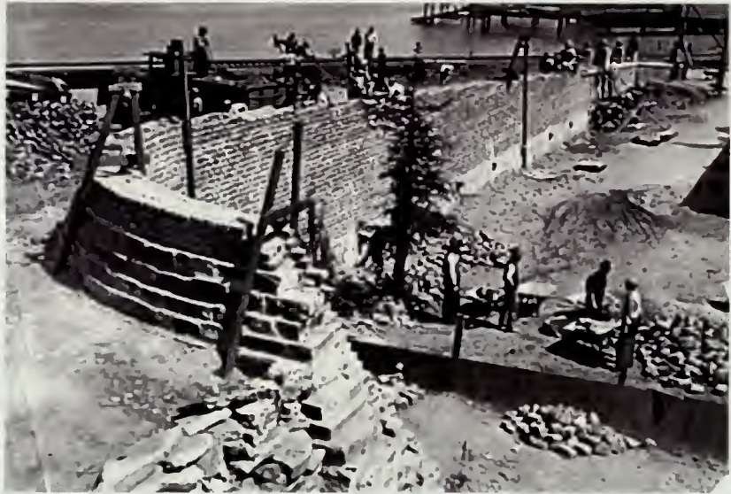
Figures 66. Constructed in 1936, the stone masonry retaining wall located on the west end of the park, was a significant structure, stepping down from the highest point near Van Ness Avenue. View looking east. (Courtesy of the San Francisco History Center, San Francisco Public Library AAA 6725)
