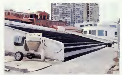
Figure 90 View of the East Bleachers showing new waterproofing material applied during rehabilitation. Note mildew on the concrete wall. Cleaning and repainting this portion of the structure is important to the character of the structure, and should be integrated into overall maintenance. (NPS, 2009)
