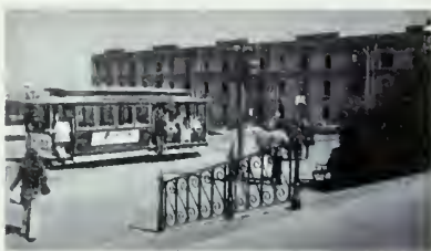
Figure 36 View of Victorian Park and the cable car turn around before the tracks were realigned. ( San Francisco Maritime NHP, Historic Documents, Karl Kortum Collection )
