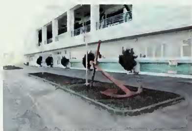
Figure 120. View of the existing juniper plants on the north side of the Bathhouse. View looking south east. (NPS, 2008)
