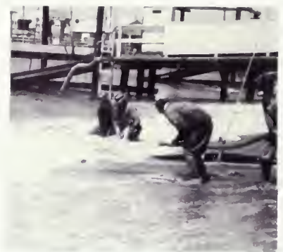
Figure 26 Agitating with hoses to redistribute sand and replenish the beach, 1939. (Courtesy of the San Francisco History Center, San Francisco Public Library, AAA 6708)
