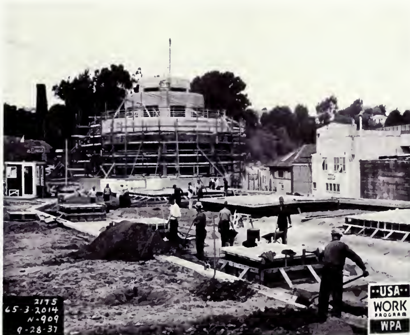
Figure 20. Site work and rough grading east of the Bathhouse moved quickly through the fall of 1937. View looking west. ( San Francisco Maritime NHP, Historic Documents, Photograph Collection, P88-035.00087 )
