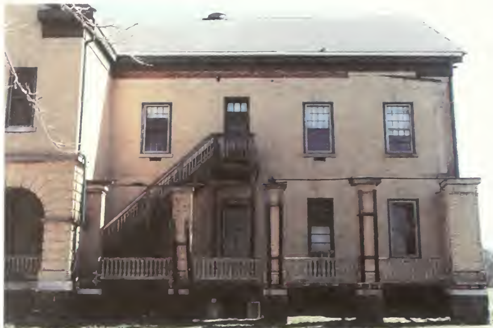
Figure 74. West elevation, showing replacement box cornice and fire escape.
