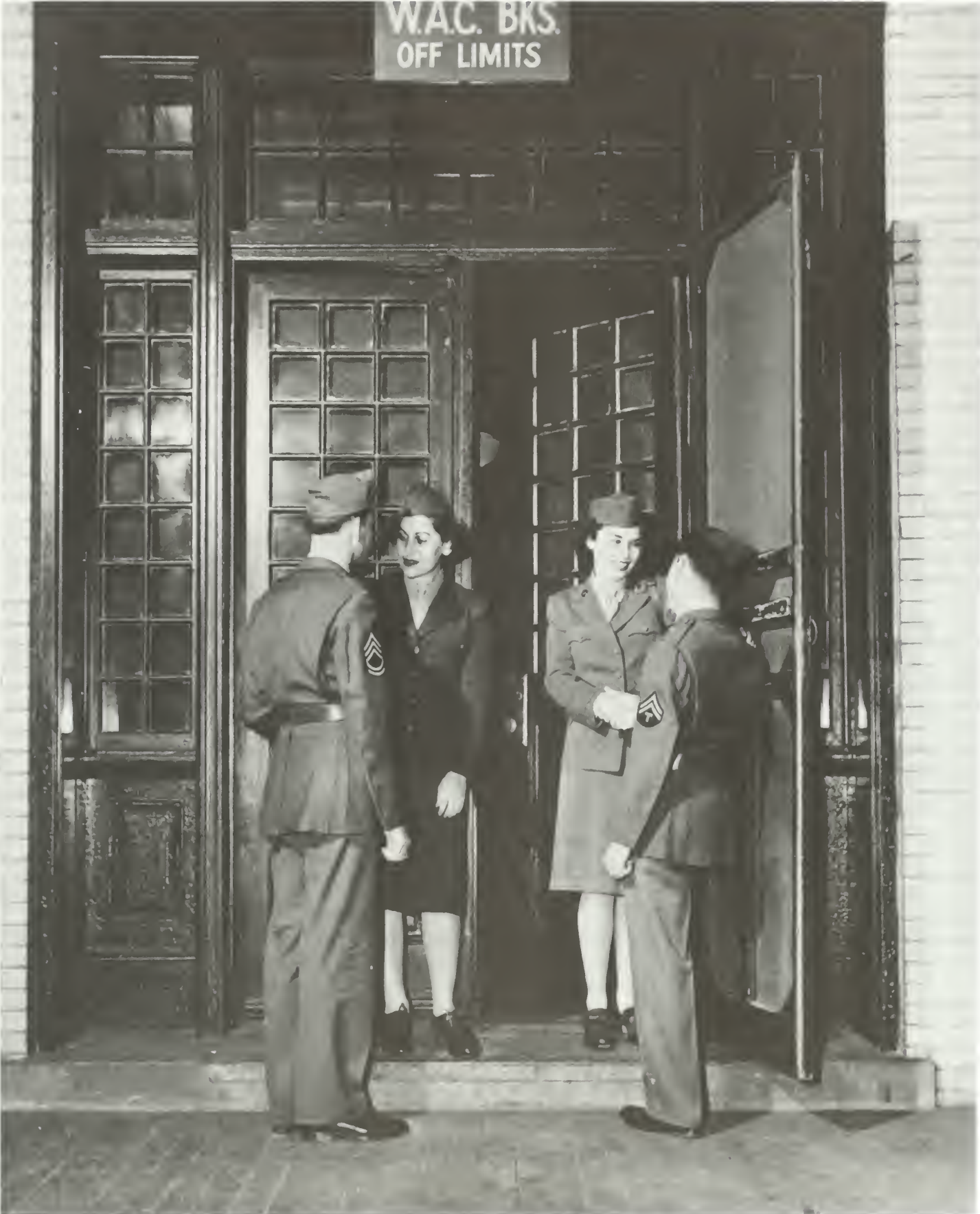
Figure 49. Members of the Women's Army Corps and their escorts, 1943-45. Photograph shows front doorway of Building 25.
