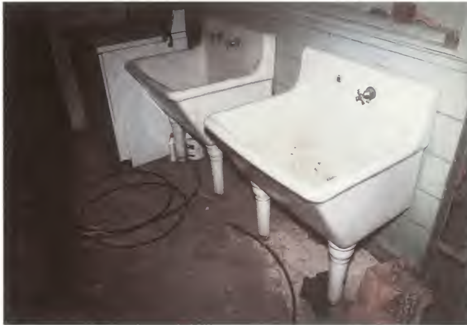
Figure 76. North side of basement, partition and laundry sinks in northeast corner.
