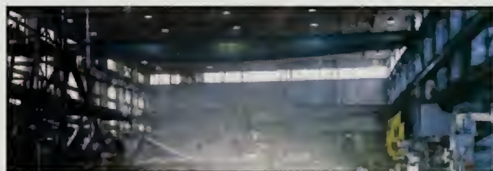
BRIDGE CRANE — Bridge cranes served most of the industrial buildings in the Navy Yard, allowing heavy materials to be moved throughout the length and width of their central bays. This pair of 5-ton capacity cranes is in the Structural Shop in the Building 104 Extension. Note how they are on different levels so they can pass each other. BOSTS-15920
