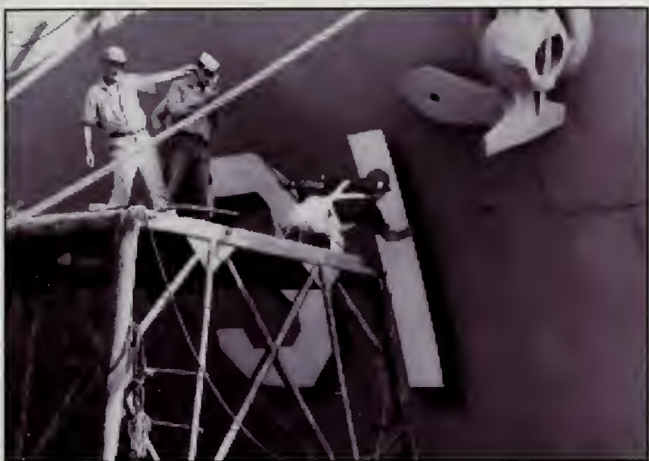
HULL NUMBER, FLOAT — Yard painters use a float as they paint the new hull number on the bow of USS Decatur (DDG-31) as her 1965-67 conversion to a guided missile destroyer nears completion. BOSTS-10895
