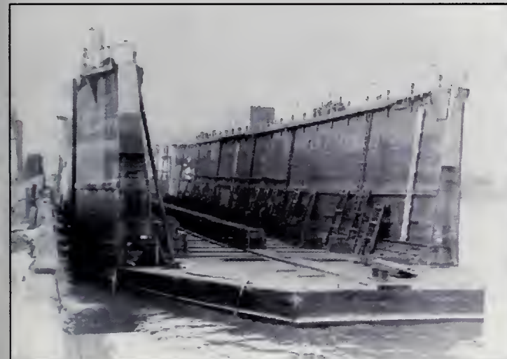
FLOATING DRY DOCK (YFD) — Floating dry docks provided the ability to service ships in locations where permanent dry docks were unavailable. During World War II, the Navy acquired numerous wooden dry docks such as YFD-24 . Capable of lifting ships up to destroyers in size, this was one of two floating docks assigned to the South Boston Annex to free up the facility's permanent docks for larger vessels. BOSTS-14960
