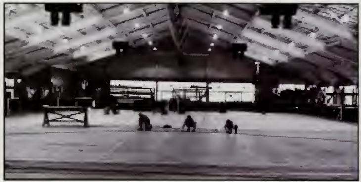
MOLD LOFT — The yard's final Mold Loft was on the upper level of the east extension of Building 104. In this photograph taken in late Dec. 1954 or early Jan. 1955, workers are laying out faring lines for hull sections of USS Suffolk County (LST-1173). BOSTS-14317
