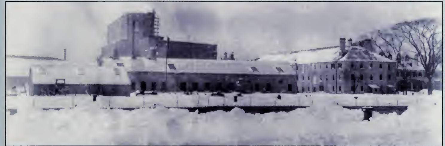
This view looks west across the Dry Dock. From left to right are the Boat House (Building 94); the Foundry (Building 16); the Store House (Building 5), then housing a variety of activities including the pay office, dispensary, labor board, museum, and paint shop; and Quarters B-F. Rising above the roof of the Foundry are the Hoosac Docks Grain Elevator and Hoosac Stores No. 1 & 2. BOSTS-14957
