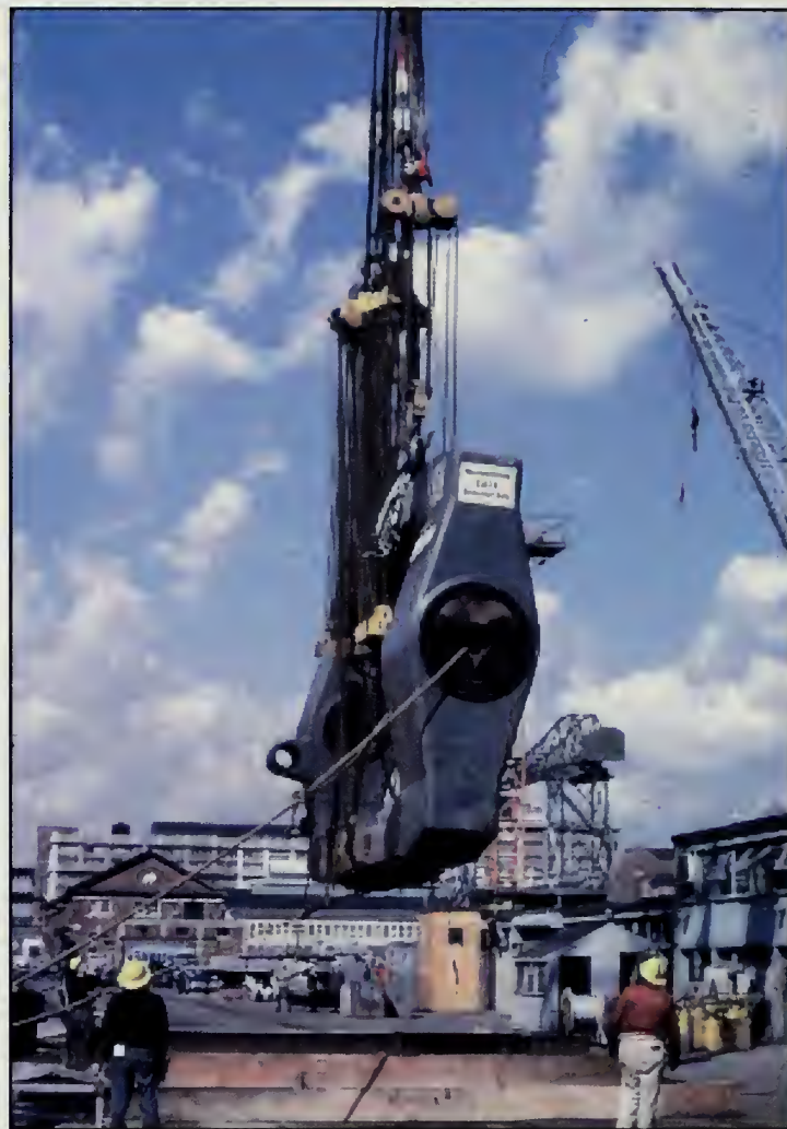
The Navy Yard possessed unique capabilities which it provided on a reimbursable basis to private industry. On Oct. 11, 1966, the yard's floating crane YD-196 was hired by the Wyman Gordon Co. of Worcester, Mass., to unload a 133-ton casting from the Dutch freighter MV Schiedyk onto a special railroad car. Here, the casting is being lifted from the deck of YD-196 at Pier 7. BOSTS-16197
