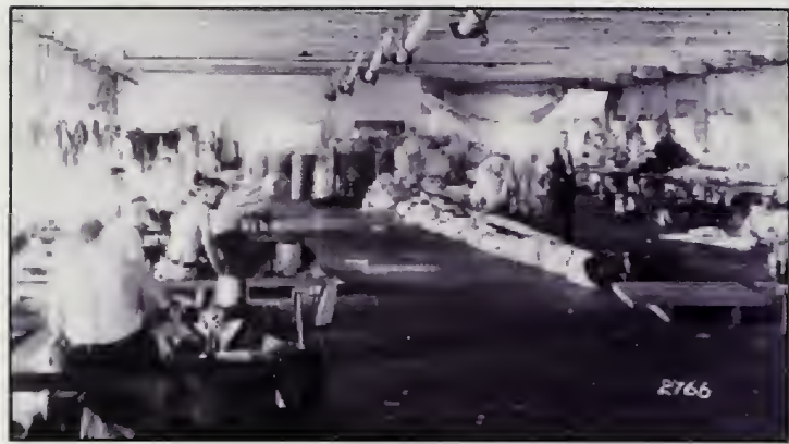
SAIL LOFT, YARD — The Navy Yard's Sail Loft in Building 33 is seen in this photograph taken around August 1917. Note the suspended yards which allowed sails to be hung. BOSTS-9333
