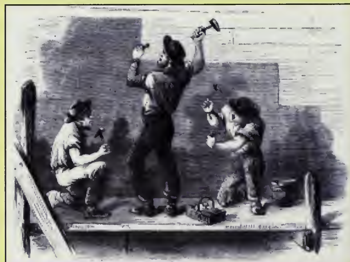
COPPERSMITH — Coppersmiths in the 19th century, in addition to making articles of copper for use onboard ships, performed the vital task of covering the underwater hull of vessels with copper sheets. Mystic Seaport
