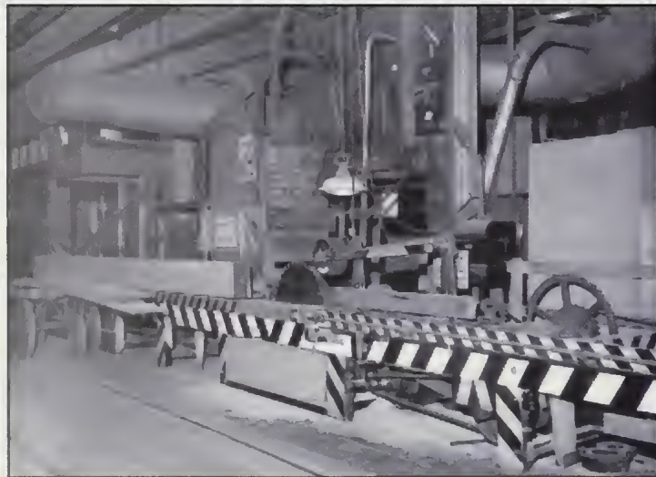
SAWMILL — Even in the age of steel ships, the Navy Yard needed a large sawmill to support its operations, in particular the manufacture of small boats. This Oct. 1949 view shows the rip saw located in the sawmill wing of Building 114. BOSTS-9836
