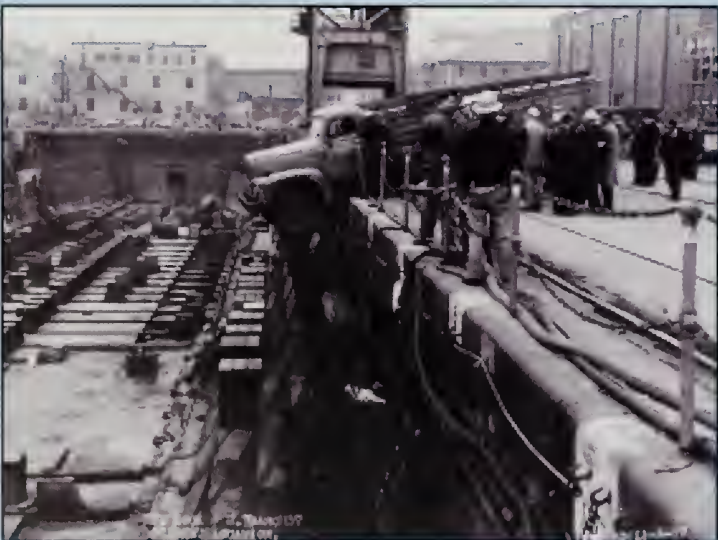
Yard photographers were called out to document accidents which happened in the yard. Image 863-57 was taken on Mar. 7, 1957, after Navy stakebody truck 97-07924 went through the railing surrounding Dry Dock 2. BOSTS-15698
