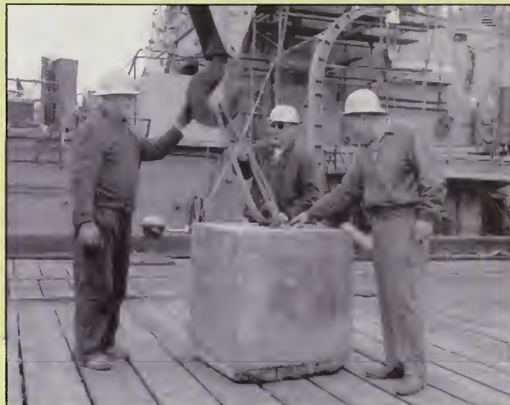
RIGGER — The term "rigger" encompassed more than one occupation. While the term is most often associated with the individuals who fabricate items out of rope, it also applied to men who were involved in the operation of cranes and other heavy lifting equipment. Here Foreman (Leadingman) Rigger Horace Grosshandler (center) supervises Riggers Jacob K. Mulley (left) and John Carr in lifting a 5-ton test weight onto the destroyer USS Fiske (DD-842) in Dec. 1967. BOSTS-7740
