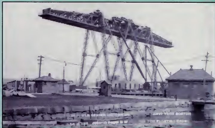
Floating Derrick No. 21 (YD-21)
