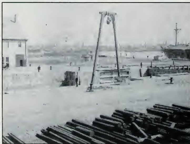
SHEARS — Resembling an A-frame, shears (or shear legs) were used for lifting heavy items using block and tackle prior to the development of mobile cranes. This shears was located near the outer end of Dry Dock 1.
