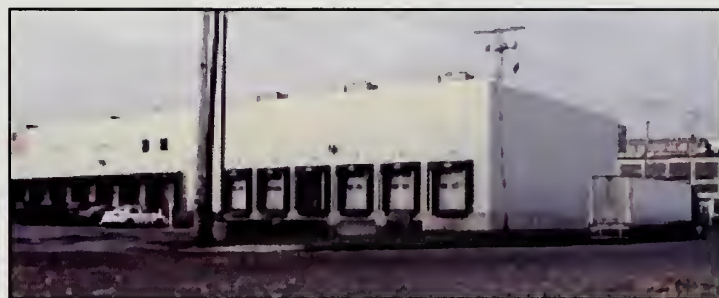
This Oct. 31, 2009, view shows the addition at the northeast corner of Building 2 of the New Boston Seafood Center. The structure was constructed by F. J. O'Hara & Sons, who already owned two of the three units in the facility.
