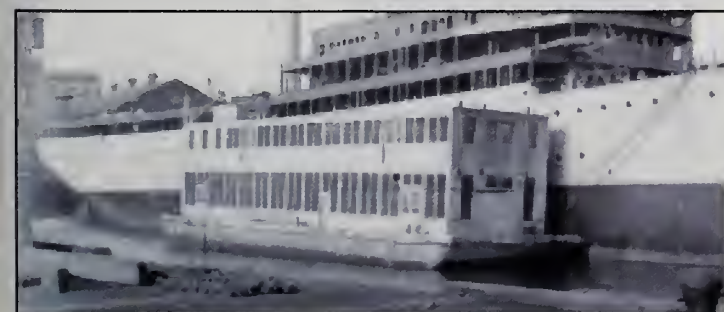
FLOATING WORKSHOP (YR) — Also known as repair barges, floating workshops supplemented shore-based shops for crews performing work on ships. Here, YR-15 is seen alongside USS Whitney (AD-4) on Nov. 3, 1923. BOSTS-14686
