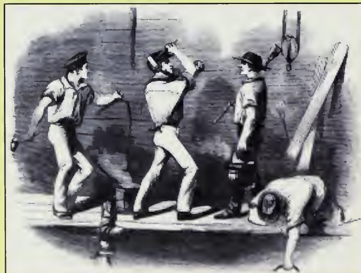
CAULKER — Caulkers performed an important task during the age of wooden ships in sealing joints to make them waterproof. This illustration appeared in Harper's New Monthly Magazine in 1862.
