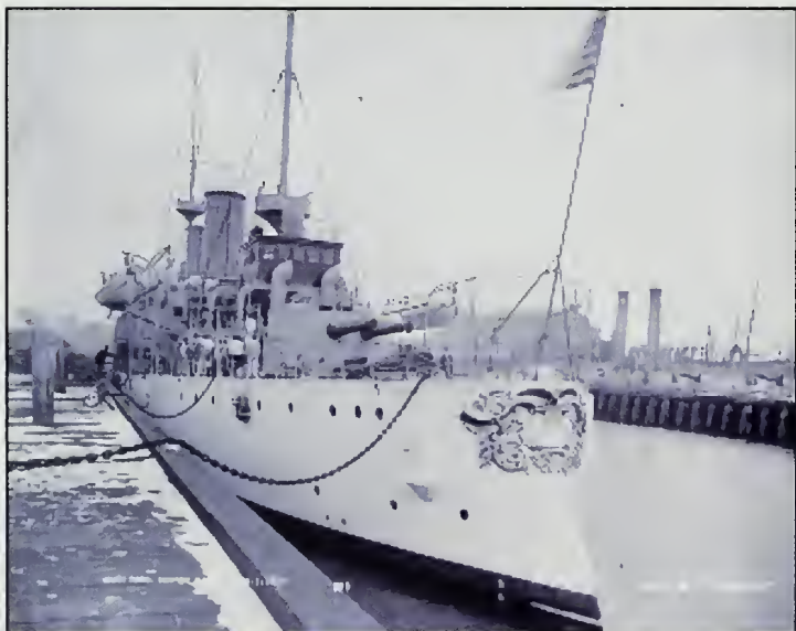
USS Olympia (C-6), the flagship of Adm. George Dewey at the Battle of Manila Bay on May 1, 1898, is tied up to Pier 6 East on Nov. 1, 1902. The pier, together with Pier 7 in the background, was a part of the major modernization effort to allow the yard to service steel vessels such as Olympia . BOSTS-13844
