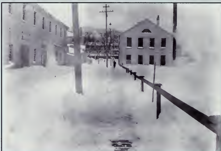
A worker shovels the wooden sidewalk of 5th St. in this image, Building 24 is at left, while Building 28, the Electric Light Station, is on the east side of the street.
