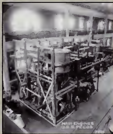
As the ship's hull began to take shape on the Shipways as seen in the Jan. 7, 1921, view at left, her engines were being fabricated by the yard's shops. At right, the main engines are seen nearing completion in Building 42's Machine Shop No. 1.
