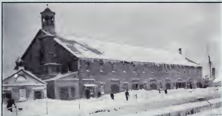
Building 23 (left), then a Plumbers Shop, was the former Chapel while Building 24 was the Carpenters Shop & Rigging Loft.
