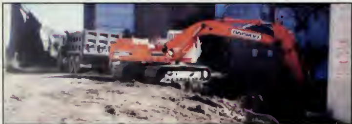
In 1994 the U.S. Army Corps of Engineers removed the underground fuel tanks outside of the Power Plant (Building 108) in the Navy Yard. Two years later, the Corps returned to the site to ensure that all contaminated soil in the area had been removed. U.S. Army Corps of Engineers
