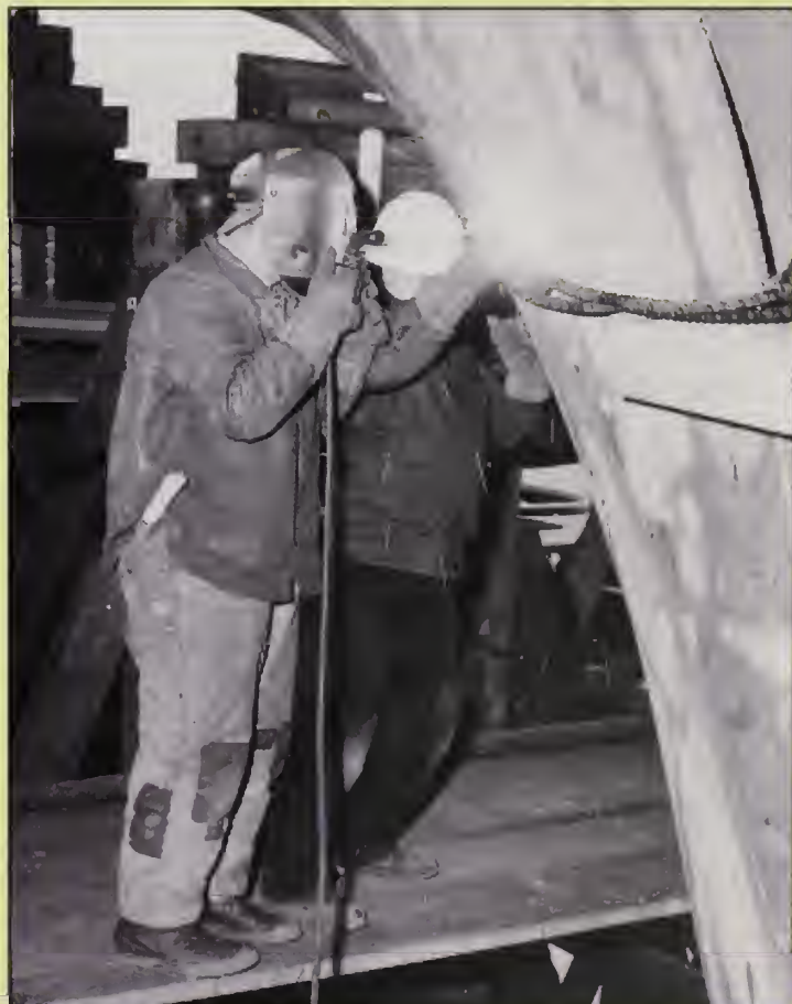
WELDER — As all-welded hulls replaced riveted hulls, the welder assumed greater importance in the yard. Here a welder works on the construction of USS Suffolk County (LST-1173) in early 1956. BOSTS-14320
