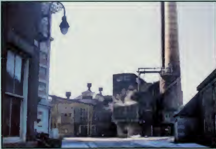
Building 108, Cooling Tower 264, Ash Silo 268
