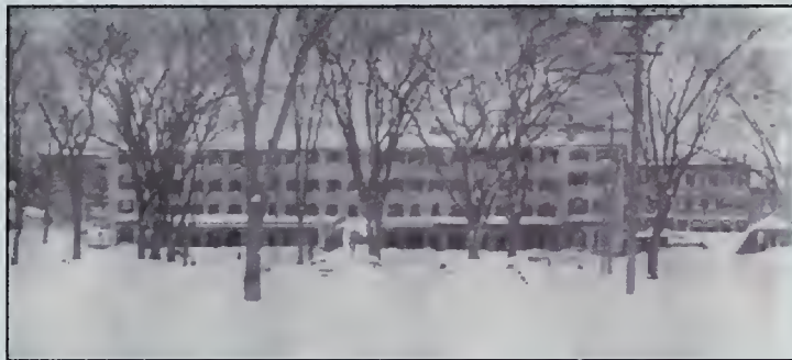
This view shows the Marine Barracks (Quarters H-I-K) looking across a depleted Shot Park. Note the USS Niagara figurehead in the center and the Marine Corps Officer of the Day Office (Building 30) at right.
