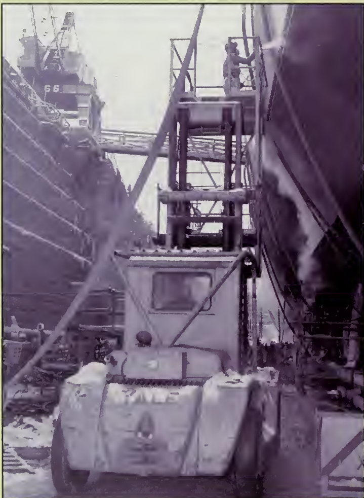
PAINTER — Shipyard painters often worked under difficult conditions. On Dec. 16, 1970, a painter sprays the hull of USS Little Rock (CLG-4) in Dry Dock 3 from scaffolding supported by a forklift.
