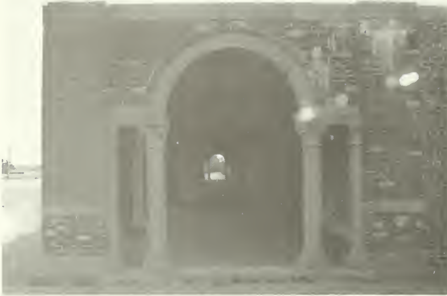
Figure 43: West end of Entrance Pavilion arcade. NPS photo, 1985.
