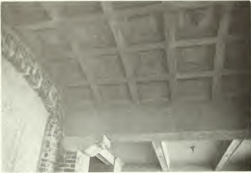
Figure 51: Coffered ceiling bay KL at the Entrance Pavilion. NPS photo, 1985.
