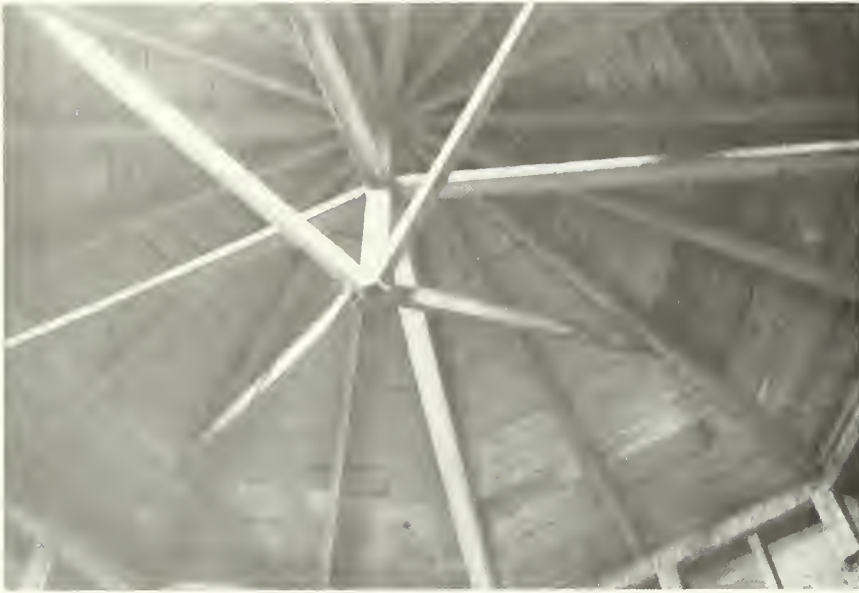
Figure 27: Tower roof framing--typical. NPS photo, October 1985.
