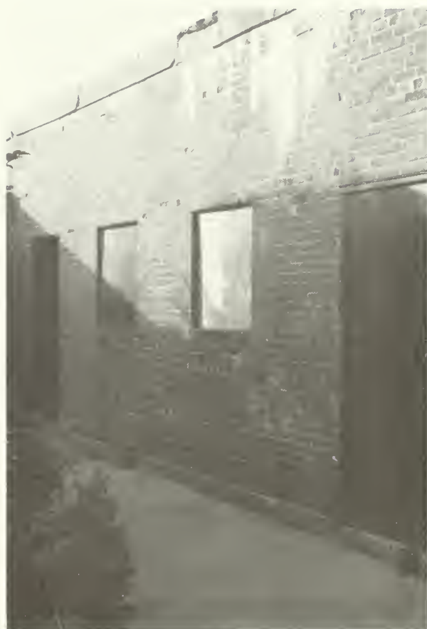
Figure 45: East side of Entrance Pavilion. NPS photo, 1985.
