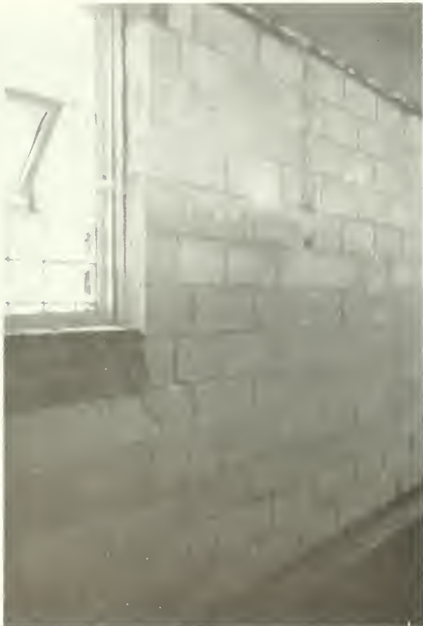
Figure 68: Rebuilt east wall, women's toilet room, West Wing. NPS photo, 1985.
