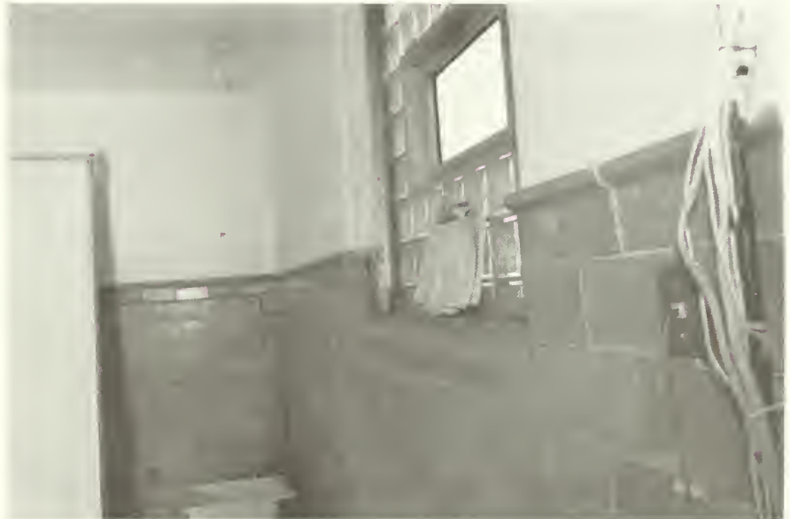
Figure 70: Bow in east wall, Window 518, West Wing. NPS photo, 1985.
