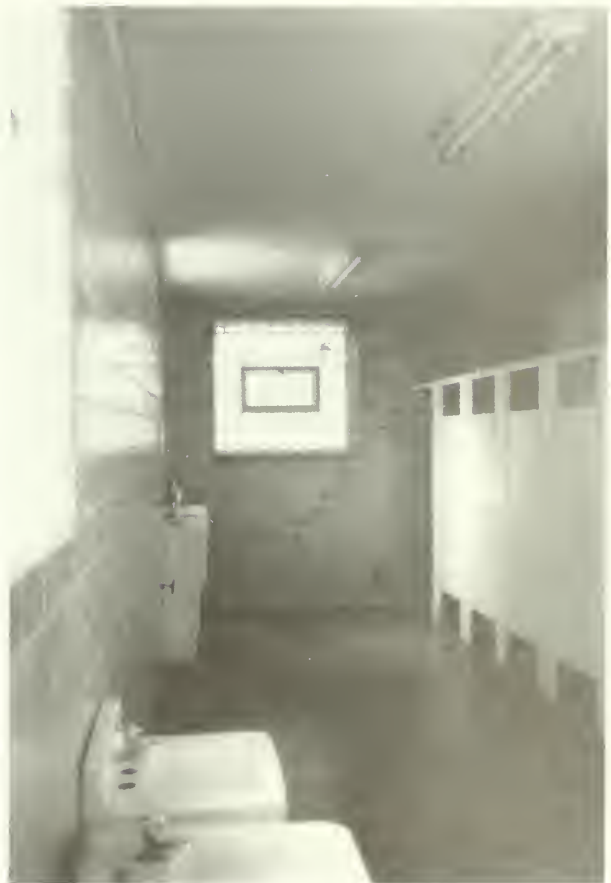
Figure 76: Men's toilet room, East Wing, looking north, showing bow in west wall. NPS photo, 1985.
