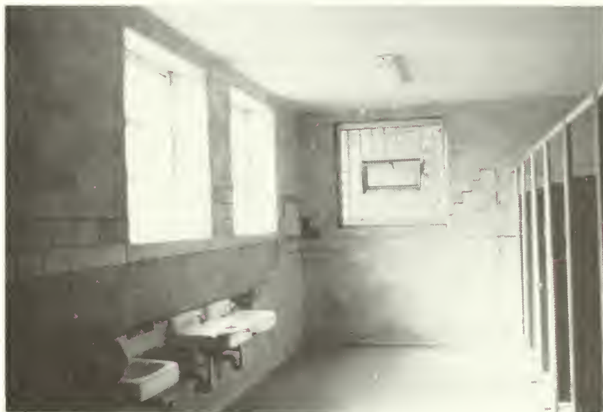
Figure 66: Interior of women's toilet room, West Wing, looking north. NPS photo, 1985.
