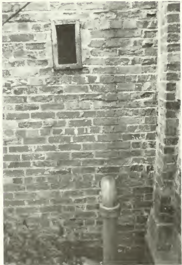
Figure 56: Door into meter room, West Screen Wall. NPS photo, 1985.
