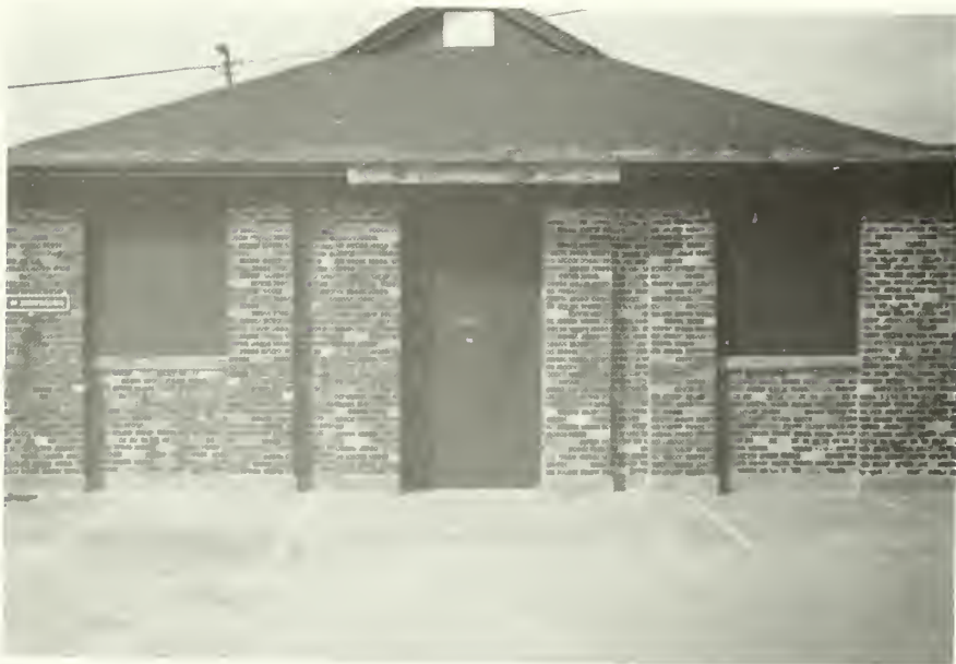
Figure 64: South end of West Wing. NPS photo, 1985.
