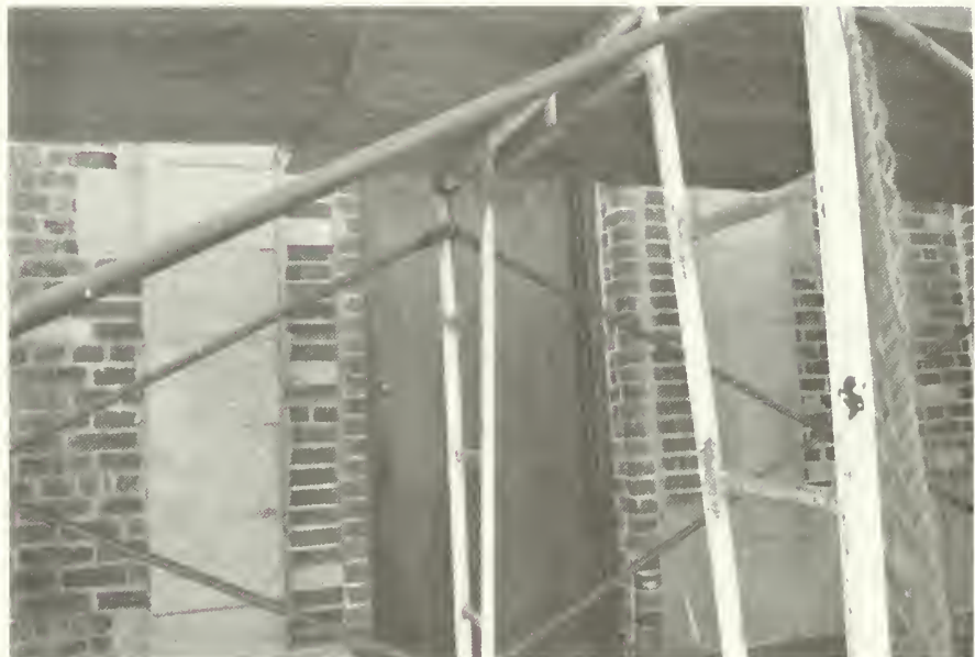
Figure 30: Flush doors at towers and penthouse. Doors typical throughout Beach Pavilion. NPS photo, October 1985.
