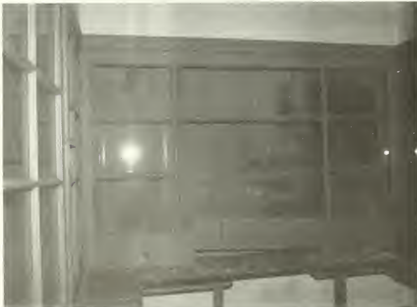
Figure 52: Typical ticket booth windows. NPS photo, 1985.
