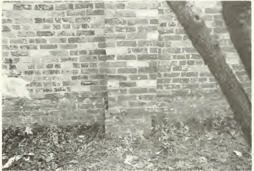
Figure 57: pier at West Screen Wall. NPS photo, 1985.
