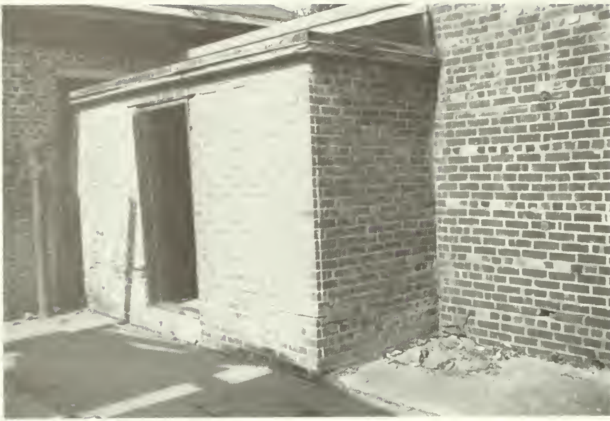
Figure 59: Meter room at West Screen Wall. NPS photo, 1985.
