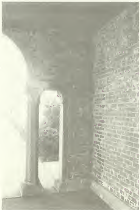
Figure 42: East end of Entrance Pavilion arcade, showing red brick infill at right. NPS photo, 1985.
