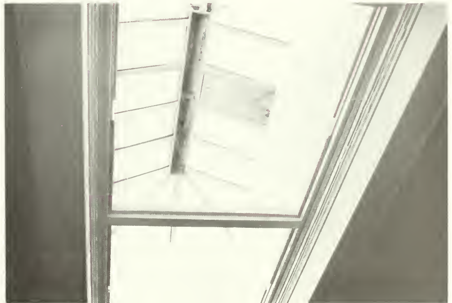
Figure 34: Typical skylight at Entrance Pavilion, interior view. NPS photo, 1985.
