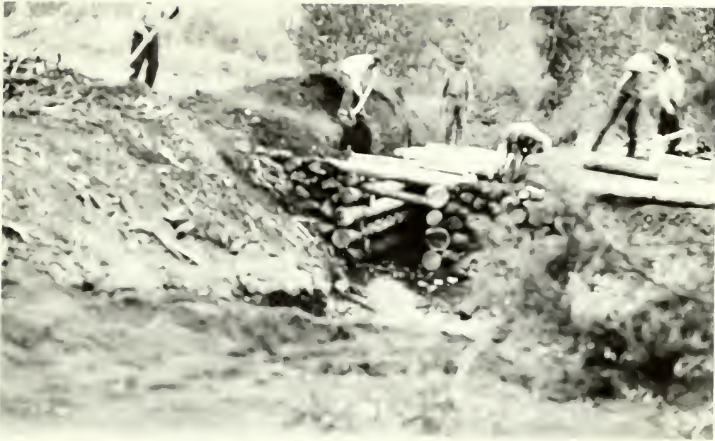
11120-2. Replacing culvert washed out by flood waters on East Forest Road.
