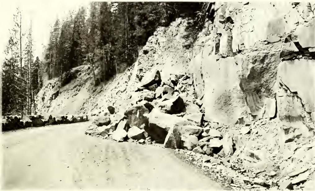
11170-5. Blasting on north entrance Road. The 1931 conditions, project #549.
