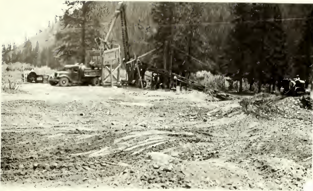
1119-5. Gravel crushing plant in operation on West Gallatin Road, project #534.
