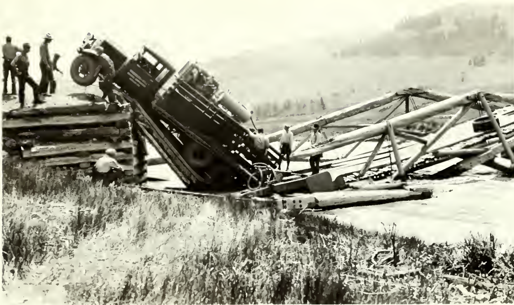
1119-4. Close view of broken section. Truck and equipment owned by contractor working on Red Lodge-Cooke road construction.
