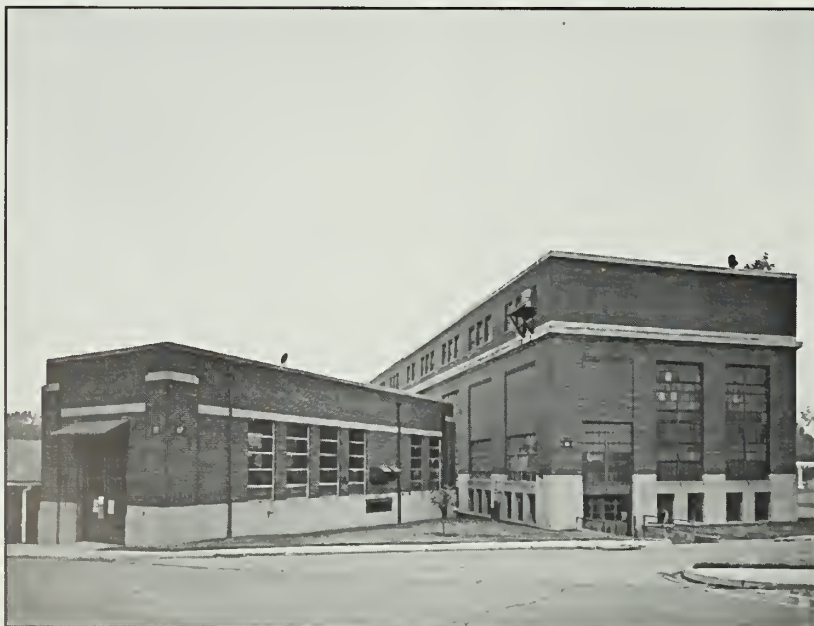
Figure 156: Building 67, looking northwest, 1991.
