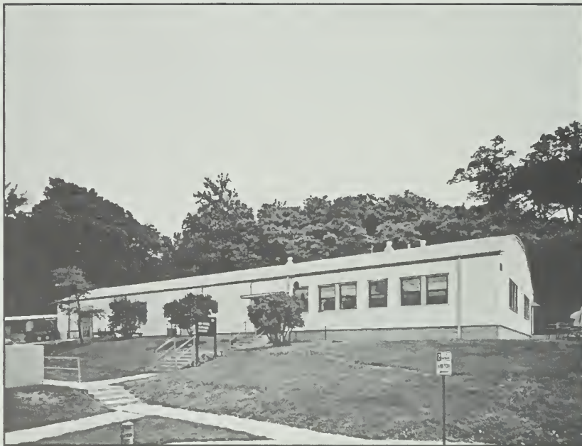
Figure 135: Building 55, looking northeast, 1992.
