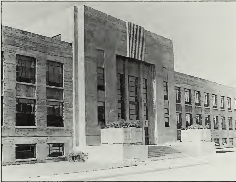
Figure 46: Main entrance to Building 14, ca. 1945. (USAF)
