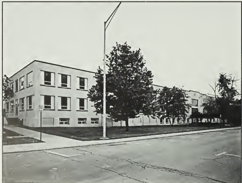
Figure 34: Building 11, looking southwest, 1992.
