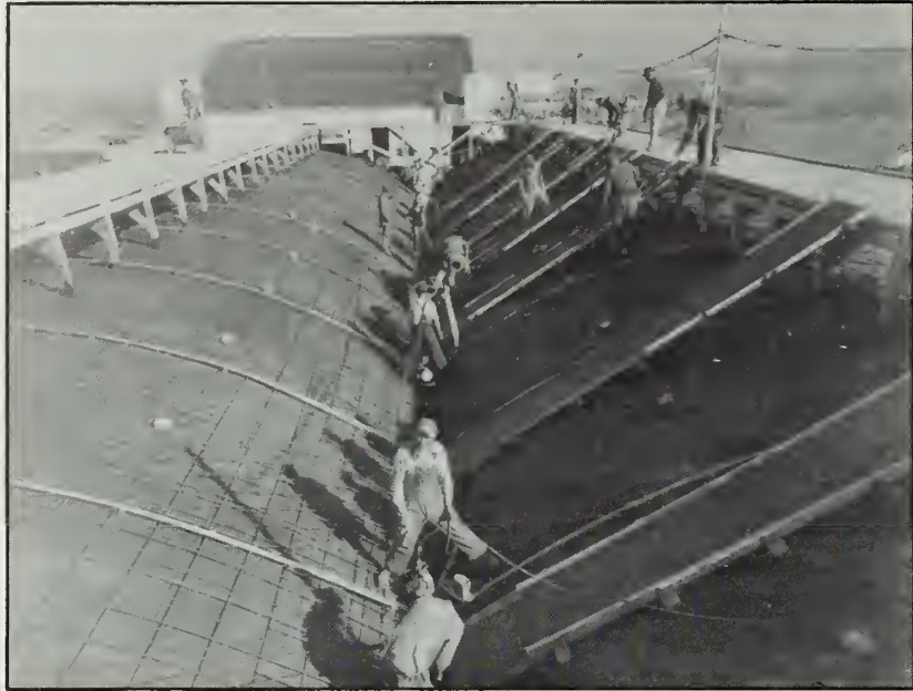
Figure 25: Building 6 under construction, showing reinforcing steel in barrel roof, 1942. (USAF)
