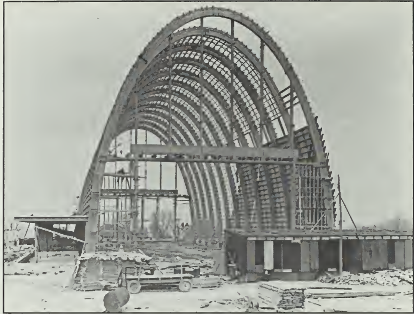
Figure 171: Wooden frame of Building 821, ca. 1947-48. (USAF)
