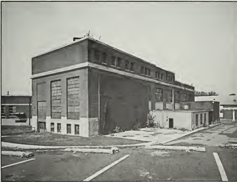
Figure 153: Building 66, looking west, 1991.
