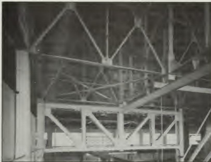
Figure 123: Ceiling trusses, Building 31, 1991.
