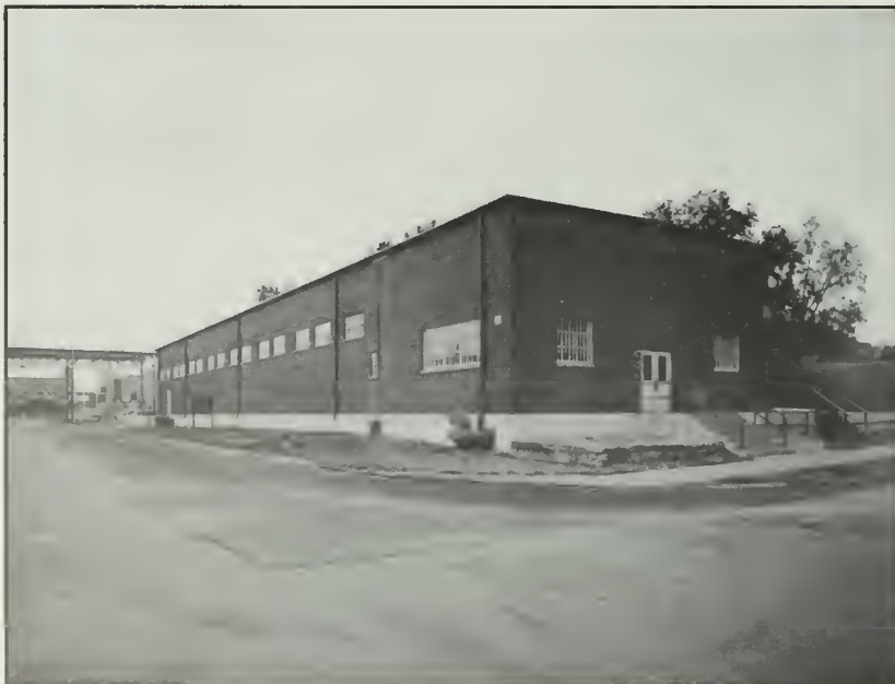
Figure 143: Building 63, looking northeast, 1991.
