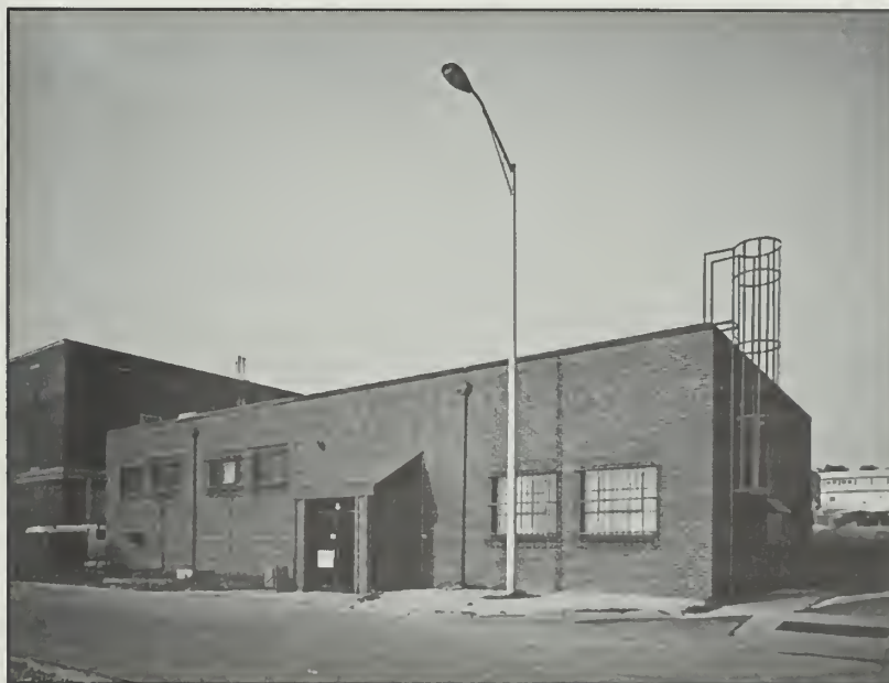
Figure 142: Building 62, looking northeast, 1991.
