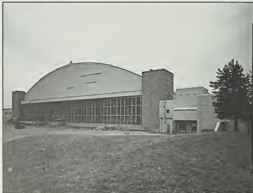
Figure 85: Rear of Building 22, looking southeast, 1991.
