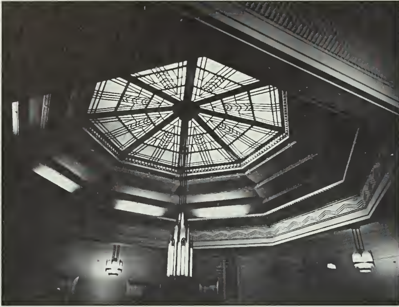
Figure 41: Skylight, foyer, Building 12, 1991.
