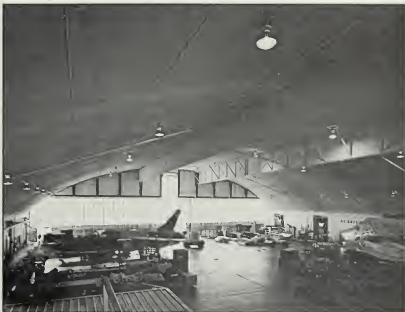
Figure 20: Interior view of one of the hangar bays, Building 4, 1991.
