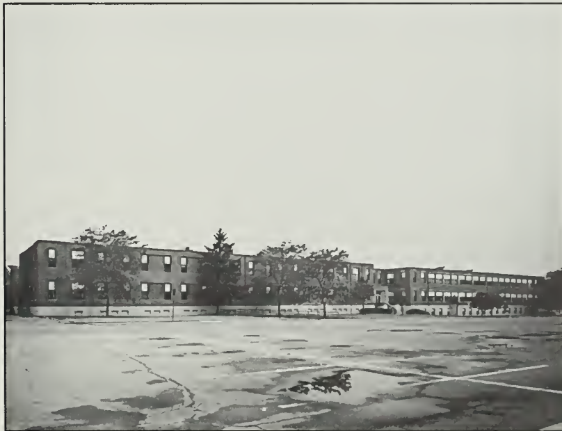
Figure 55: North facade, Buildings 18A-D, 1992.
