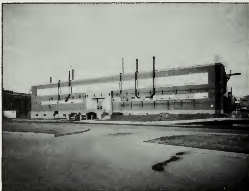
Figure 157: Building 70, looking northeast, 1991.
