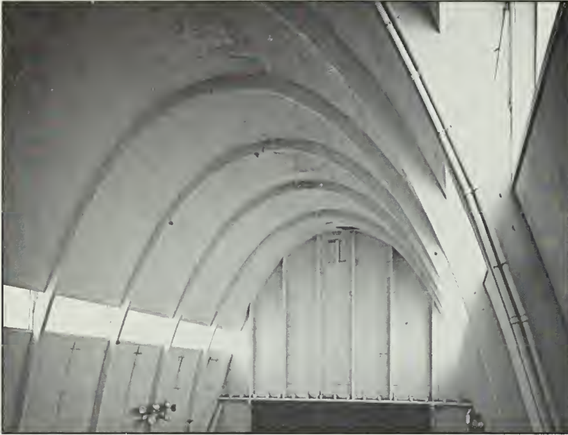
Figure 175: Interior view of ceiling, Building 821, 1991.
