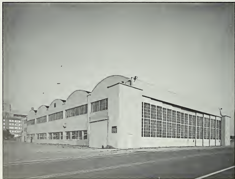
Figure 26: Building 6, looking southeast, showing sections and hangar door, 1991.
