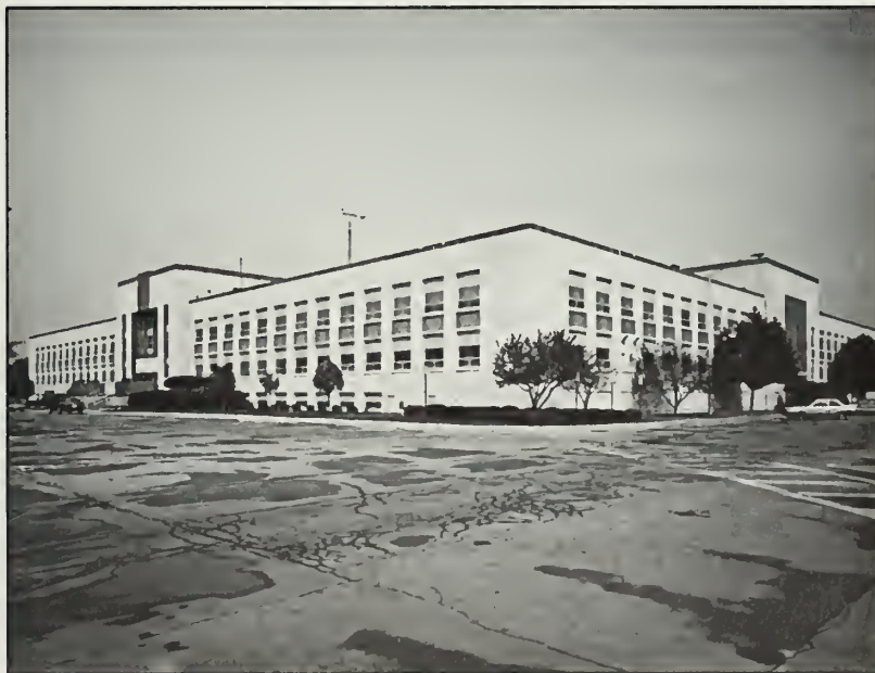
Figure 47: Building 14, looking northwest, 1991.
