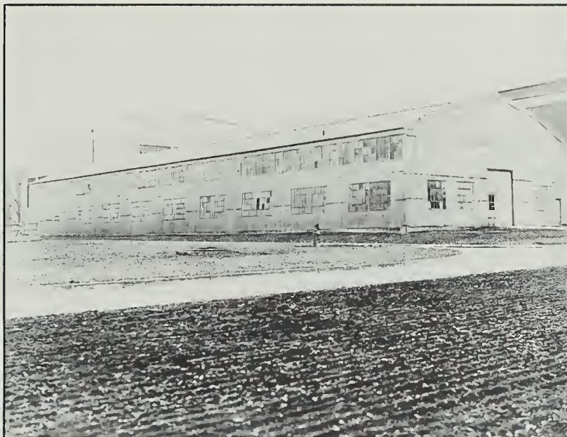
Figure 56: Temporary structure for Building 19, ca. 1927-29. (USAF)
