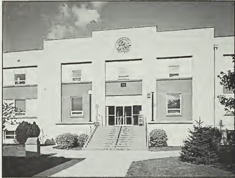
Figure 33: Entrance, west side of Building 11, 1992.
