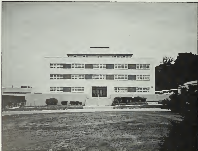
Figure 119: Building 29, looking north, 1992.
