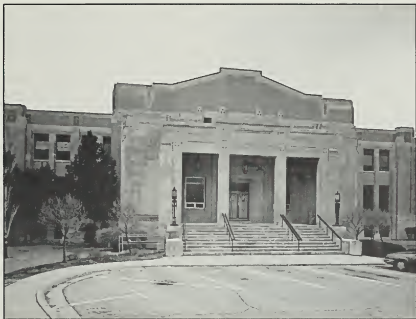
Figure 39: Building 12, west facade, 1991.
