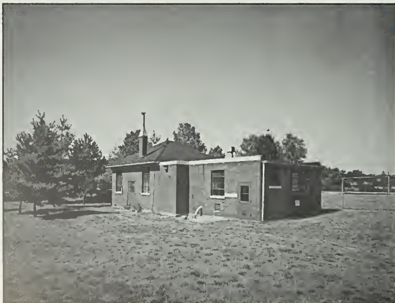
Figure 168: Building 86, looking west, 1991.
