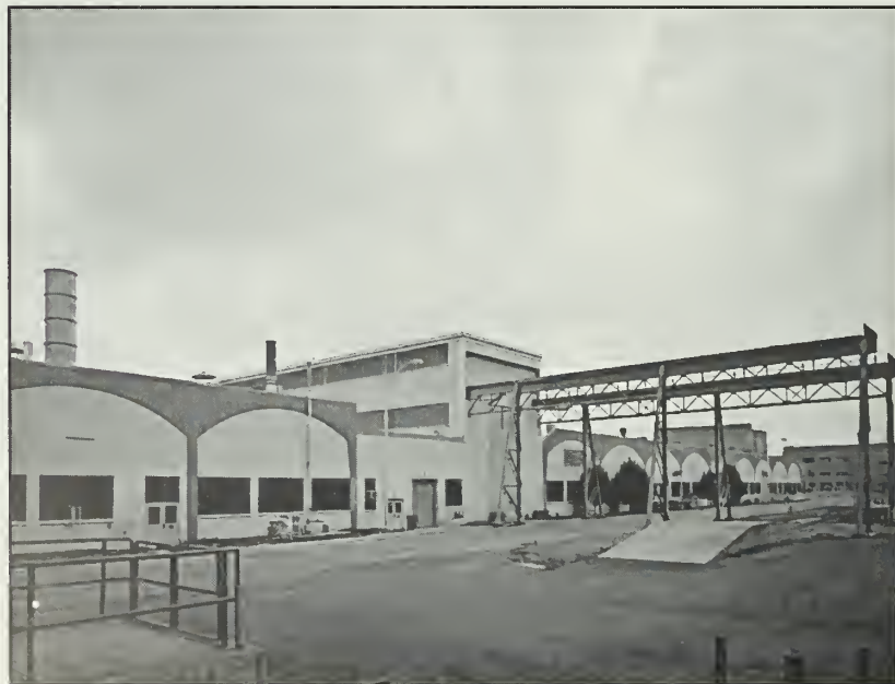
Figure 24: Building 5, showing crane structure, 1991.
