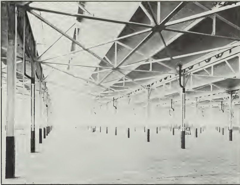
Figure 49: Interior of Building 16, ca. 1927. (USAF)
