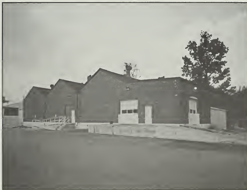
Figure 144: Building 64, looking northeast, 1991.
