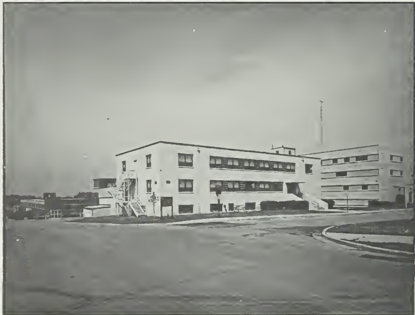
Figure 120: Building 30, looking northwest, 1991.
