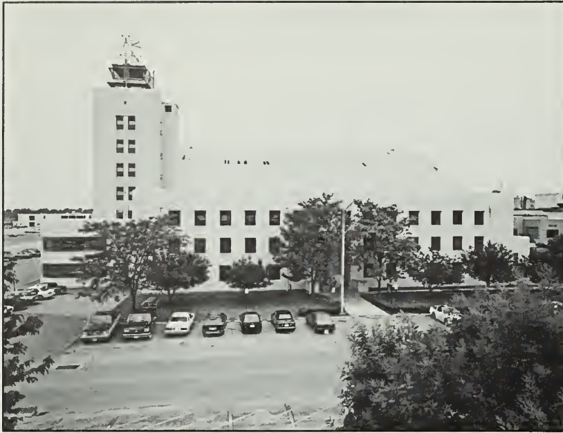
Figure 29: Building 8, looking north, 1992.
