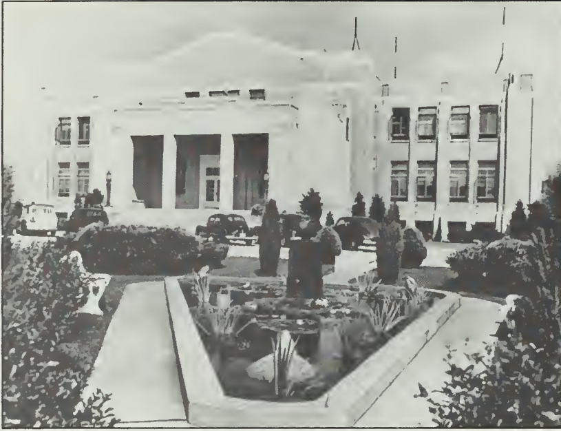
Figure 37: Building 12, ca. 1930s, and ornamental pond. (USAF)
