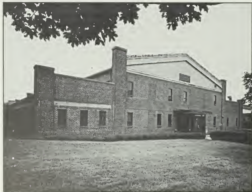
Figure 53: Building 17, east facade, 1991.
