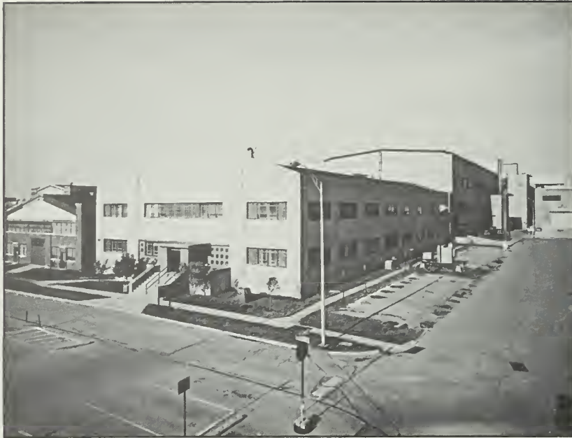
Figure 68: Building 20, looking northeast, 1991.
