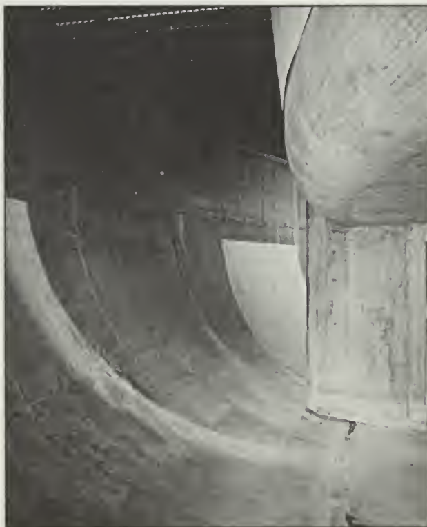
Figure 111: Interior view of basement, Vertical Wind Tunnel, 1991.
