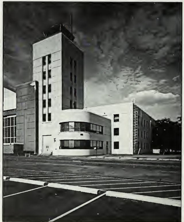
Figure 30: West facade of Building 8, 1991.
