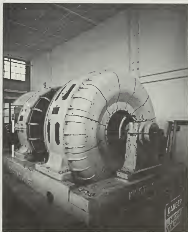
Figure 61: One of two generators for 5-Foot Wind Tunnel, 1991.
