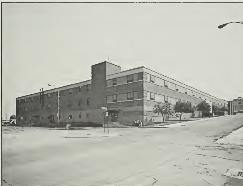
Figure 117: Building 28, looking northeast, 1991.
