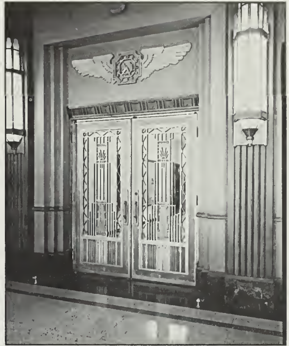
Figure 5: Entrance detail, ground floor, Building 12, 1991.
