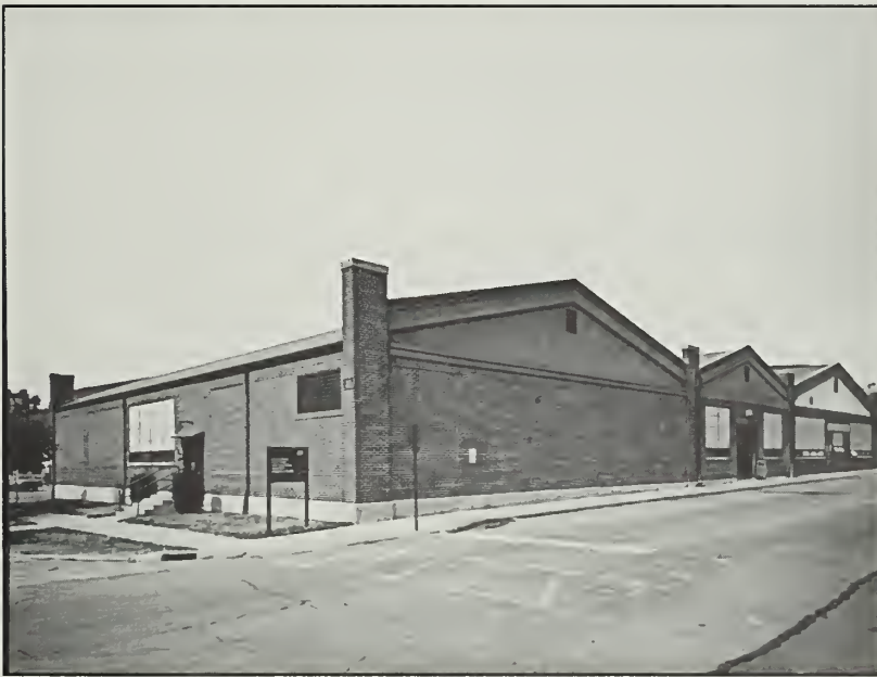
Figure 132: Building 39, looking northeast, 1991.
