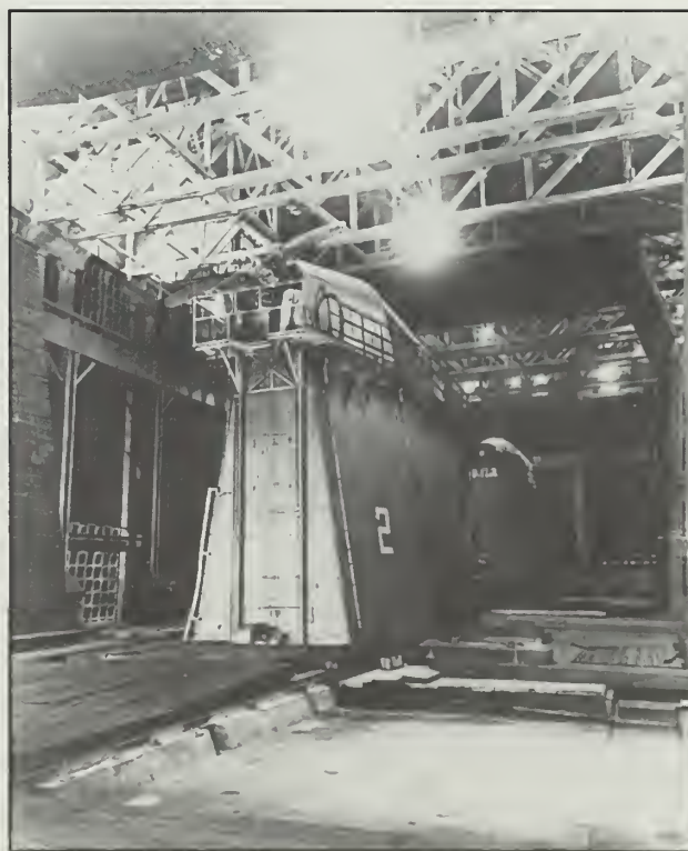
Figure 72: Propeller test stands, Building 20A. (USAF)
