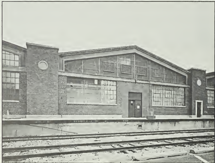
Figure 137: Detail of single bay, Building 56, 1991.
