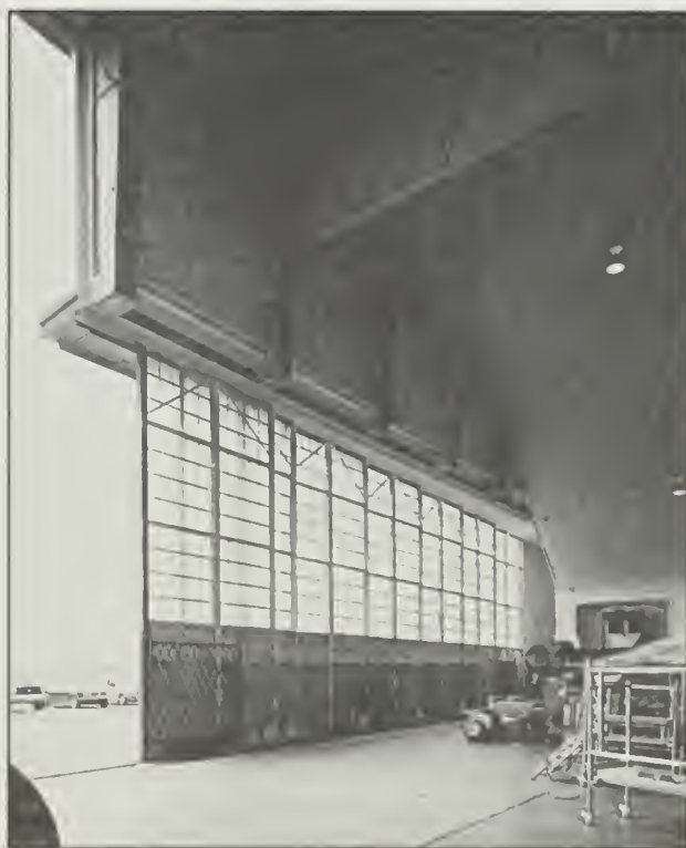
Figure 21: Hangar doors, Building 4, 1991.
