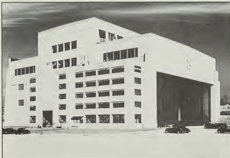
Figure 145: Building 65, 1944. (USAF) [See also photograph on page 26.]
