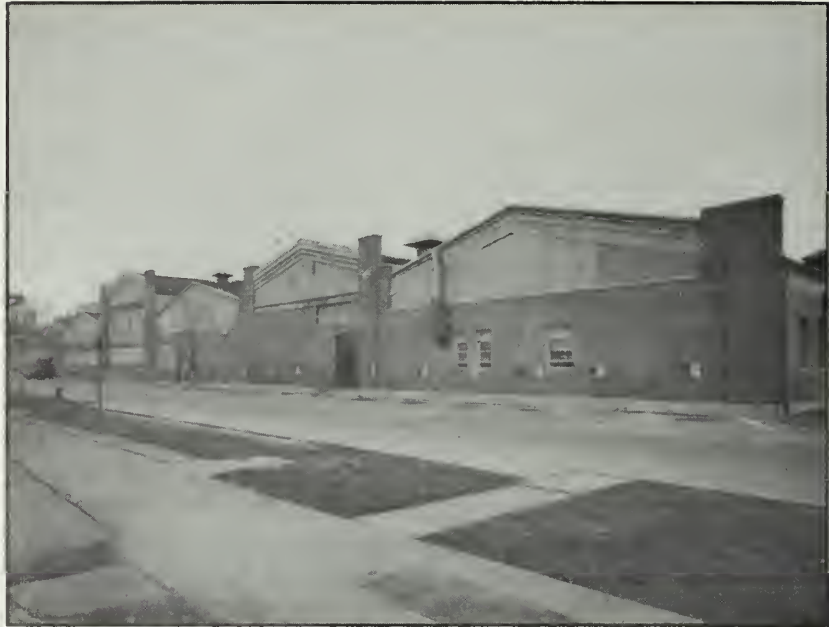
Figure 128: North facade of Building 32 complex, 1991.
