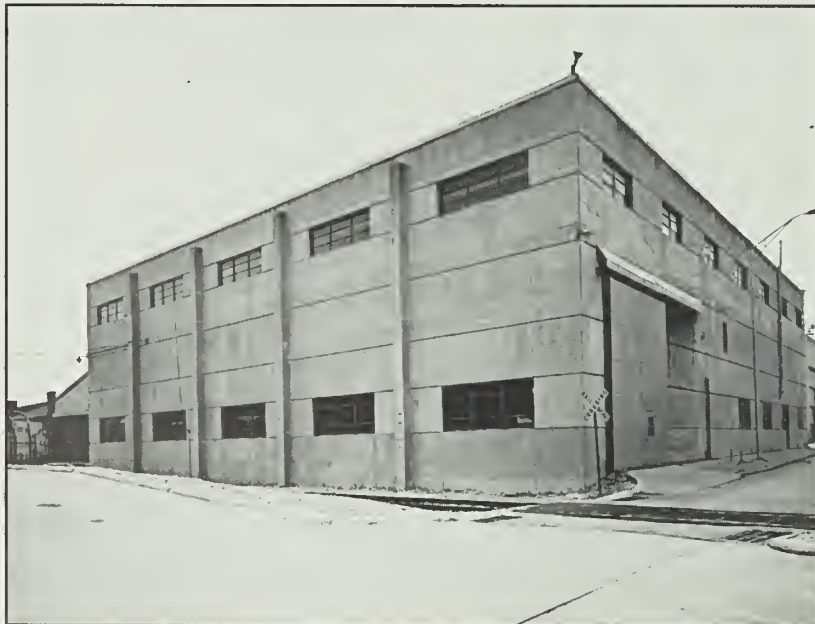
Figure 80: 1953 addition to Building 21, 1991.
