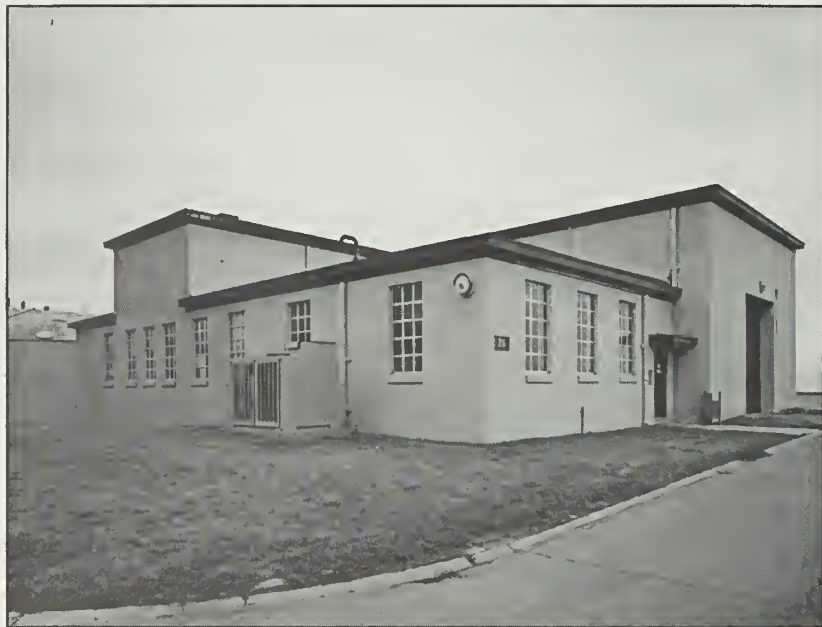
Figure 106: Building 26, looking northwest, 1991.
