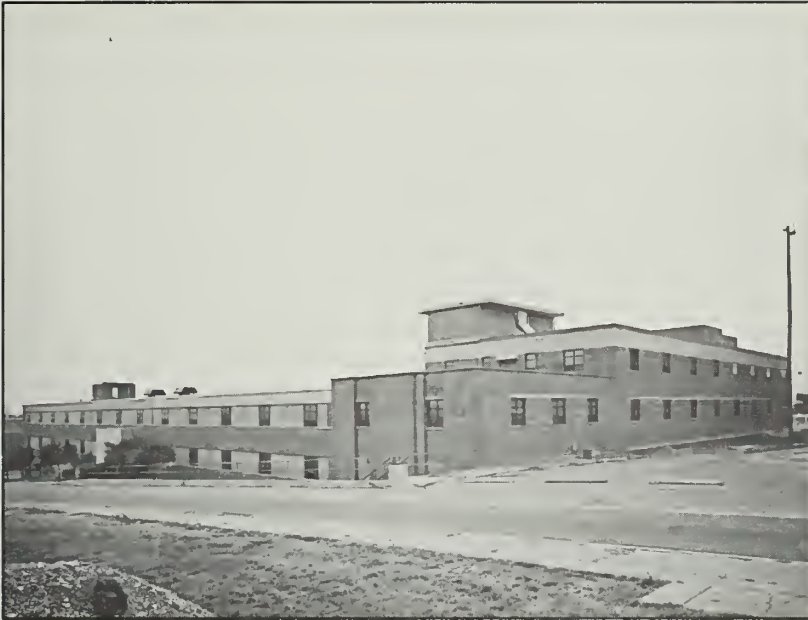
Figure 116: Building 28, looking northwest, 1991.
