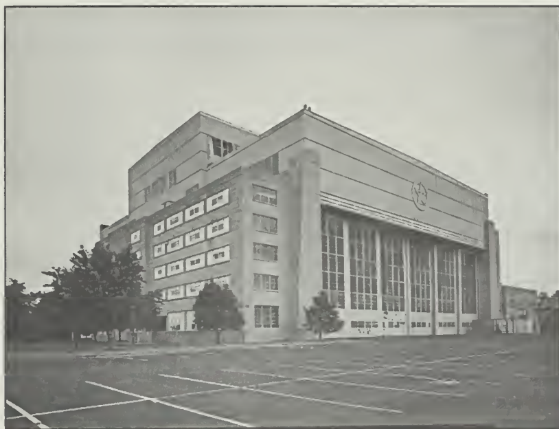
Figure 148: Building 65, looking northeast, 1991.
