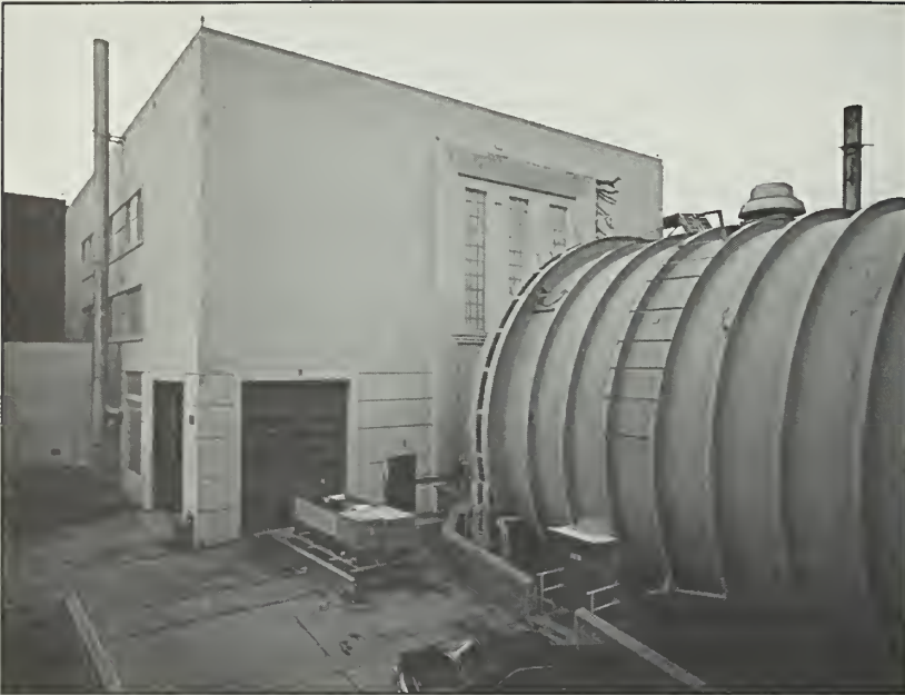
Figure 99: Building 25B (Test Chamber), looking northwest, 1991.
