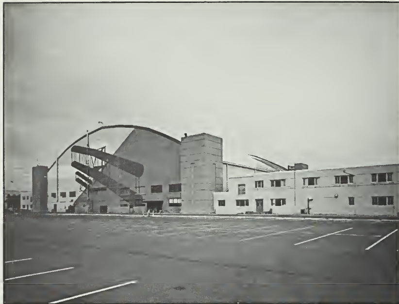
Figure 84: Building 22, looking northeast, 1991.
