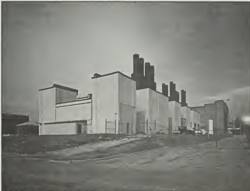
Figure 159: Building 71 complex, looking northeast, 1991.
