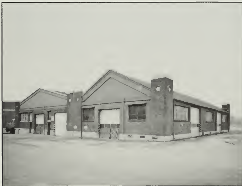
Figure 131: Building 38, looking northwest, 1991.
