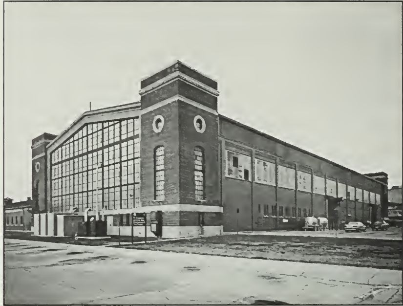
Figure 121: Building 31, looking northeast, 1991. [See also photograph on page 10.]
