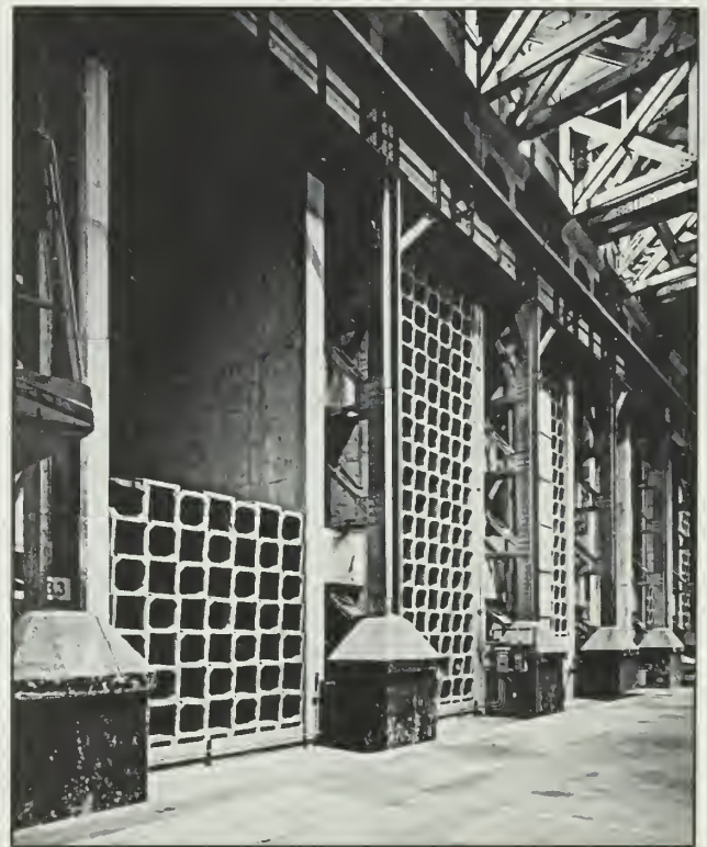
Figure 74: Interior wall of Building 20A, showing concrete sound baffles, 1991.
