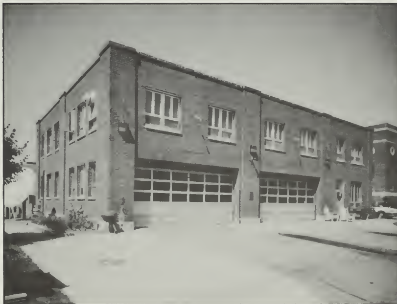
Figure 162: Building 76, looking northeast, 1991.
