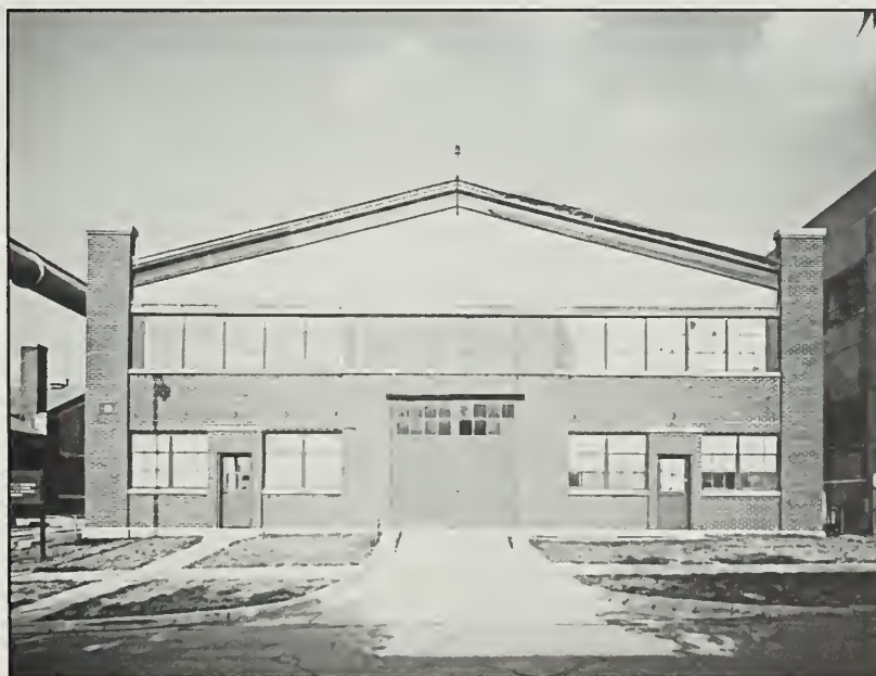
Figure 57: West facade of Building 19, 1991.
