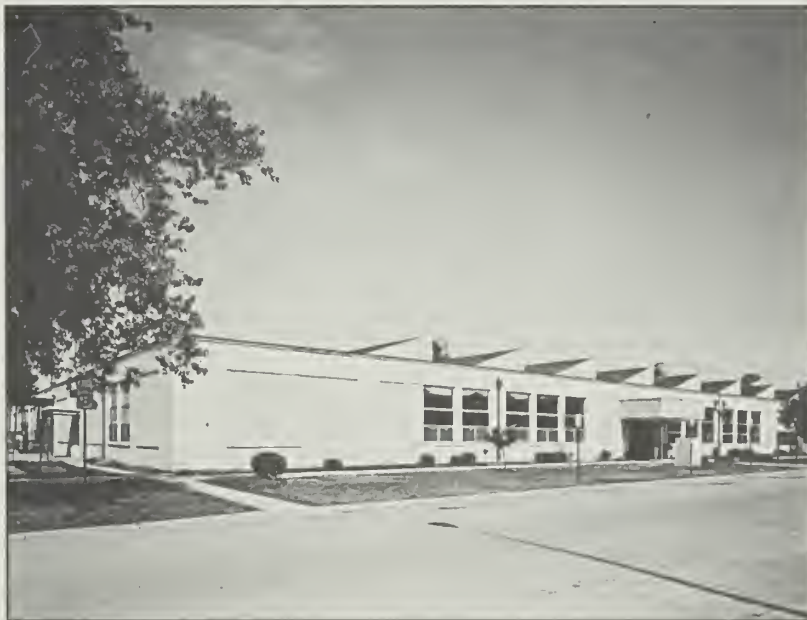
Figure 50: Building 16, looking northwest, 1992.
