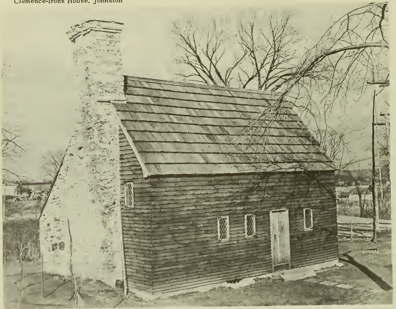
Clemence-Irons House, Johnston
