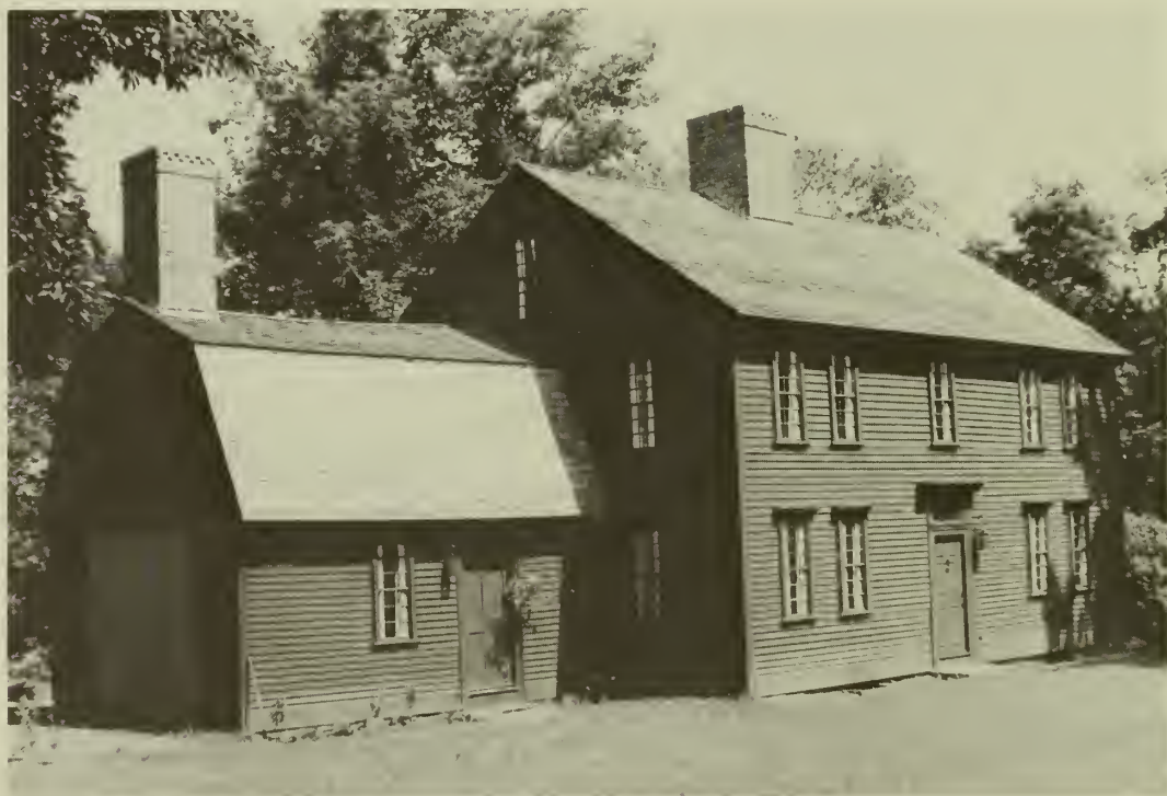
Exterior, Completed restoration
