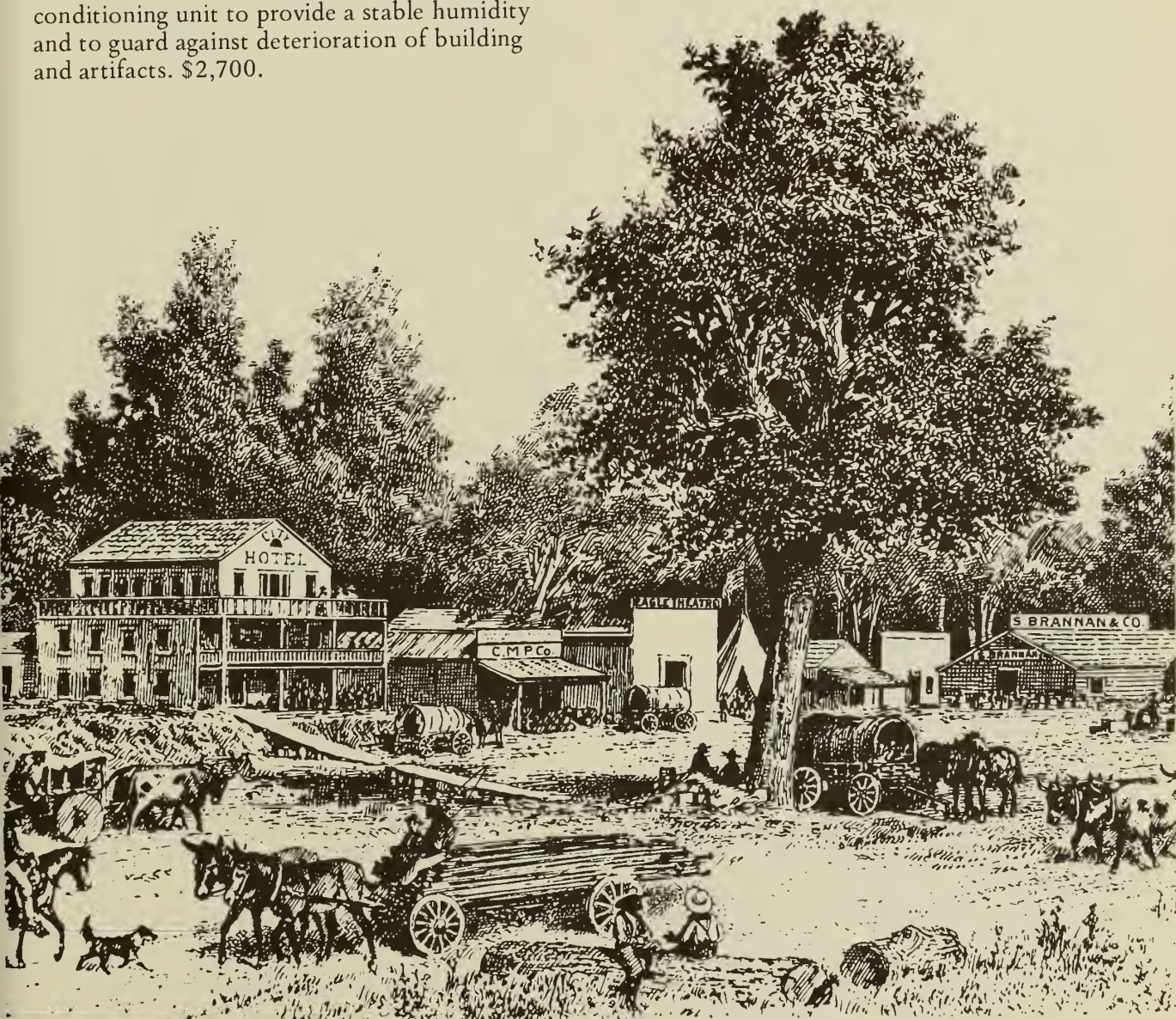
Old Sacramento Historic District: Eagle Theater, Sacramento
