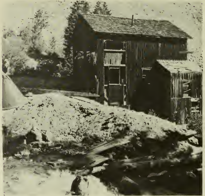
Ore Processing Mill and Dam, Georgetown vic.
