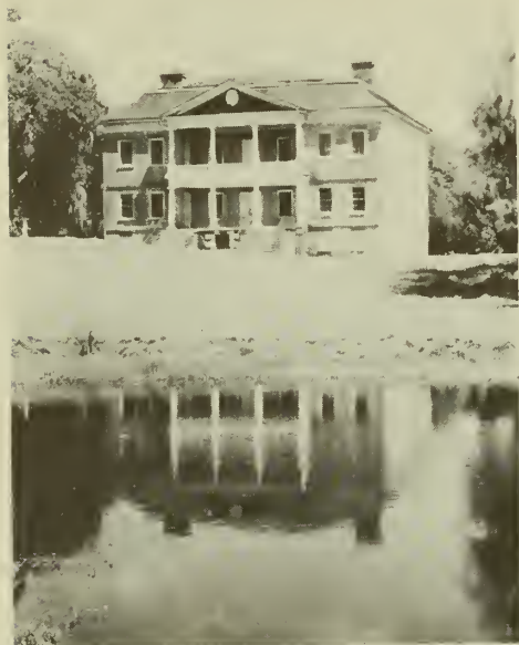
Drayton Hall, National Trust, Charleston, South Carolina
