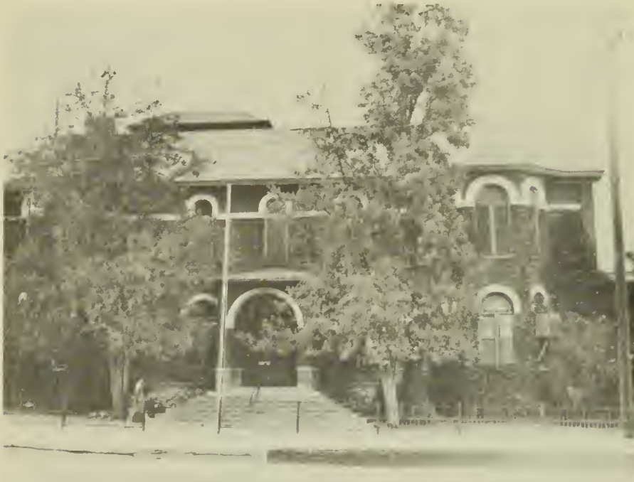
Phelps Dodge General Office Building, Cochise Co.
