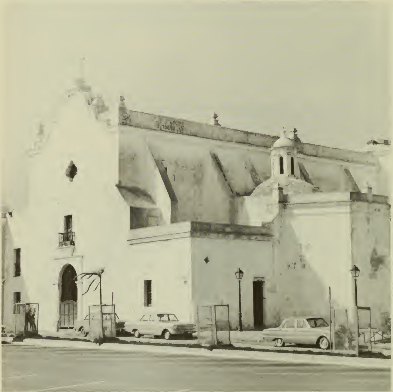
San Juan Historic District; San Jose Church, San Juan
