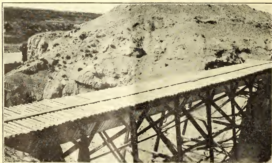
J. C. COULEE FLUME, WILLWOOD DIVISION, SHOSHONE PROJECT, WYOMING
