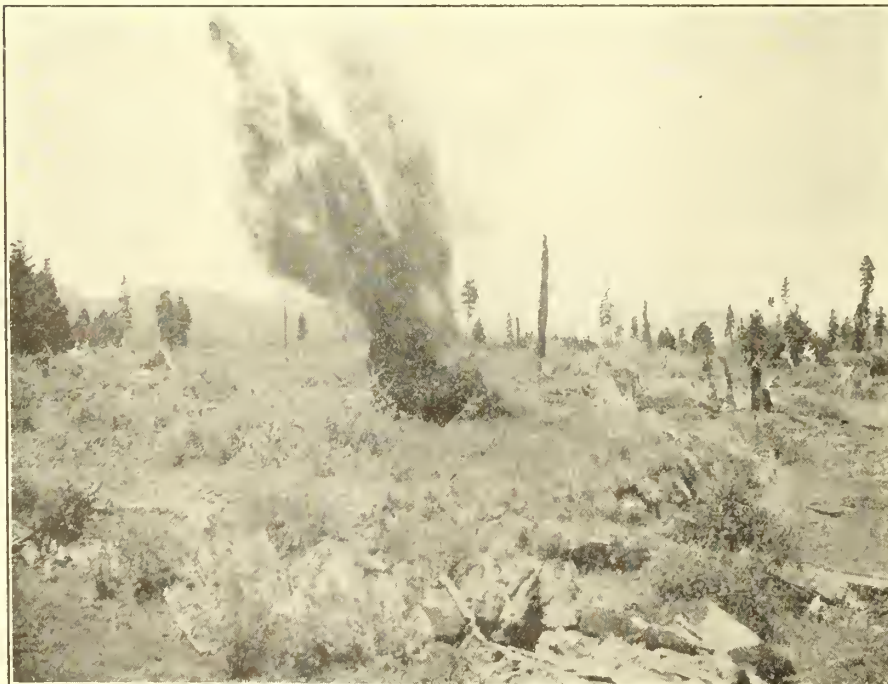
Blasting stumps in land-clearing operations, Kittitas division, Yakima project, Washington
