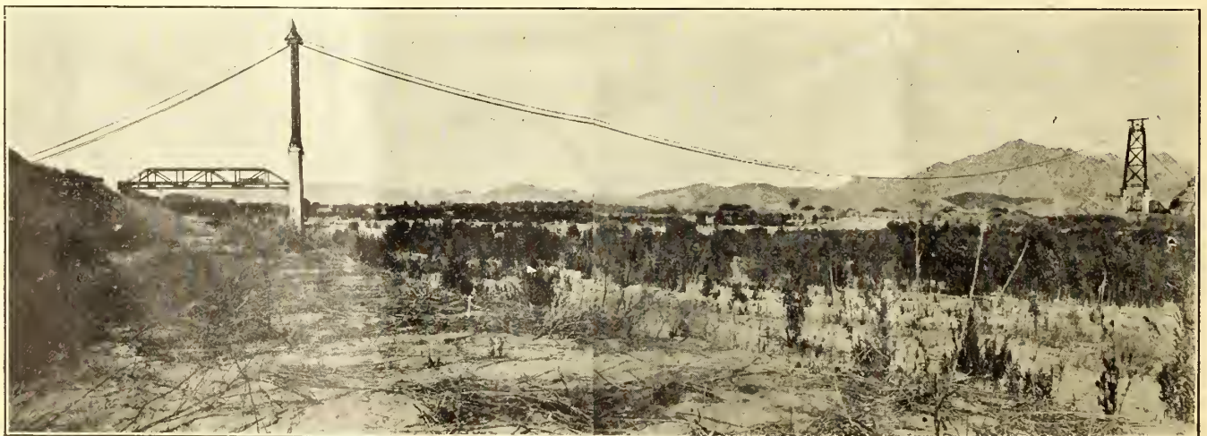
GILA RIVER SUSPENSION BRIDGE
