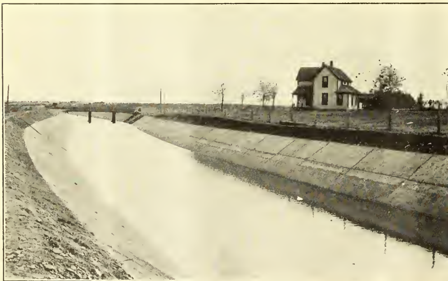
Main canal, Boise project, Idaho
