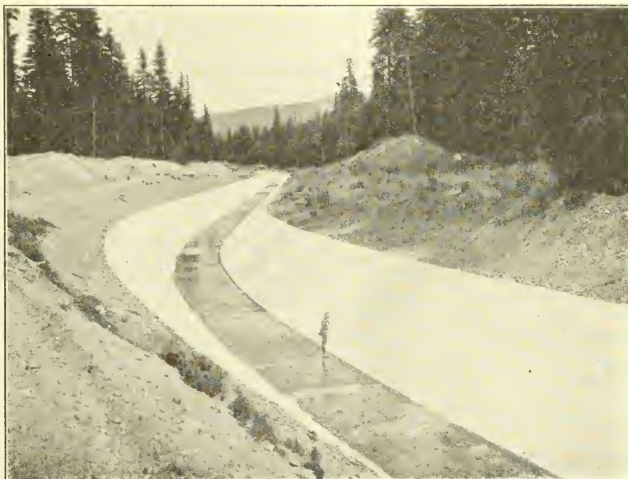
Looking down the Main Canal, near Easton, Washington, Kittitas division, Yakima project
