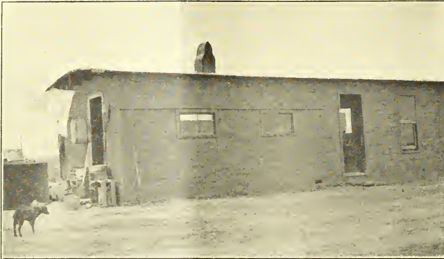
The adobe home of a new settler on the Willwood division, Shoshone project, Wyoming
