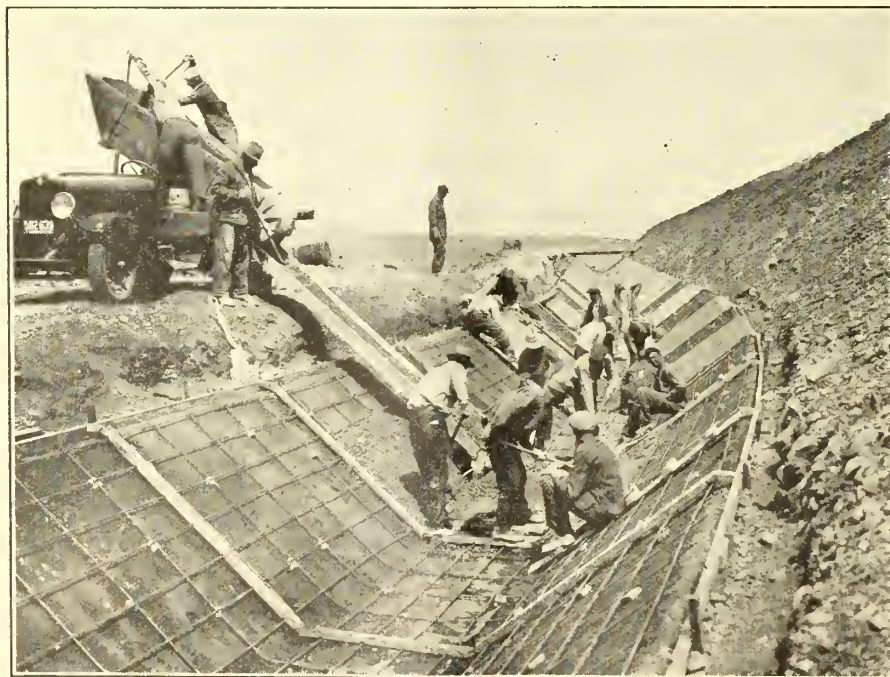
Concrete canal lining (concrete placed by hand), South Branch Canal, Kittitas division, Yakima project, Washington
