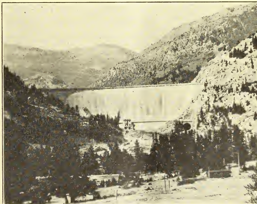
Gibson dam, Sun River project, Montana
