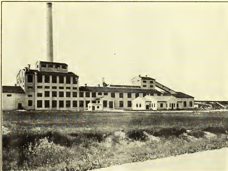
Beet sugar factory at South Torrington, Wyo., on the North Platte project, Nebraska-Wyoming
