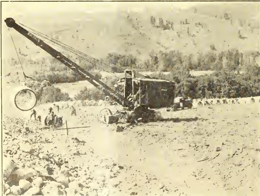
Dragline handling 54-inch lock-joint pipe, South Branch Canal, Kittitas division, Yakima project, Washington
