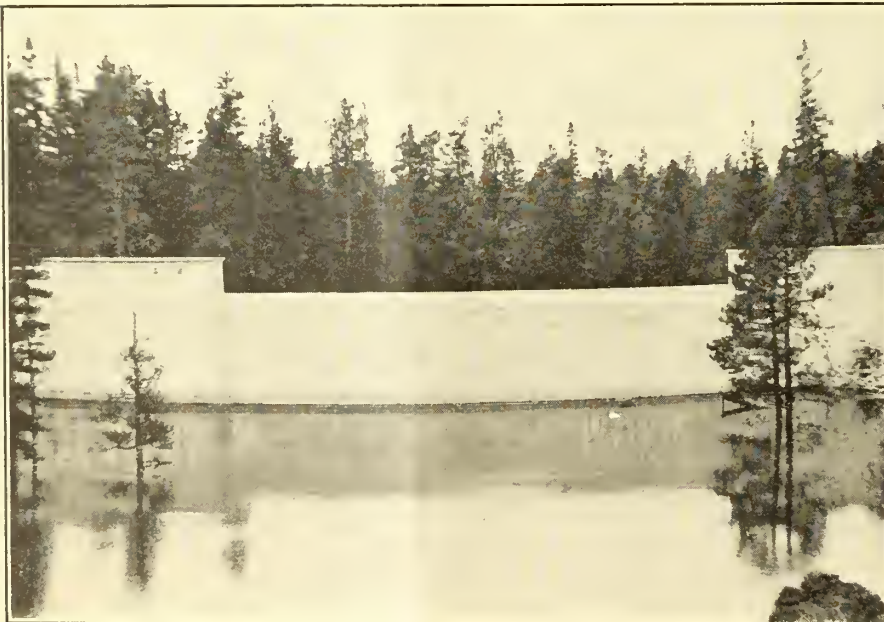
Gerber dam, Klamath project, Oregon-California
