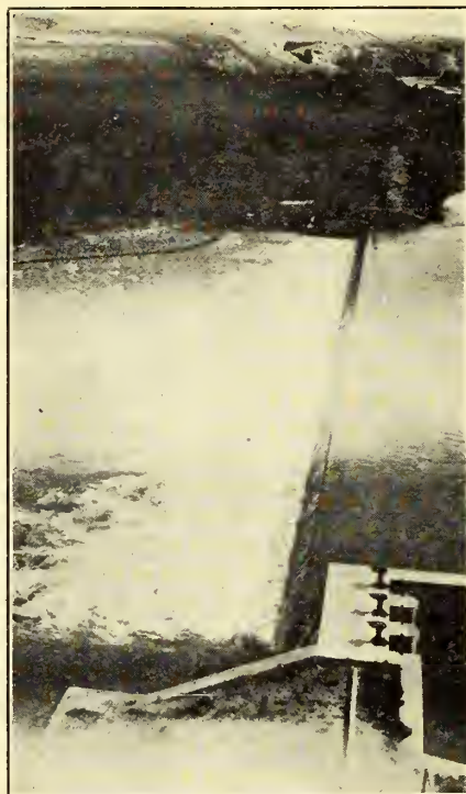
CORBETT DIVERSION DAM, SHOSHONE PROJECT, WYOMING
