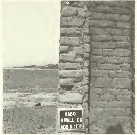
Figure 31. Brick pattern and interior veneer of adobe A.
