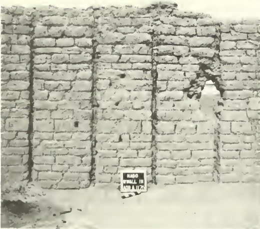
Figure 32. Interior vertical notches in adobe A.
