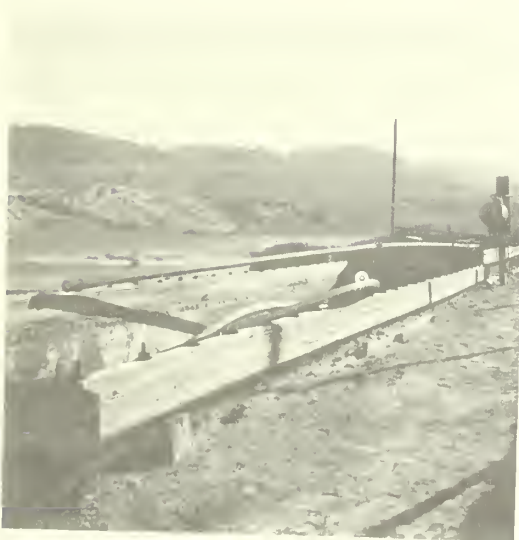
Figure 14. Dissolving tanks with lumber bolted around rim.
