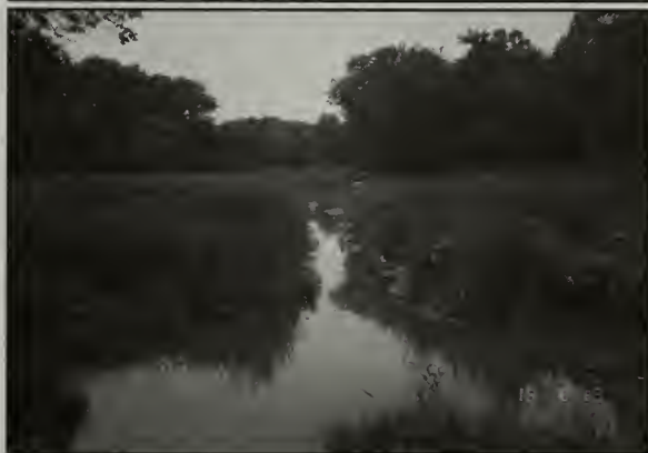
Before (top) and after (bottom) reconstruction of mass fill area #1 at Kenilworth Marsh. A tidal gut, or channel, was also installed in the restoration effort and shows in the bottom image of the completed marsh.
