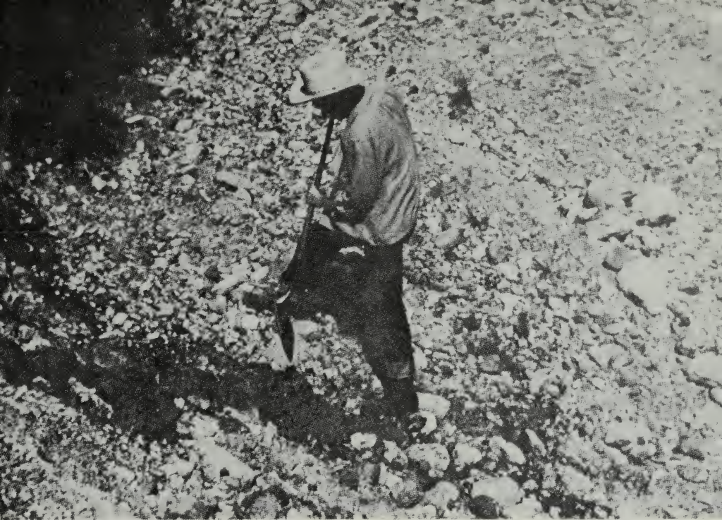
Figure 21. —Rehabilitation of Navel Spring consisted of digging back to the source of each trickle, then channeling it into one or more troughs made from half an oil drum, which we sank flush with the ground. Before the work, the seep shown here produced only 5 gallons per day.
