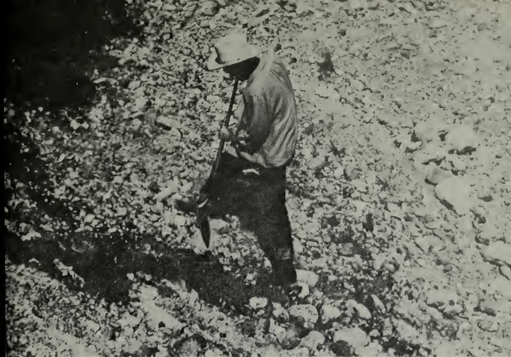
Figure 21. —Rehabilitation of Navel Spring consisted of digging back to the source of each trickle, then channeling it into one or more troughs made from half an oil drum, which we sank flush with the ground. Before the work, the seep shown here produced only 5 gallons per day.
