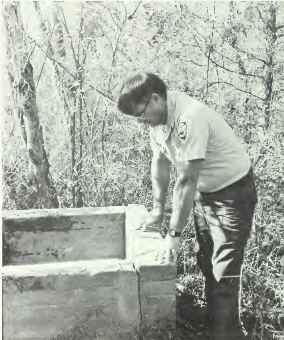
Ranger Paul Petty of the Pickens County Unit examines another abandoned well that is scheduled to be filled in by his personnel in a continuing effort to make the county safer for firefighters and the general public.
