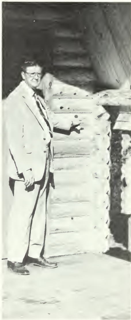
Fred Herndon, co-owner and manager of the Forsyth Campground, points to insulated tongue-and-groove joint in one of 14 log cabins at his facility. The picturesque cabins are designed to offer travelers an alternative to tents and motels.
