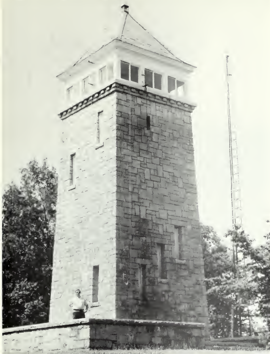
Ranger Brion Williams of the Habersham County Forestry Unit, who supervised much of the structure's renovation, stands on the stone platform at the base of historic Chenocetah Tower.
