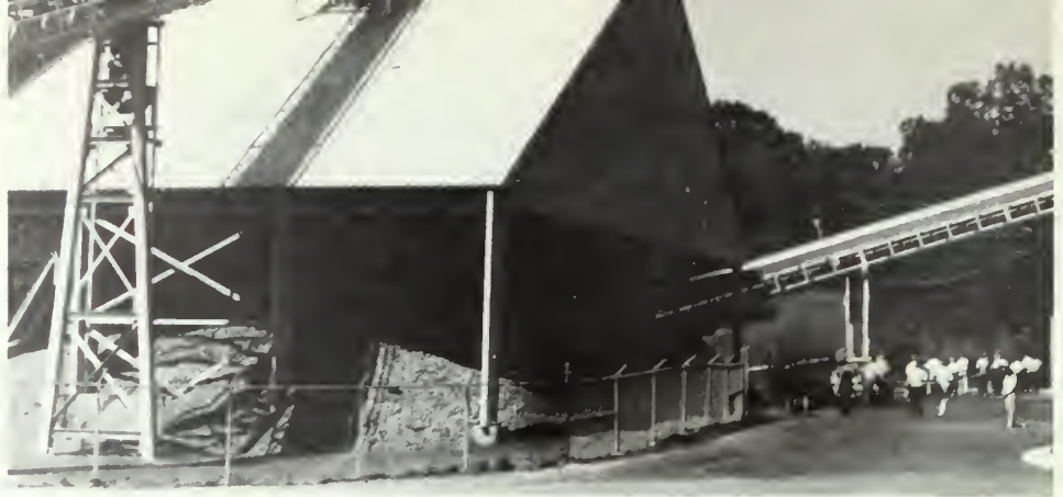
One conveyor moves chips into a storage area, while another conveys the material to the boiler section of the complex.
