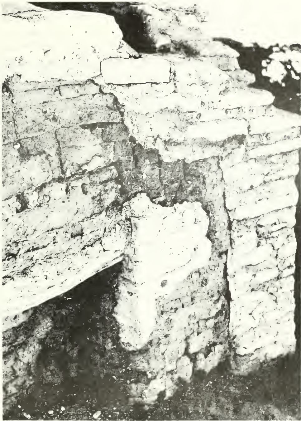
5. Northeast corner of granary showing effects of dissimilar materials.
