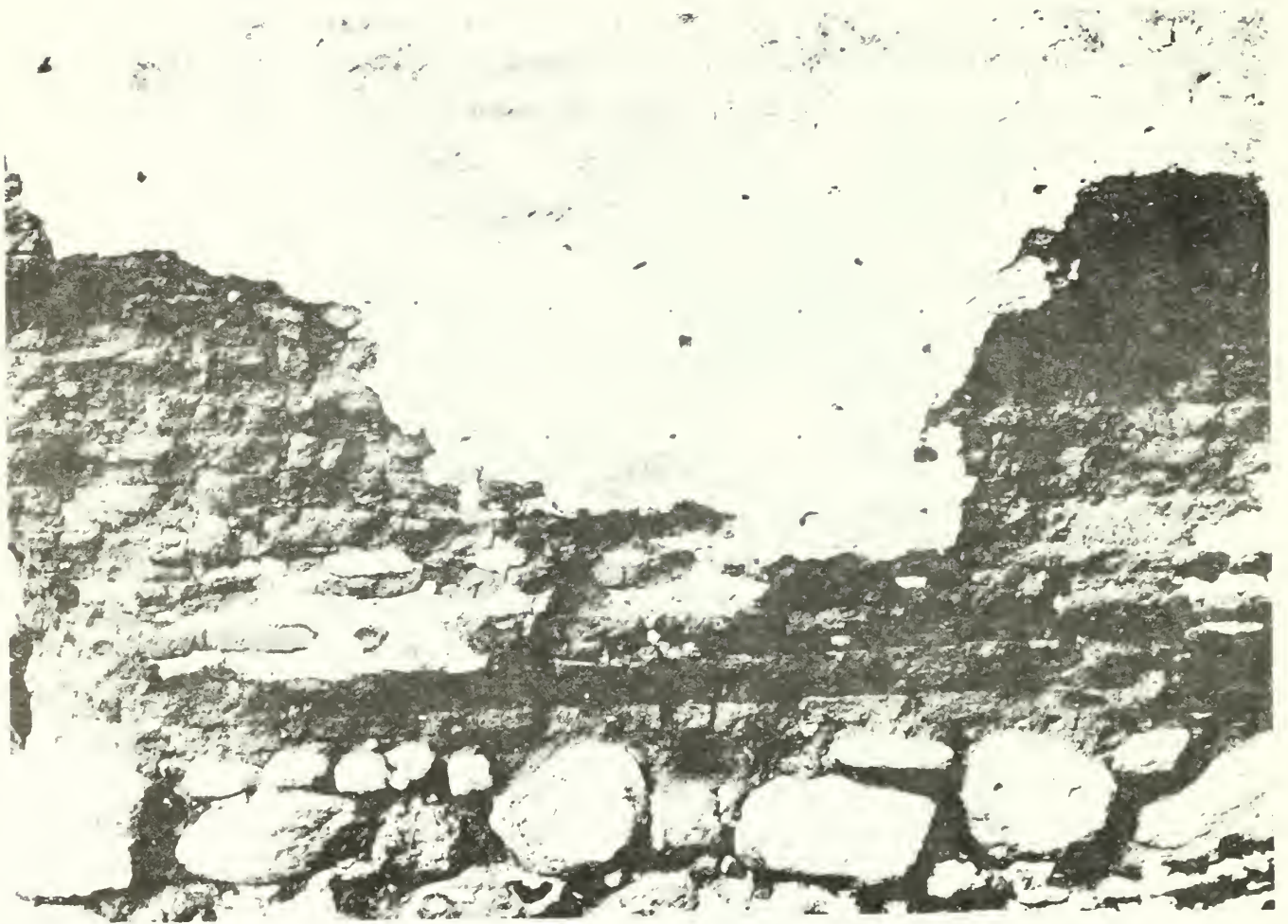
3. The north side of the bell tower after the removal of the hard cement stucco.
