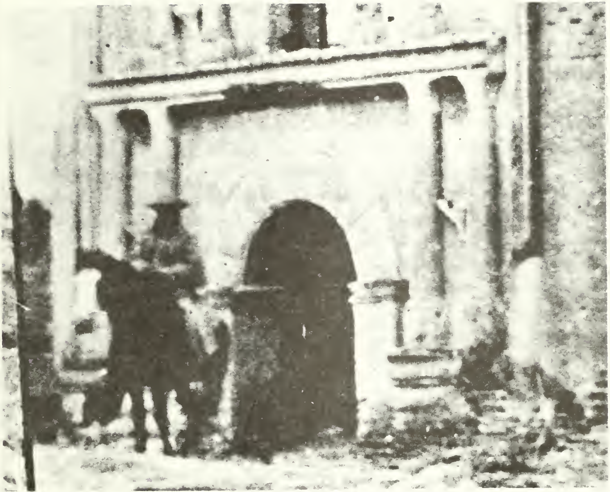
11. Detail of the front of the church ca. 1882.
