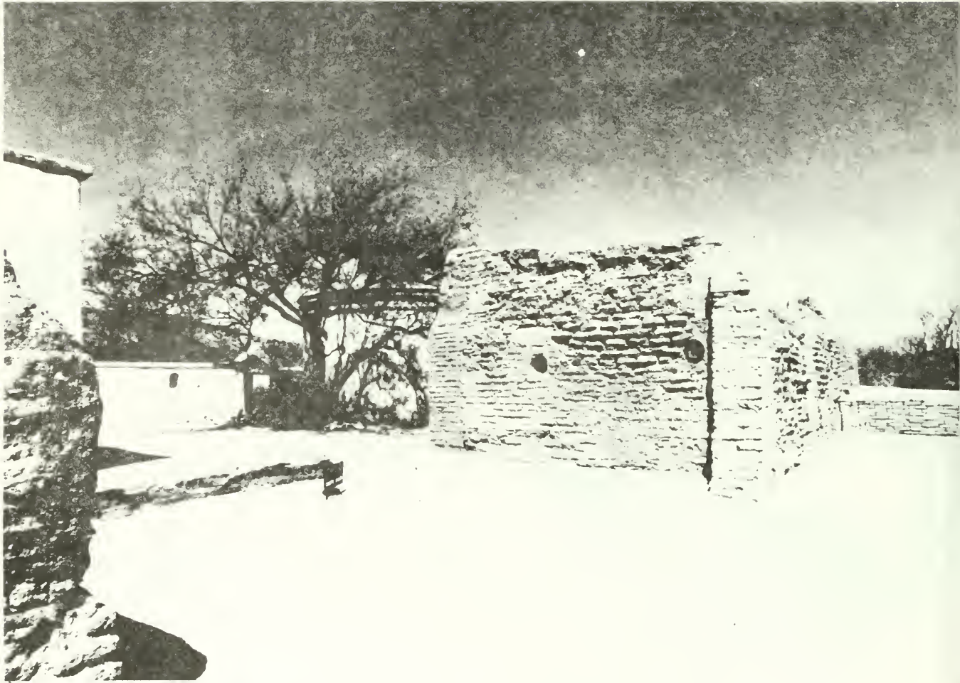
7. The granary from the southeast after the removal of the protective roof.
