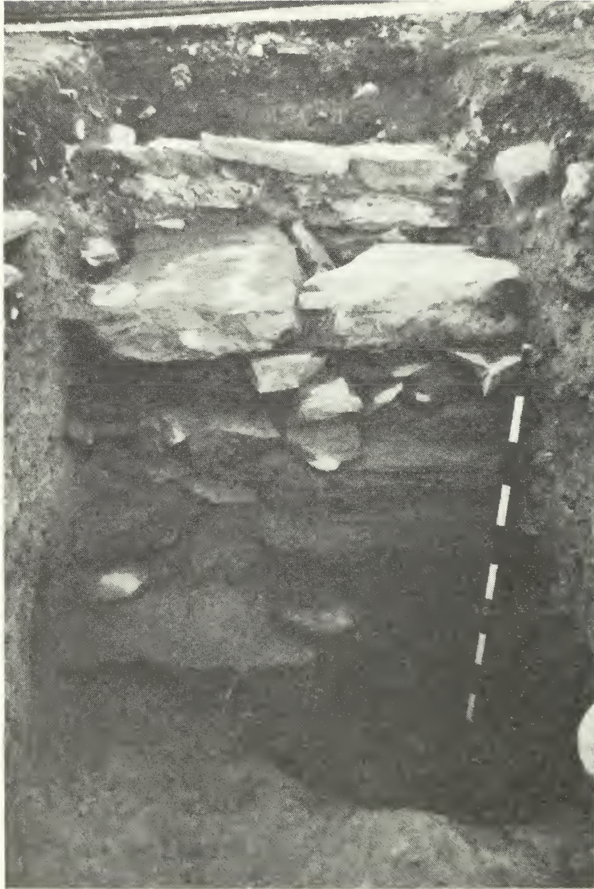
Figure 7-9. The exterior of Feature 1. The foundation was built of rough slate slabs derived from blasting out the ledge to construct the cellar. Camera faces east.
