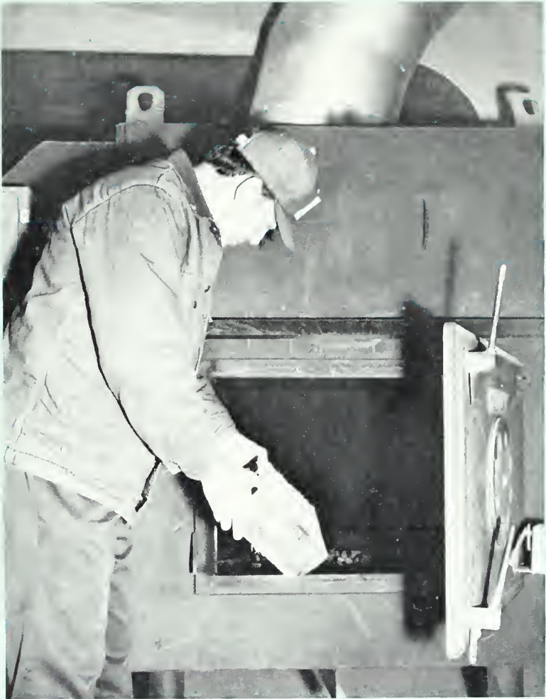
Wood is also being used for heating purposes in many commercial and industrial buildings around the state. Shown here is Marc Boyd of Boyd's Industrial Woodwork of Byron getting ready to fire up the big furnace of the Rettew System that provides comfortable heat for the employees of his 9,000 square foot plant. Boyd and his brother, Bob, co-owners of the manufacturing plant, had the system installed last year and they said they are well pleased with its efficiency. They burn scrap wood that formerly went to the trash pile. On cold days, wood is fed into the furnace at 7:30 a.m. and again at about 1:00 p.m. and that provides constant heat throughout the working day. Many plants, stores, shops and offices have converted to wood as a heating source, with manufacturing residue and forest waste wood making it economically feasible.
