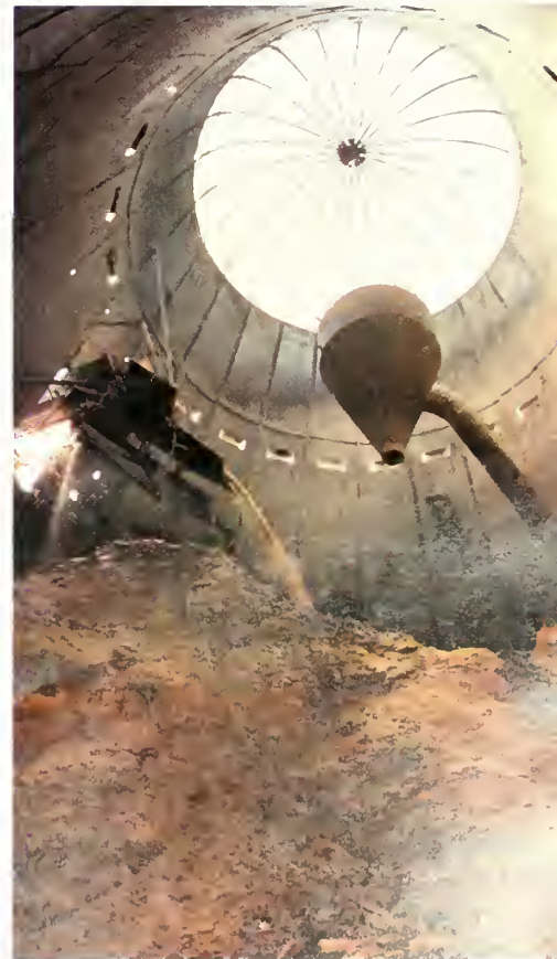
TODAY – Fuel Storage
