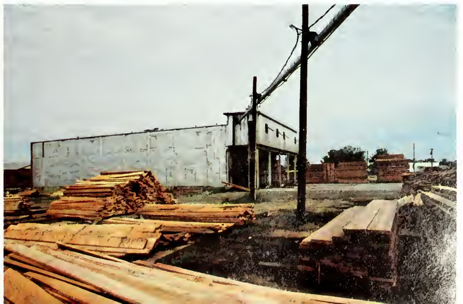
Modern lumber dry kilns are once more being operated with steam from wood residue boilers.
