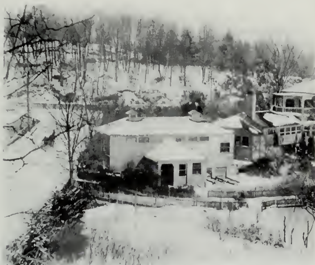
(2.52) View of office wing and service area, [ca. 1892-1900]. Photograph [probably by John Charles Olmsted].
