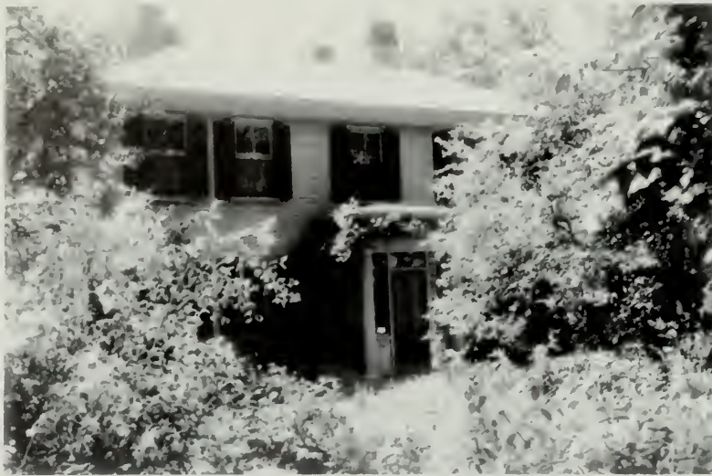
(6.1) North facade, 1964. Photograph #673-[not numbered] (loose photos).
