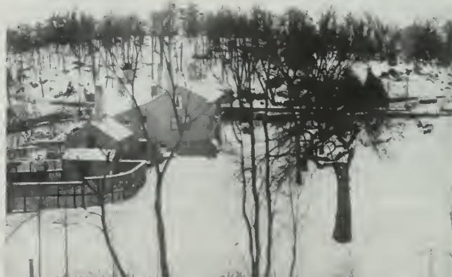
(2.35) View east over lawn and service area before barn was moved. Undated. Photograph by John Charles Olmsted, JCO-#3.
