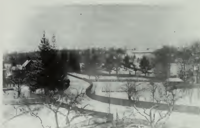
(2.50) View from second story toward Dudley Street and rear entrance, March 1885. Photograph by John Charles Olmsted, JCO-#61-62.
