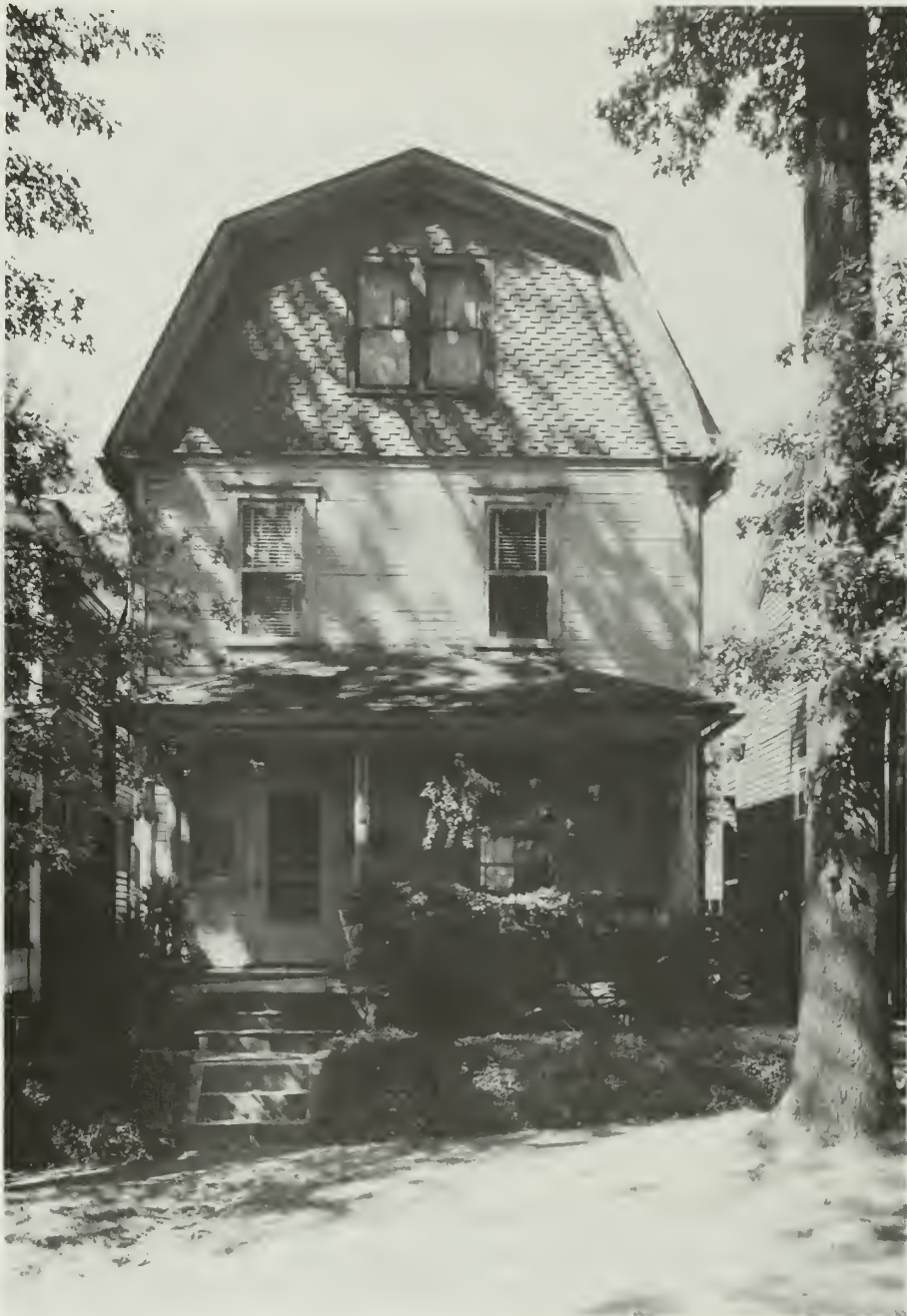
5.18 Peter Mulvehill House, 212 Mifflin St., Westmont. Peter Mulvehill, a laborer born in Ireland, purchased this lot from Cambria Iron in 1893 for $900; he built this house by 1895.
