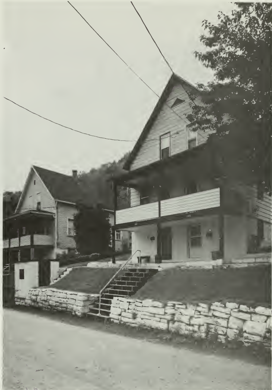
4.27 Cambria Iron Company House, 248-50 Iron St., Minersville. No. 248-50 Iron St. was part of a series of company houses built by Cambria Iron in Minersville after 1889. Each half of the building contained five rooms, a water closet, and running water and rented for $5.40 per month. John Martinek purchased this house in 1914 for $1,500, the standard price for these double houses.
