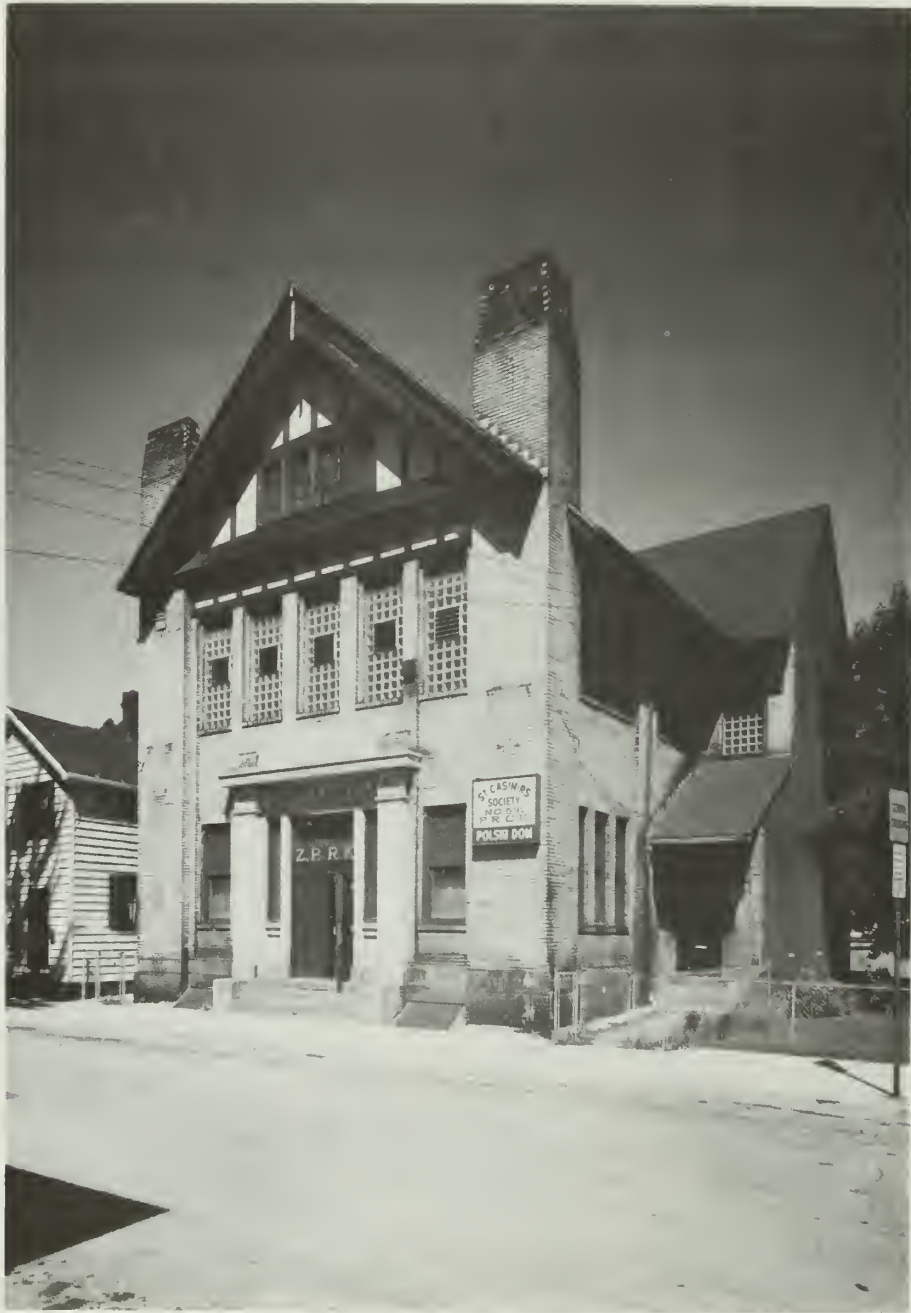
4.19 Dom Polski, 306 Power St., Cambria City. In July 1915, the Polish St. Casimir's Society awarded a contract for the erection of a clubhouse to contractor Charles A. Clawson. Architect Walter Myton planned the first floor to be used for "society rooms and club purposes" and designed the second floor as a ballroom.
