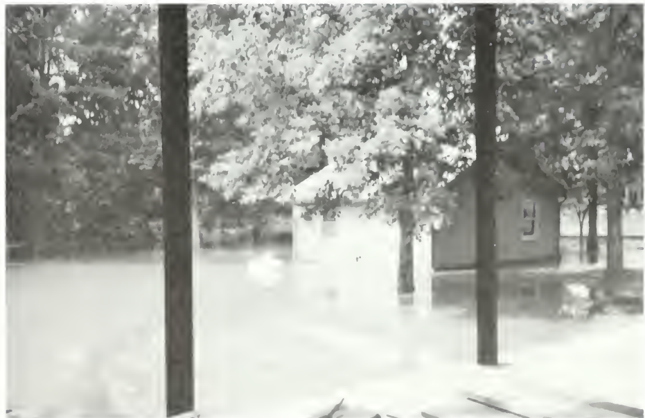
The office of the Macon County Forestry Unit, the only unit under water during the flood, had to be completed renovated inside.
