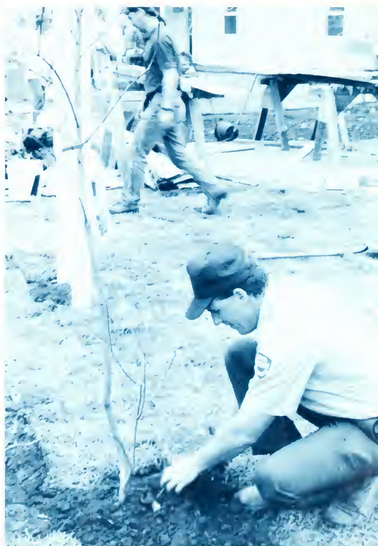
Foresters plant trees while other volunteers are involved in completing housing construction, landscaping and other work.
