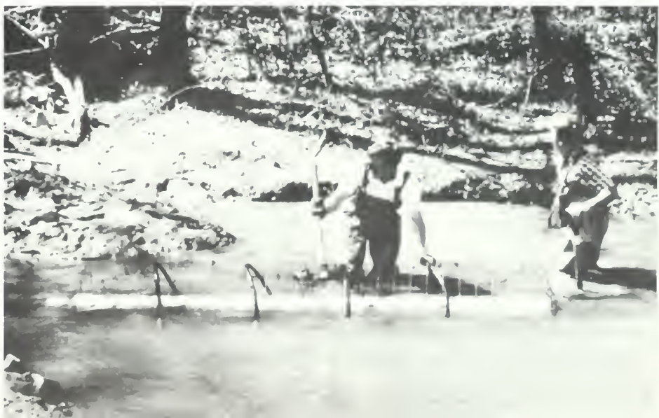
Chief Ranger Randy Kirksey of the Commission's Grady County Unit looks over a beaver dam that has caused backwater to kill a tract of timber. Below, a pond leveler is being installed at another site to help prevent timber loss due to flooding.
