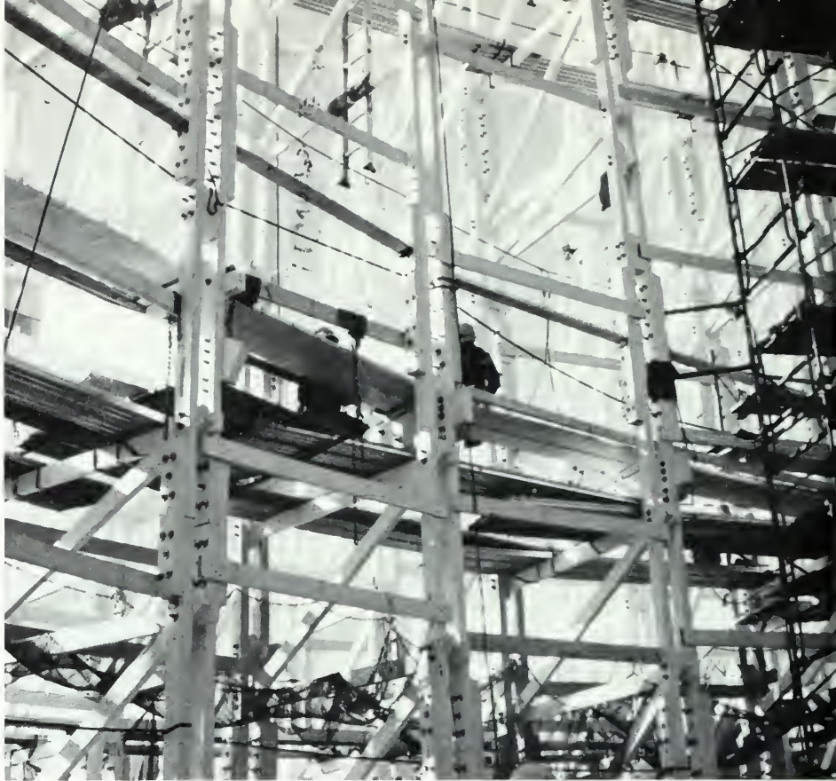
Like a giant erector set, roller coaster sections of the world's highest cyclone-style coaster are fastened together in Japan. Technical expertise and lumber were furnished by Atlanta's RCCA company.
