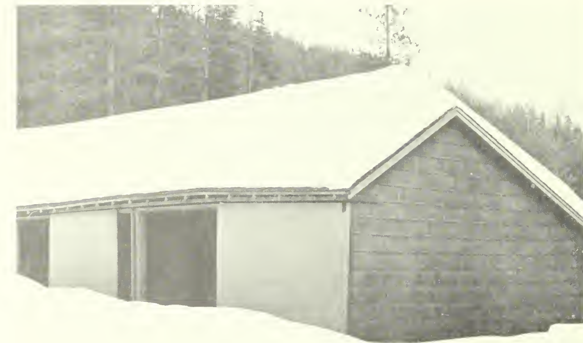
Figure 1.—Garage where snow accumulation was measured. Depth near eaves was about 40 inches on March 12, 1964.
