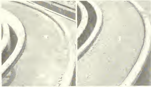
FIGURE 3. TYPICAL SECTIONS OF TRACK 1 AT 118,200 WHEEL-TRIPS, JUST BEFORE THE FIRST SPRINKLING. LEFT, SECTION 2, WHICH IS ALSO REPRESENTATIVE OF SECTIONS 1 AND 3; RIGHT, SECTION 5, WHICH IS ALSO REPRESENTATIVE OF SECTION 4.
