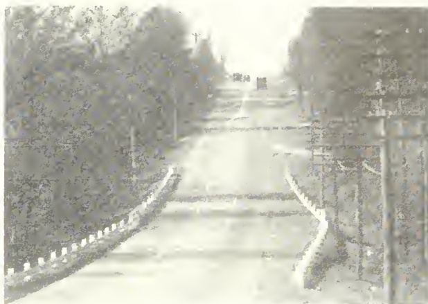
THREE-LANE HIGHWAY MARKED TO RESTRICT TRAFFIC TO TWO LANES OVER THE CREST OF A HILL WHERE SIGHT DISTANCE FOR UP-HILL TRAFFIC IS RESTRICTED. SUCH NON-DIRECTIONAL MARKING UNNECESSARILY RESTRICTS DOWN-HILL TRAFFIC WHICH HAS ADEQUATE SIGHT DISTANCE FOR PASSING, THUS ENCOURAGING DISREGARD FOR RESTRICTIVE LINE AND PASSING AS SHOWN.
