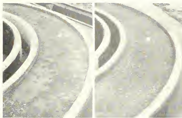
FIGURE 4.—TYPICAL SECTIONS OF TRACK 1 AT 151,200 WHEEL-TRIPS, JUST BEFORE CONSTRUCTION OF THE BITUMINOUS SURFACE. LEFT, SECTION 2, WHICH IS ALSO REPRESENTATIVE OF SECTIONS 1 AND 3; RIGHT, SECTION 5, WHICH IS ALSO REPRESENTATIVE OF SECTION 4.
