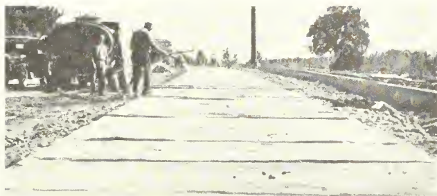
FIGURE 1.—COTTON MATS IN PLACE BEING WET DOWN.
