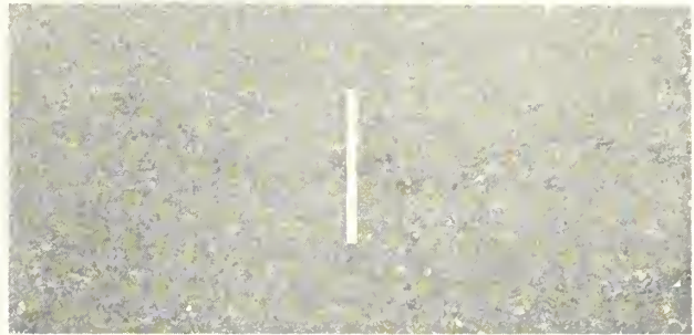
FIGURE 3.—TYPICAL FINE CRACK IN A HEAVILY REINFORCED SLAB CONSTRUCTED IN THE ARLINGTON CURING TESTS, 13 YEARS AFTER CONSTRUCTION.
