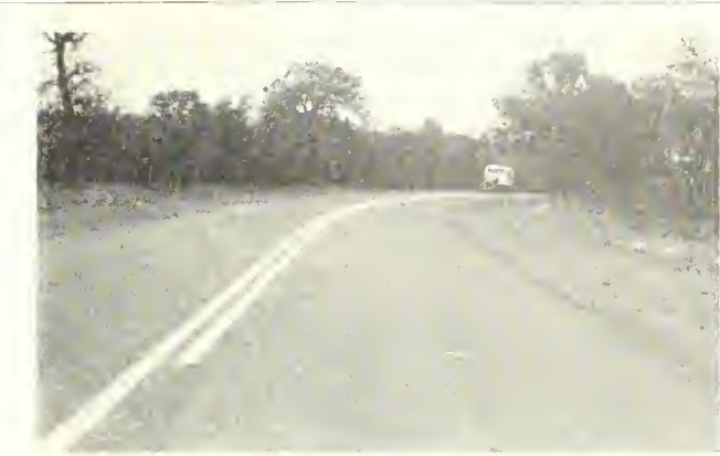
CENTERLINE STRIPE AND DIRECTIONAL STRIPE TO RESTRICT TRAFFIC APPROACHING THE CURVE. THE MARKING WOULD BE MORE EFFECTIVE WERE THE CENTERLINE STRIPE BROKEN INSTEAD OF SOLID OR DIFFERENT IN WIDTH OR COLOR.
