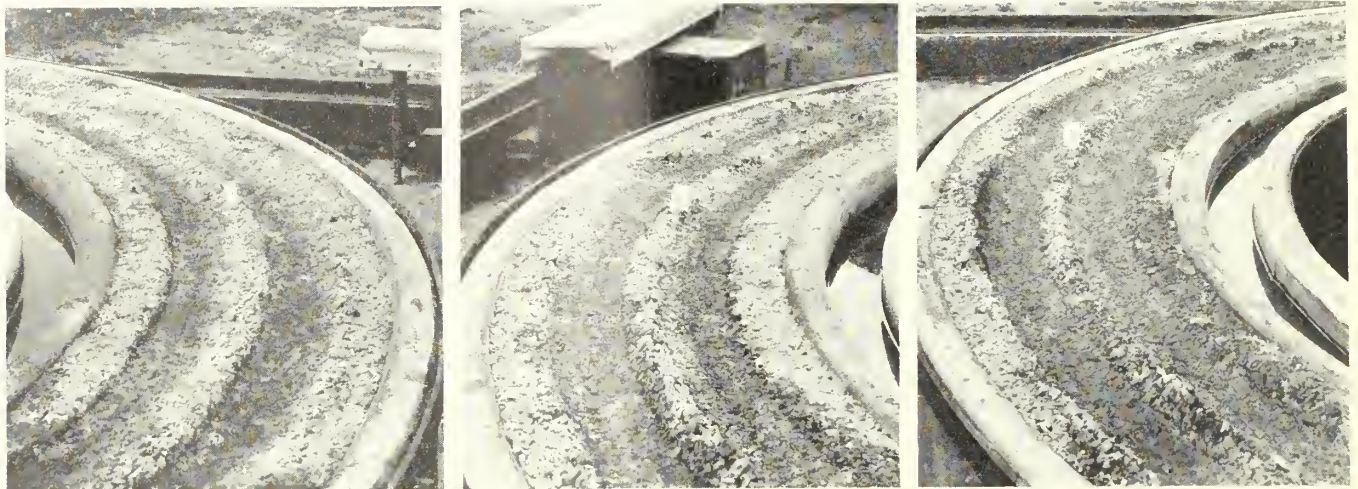
FIGURE 9.—SECTIONS OF TRACK 2 AT THE CONCLUSION OF THE TEST. LEFT, SECTION 1; MIDDLE, SECTION 3, WHICH IS ALSO REPRESENTATIVE OF SECTIONS 2 AND 4; RIGHT, SECTION 5.
