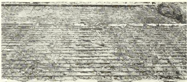
FIGURE 11.—SHEAR DOWEL BARS IN PLACE AT LOCATION WHERE WEAKENED-PLANE JOINT IS TO BE FORMED.
