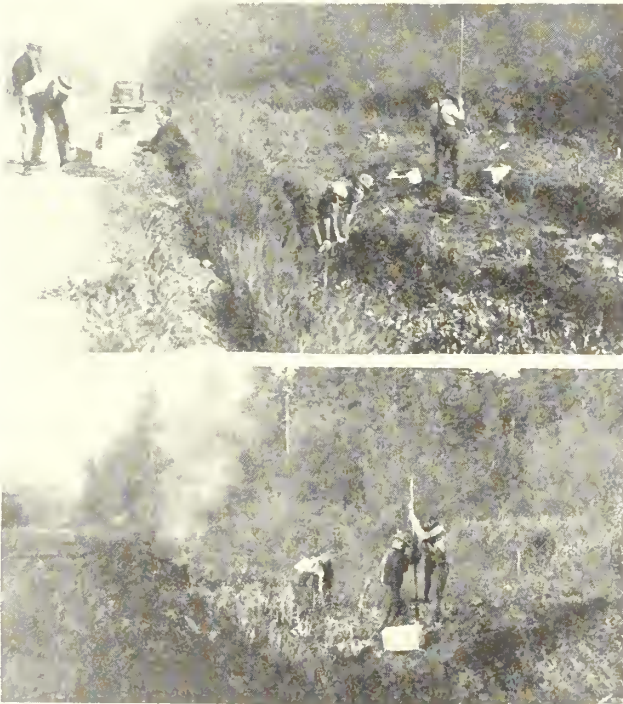
FIGURE 5.—PUNCHING AND LOADING HOLES FOR SWAMP MAT BLASTING.
