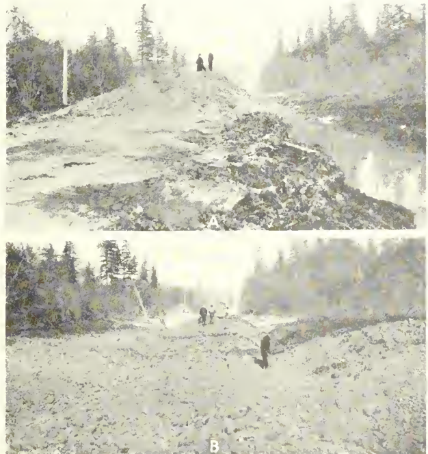
FIGURE 8.—A, OLD ROAD LOADED WITH BORROW MATERIAL BEFORE UNDERFILL BLASTING; B, THE SAME SECTION OF ROAD SHOWN IN A AFTER BLASTING. THE FILL MASS SETTLED APPROXIMATELY 15 FEET. NOTE THE SWAMP MUCK PUSHED OUT ON EACH SIDE.
