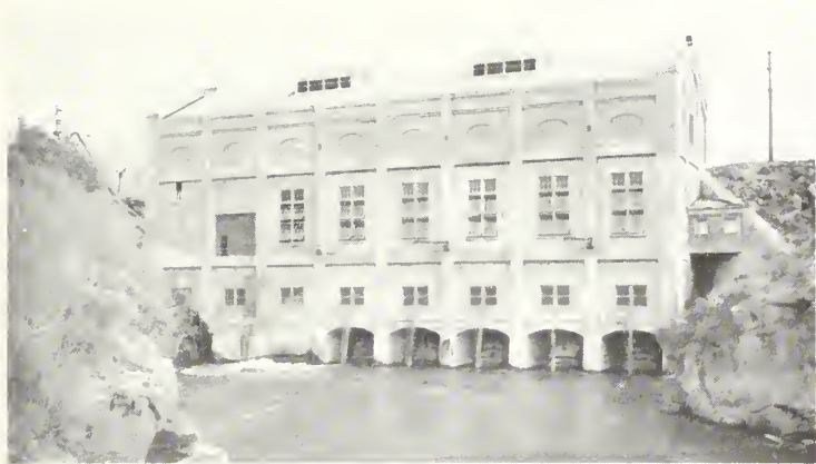
Minidoka Power House, downstream side
