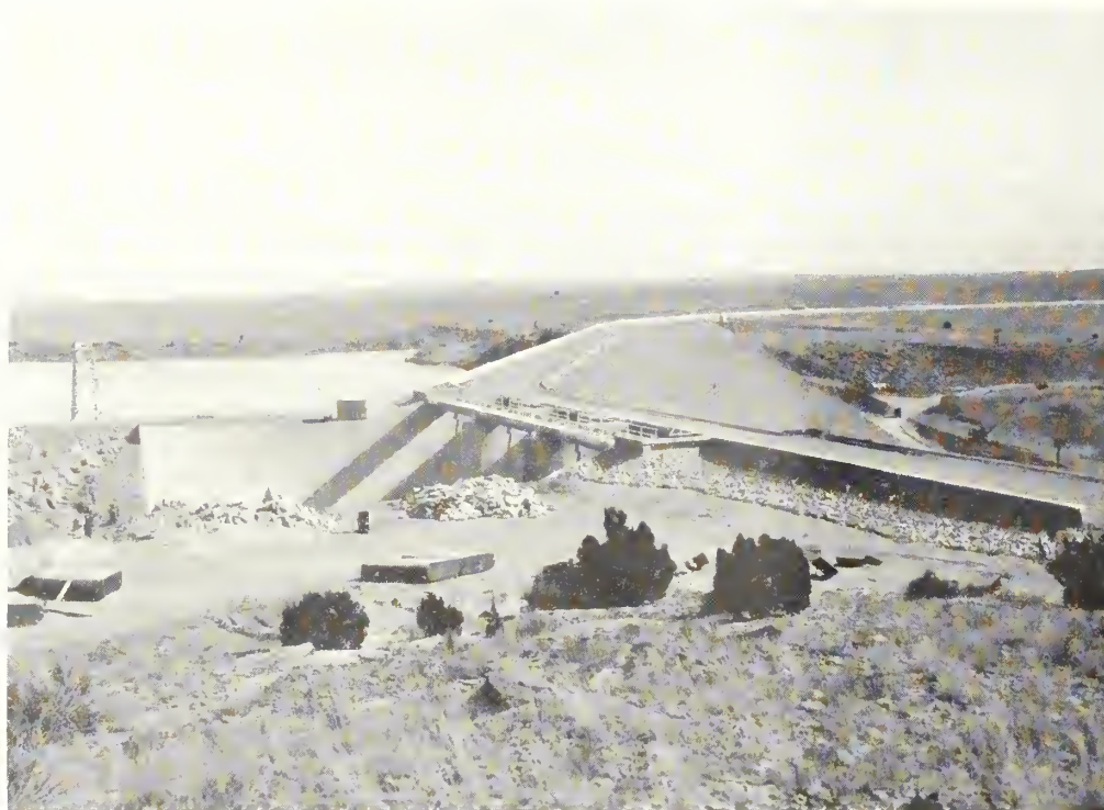
Spillway, dam, and dike looking east
