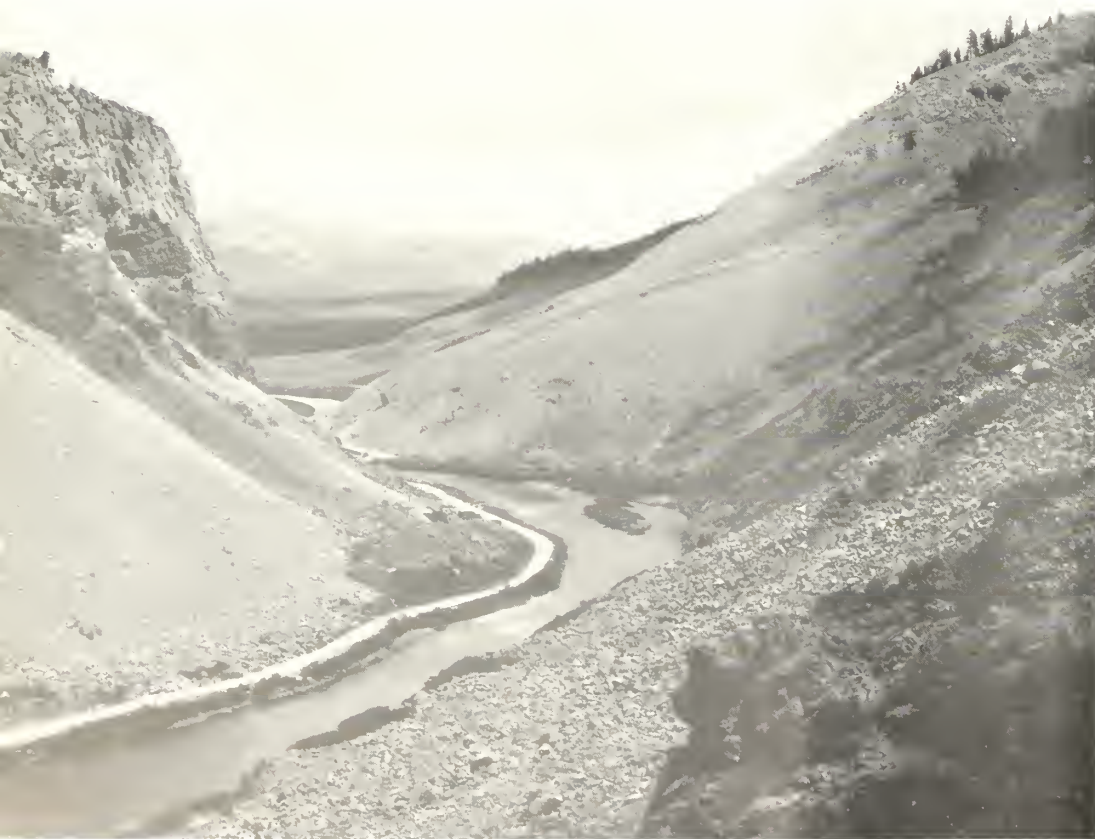
View of dam site from opposite the outlet works.
