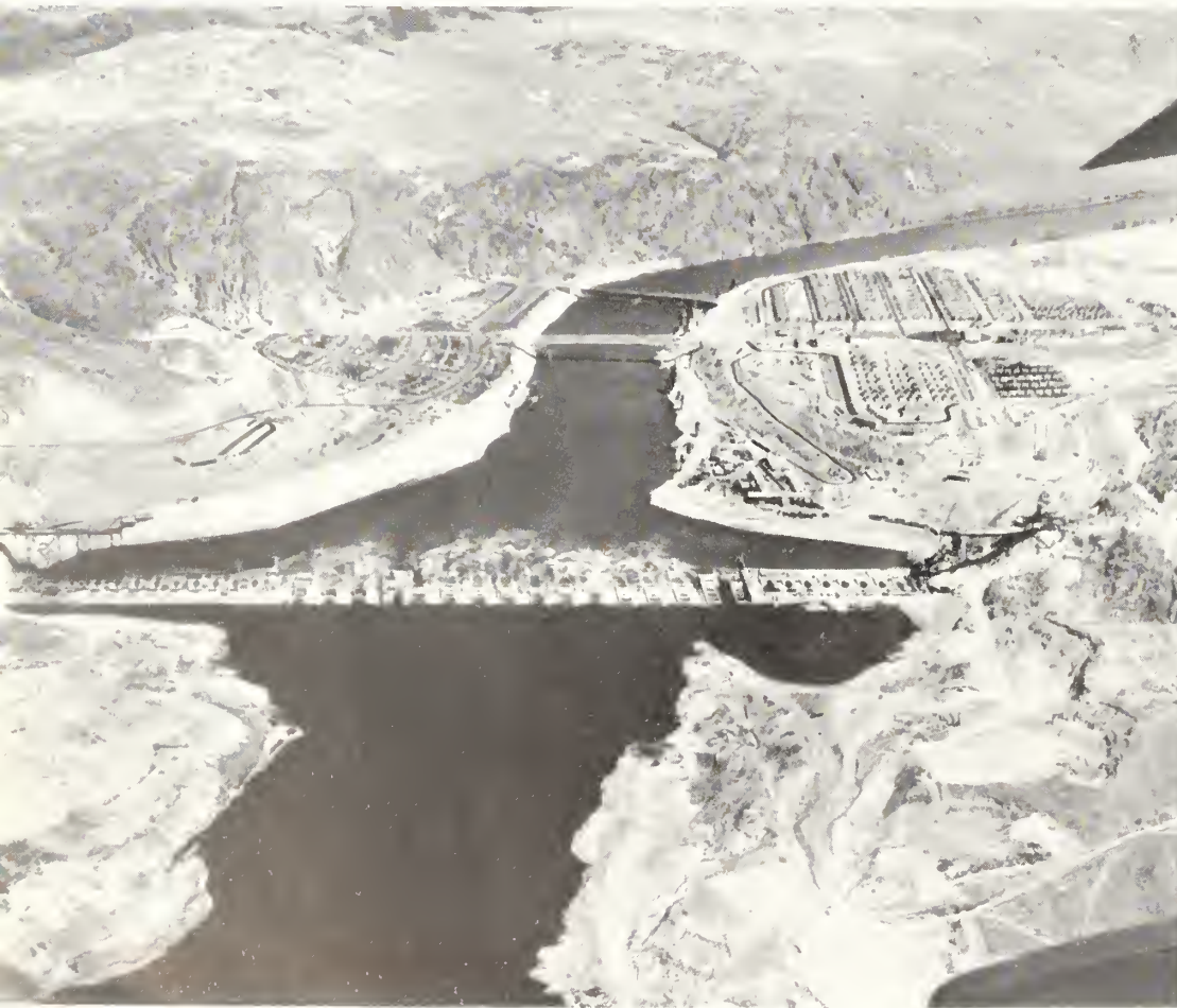
Grand Coulee Dam, Columbia Basin project, Washington This view greeted visitors to the dam in July 1938
