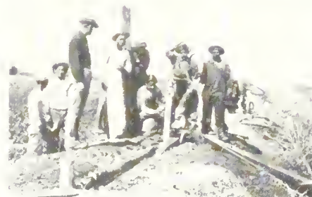
Crews of enrollees from CCC Camp BR-4, located at Ysleta, Tex., digging trench down a canal bank in which concrete is poured to stop gophers burrowing through. Lower right, placing precast concrete slabs for the same purpose.
