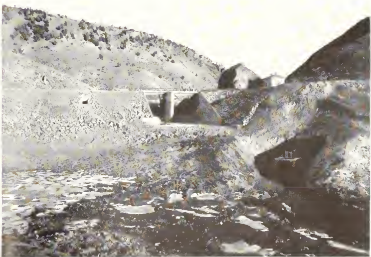
Upstream view of completed dam.
