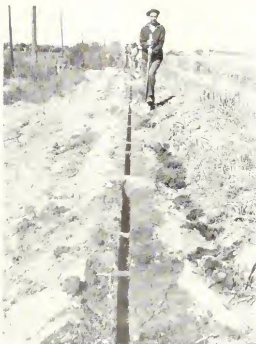
Crews of enrollees from CCC Camp BR-4, located at Ysleta, Tex., digging trench down a canal bank in which concrete is poured to stop gophers burrowing through. Lower right, placing precast concrete slabs for the same purpose.
