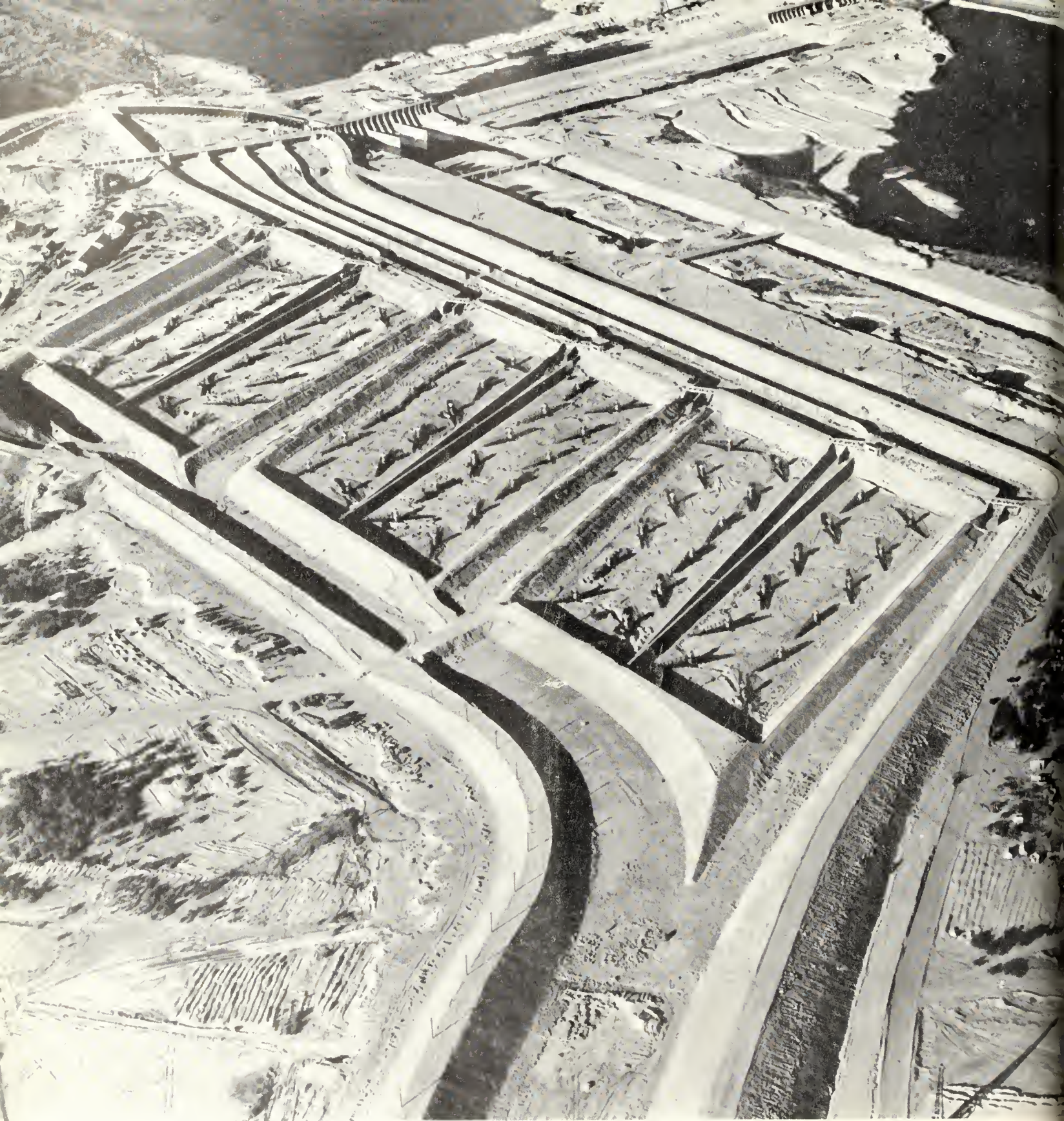
DESILTING WORKS, ALL-AMERICAN CANAL; IMPERIAL DAM, UPPER RIGHT
