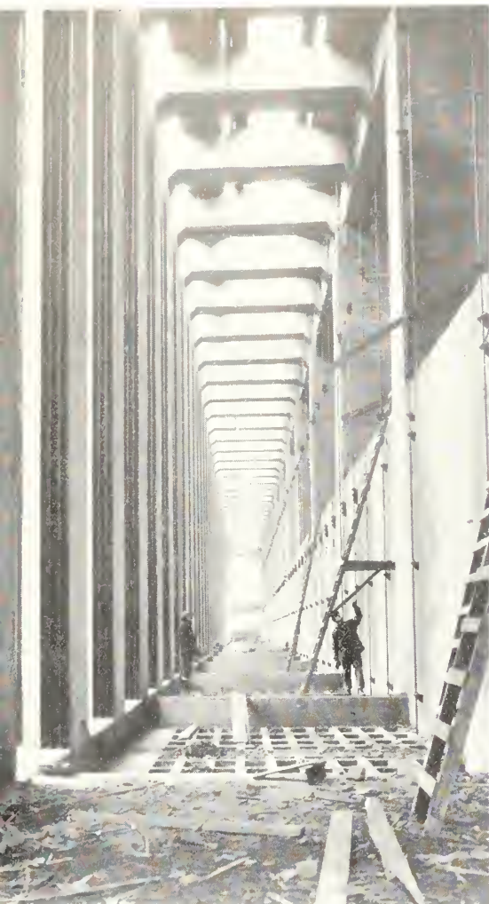
Bonneville Dam. Collection channel along face of powerhouse.
