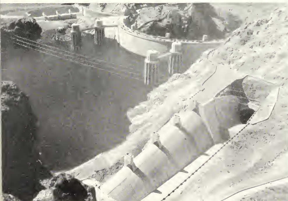
Upstream face of Boulder Dam, spillways, and intake towers, taken from Nevada side. Lake Mead, when this picture was taken, contained 16,650,000 acre-feet. The reservoir has a capacity of 30,500,000 acre-feet
