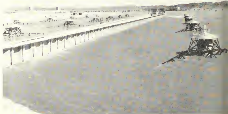
Clarifiers clear water of silt
