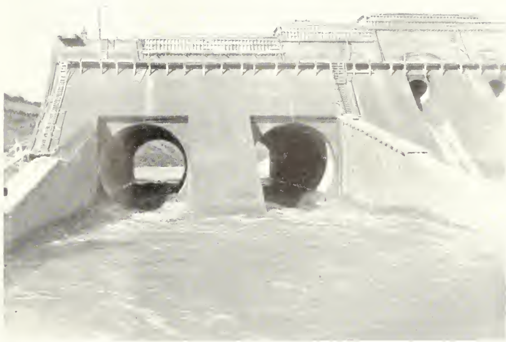
Diversion of Colorado River of Texas through Marshall Ford Dam was accomplished May 24, 1938. The conduits shown are 26 feet in diameter; the discharge at the time of this exposure was approximately 1,000 second-feet
