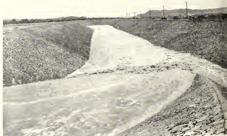
Diverted at Imperial dam, the Colorado River enters All-American Canal. Twenty miles of the 80-mile canal are now ready for seasoning
