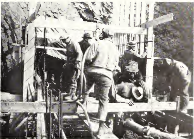
Dam site and clearing operations.
