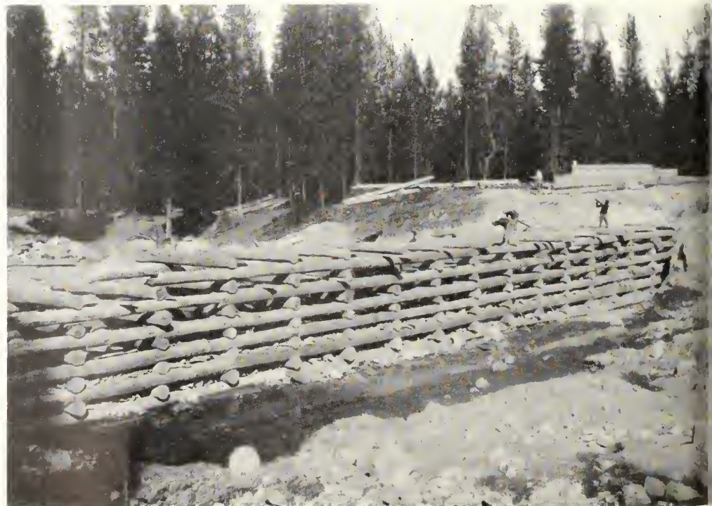
Cascade Creek diversion dam
