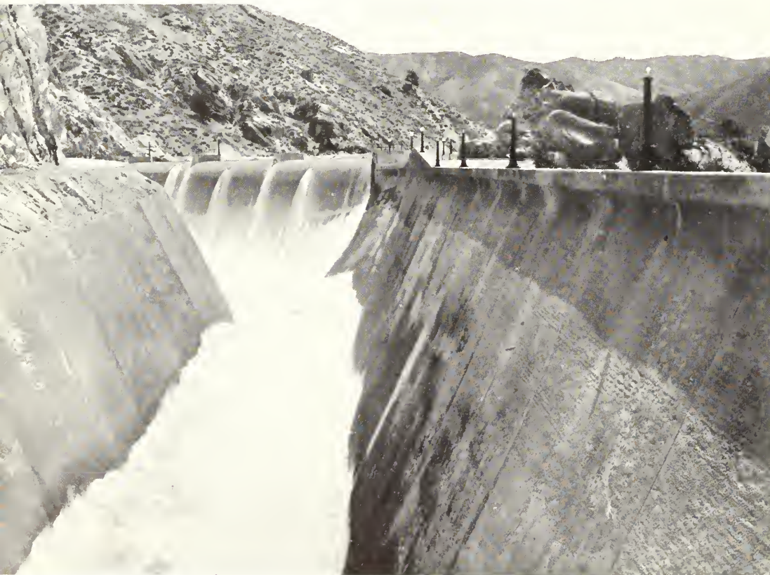
Upstream view of Arrowrock Dam spillway carrying 6,822 second-feet
