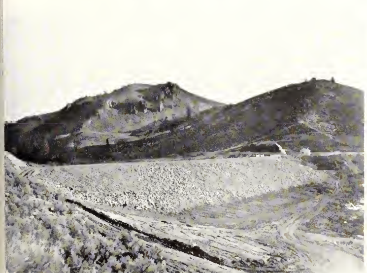
Spillway inlet, tunnel inlet, and control house.
