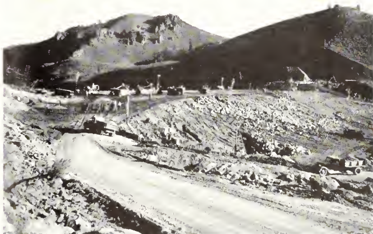
Ten-day progress view of earth fill.
