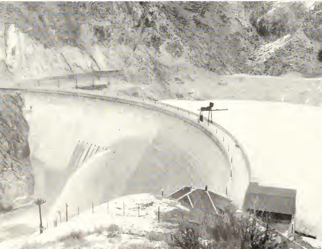
Arrowrock Dam, Boise Project, Idaho, showing newly surfaced face
