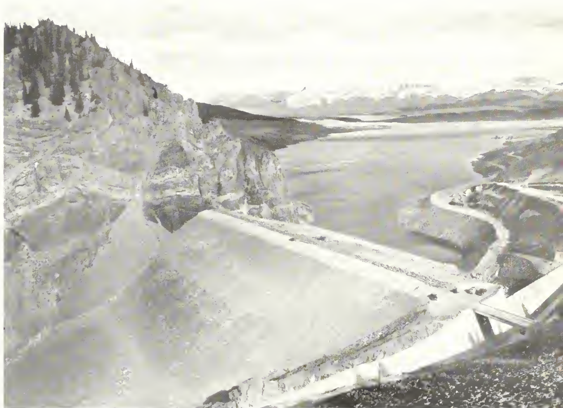
Earth- and rock-fill complete except parapet wall, lower road, and spillway.
