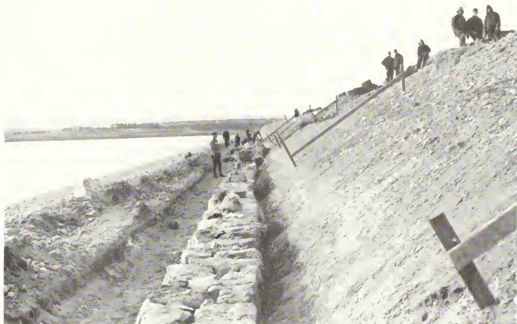
Toe wall and gravel slope ready for rock riprapping
