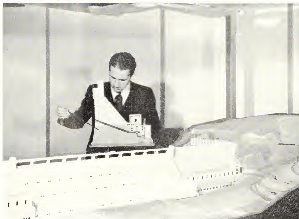
A demonstrator with a model of the cross-section of the dam and powerhouse
