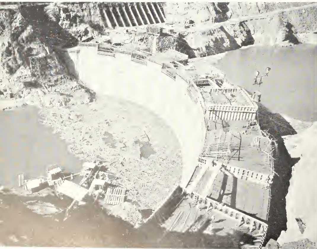
Parker Dam and trashrack structure shown from above Arizona abutment.
