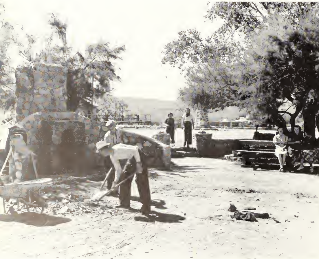
Park improvements built by CCC at Leasburg Dam, Rio Grande Project, New Mexico-Texas.
