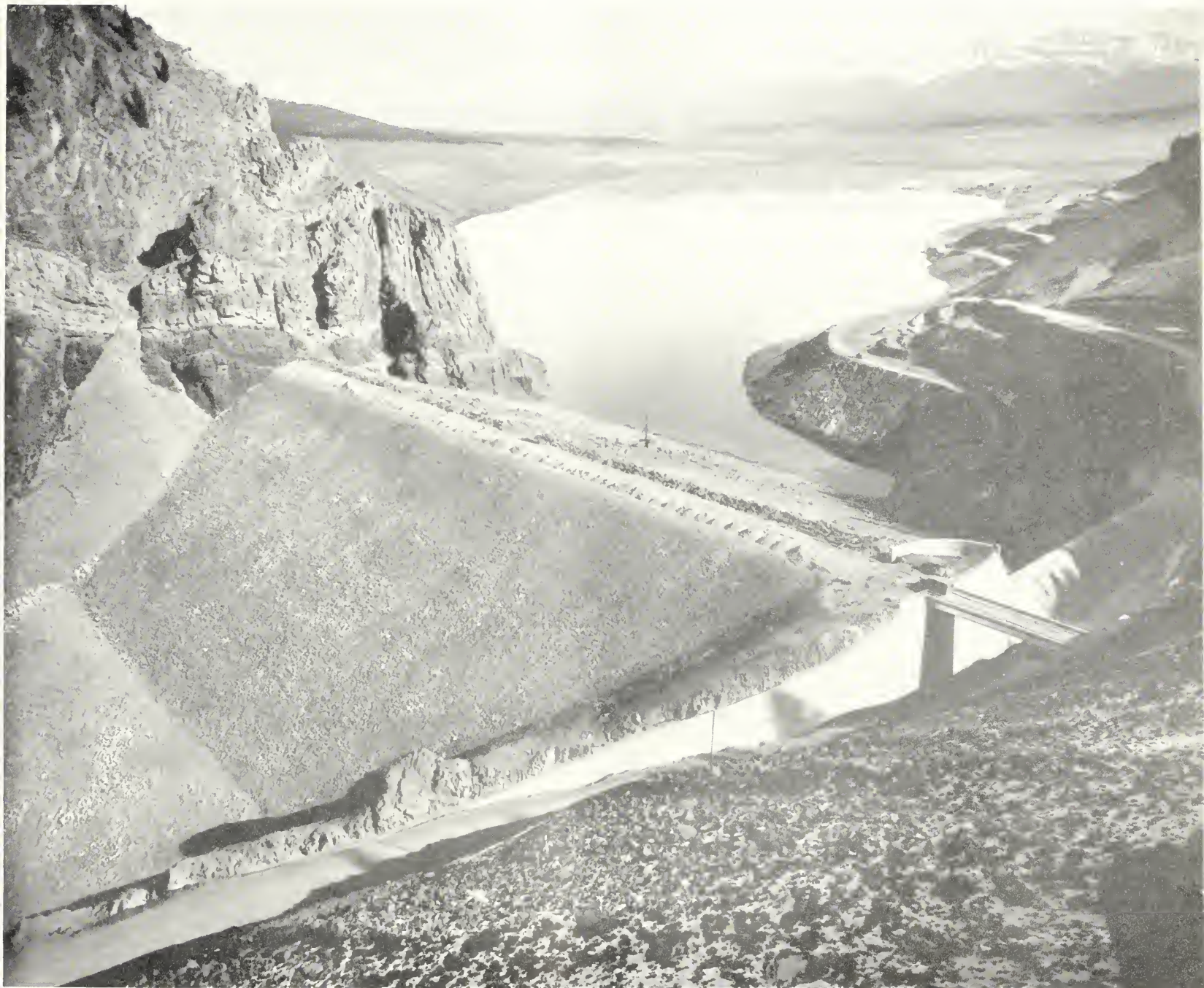
Taylor Park Dam, Uncompahgre project, Colorado, recently completed by the Bureau of Reclamation to supply a supplemental water supply for the project. Of earth-filled construction, Taylor Park Dam is 168 feet high and has created a reservoir on the Taylor River, a tributary of the Colorado, of 106,200-acre-feet capacity. Already 10,000 acre-feet are stored. The dam will begin regulation of this river next spring.
