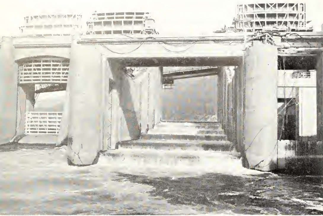
Bonneville Dam. Looking upstream through temporary fish ladder in bay No. 18 at south end of spillway dam.
