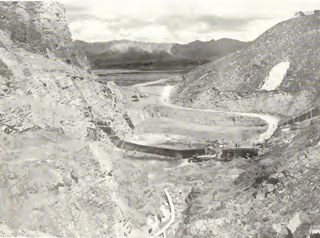
Starting earth-fill between first and second cut-off walls.
