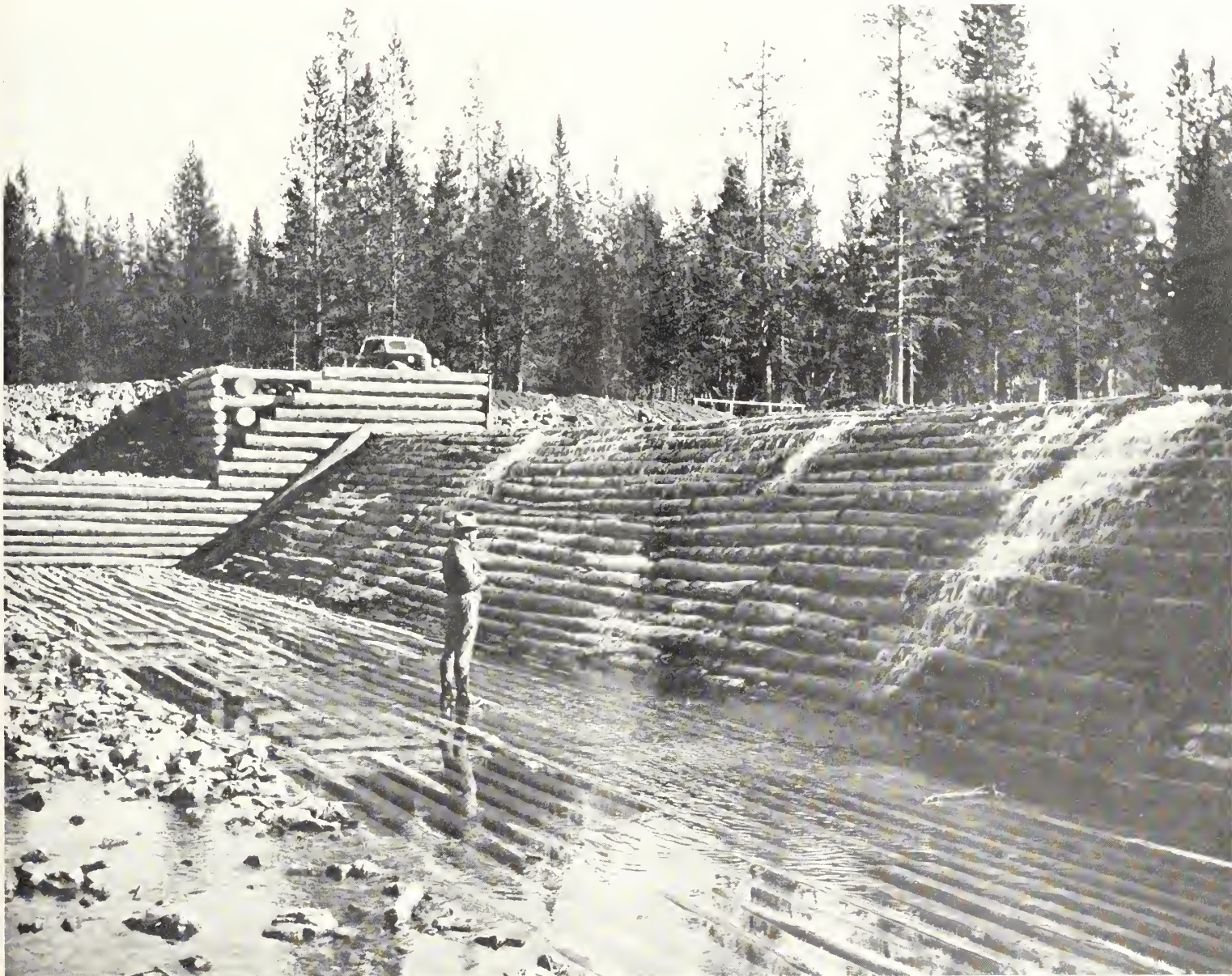
The Cascade Creek Diversion Dam, a part of the new Upper Snake River Project, Idaho, designed to serve irrigators of the Snake River Valley with supplemental water. The dam is of rock-filled, log-crib construction.
