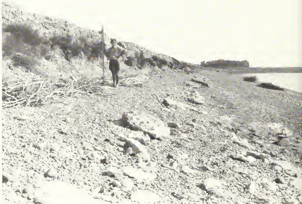
Upstream face lower embankment prior to reconstruction
