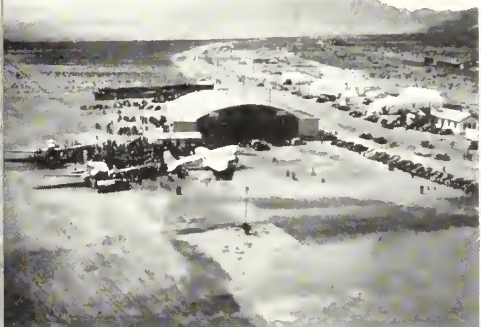
Boulder City airport on occasion of TWA schedules April 3, 1938, when an impromptu rodeo was staged. Work of extending and surfacing the runways was done by CCC forces
