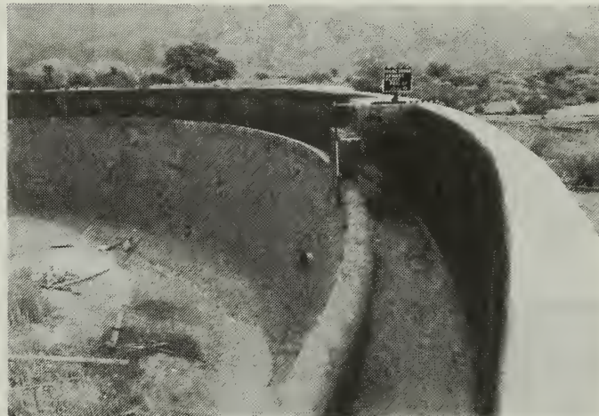
Figure 10.39. Detail of Clarifier (MANZ 1993 B-28, Feature 4).
