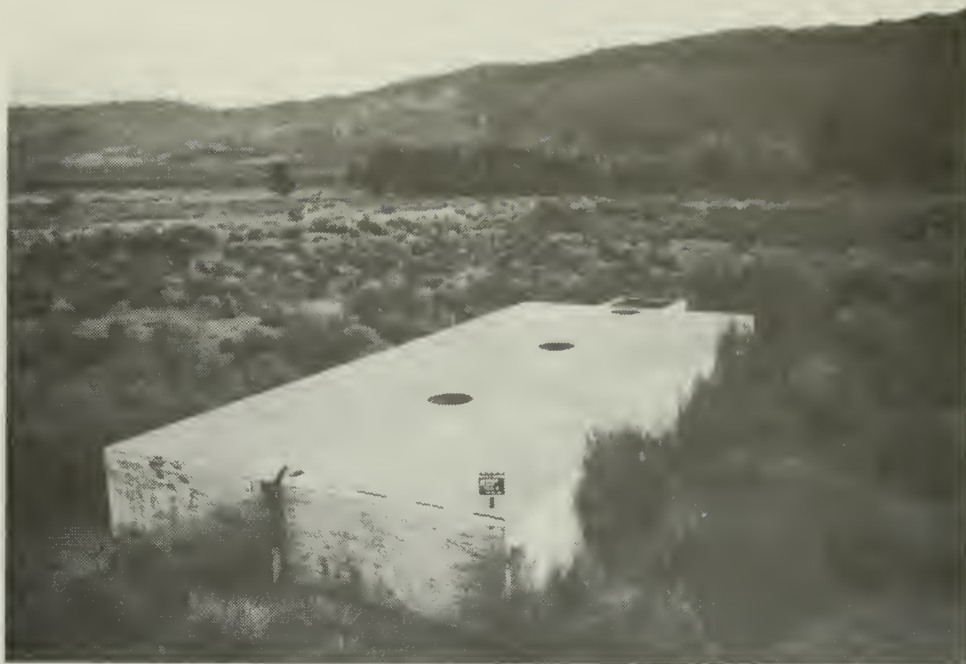
Figure 10.41. Chlorine Contact Tank (MANZ 1993 B-28, Feature 5).
