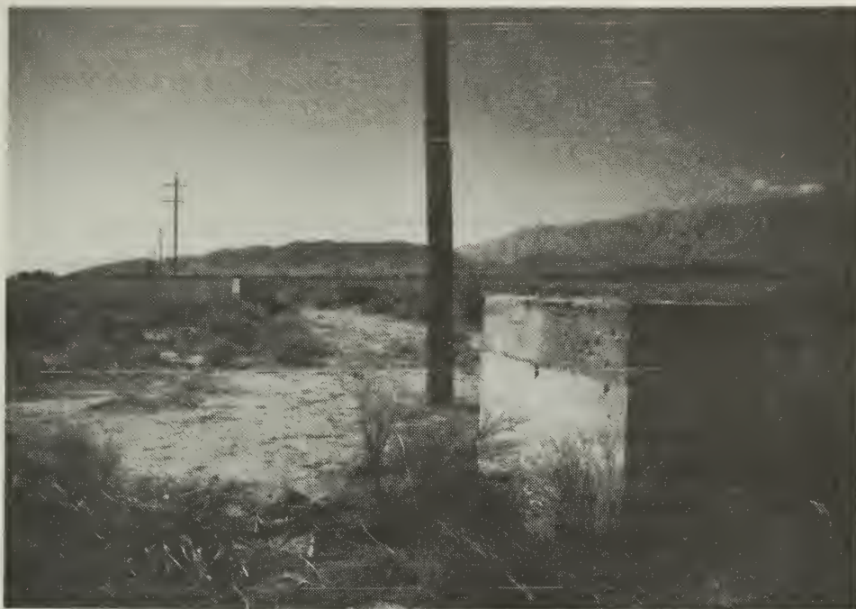
Figure 12.65. Concrete diversion boxes (MANZ 1994 A-6).
