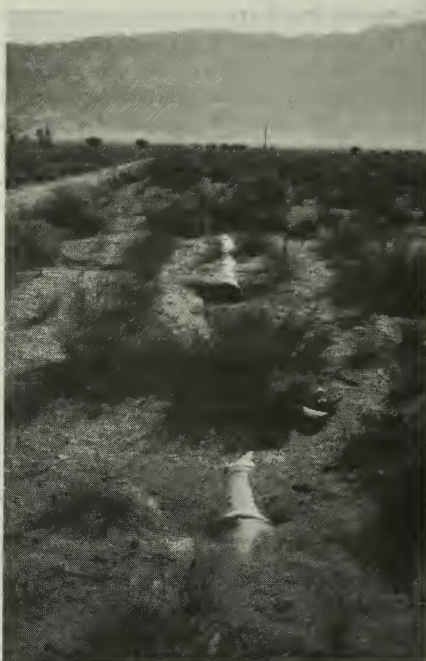
Figure 12.69. Exposed concrete pipeline (MANZ 1994 A-5).
