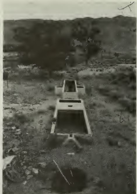
Figure 10.35. Detail of headworks showing grit chamber and flow meter structure (MANZ 1993 B-28, Feature 2).
