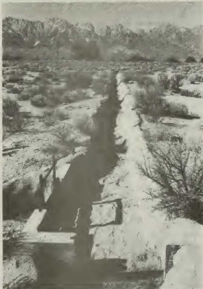
Figure 10.59. Concrete-lined ditch and sluice box (MANZ 1993 B-12, Feature 3).
