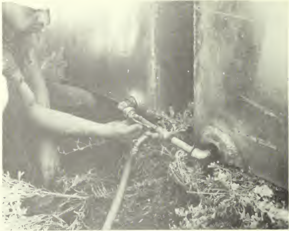
Figure 3.--Siamese coupling between storage tanks showing valve and plastic gravity hose.
