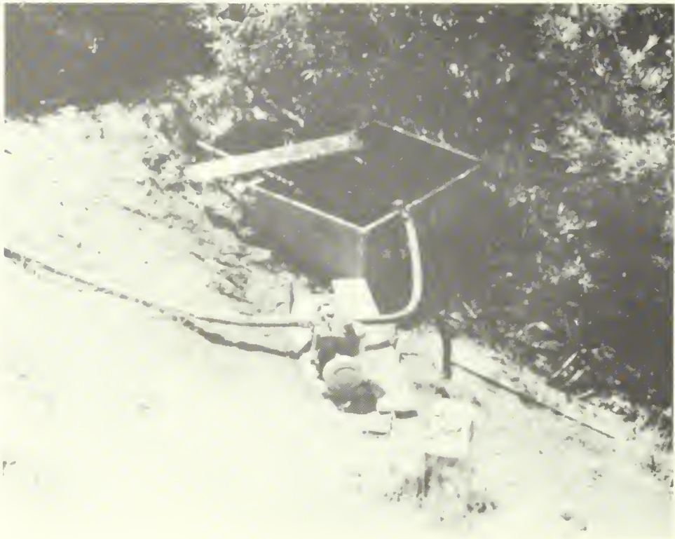
Figure 1.--Typical water development in small stream showing earthen dam, water supply pipes, open-top tank, suction hose, pump, and discharge hose.
