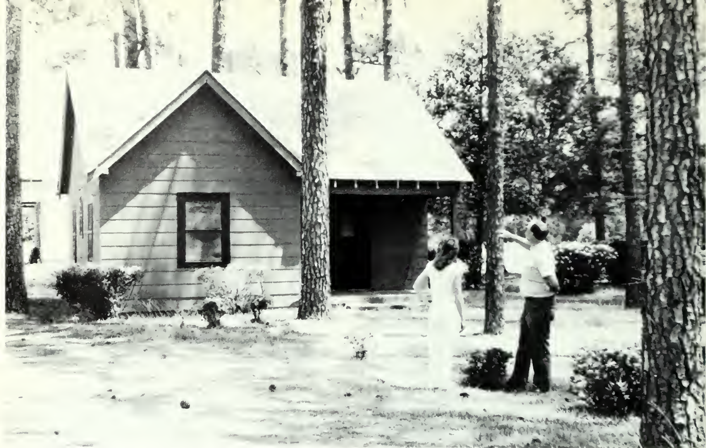
This little office building in Nahunta, constructed almost 50 years ago by the Civilian Conservation Corps, is said to have been the first county unit building in the Commission. It was occupied by the Brantley County Unit until last year, when the office was moved to spacious new quarters two miles east of the city. Forest Ranger Barry Chesser is shown pointing out the historic and now vacant building to a visitor to his city.
