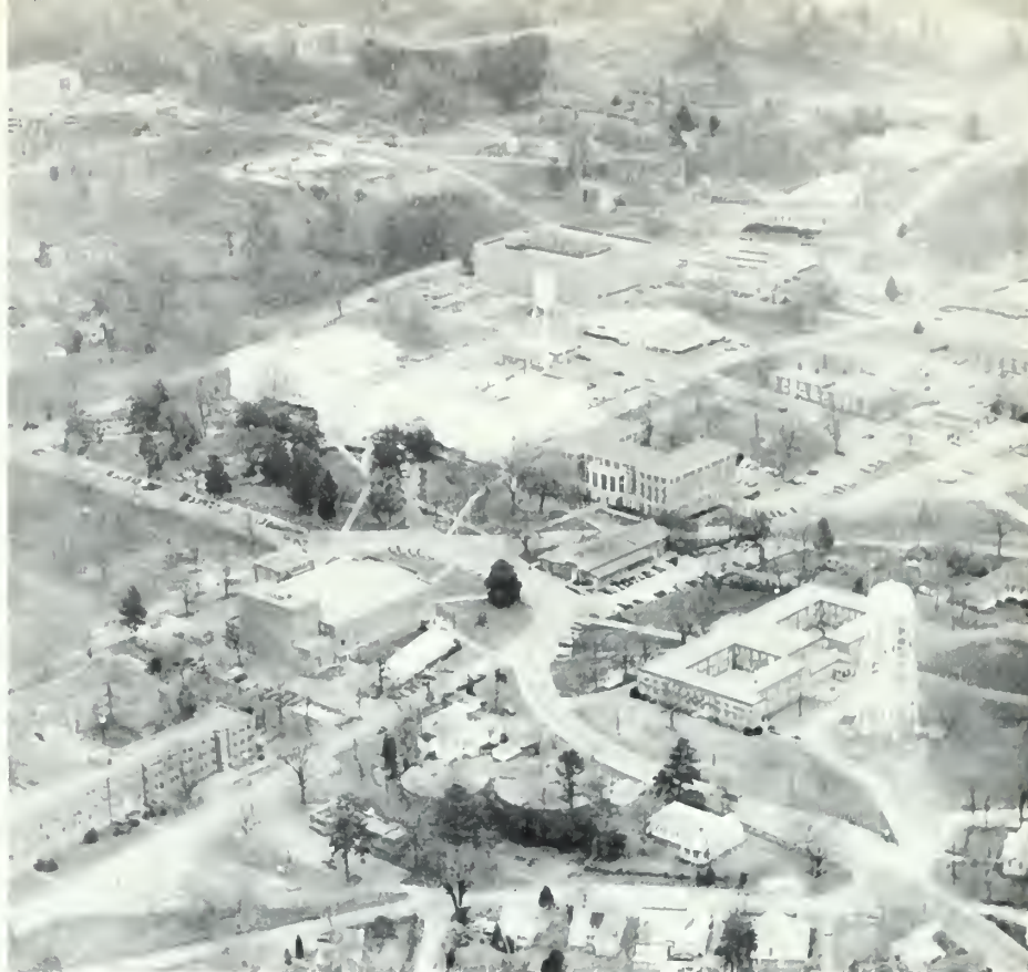
Sprawling hospital and prison complex now depends on wood energy system for heating and cooling.
