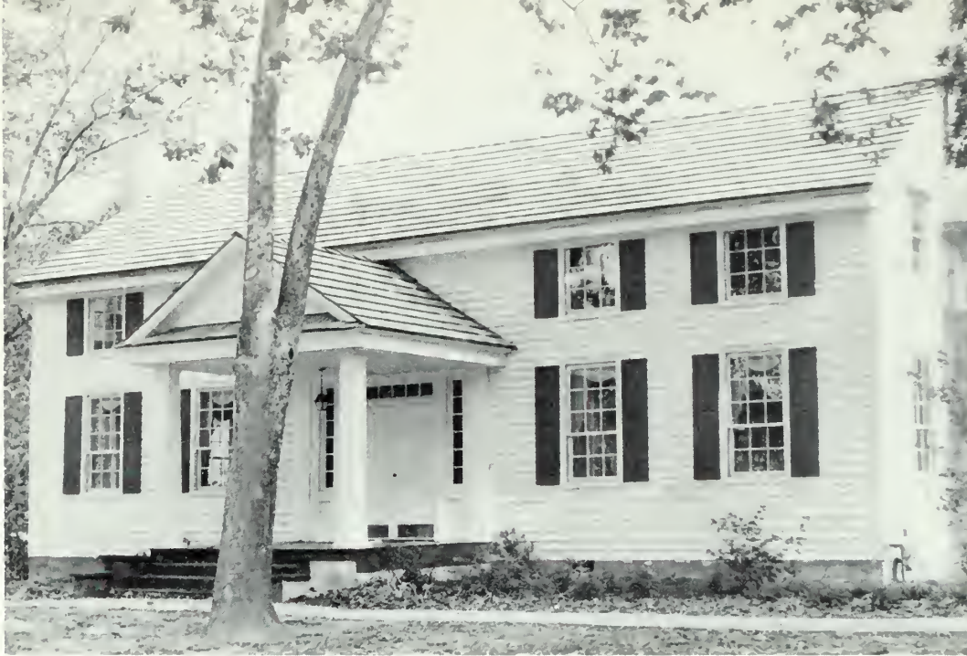
Historic Mable House in Mableton, originally roofed with pine shakes when it was constructed of heart pine in 1843, was recently reroofed with Southern yellow pine shingles to enhance authenticity. The antebellum home, named after Robert Mable, serves as a Cobb County Center for the arts, business groups and civic program. A thousand-seat amphitheater is scheduled to be constructed behind the house.
