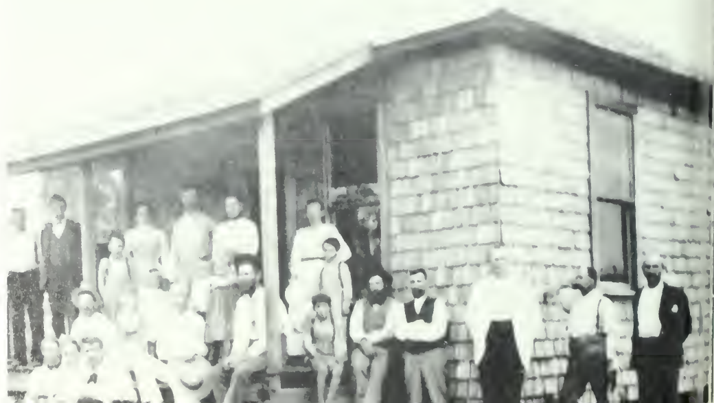
This 1902 photo of a South Georgia house shows how previous generations used indigenous wood species for roofing. These shingles (or shakes) are probably all Southern yellow pine cut from nearby forest land. This particular house, apparently the site of a family reunion, also indicates an unusual enthusiasm for the use of pine shingles, since the entire house is covered with them. (Georgia Archives photo.)
