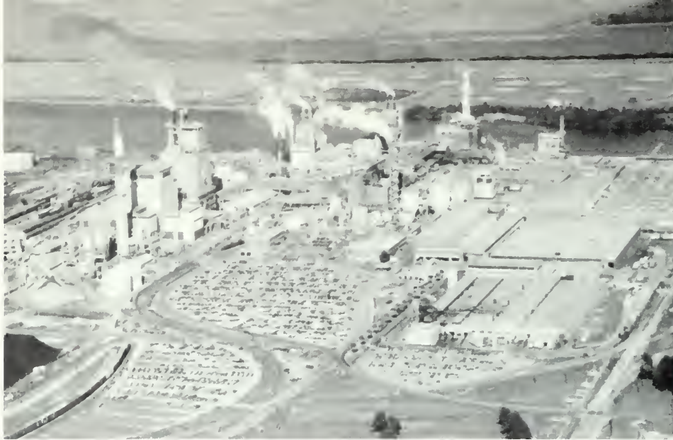
Aerial view of Union Camp Corporation's Savannah mill.
