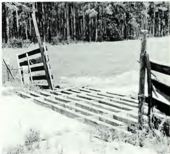
They are not as common as they were years ago, but cattle gaps are still found in rural Georgia. This device in Irwin County is typical of gaps farmers use in lieu of a gate to keep livestock fenced in.
