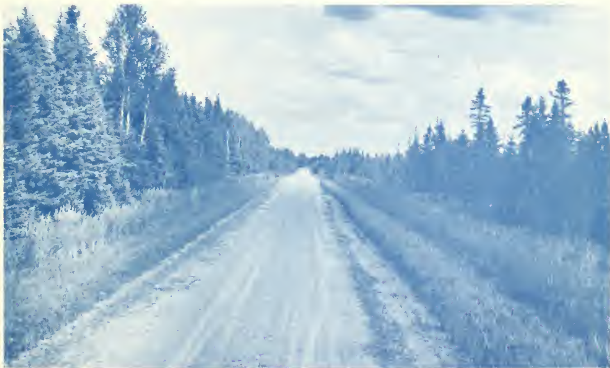
Figure 1.—Trees at the right on the "uphill" side of this road crossing a black spruce swamp show depressed growth and poor vigor compared with the normal trees at left on the "downhill" side. Because no culvert was used here the water table was raised about 10 inches. Cattails predominate on the flooded side of the crossing showing site retrogression. Alder, fern, and willow make up the ground cover on the other side.
