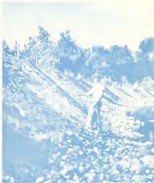
Figure 1.—Liquid mulch being sprayed on a bank above rock rip-rap.
