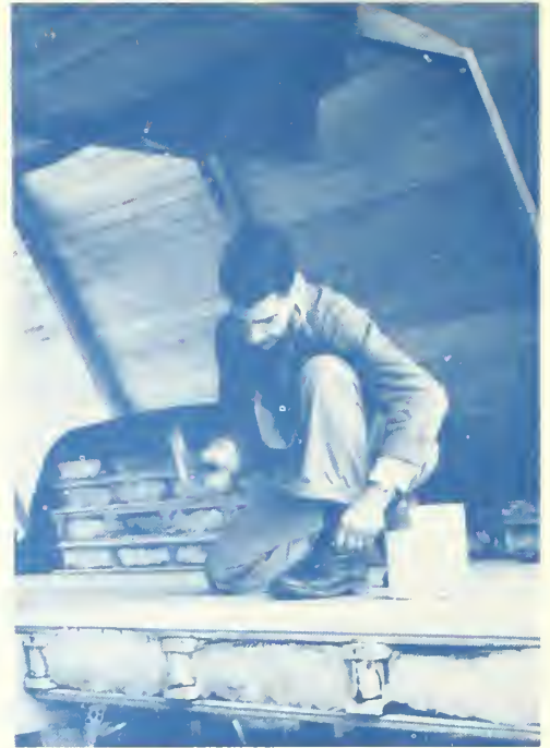
Figure 4.—Combination units. Shows I-beam stiffeners and insulation in place. Visible face is solid red oak paneling.
