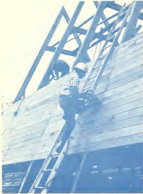
Figure 3.—Installing roof units on A-frame beams with a portable pneumatic nailer.
