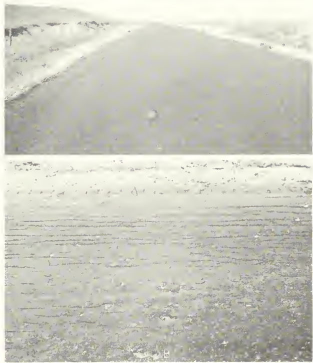
FIGURE 9.—ROAD-OIL SECTION AFTER ADDITION OF FINE SOIL FILLER. A, NOTE VEGETATION COVERING THE SHOULDERS AND SLOPES; B, CRACKING APPEARED IN THE OUTER WHEEL LANE, AND ROUGHNESS, DUSTING, AND POT-HOLING DEVELOPED.
