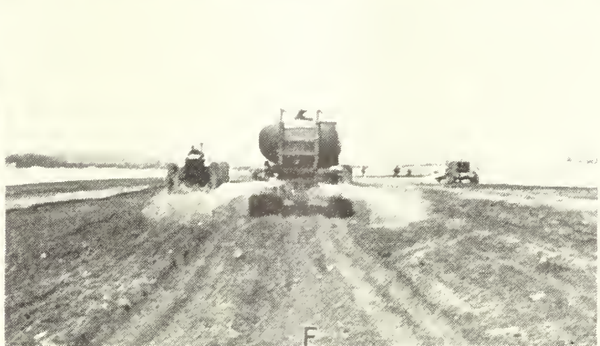
FIGURE 9.—STABILIZATION OF RUNWAYS: A, LOADING BINDER SOIL IN 2-CUBIC YARD BOXES; B, DEPOSITING AND SPREADING BINDER SOIL; C, CUTTING IN BINDER SOIL WITH FIELD CULTIVATOR; D, MIXING WITH TWO-WAY TANDEM DISK HARROW; E, TURNING DISKED MATERIAL WITH FOUR-BOTTOM GANG PLOW; AND F, SPRINKLING DURING MIXING OPERATIONS.
