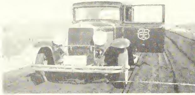
FIGURE 7. THE ROAD-OIL SECTIONS REMAINED IN A LOOSE CONDITION EXCEPT IN COLD WEATHER. AFTER FINE SOIL FILLER WAS ADDED THE MIXTURE COMPACTED AND BECAME STABLE.
