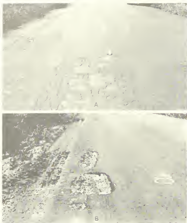
FIGURE 10. PLACES WHERE SURFACE FAILURE OCCURRED. A, THE RECTANGULAR PORTION IN THE CENTER WAS REMIXED AND TAMPED BY HAND; SHINY AREAS ARE POOLS OF BITUMEN. B, BREAK-UP CAUSED BY UNTREATED SAND LYING BETWEEN UPPER AND LOWER PORTIONS OF THE MAT.
