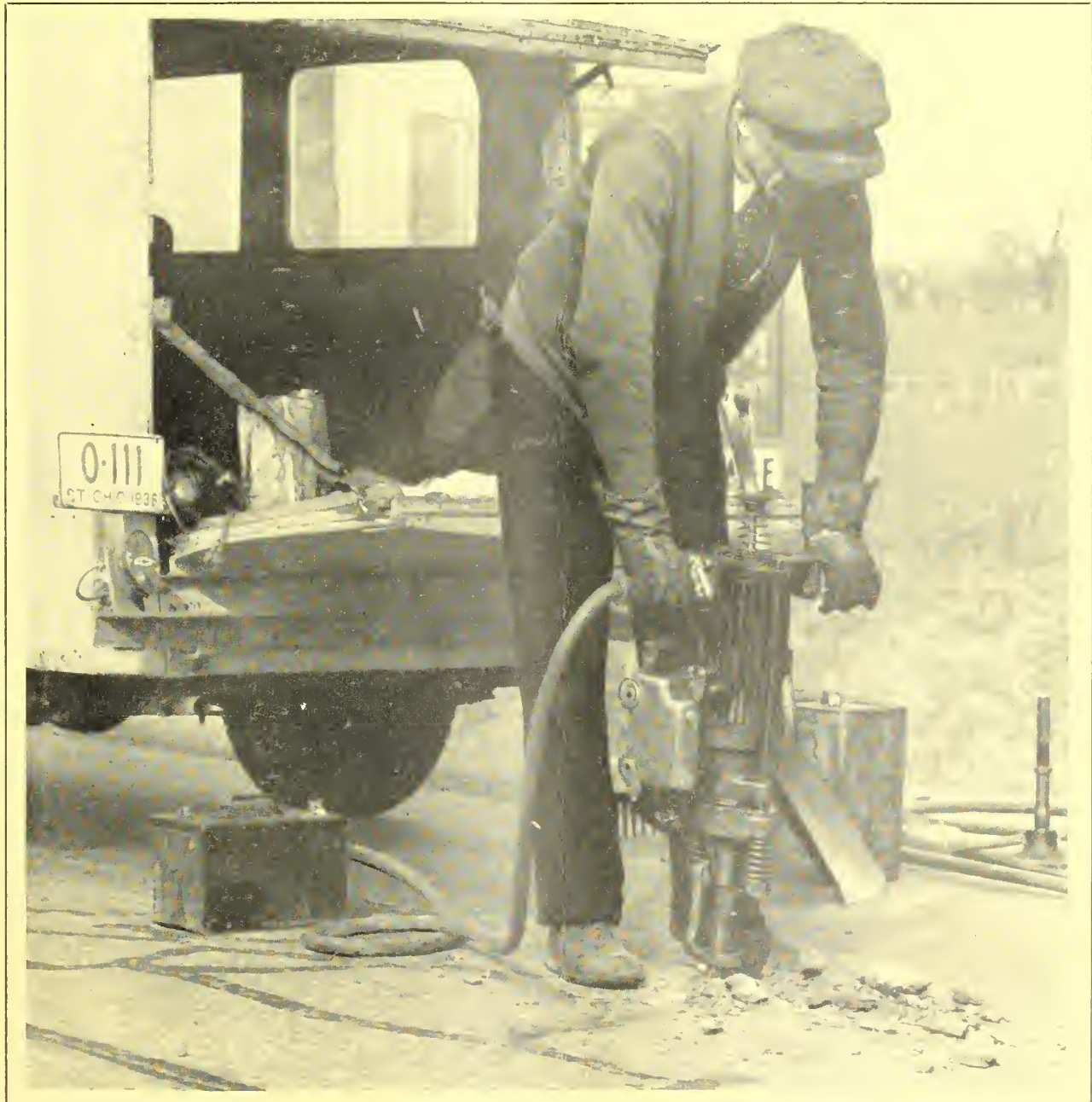
CUTTING A SAMPLE OF ASPHALTIC CONCRETE PAVEMENT IN OHIO
