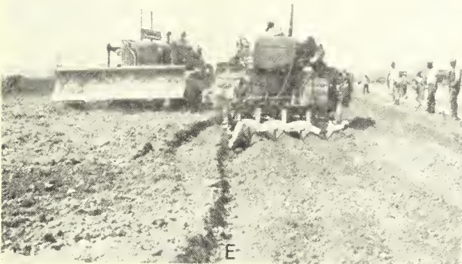
FIGURE 9.—STABILIZATION OF RUNWAYS: A, LOADING BINDER SOIL IN 2-CUBIC YARD BOXES; B, DEPOSITING AND SPREADING BINDER SOIL; C, CUTTING IN BINDER SOIL WITH FIELD CULTIVATOR; D, MIXING WITH TWO-WAY TANDEM DISK HARROW; E, TURNING DISKED MATERIAL WITH FOUR-BOTTOM GANG PLOW; AND F, SPRINKLING DURING MIXING OPERATIONS.
