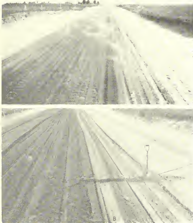
FIGURE 5.—A, SAND DRIFTING ACROSS A CUT-BACK SECTION. THE WIND WAS BLOWING TOWARD THE CAMERA AND AT A SLIGHT ANGLE TO THE CENTERLINE OF THE ROAD. B, DRIFTED SAND ON A LOOSE, ROAD-OIL SECTION. THE SPADE MARKS THE RIGHT EDGE OF THE BITUMINOUS MAT.
