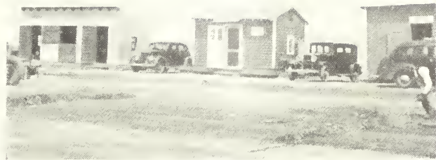
FIGURE 7.—PORTABLE LABORATORY (CENTER) AND OFFICES ON RUNWAYS.
